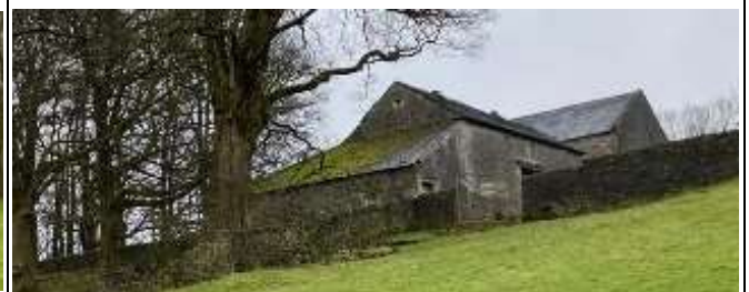
Looking South Towards Proposed New Access Point
