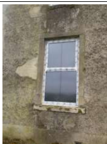
Ground Floor Window, West End of Elevation
