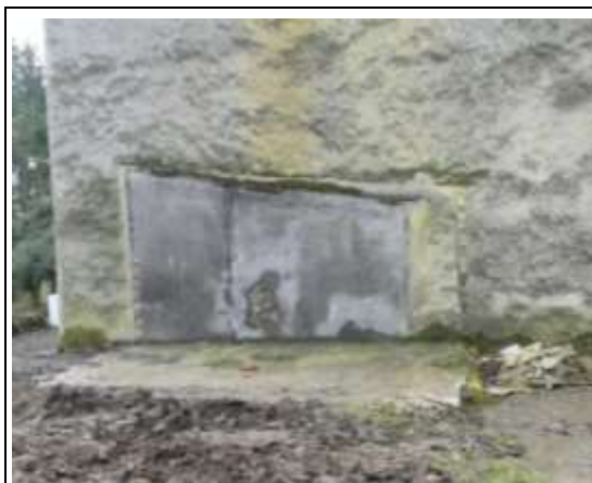
Former Extension with Hardstanding
