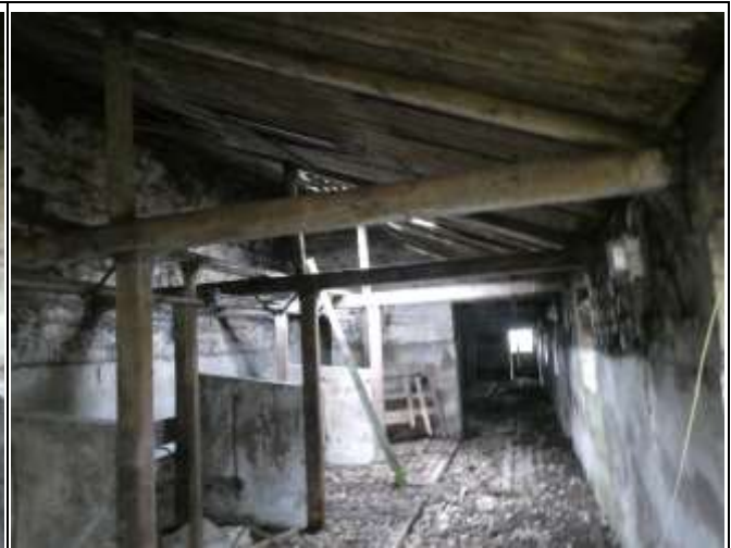
Timber Roof Structure
