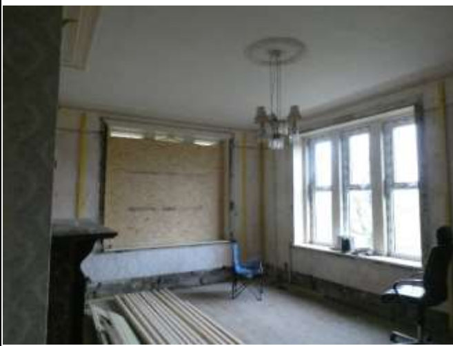
Windows at the Northwest Corner
