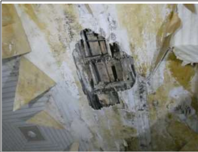
Exposed Ceiling Timber Slats
