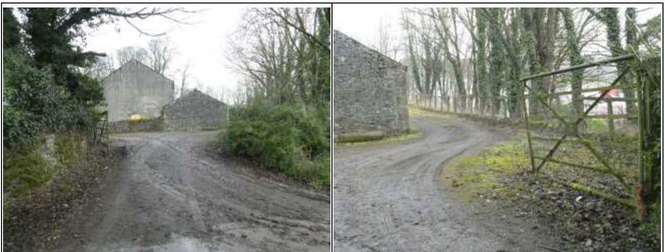
Existing Entrance into the Site off the Shared Road, Fencing to the Boundary at the South
