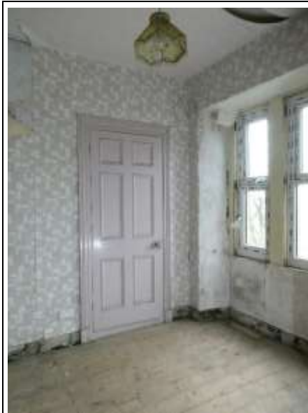
Cupboard Door and Replacement Window at the North
