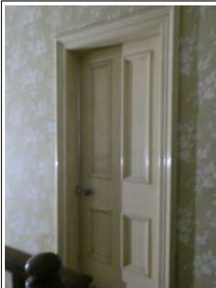
Panelled Door at Hall 4
