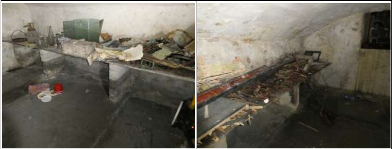
Stone Shelf and Brick Base at the North Wall
