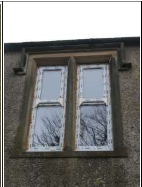
Double First Floor Window with Replacement Window Frames
