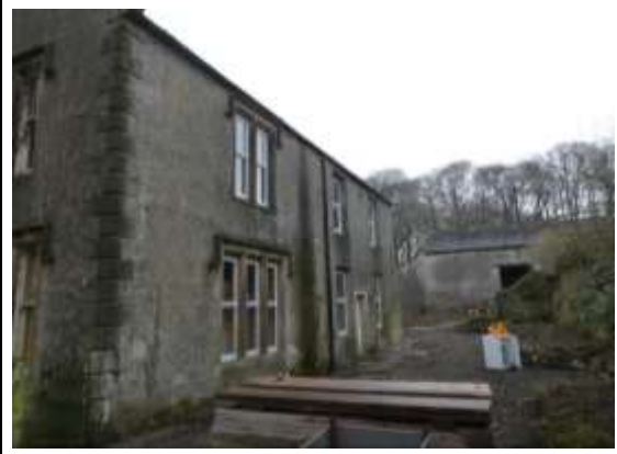
Looking Towards the Grade II Listed Barn
