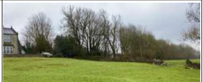
Looking Southwest, Partially Collapsed Stone Walling
