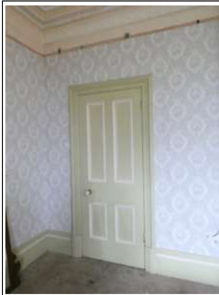
Painted Panelled Door Leading to Hall 1
