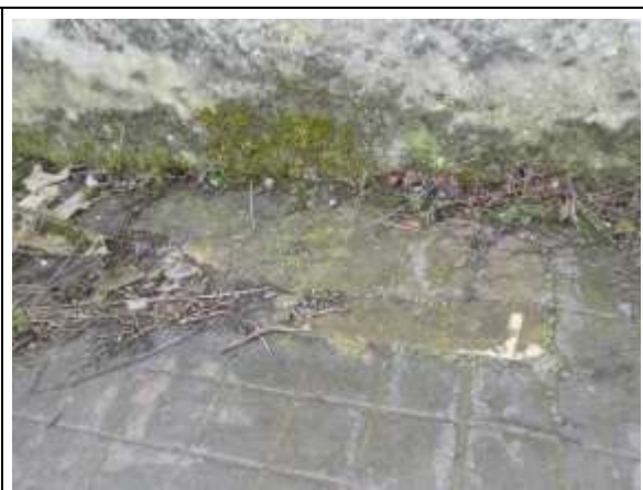
Former Basement Opening
