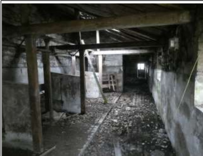
Former Cow Stalls at the Outshut
