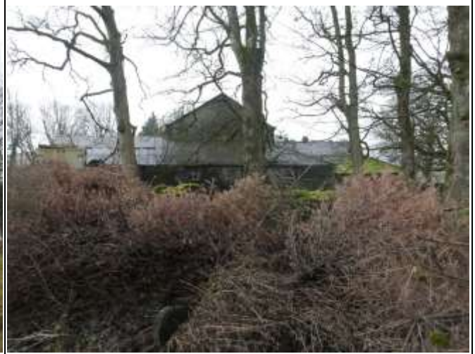
Looking North Towards Outshut and Outbuilding
