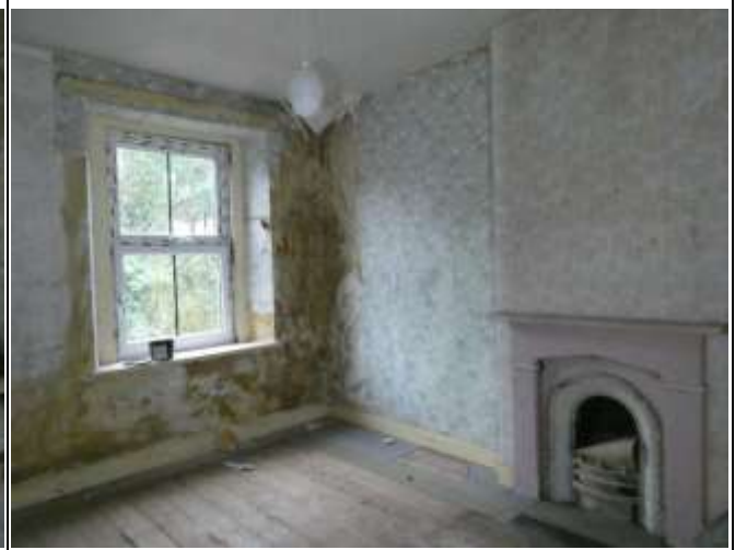
Replacement Window to the South
