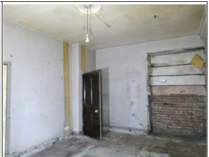
Painted Panelled Door Leading to the Scullery
