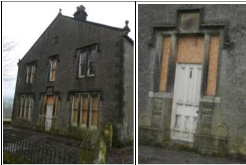
Painted Timber Door and Dressed Stone Surround, with Stained Glass Windows (Boarded Up)
