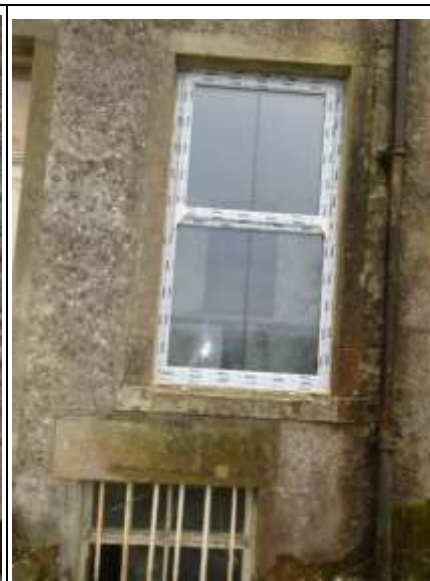
Adjacent Ground Floor Window, Basement Timber Framed Window with Painted Metal Window Bars and Stone Lintel.
