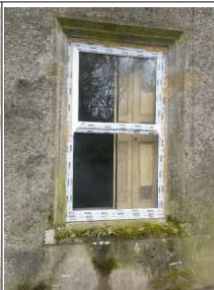
Window to the East of the Door with Shutters
