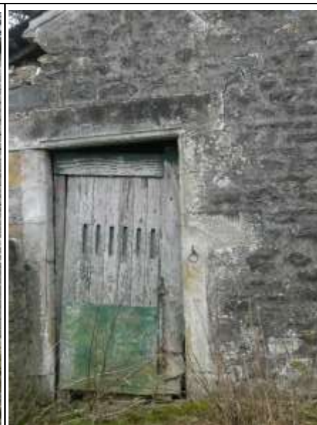
Stone Architrave and Timber Door
