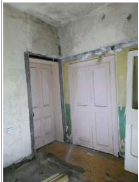
Built-in Cupboard at North Wall
