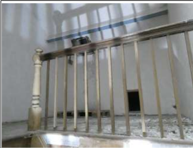
Looking Towards Void 2
