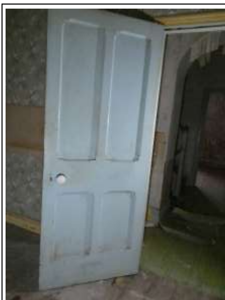
Painted Panelled Door
