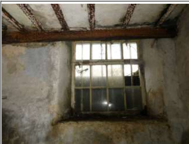
Timber Framed Window, Ironwork at the Ceiling
