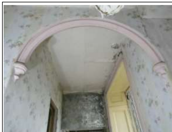
Archway Architrave at Hall 2 into Vestibule
