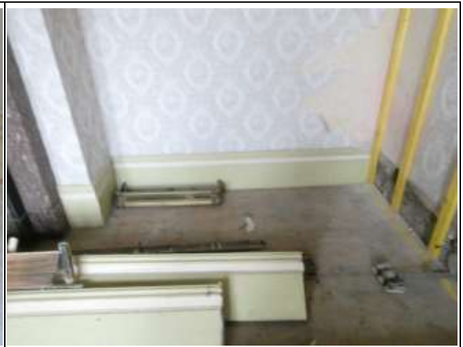
High Skirting Board in Situ
