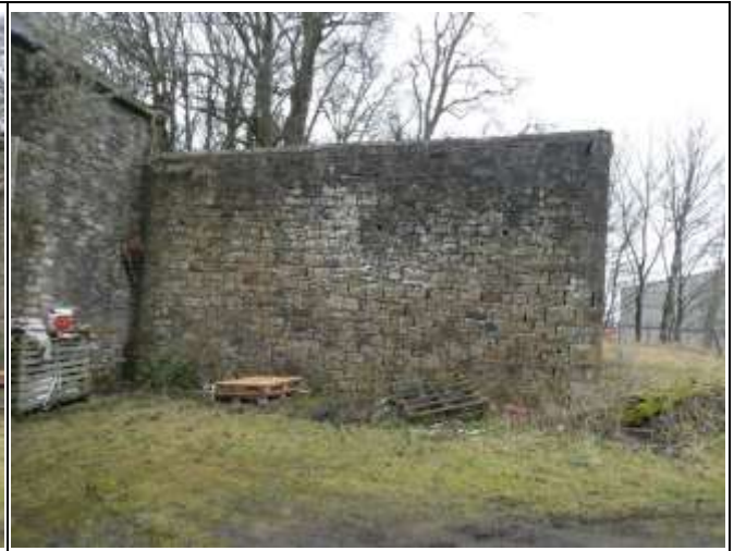
West Elevation of Outshut
