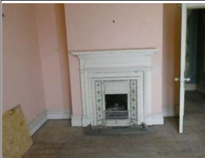
Cast Iron Surround at Fireplace
