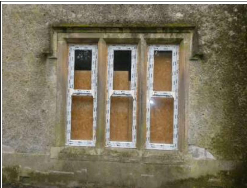
Triple Ground Floor Window with Dressed Stone Surround and Hoodmould and Replacement Window Frames
