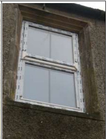
Window at the First Floor
