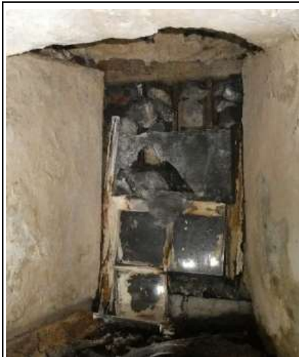
Small Blocked-up Opening at the East Elevation
