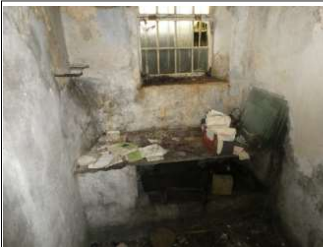
Looking North, Timber Framed Window, Iron Bracket at Wall
