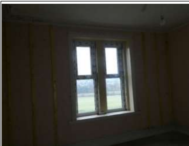
Replacement Window to the North
