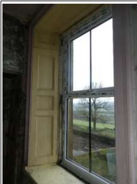
Replacement Window with Traditional Shutters and Architrave
