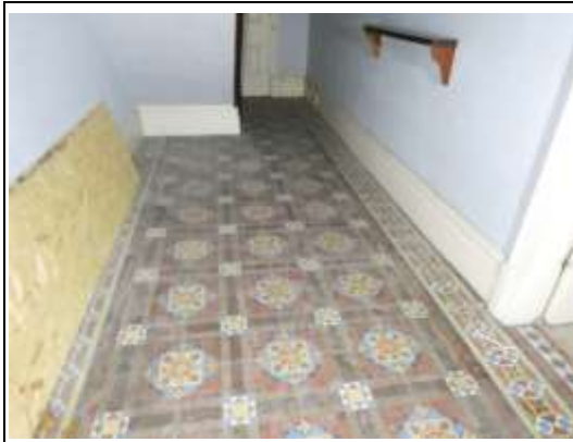
Tiled Flooring Under Stairs
