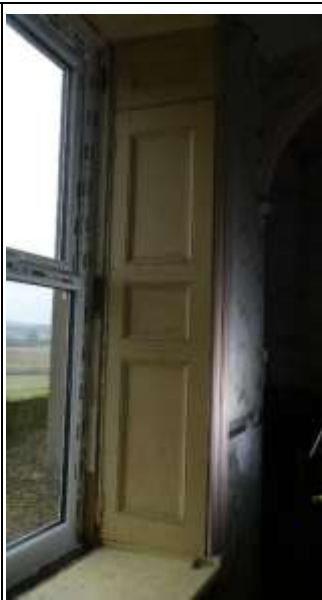
Replacement Window with Traditional Shutters and Architrave
