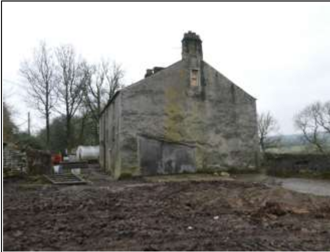
Cleared Area to the East of the Farmhouse
