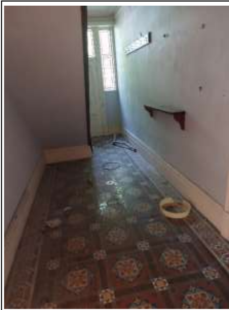
Hall 1, Front Entrance
