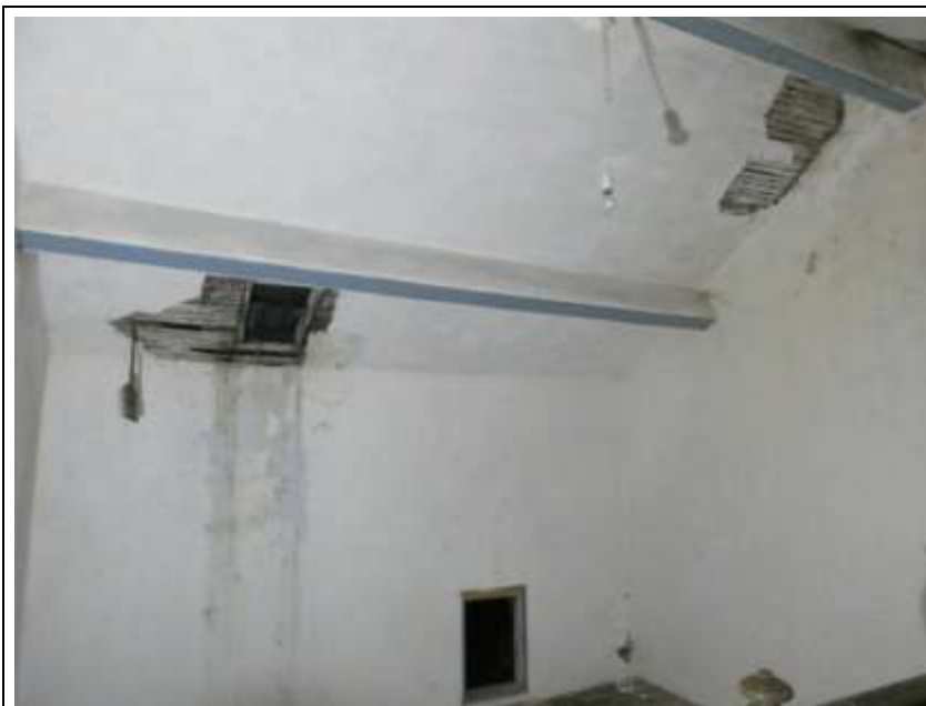
Painted Beam, Early Roof Light and Access Point
