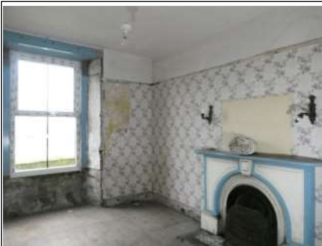
Replacement Window at the North Elevation
