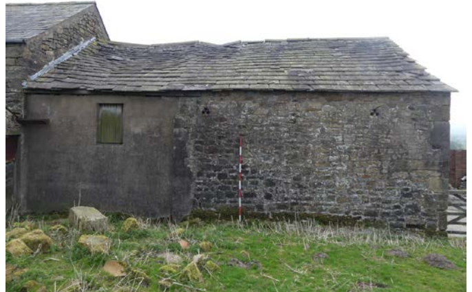
Plate 22 (left): Blocked window on the south-west side of the lower extension to the north-west external elevation of the barn, viewed from the north-west
