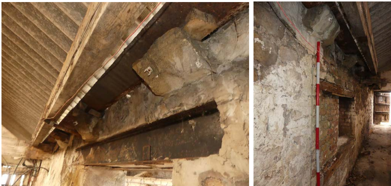
Plate 66 (left): Corbels supporting the gutter along the south-east side of Room G2 of the barn, viewed from the west
