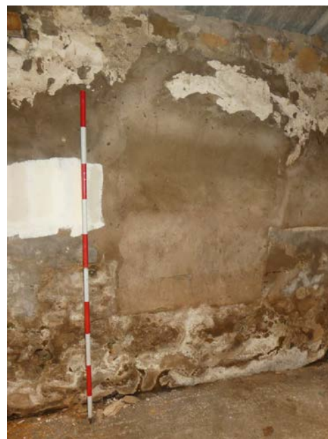
Plate 74 (left): Blocked window, south-west side of the north-west elevation, Room G2 of the barn, viewed from the south-east
