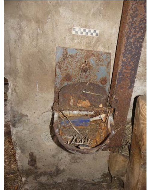
Plate 78 (left): Concrete division and hay rack on extending across the centre of the north-west side of Room G3 of the barn, viewed from the east
