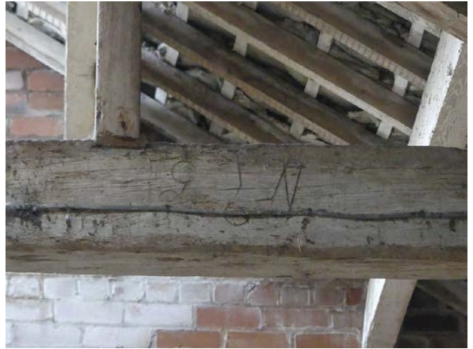
Plate 91 (left): Baltic marks on the north-east face of the north-east tie beam, Room F2 of the barn, viewed from the north-east
