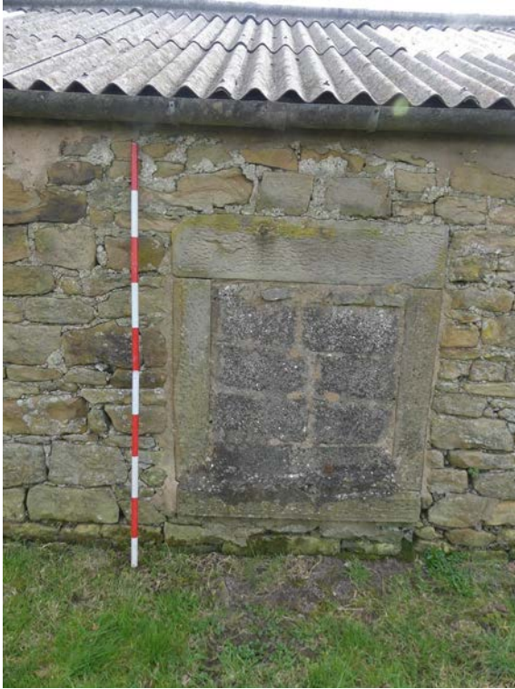
Plate 20 (left): Blocked window on the north-east side of the lower extension to the north-west external elevation of the barn, viewed from the north-west
