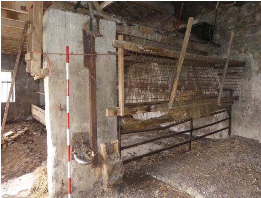
Plate 78 (left): Concrete division and hay rack on extending across the centre of the north-west side of Room G3 of the barn, viewed from the east
