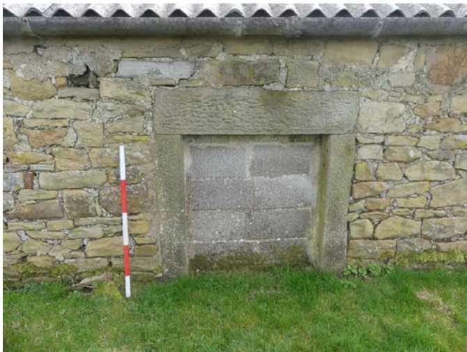
Plate 22 (left): Blocked window on the south-west side of the lower extension to the north-west external elevation of the barn, viewed from the north-west
