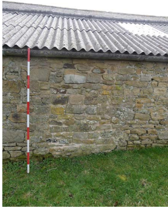
Plate 20 (left): Blocked window on the north-east side of the lower extension to the north-west external elevation of the barn, viewed from the north-west
