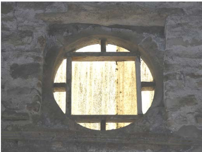
Plate 93 (left): Circular pitching window in the south-east elevation, Room F2 of the barn, viewed from the north-west
