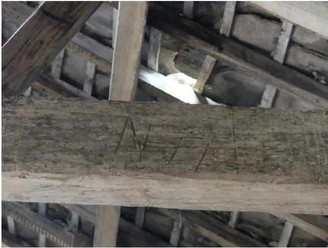
Plate 91 (left): Baltic marks on the north-east face of the north-east tie beam, Room F2 of the barn, viewed from the north-east
