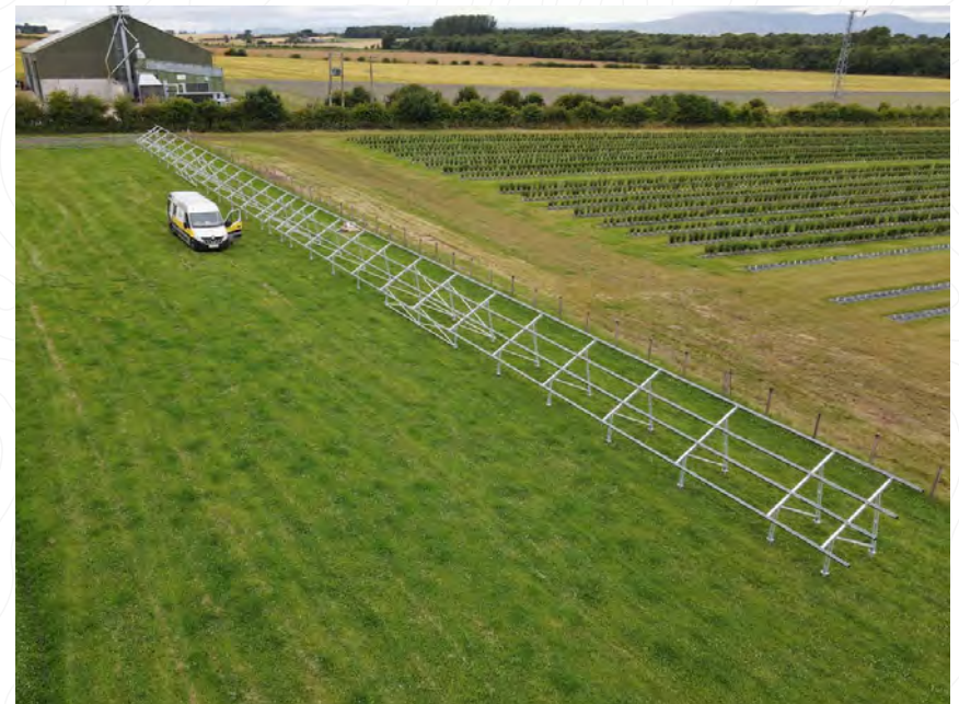
50kW Solar PV, screw piles and racking installed in three days
