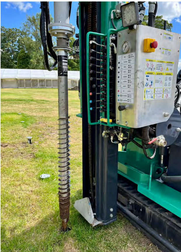
Removal of screw piles
