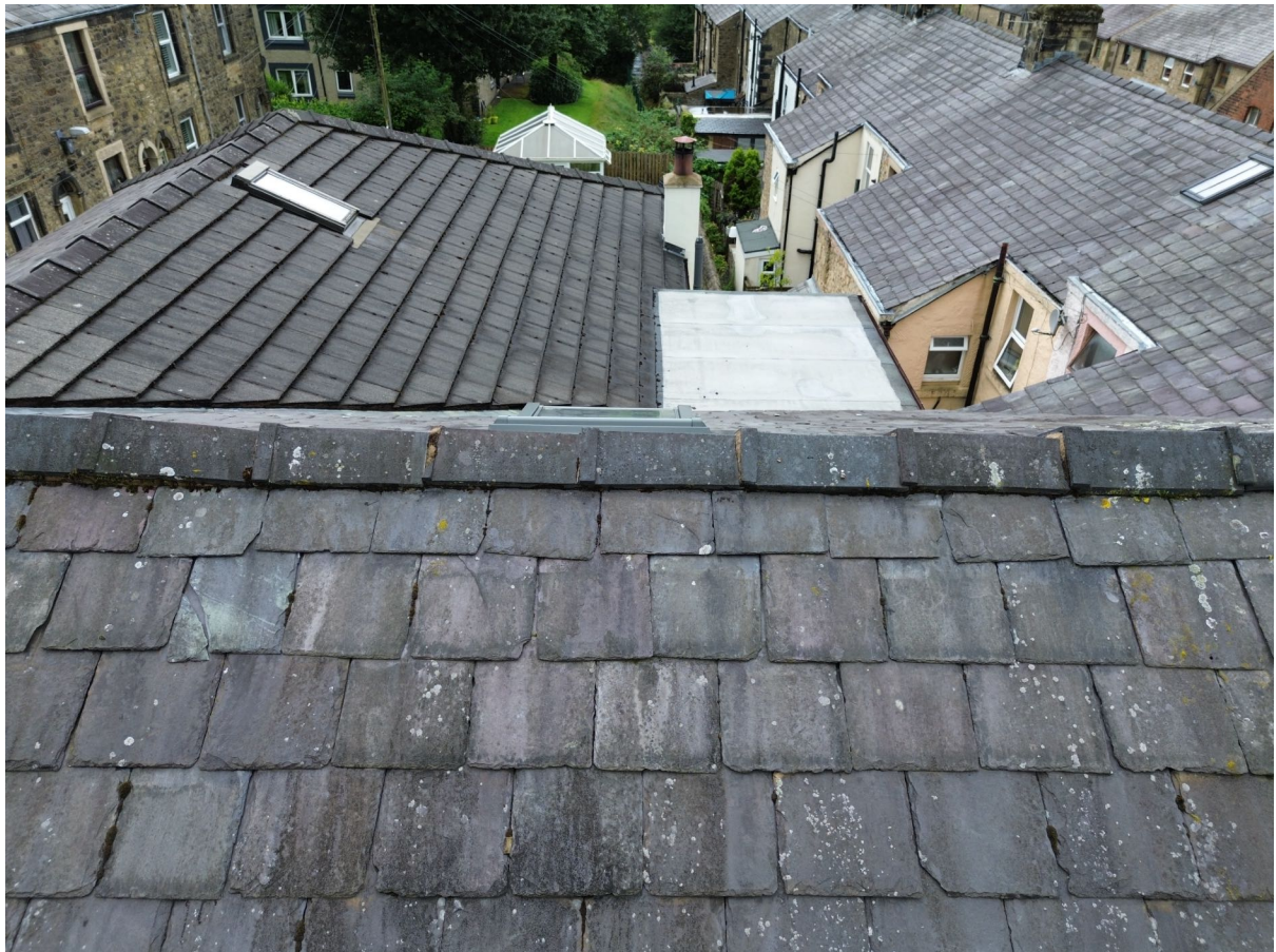
2 – Roof and ridge tiles are in good condition with no suitable gaps.
