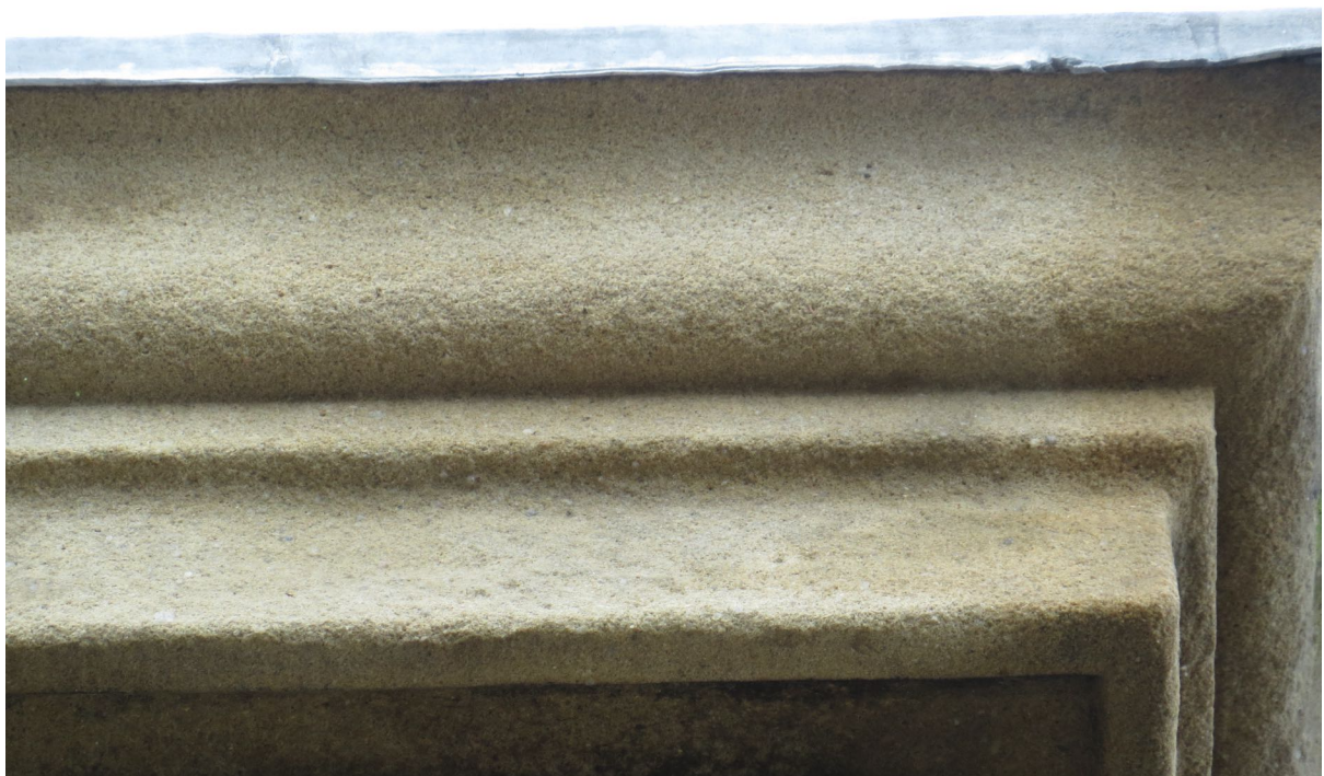
4 – Stonework and hidden gutters at the eaves are in good condition with no viable gaps.
