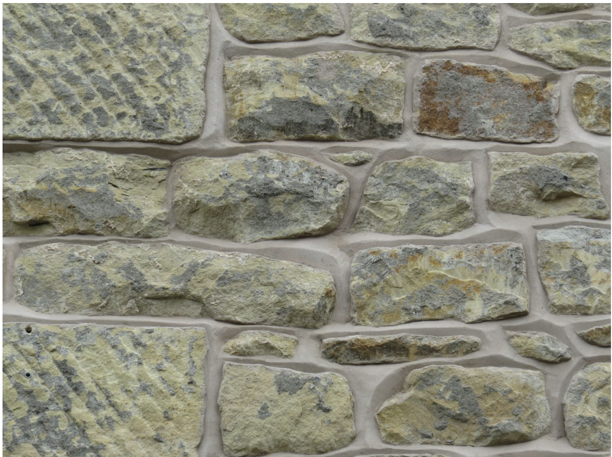
6 – Stonework and mortar are in good condition with no suitable gaps.
