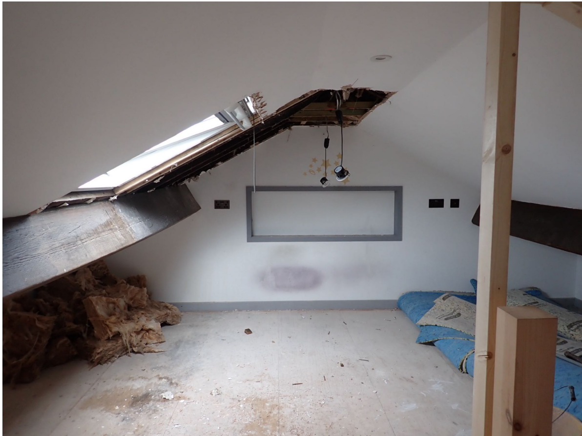
3.2a – The roof void.
