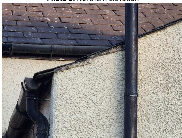
Photo 7: Gaps at roof verge at gable end
