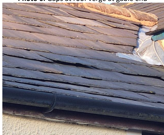
Photo 8: Lifted slates at west-facing roof pitch
