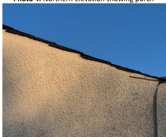
Photo 6: Gaps at roof verge at gable end
