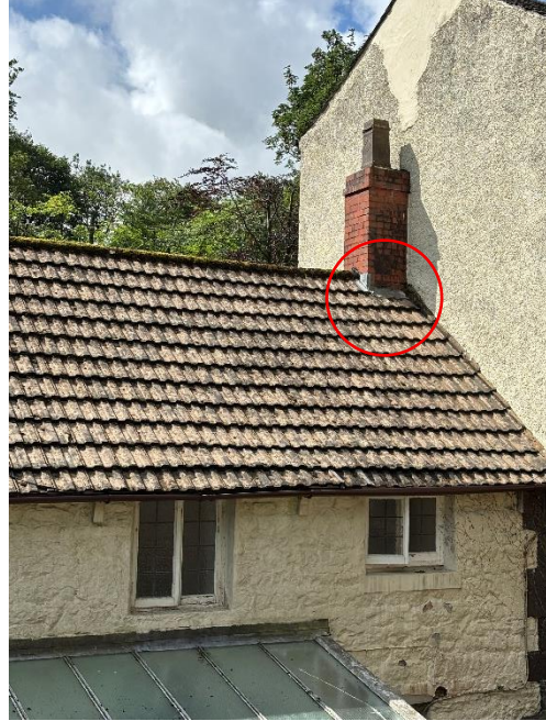
Photograph 2: Raised lead flashing around chimney on northern aspect.
