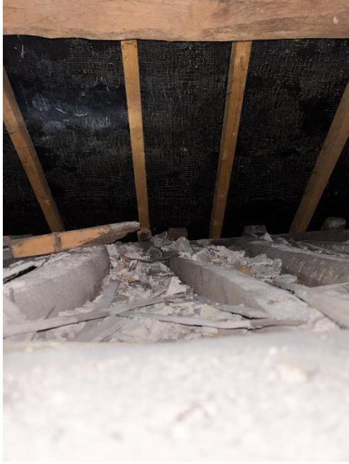
Photograph 9: Overview of the loft space.
