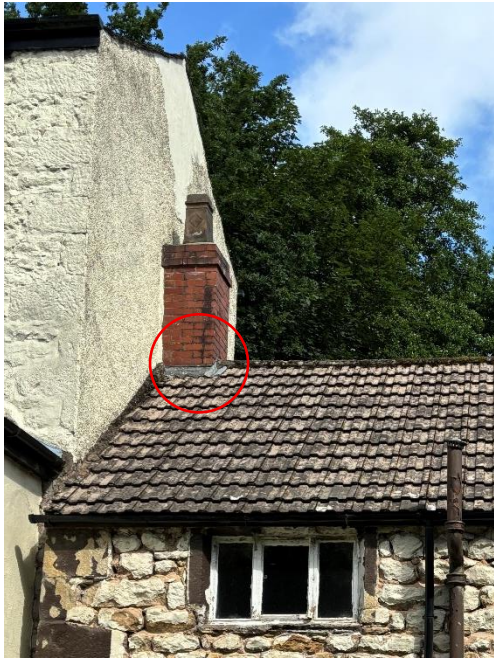
Photograph 5: Raised lead flashing around chimney on southern aspect.
