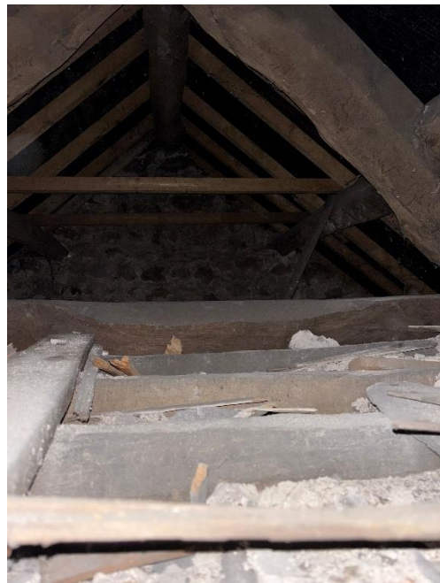
Photograph 8: Overview of timber beams and rafters in the loft space.
