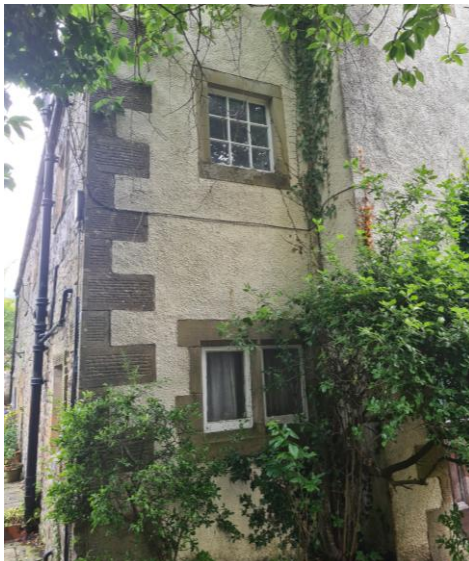
Side Southwest Elevation
