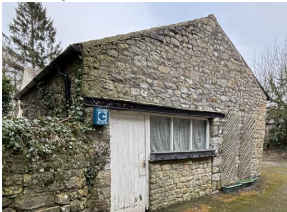
Southwest Elevation of Outbuilding
