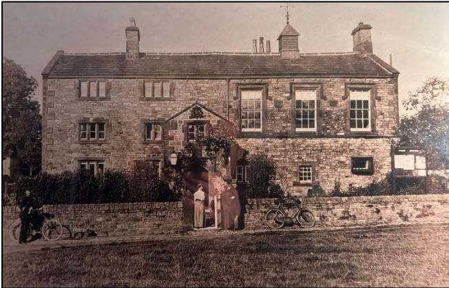
Fig 05: Image of an Historic Photograph of the Old Courthouse taken c. early 20 th century (image provided by client)
