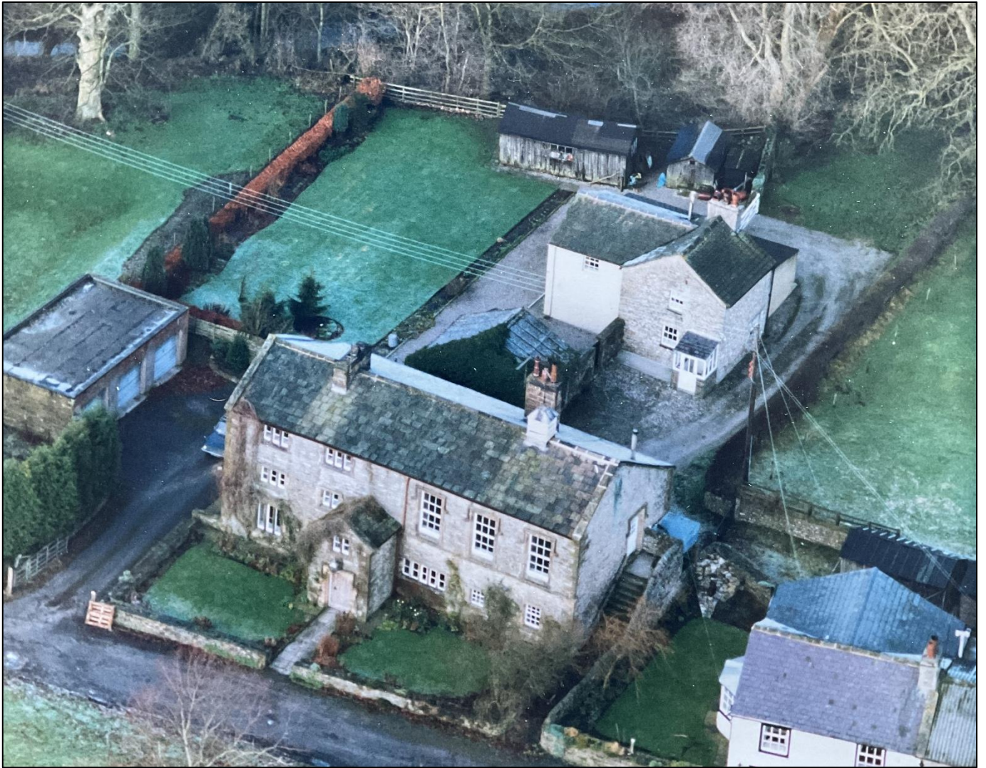
Fig 02: Aerial Photograph showing the Old Courthouse and the now demolished garage building located to the west.
