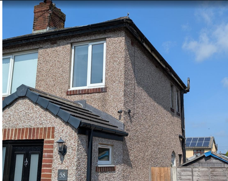
Photo 1. Front and side elevation (area of proposed extension).
