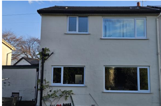
Rear Southwest Elevation
