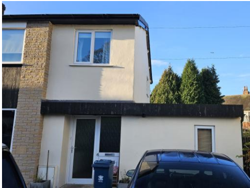
Part Front Northeast Elevation
