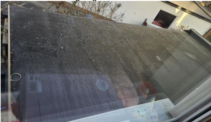
Flat roof from above
