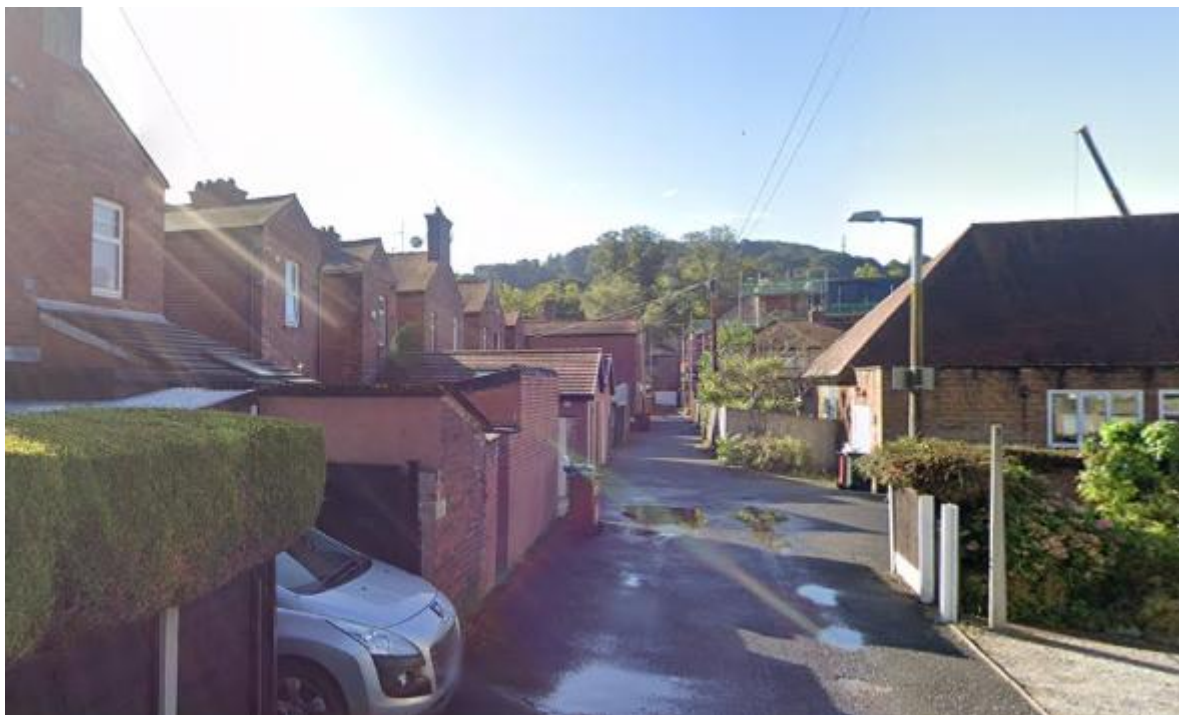
Figure 5. There is more modern development to the rear elevation of the site and many of the nearby properties have more modern rear extensions / outbuildings. The proposed extension would be seen within this context
