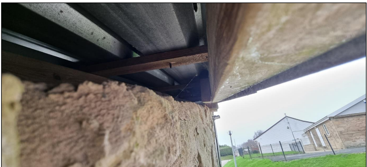
Plate 8: The gaps below the verges opened to the wall tops and offered potential access to internal voids.
