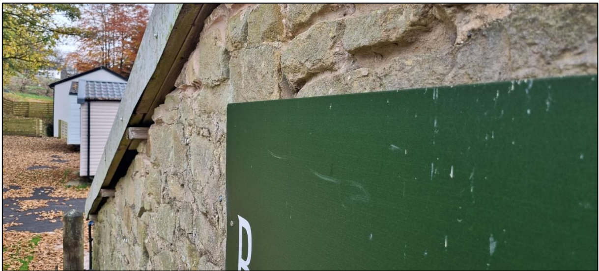
Plate 7: The dry verge capping was intact although there were significant gaps below the verges.
