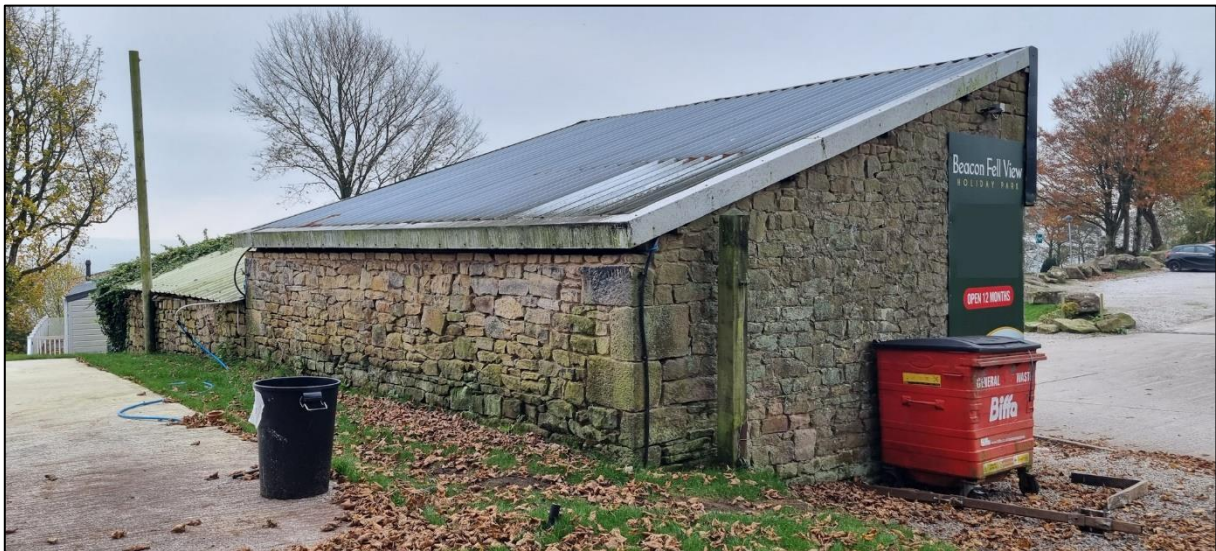
Plate 3: The pitched roofs of profiled sheets were intact and offered no roosting potential.
