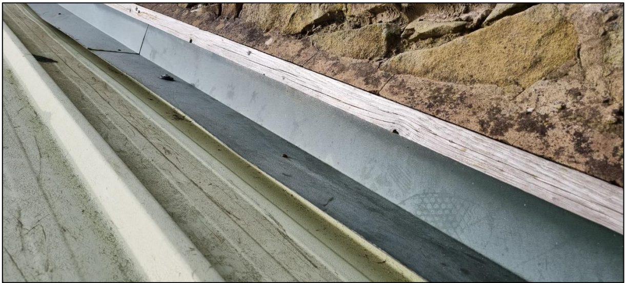
Plate 6: The apron along the lower roof was intact and offered no roosting potential.
