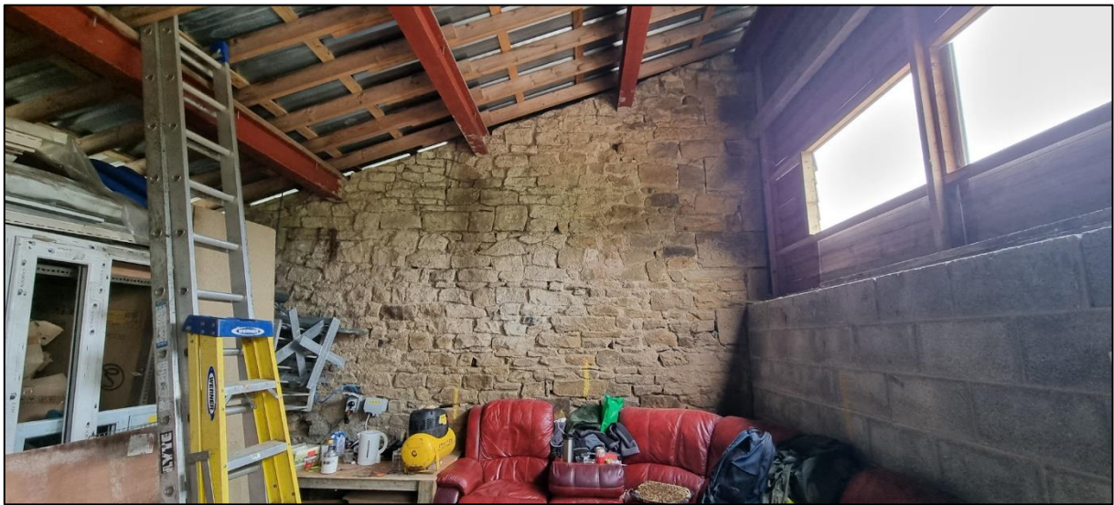
Plate 18: The largest of internal voids (Void 1) was open to the roofing sheets and support structures.
