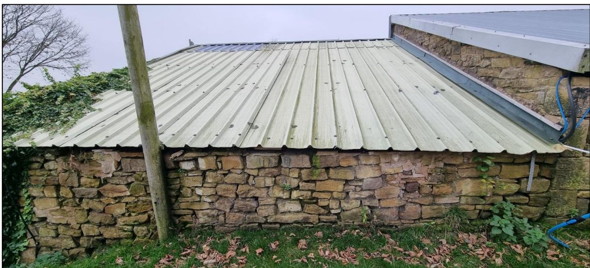
Plate 5: The lower pitch was intact with no roosting potential although gaps were noted beneath the sheet ends.
