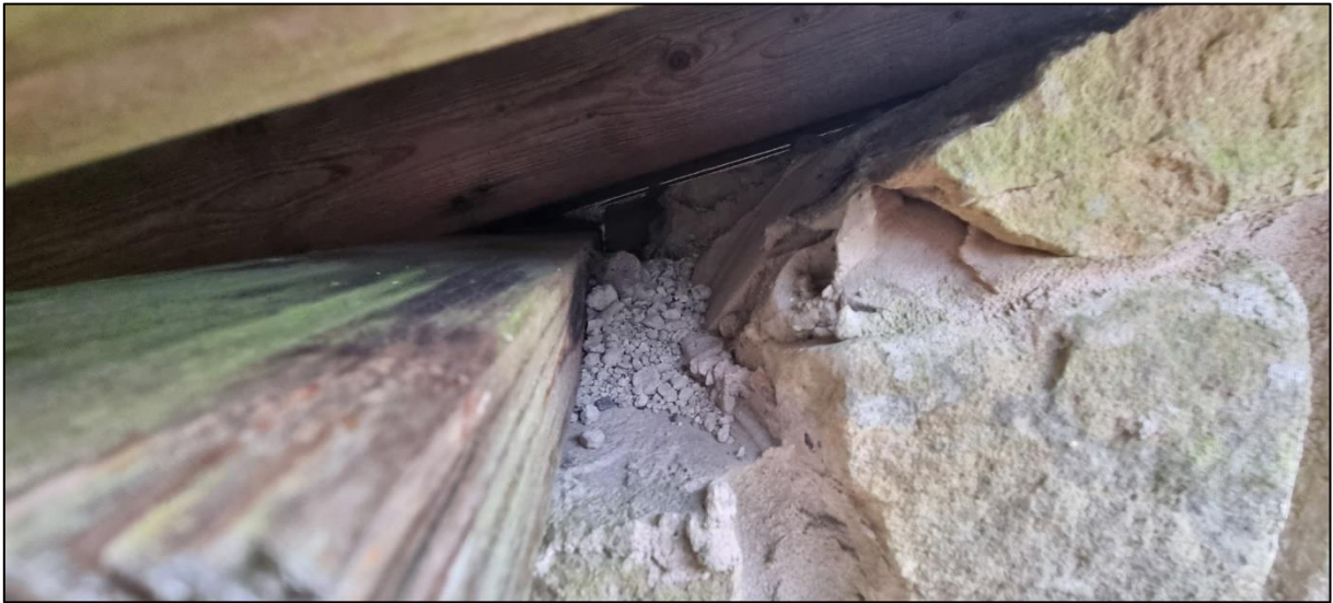
Plate 9: The gaps in the verges lead to the internal void and offered bats potential access to the wall interior.
