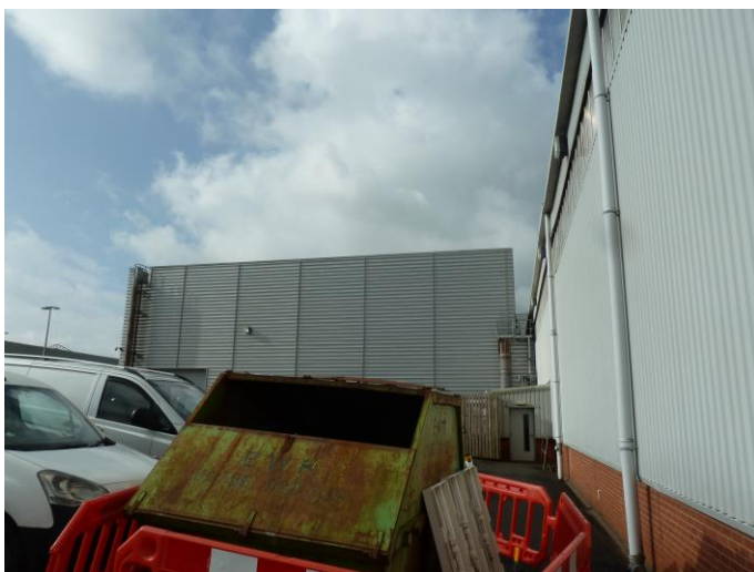
Photograph 10: S■■■■ general view of north-east elevation with S■■■■ on the right.
