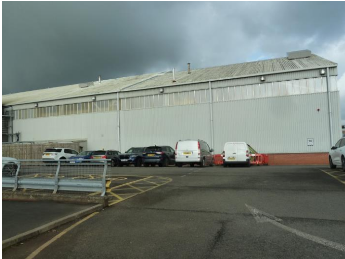
Photograph 8: S■■■■ – general view of the south-east elevation.
