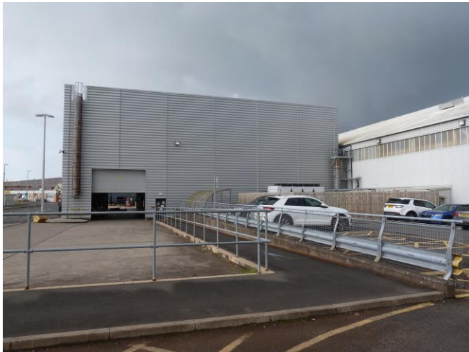
Photograph 1: Typical view of hardstanding and the north-east elevation of the ■■■■ Building.
