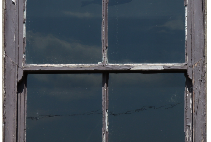
Photograph 4. Repairs to sash boxes.
