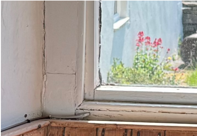
Photograph 3. Repair to sash box.
