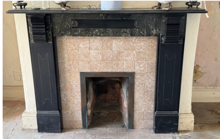
Photograph 24. A slate fireplace surround in the eastern ground floor room.
