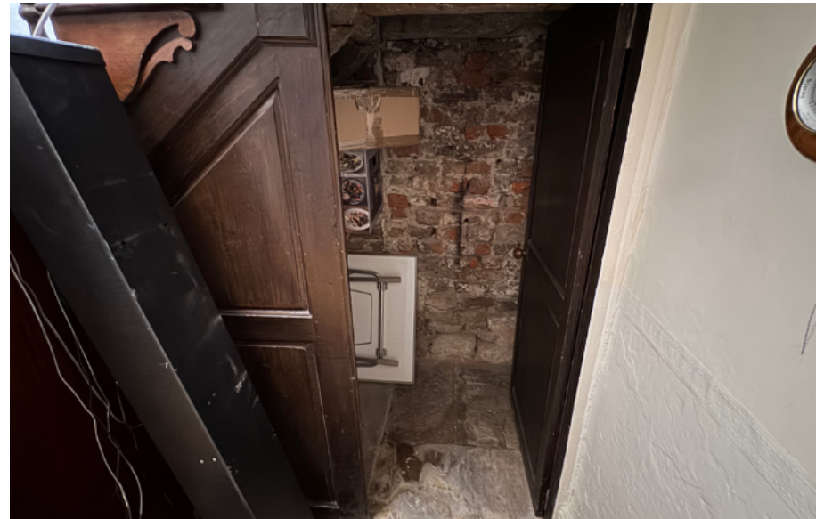
Photograph 20. The cupboard below the staircase.
