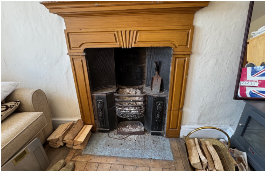
Photograph 31. The fireplace in the western bedroom.
