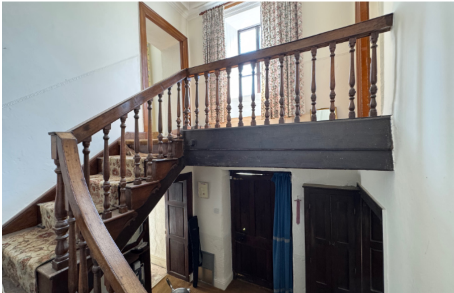
Photograph 27. The staircase and first-floor landing.
