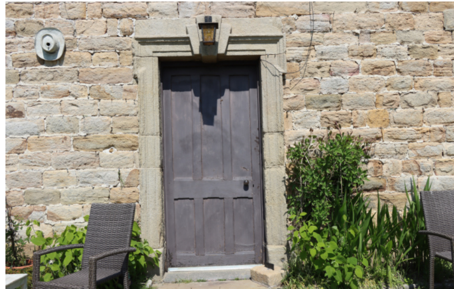
Photograph 4. The front door.
