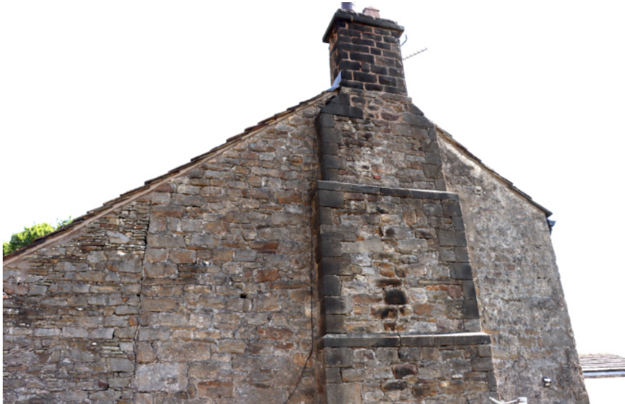
Photograph 7. The west gable wall.
