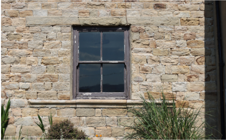
Photograph 5. The right-hand ground-floor window at the front.
