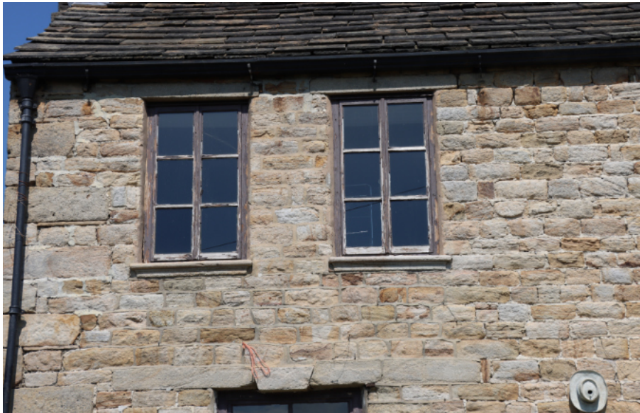
Photograph 3. The left-hand upper windows at the front.
