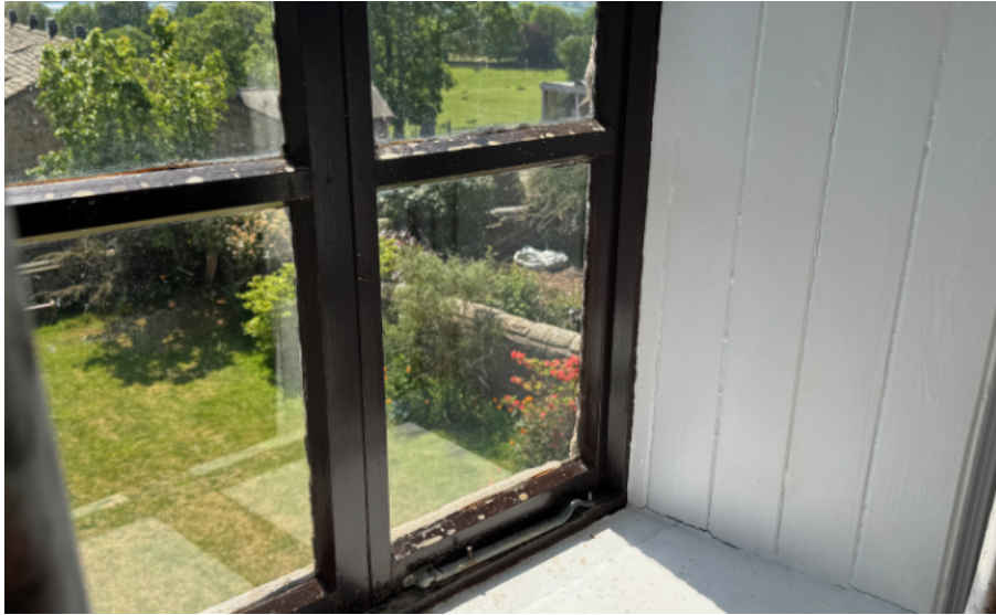
Photograph 29. A first-floor window at the front.
