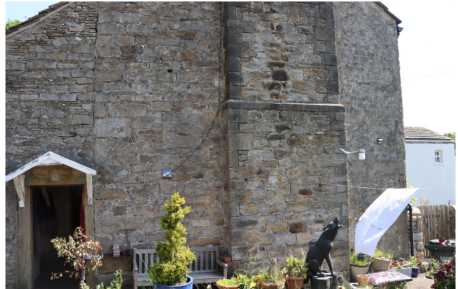
Photograph 8. The west gable wall.
