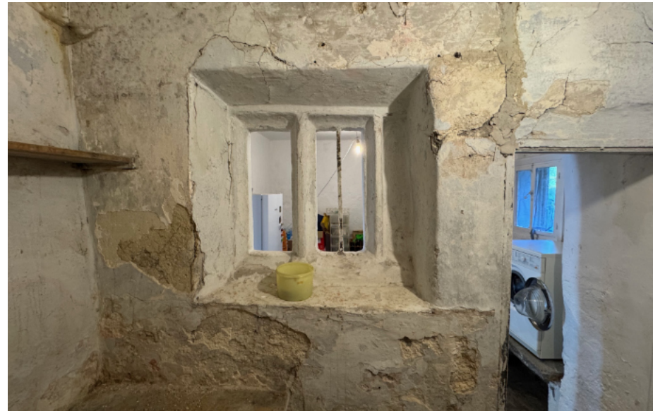
Photograph 16. Mullioned window within the ground-floor store.
