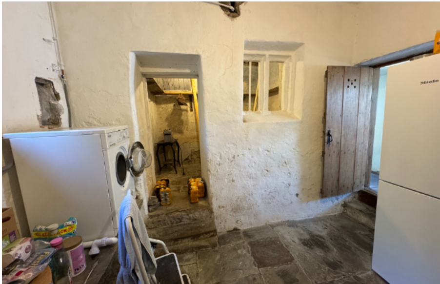
Photograph 15. The interior of the dairy /pantry.
