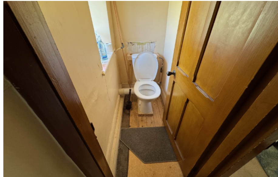
Photograph 36. The first floor WC.
