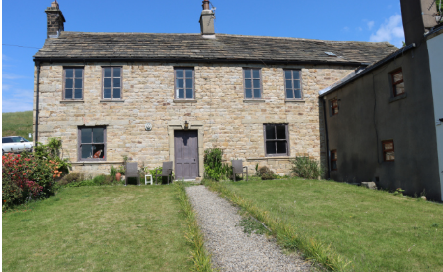
Photograph 1. The front elevation.
