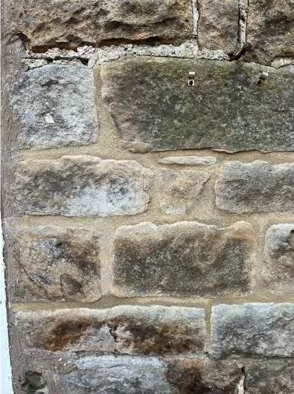
Sample images of re-pointing in lime
