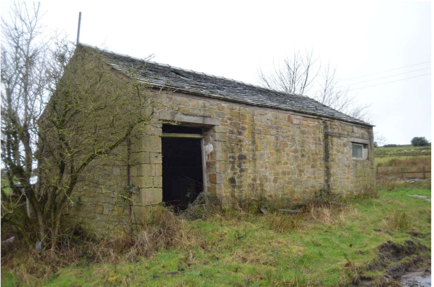
Fig 15 View of the stone outbuilding from the south east
