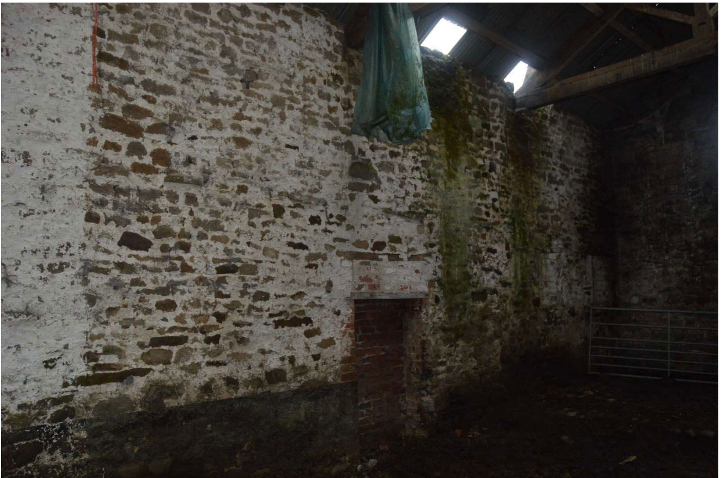
Fig 7 View south west within the barn core
