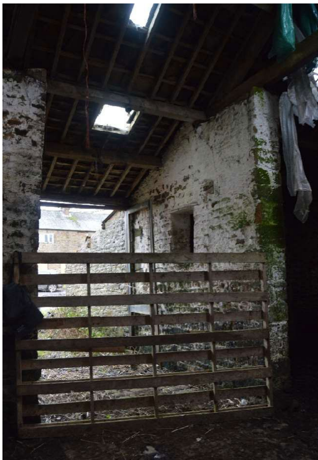
Fig 10 Internal view of the cart entry porch (north)
