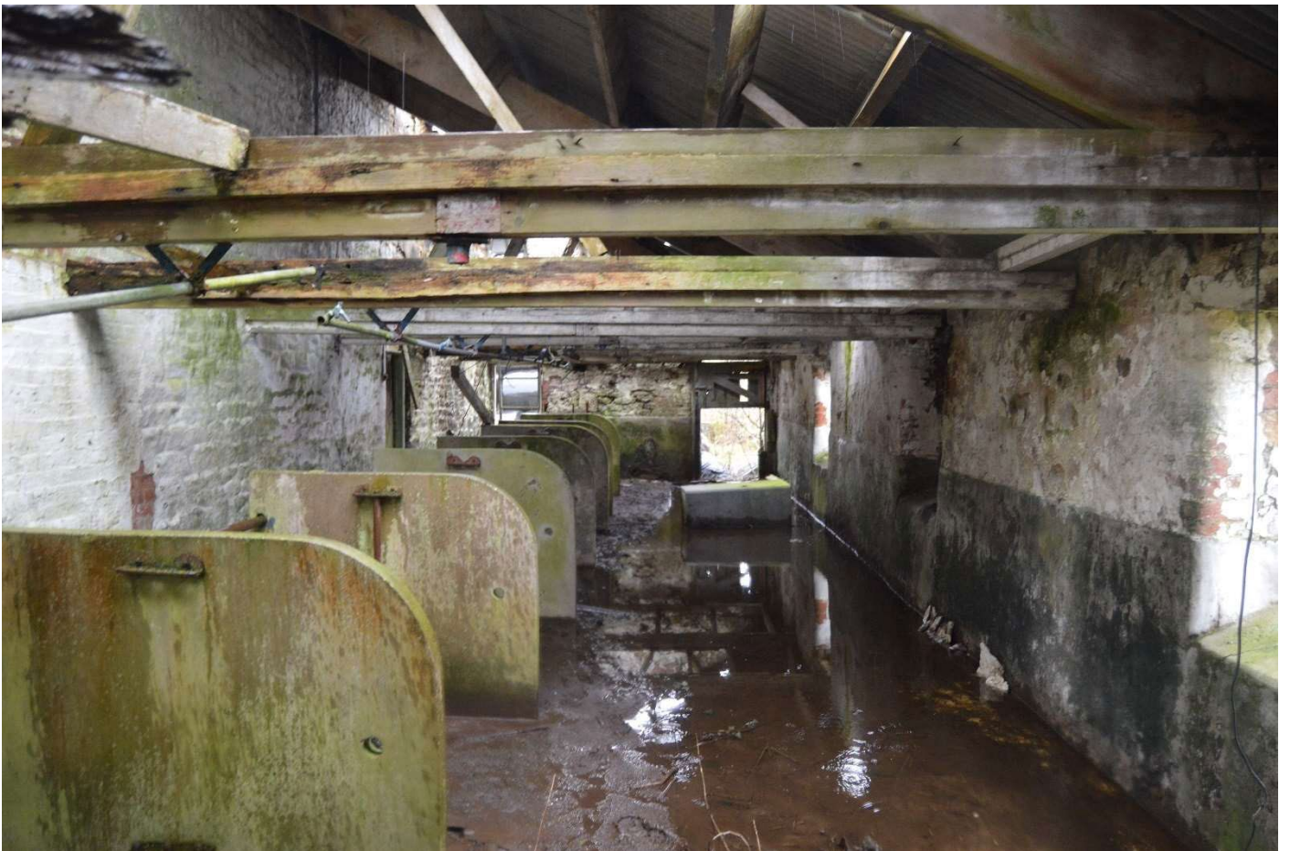
Fig 14 Internal view (east) within the south shippon
