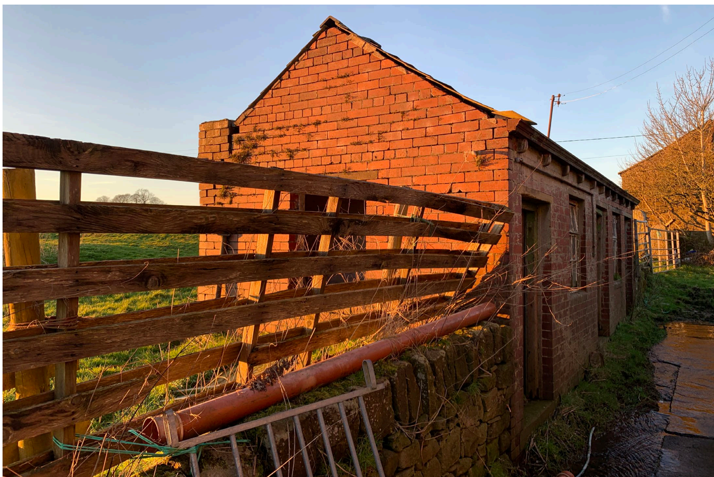
Fig 20 View of the brick outbuilding from the south
