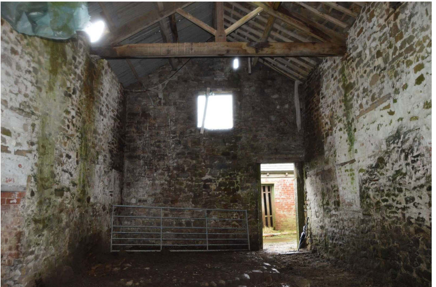
Fig 9 View west within the barn core
