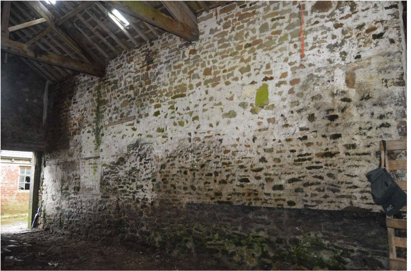
Fig 8 View north west within the barn core
