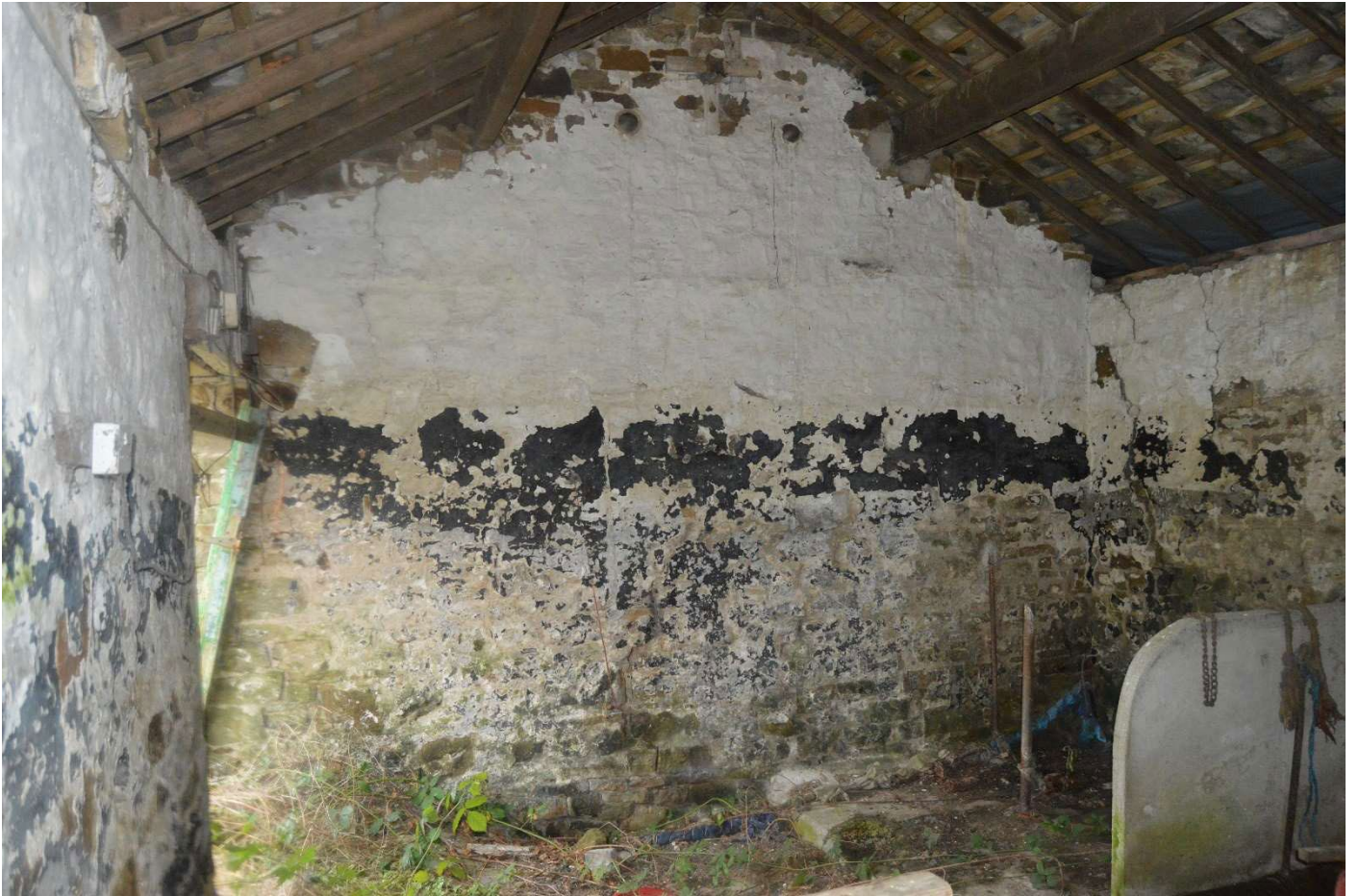
Fig 17 Internal view (south) of the stone outbuilding
