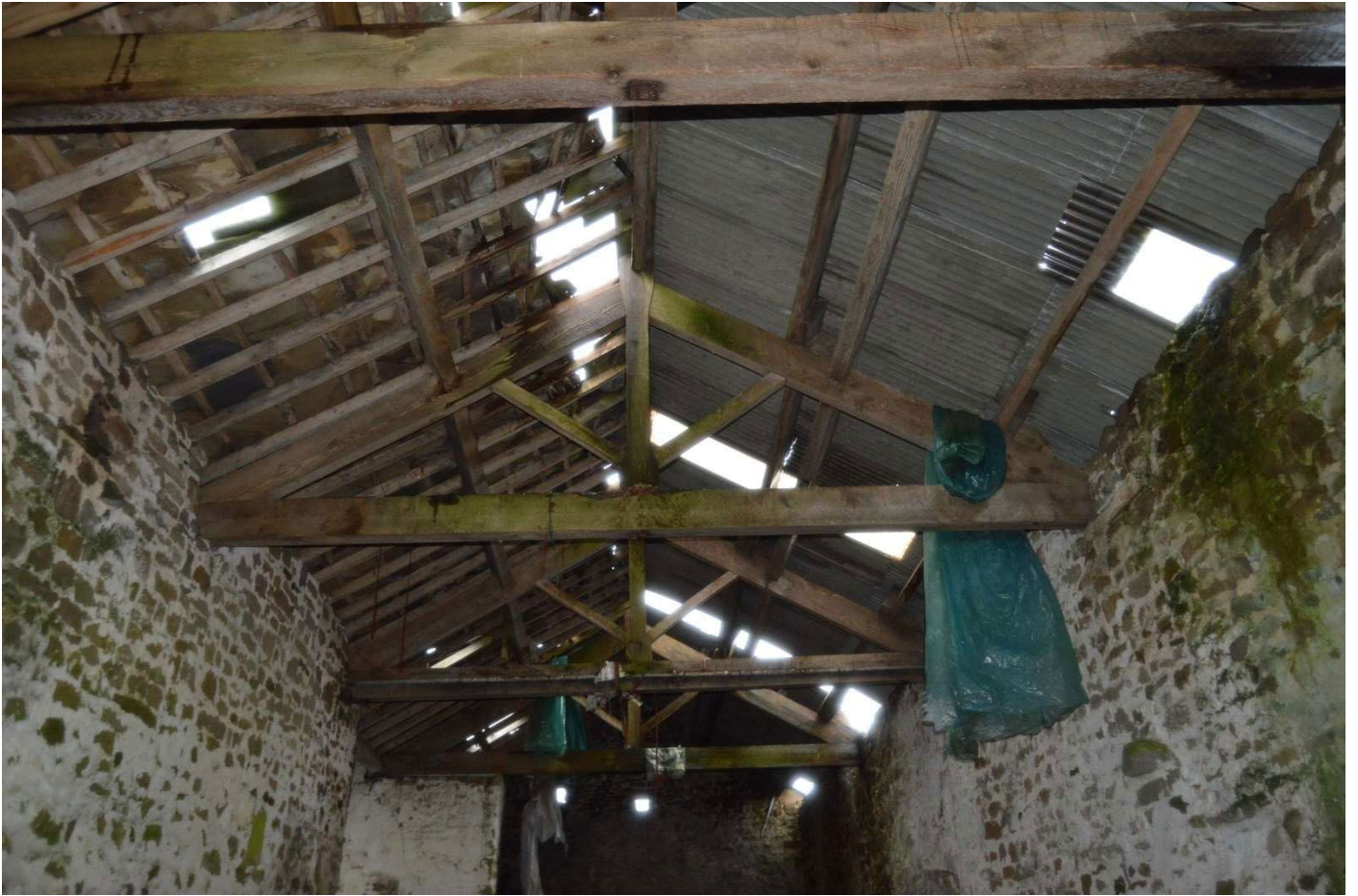
Fig 13 View of roof structure over the main barn core
