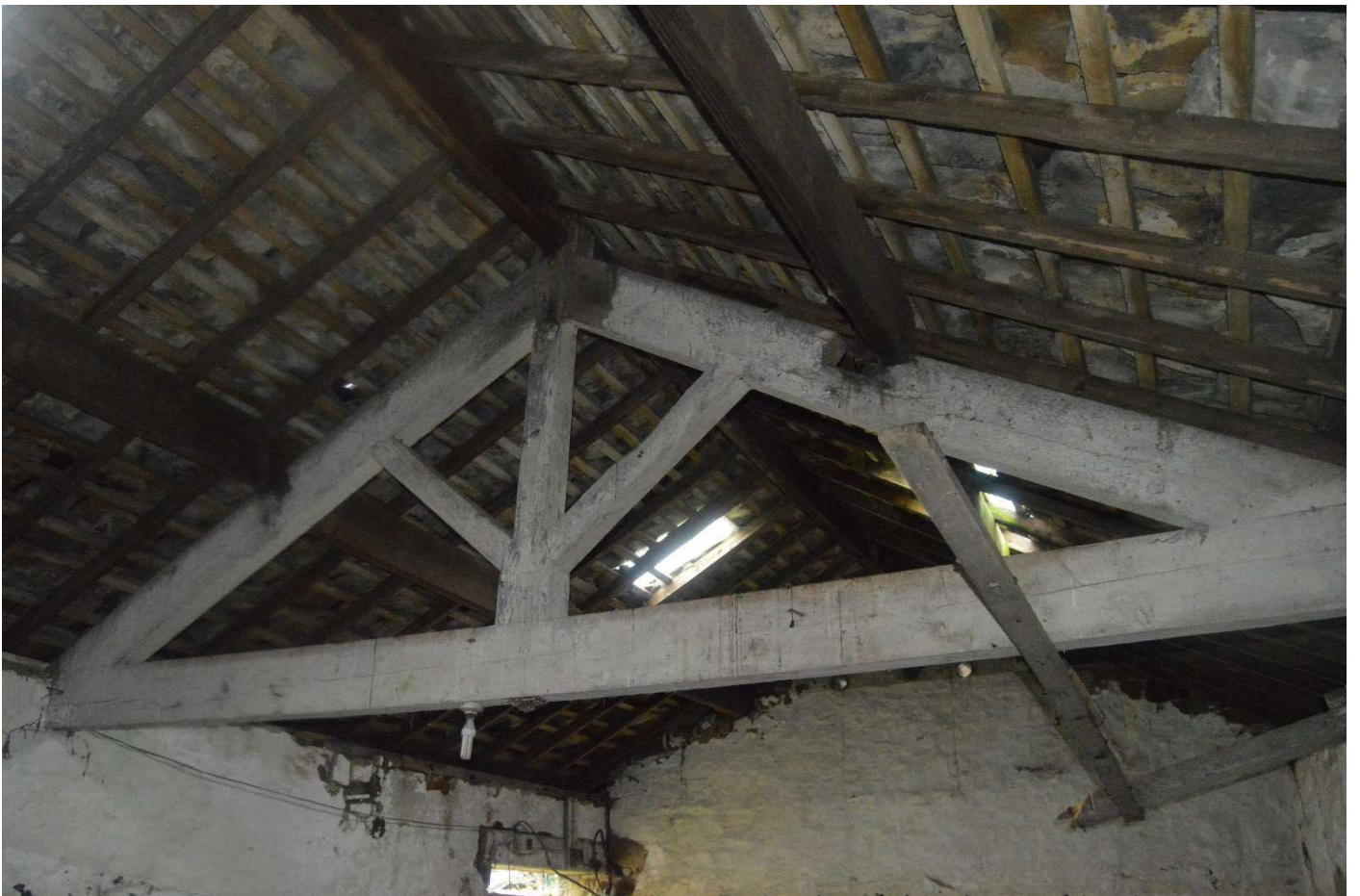
Fig 18 View of the roof structure to the stone outbuilding
