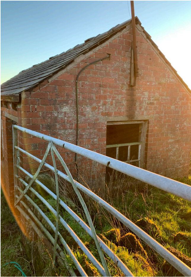
Fig 21 View of the brick outbuilding from the north
