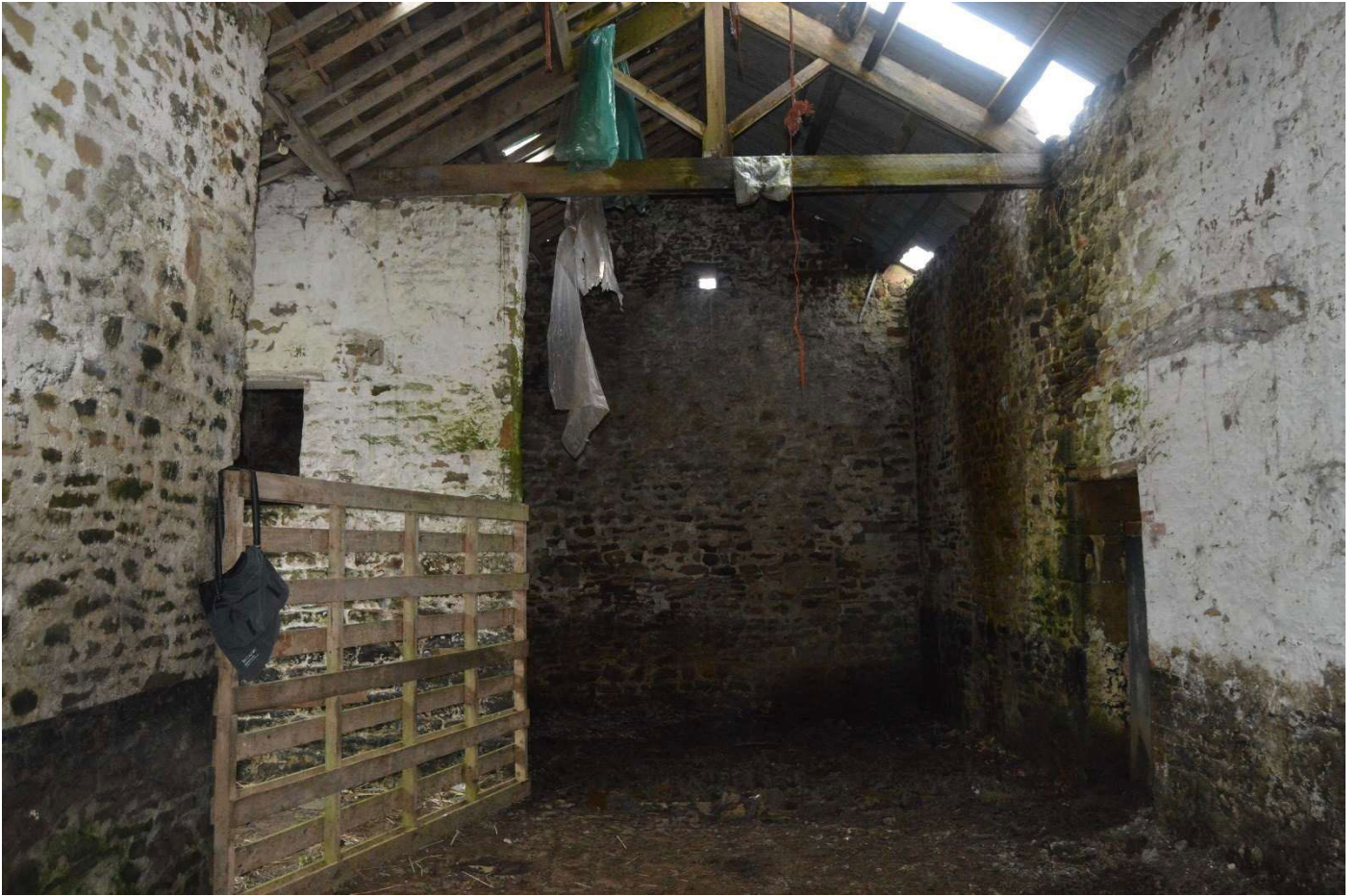
Fig 6 View east within the barn core
