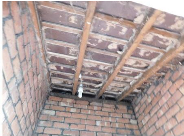
PHOTO 26 Underside of Kitchen Roof
