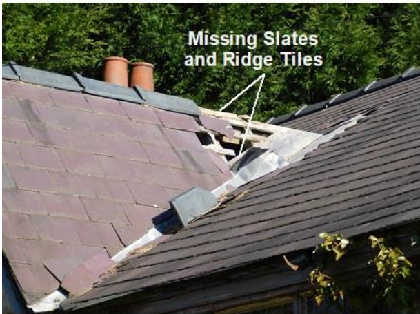
PHOTO 5 Southern Elevation of Porch Roof
