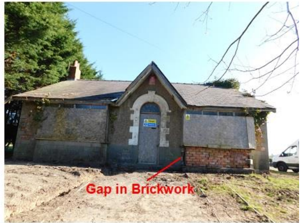
PHOTO 4 Southern Elevation of Bungalow
