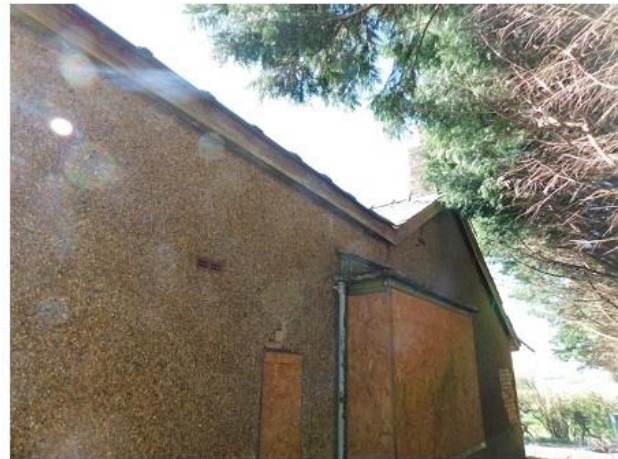
PHOTO 12 Western Elevation of Kitchen Extension
