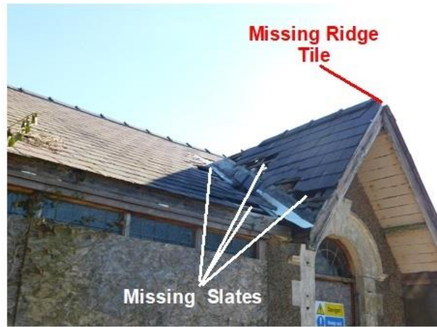
PHOTO 8 North-western Edge of Entrance Porch Roof
