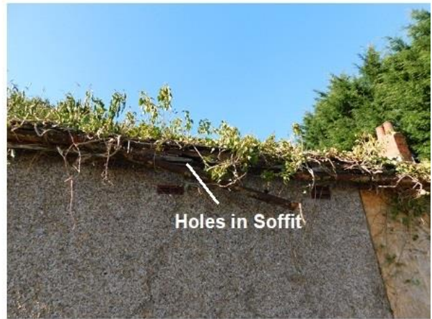
PHOTO 22 Upper Northern Elevation of Bungalow
