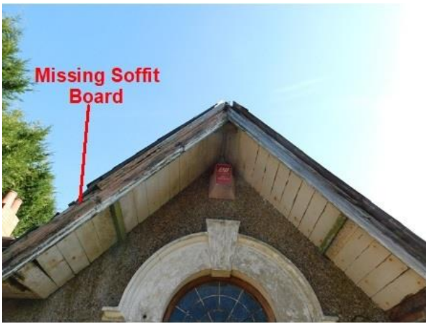
PHOTO 7 Southern View of Entrance Porch Roof
