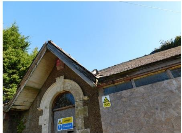
PHOTO 6 Southern View of Porch Roof
