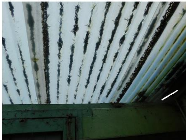
PHOTO 27 Underside of Utility Building Roof
