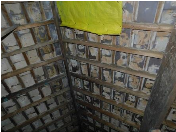
PHOTO 25 Underside of Extension Roof
