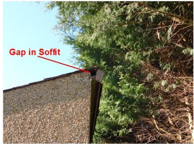
PHOTO 16 Upper Northern Corner of Kitchen
