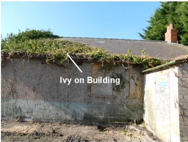
PHOTO 21 Northern Elevation of Bungalow
