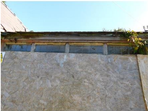
PHOTO 23 Upper Northern Elevation of Bungalow
