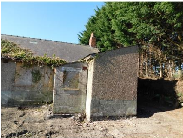
PHOTO 17 North-eastern Corner of Bungalow
