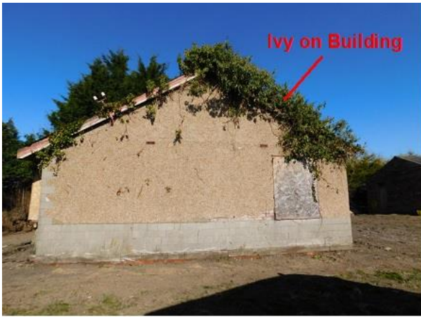
PHOTO 1 Eastern Elevation of Bungalow
