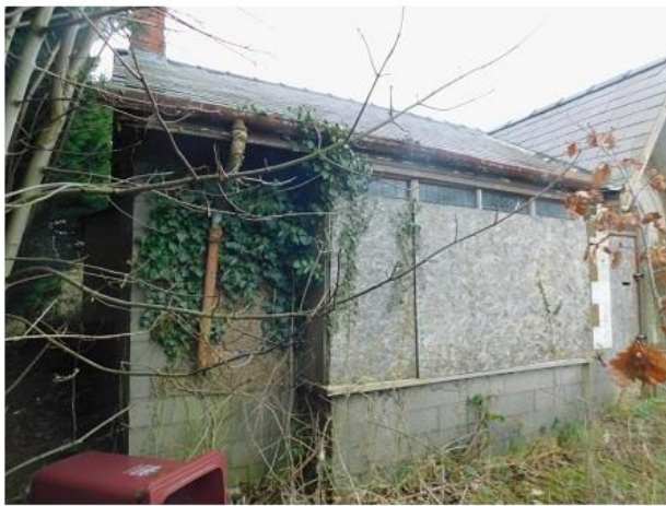
PHOTO 9 South-western Elevation of Bungalow
