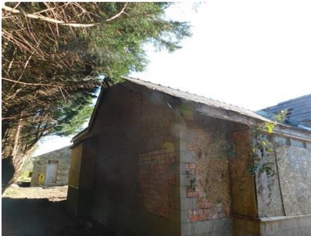
PHOTO 15 North-western Corner of Kitchen
