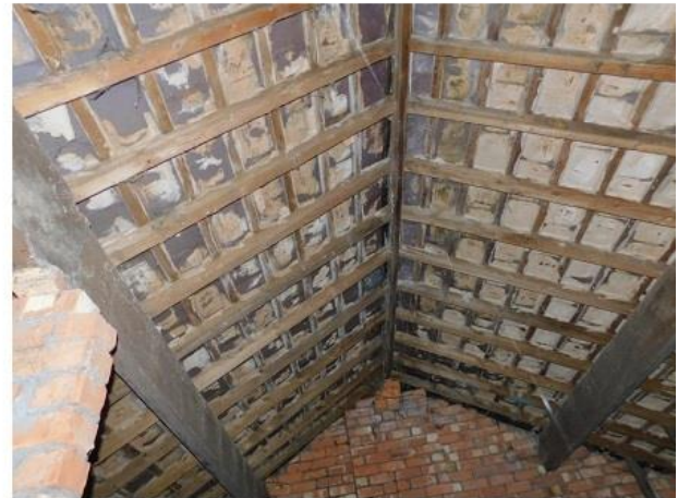
PHOTO 24 Underside of Bungalow Main Roof
