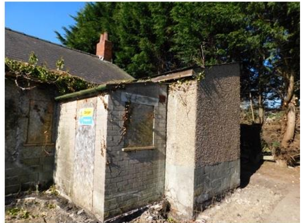
PHOTO 18 North-eastern Corner of Utility Building
