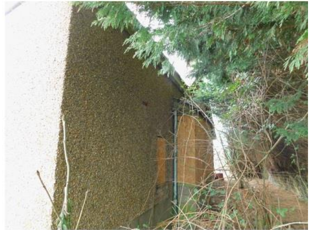
PHOTO 14 North-western View of Kitchen Elevation
