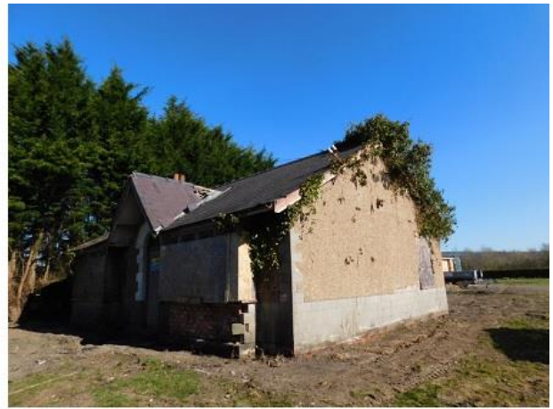
PHOTO 2 South-eastern Corner of Bungalow
