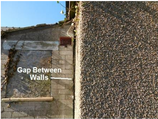
PHOTO 19 Part Northern Elevation of Utility Building
