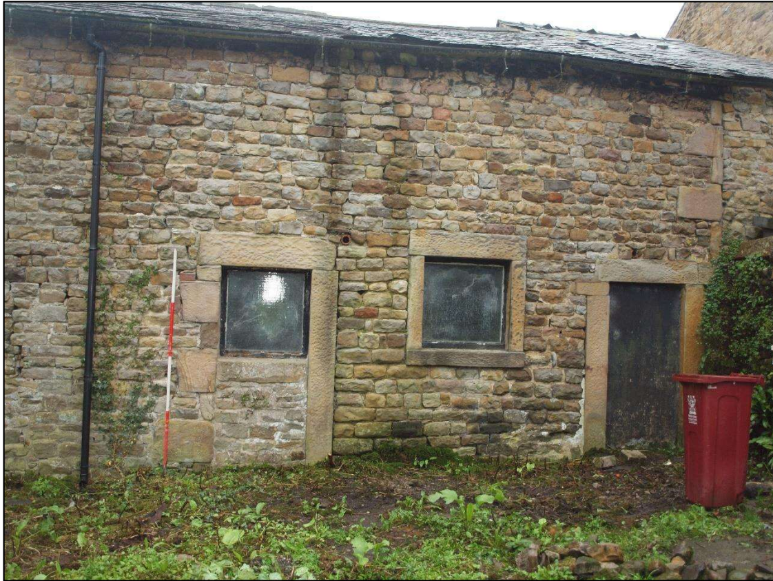
Plate 11: Doorways with cills and lintels to be raised and location of inserted first floor windows
