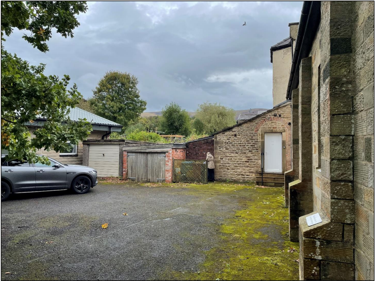
PL07: View of the garages to be demolished to the rear of the building.
