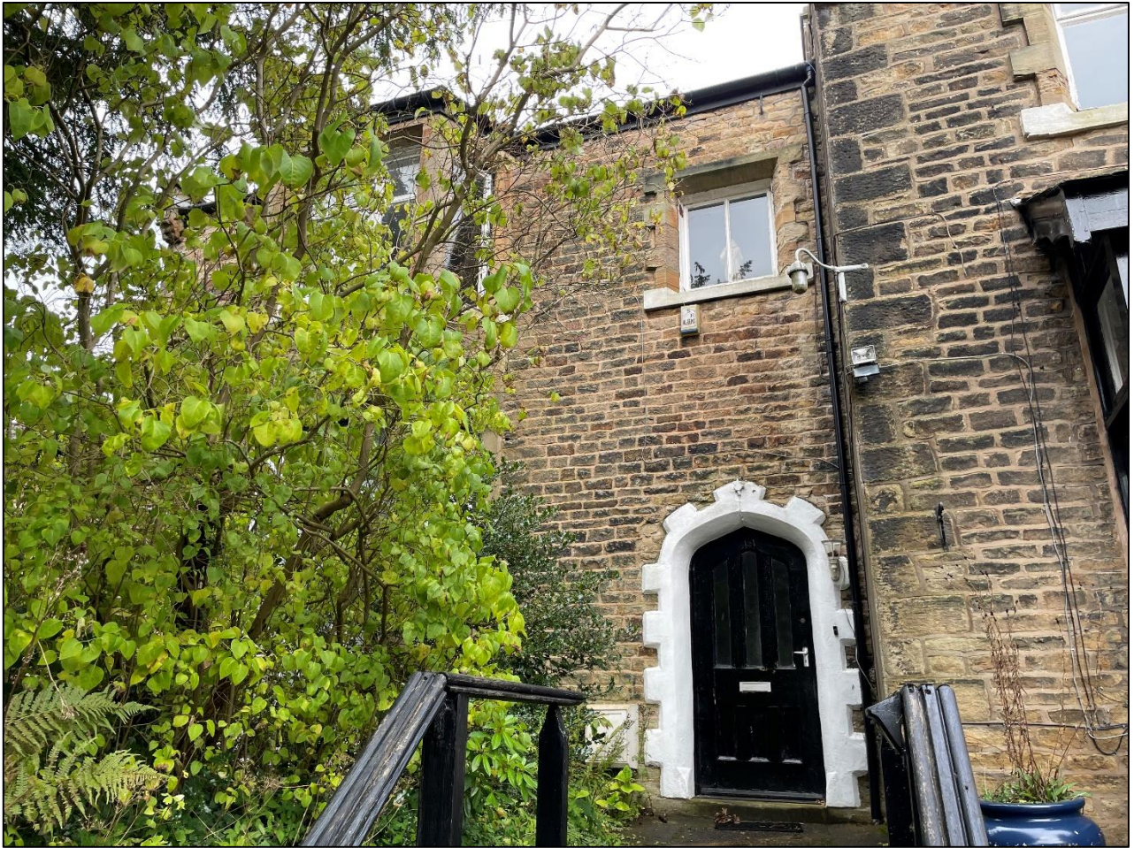
PL01: South east front elevation of the south western half of the building.
