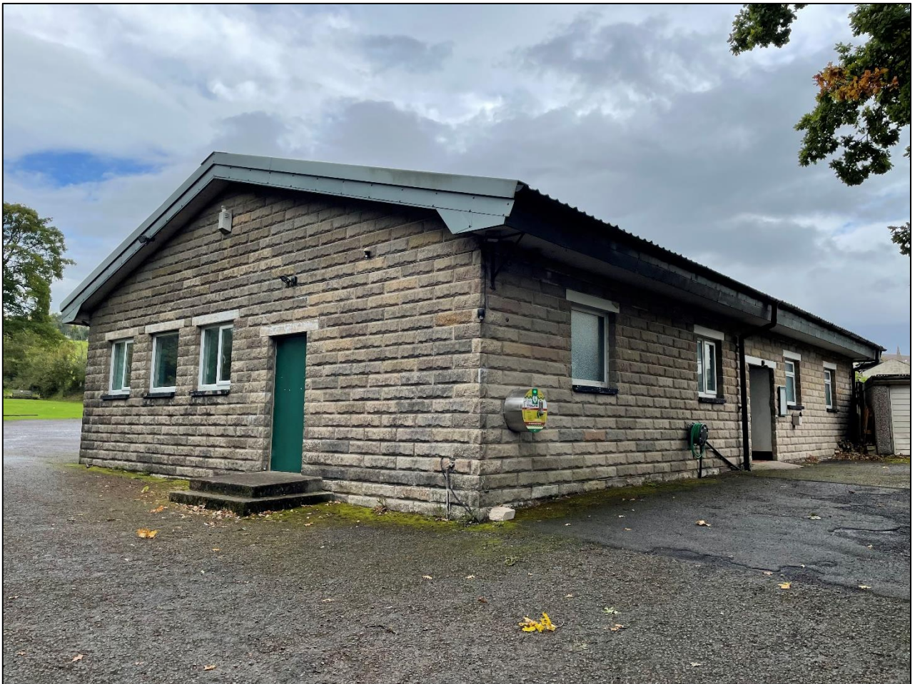
PL06: View of the existing church hall to the north east of the building.
