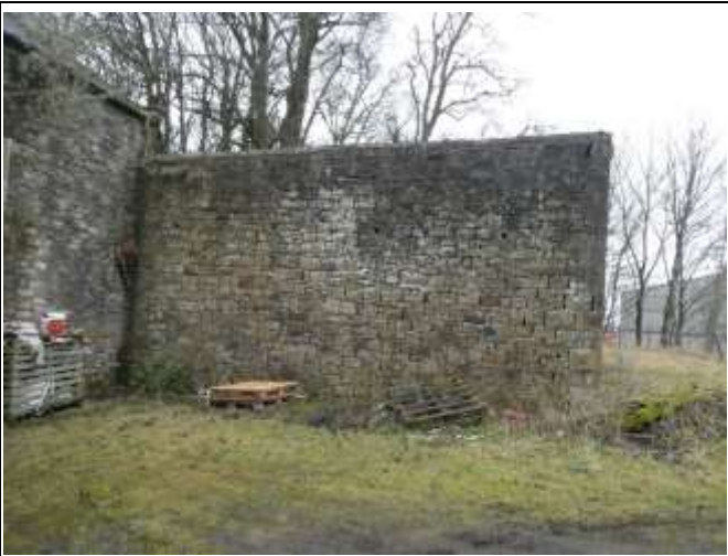
West Elevation of Outshut
