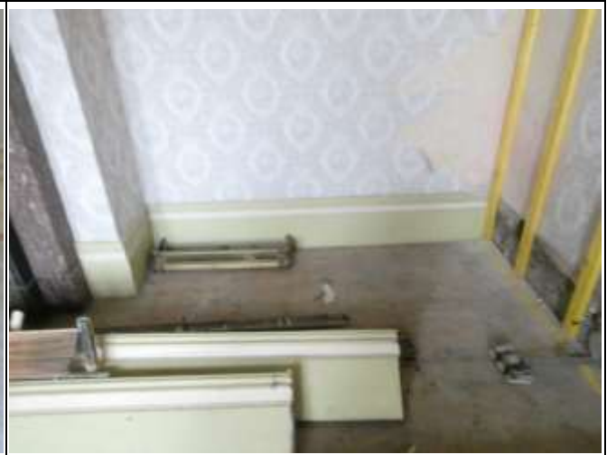
High Skirting Board in Situ
