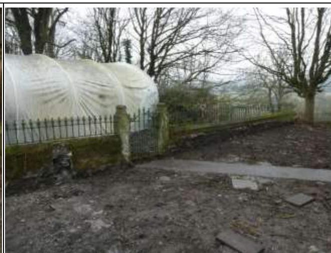
Former Front Garden with Stone Walling, Cast Iron Railing Top
