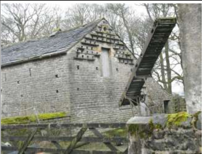
South Elevation with Dovecote
