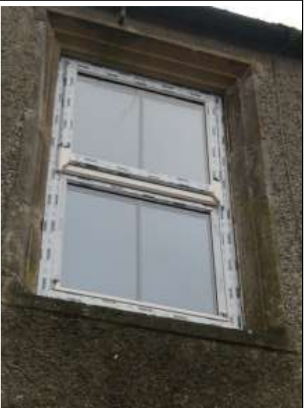
Window at the First Floor
