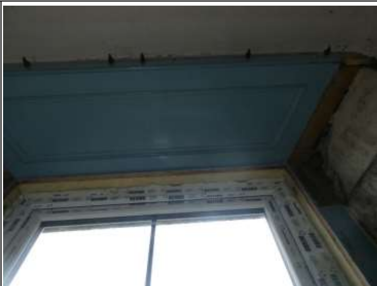
Remnant of Timber Shutters
