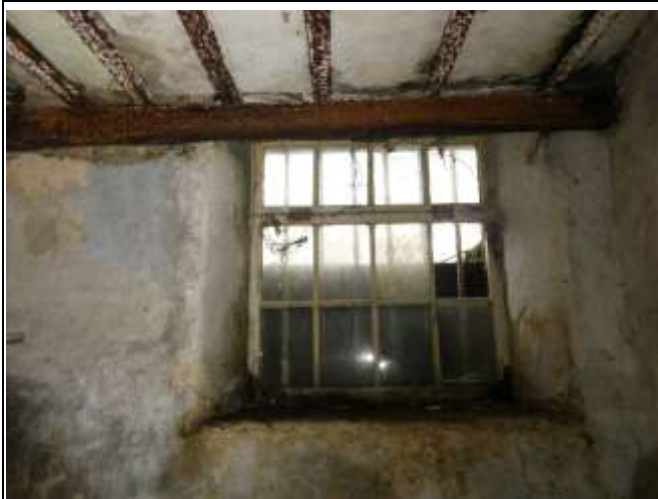
Timber Framed Window, Ironwork at the Ceiling
