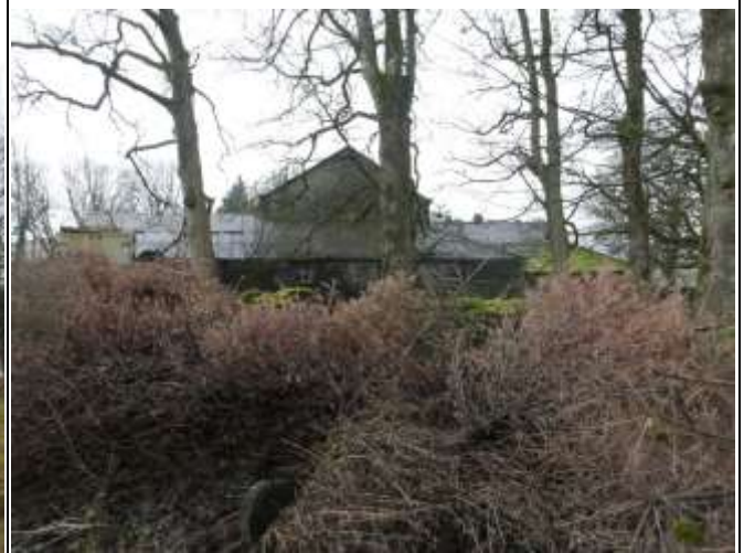
Looking North Towards Outshut and Outbuilding
