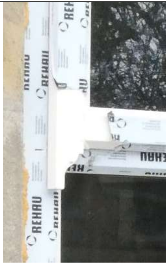
Horns and Joints of Replacement Window
