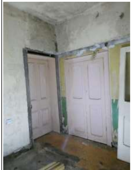
Built-in Cupboard at North Wall
