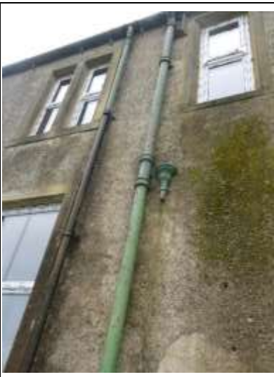
Plastic and Painted Cast Iron Downpipes
