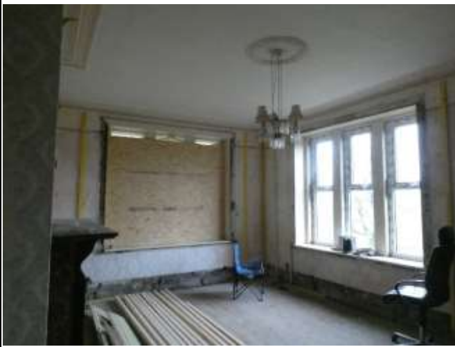
Windows at the Northwest Corner
