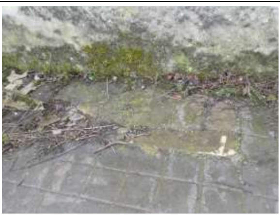
Former Basement Opening
