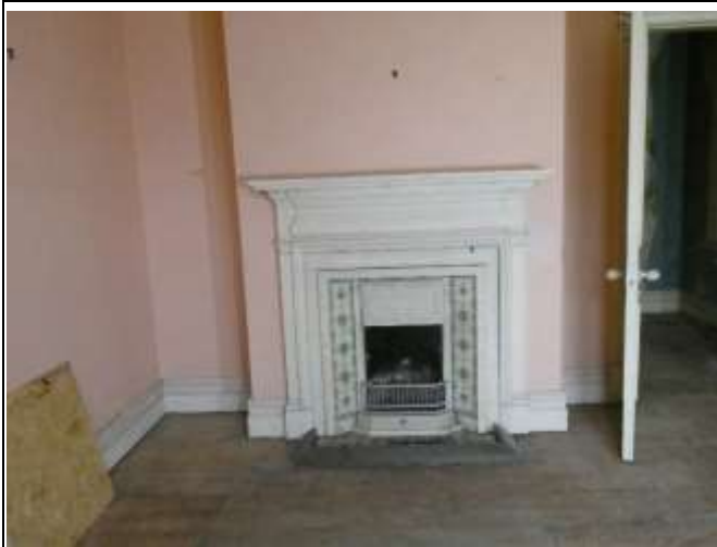
Cast Iron Surround at Fireplace
