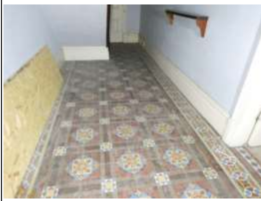
Tiled Flooring Under Stairs
