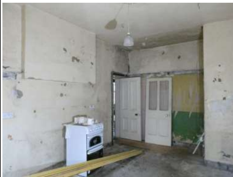
Looking Towards Door Leading to Hall 1
