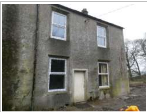
East Side of Elevation with Entrance
