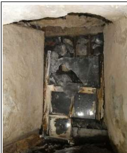
Small Blocked-up Opening at the East Elevation
