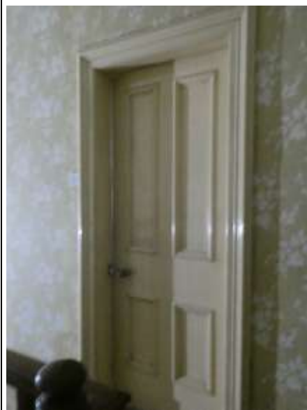
Panelled Door at Hall 4
