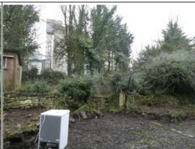
Stone Walling and Remaining Stone Pier
