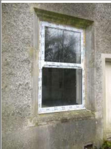
Window to the West of the Door
