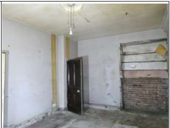
Painted Panelled Door Leading to the Scullery
