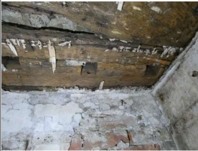
Ceiling at the Former Built-in Cupboard
