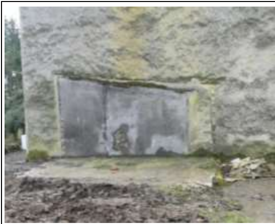
Former Extension with Hardstanding
