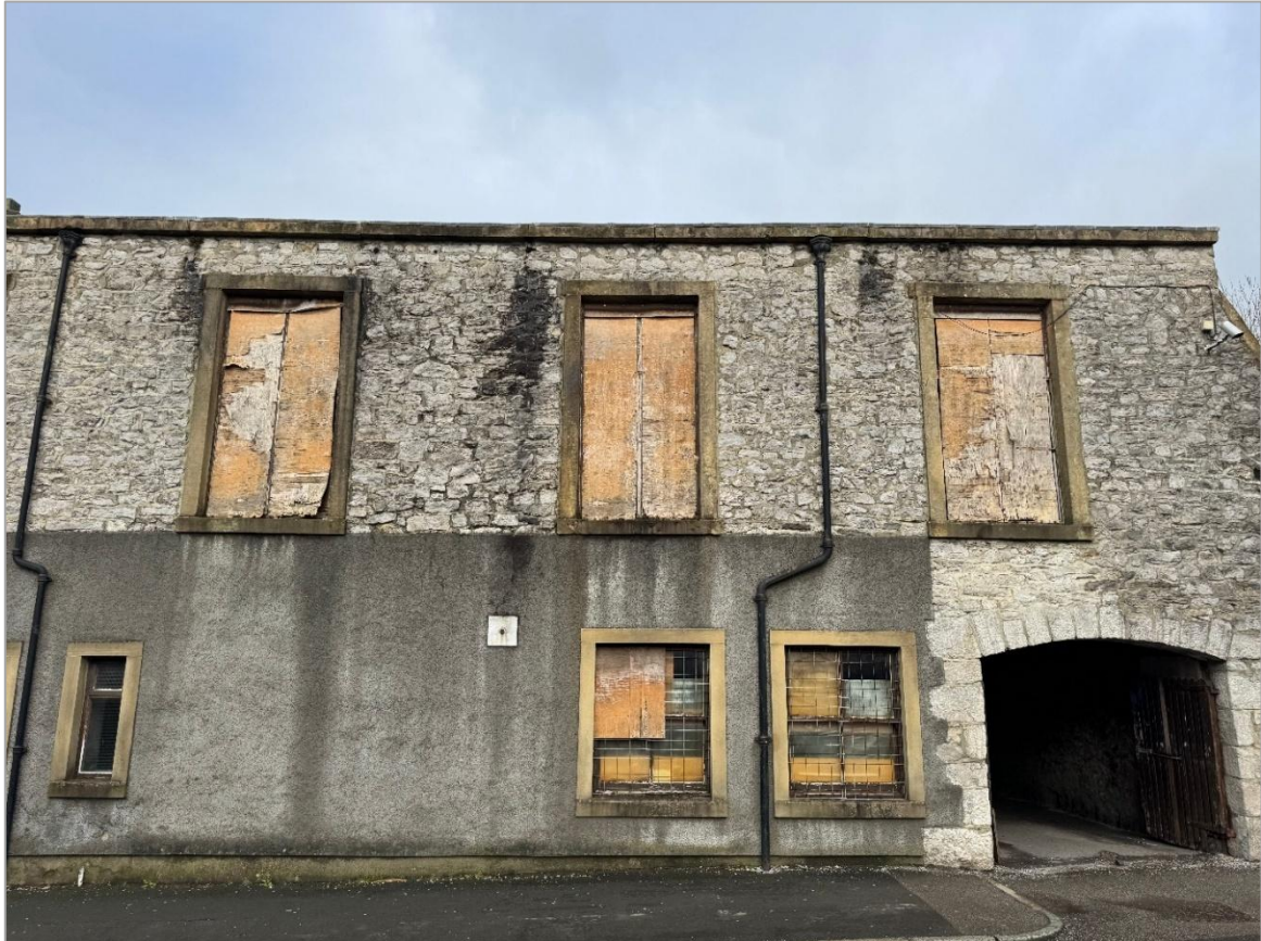
Figure 12) Turner Street elevation with tunnel
