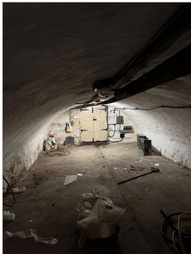
Figure 17) Vaulted cellar to number 45
