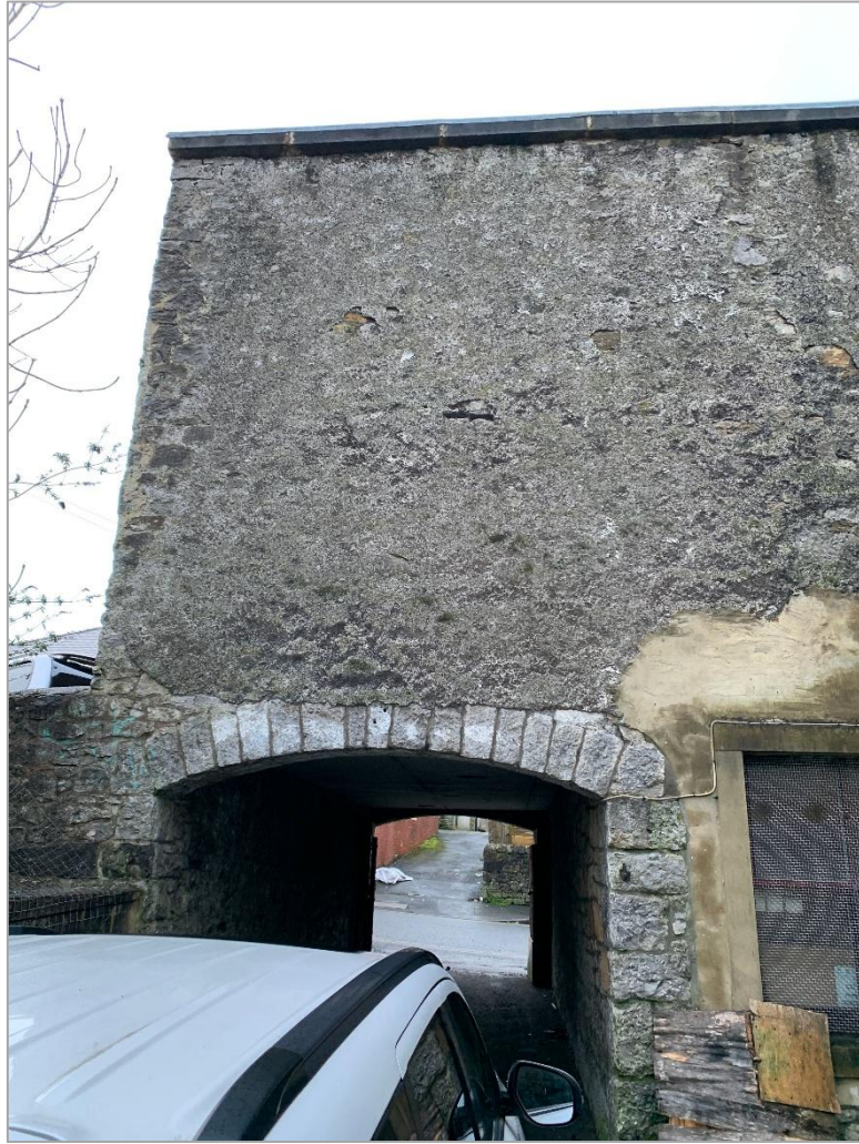
Figure 14) Tunnel from within rear courtyard
