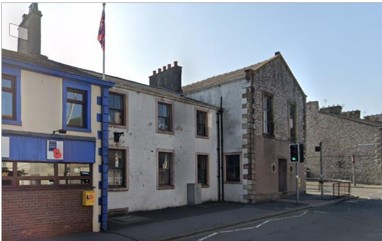
Figure 11) The Whalley Road frontage – the central ground floor window to number 45 was formerly a door (2021)
