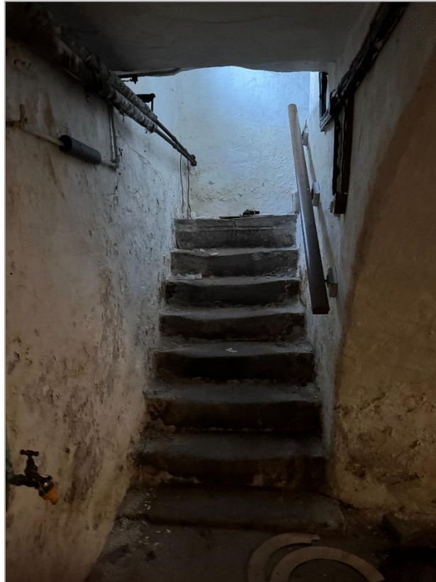
Figure 16) Stone cellar stair to number 45
