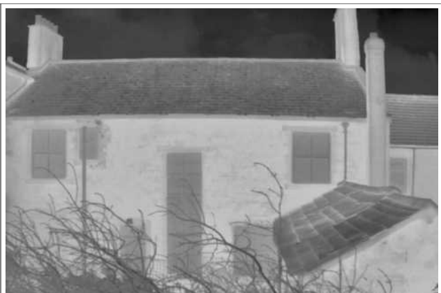
Thermal camera coverage
