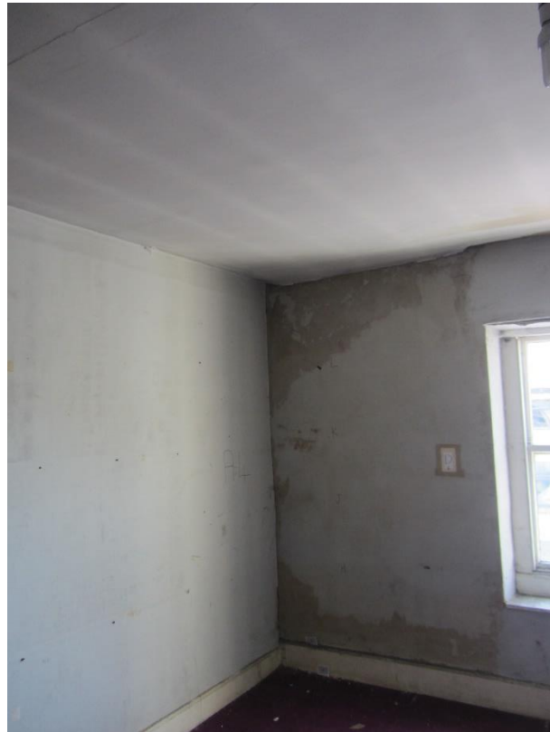
Photo 5 – Penetrating damp
