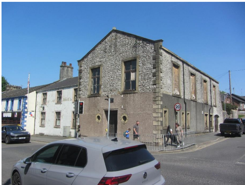
Photo 2 – View barn from south west
