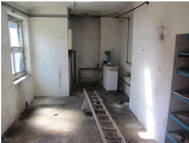
Photo 20 – External store room
