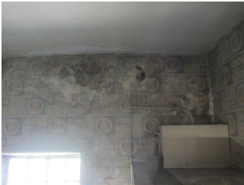
Photo 7 – Penetrating damp
