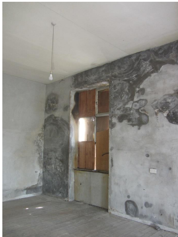
Photo 12 – Penetrating damp
