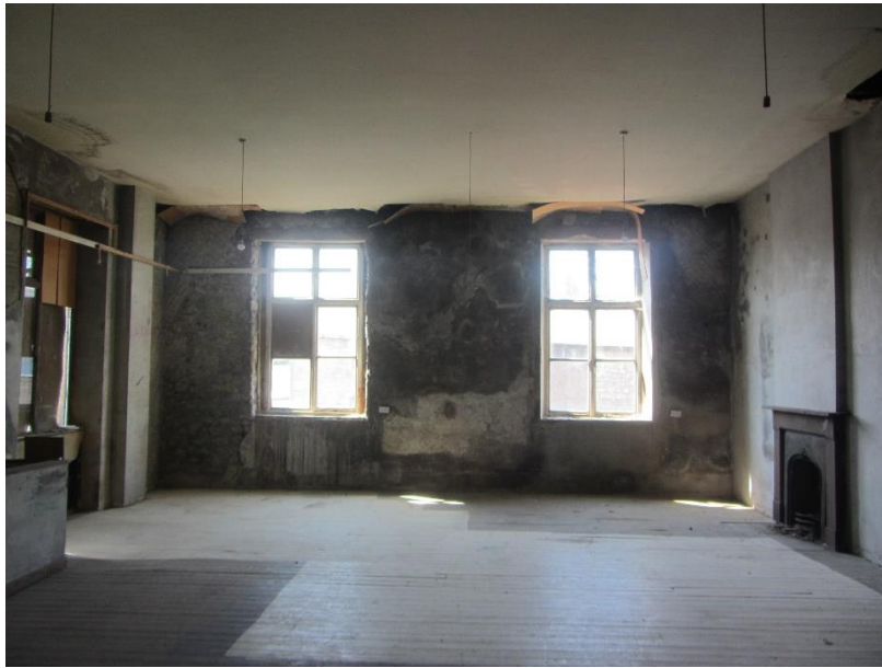
Photo 11 – Penetrating damp
