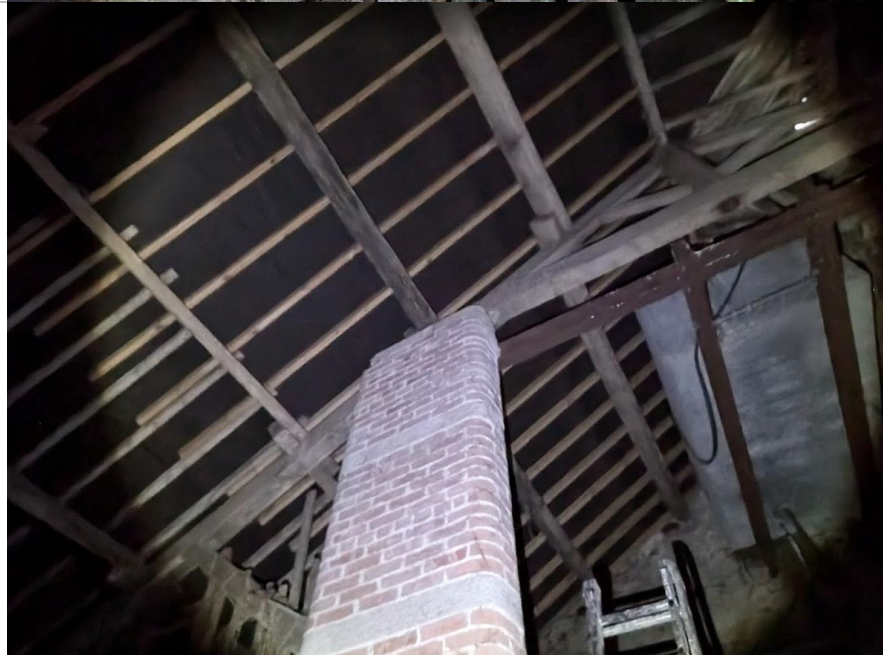
Photo 6. Centre column of barn.
