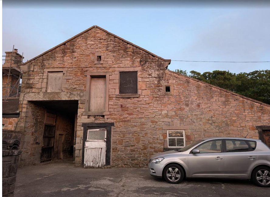
Photo 1. North-east elevation of barn
