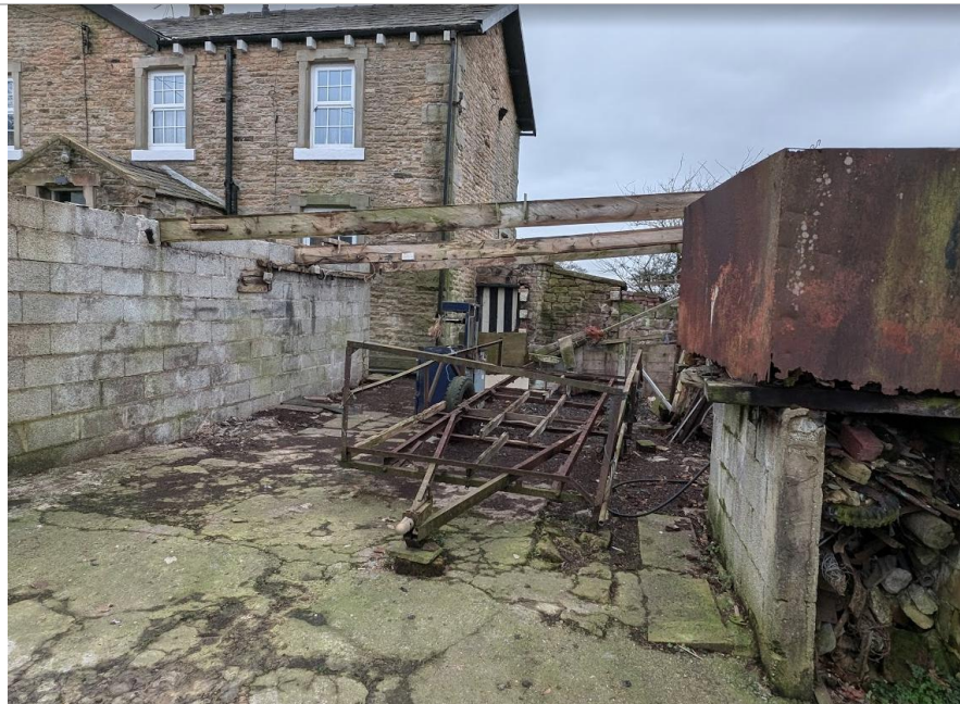
Photos 9a & 9b Areas of former outbuildings (stone lean-to in background).
