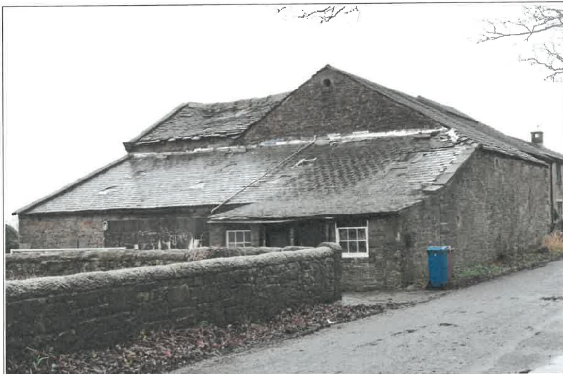
Photo 4: Barn, from the south. Lean-to shippon with later dairy on south-west end. Garden boundary wall in foreground.
