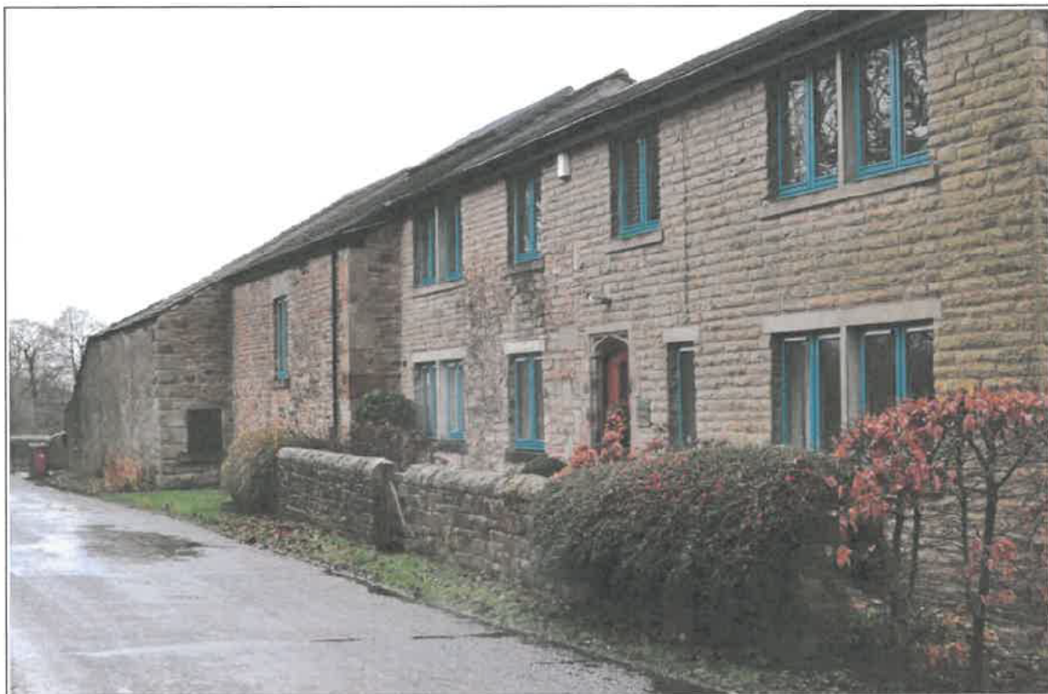
Photo 6: Holmes Cottage, incorporating previously converted part of barn
