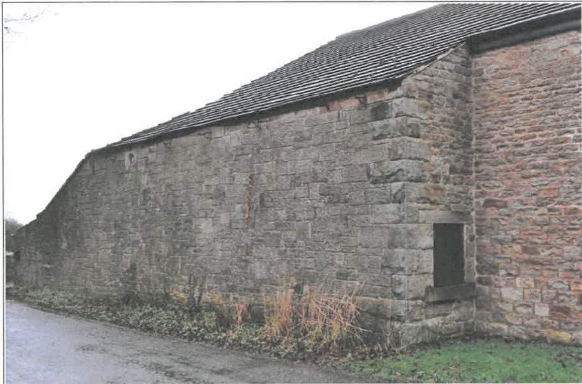
Photo 5: Roadside elevation of barn, in distinctly modern style of stonework
