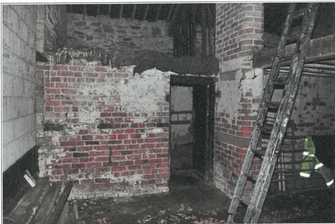
Photo 7: Barn interior, looking south-east from cart entrance
