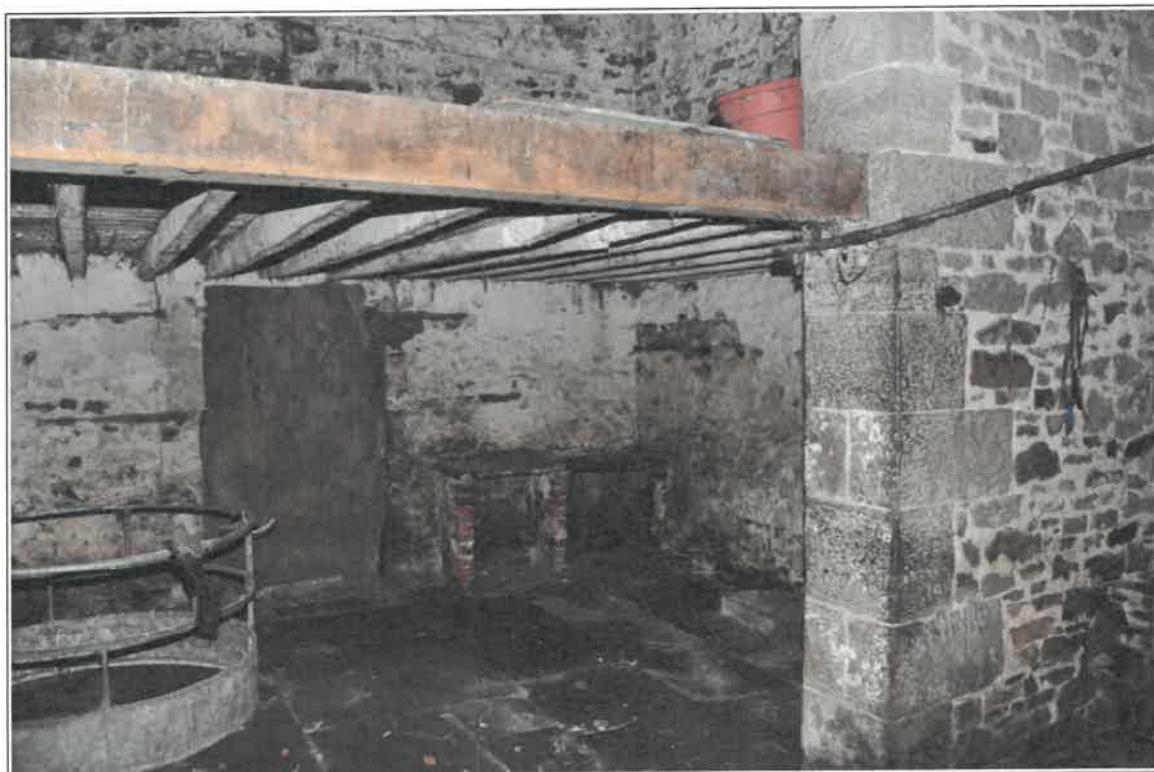
Photo 8: Barn interior: hayloft next to cart entrance
