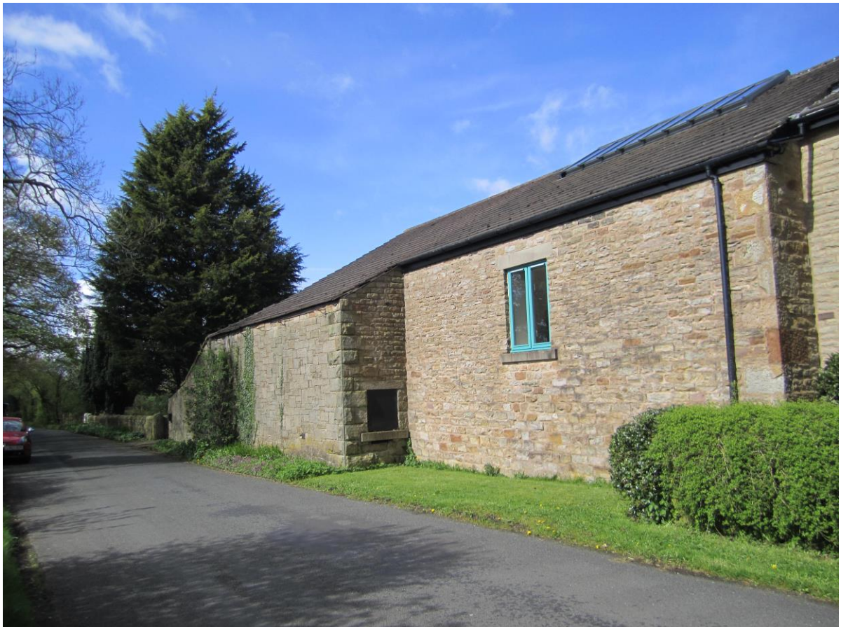
2 Rooflights positioned at the ridge line of Holmes Cottage
