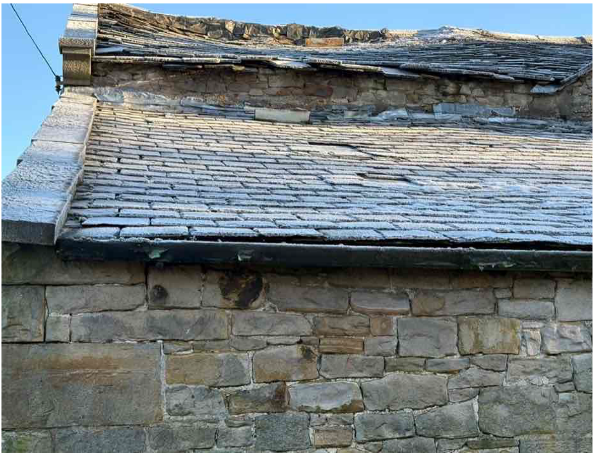
Photo 7 – South West Elevation
