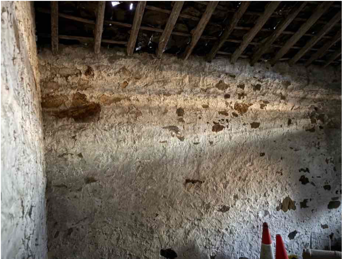
Photo 24 – Walls in loft area
