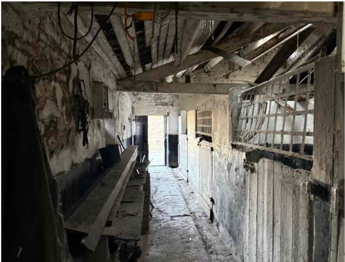
Photo 39 - Lean to stable area to south west elevation
