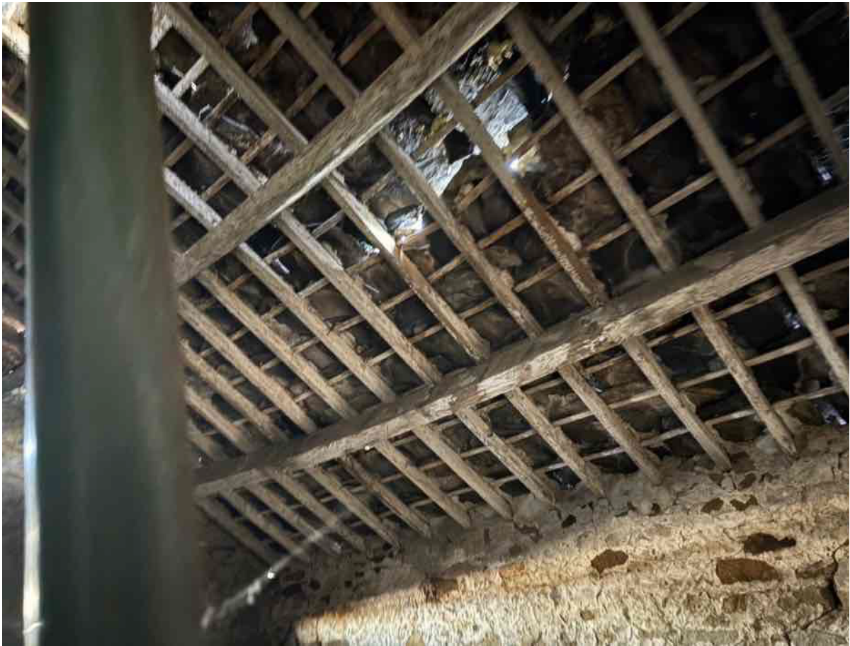
Photo 22 - Internal – original roof over rear (north west) area
