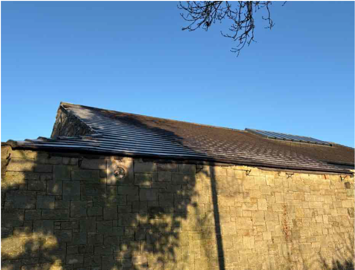
Photo 12 - South East Elevation
