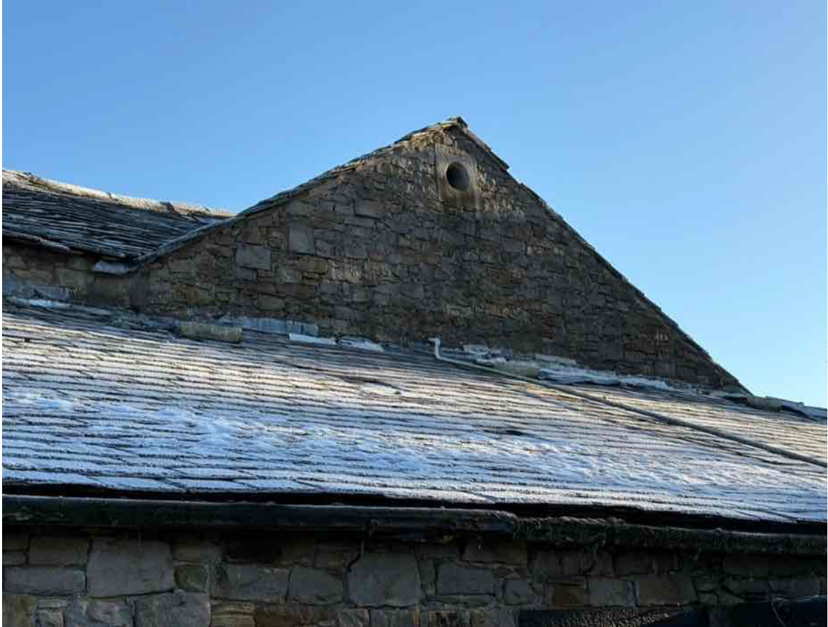
Photo 6 – South West Elevation
