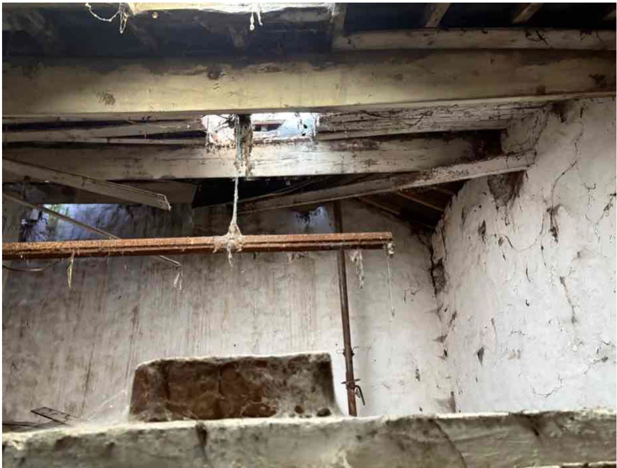
Photo 40 - Lean to stable area to south west elevation
