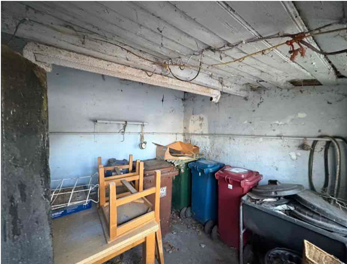
Photo 42 - Outbuilding on south west elevation
