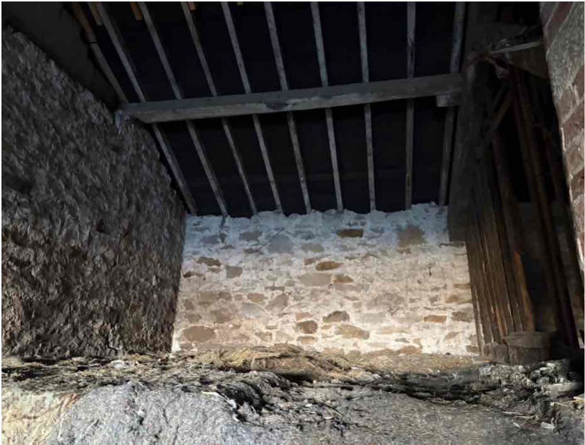
Photo 26 – Loft area adjacent to south east elevation
