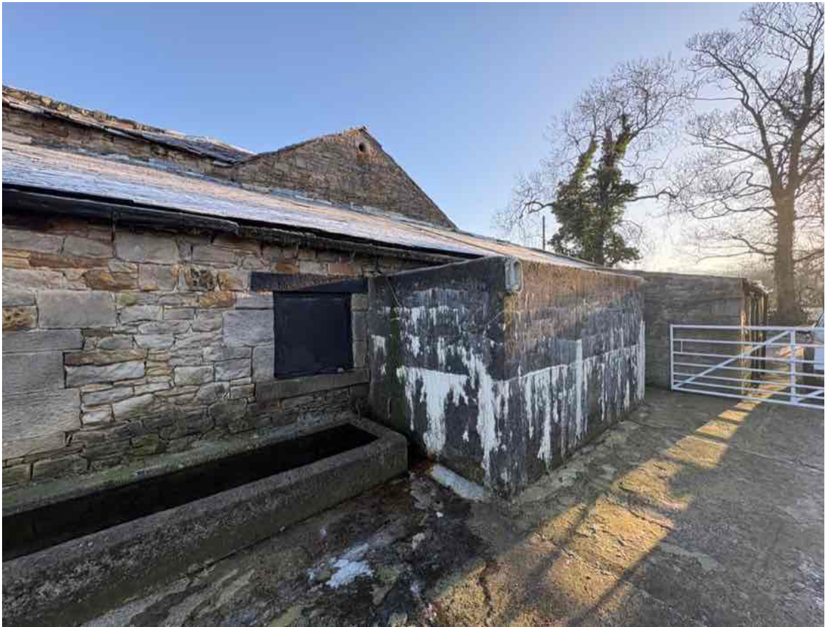
Photo 8 – South West Elevation
