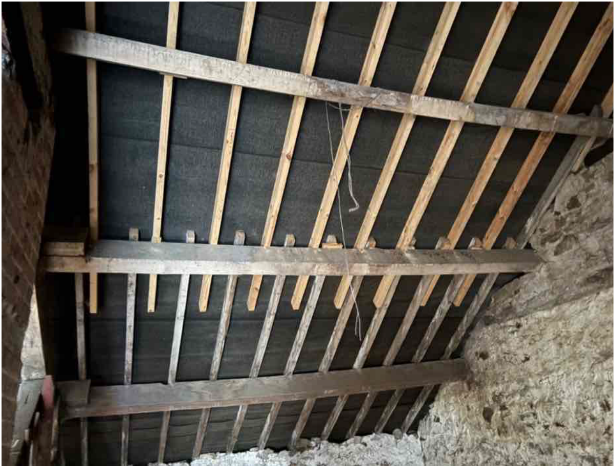
Photo 18 – Internal new roof to south east
