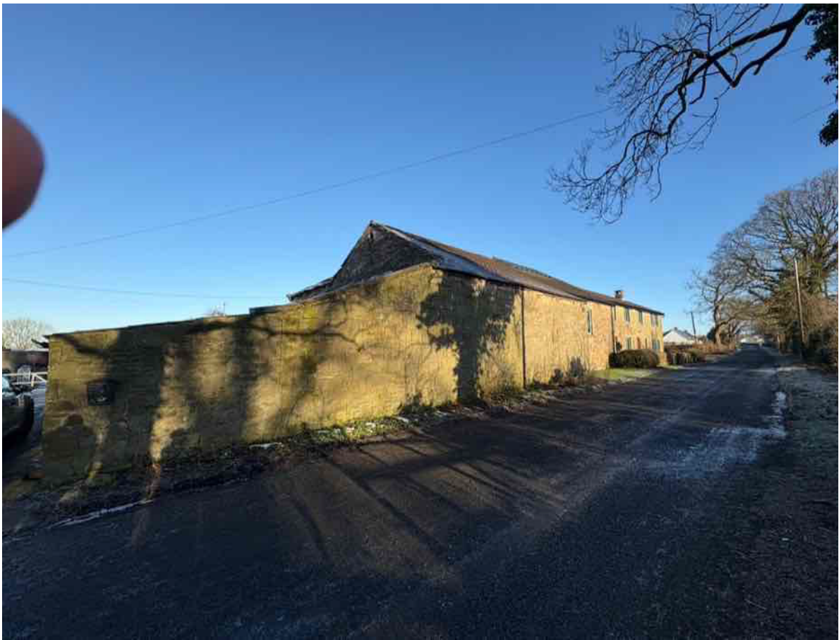
Photo 11 - South East Elevation
