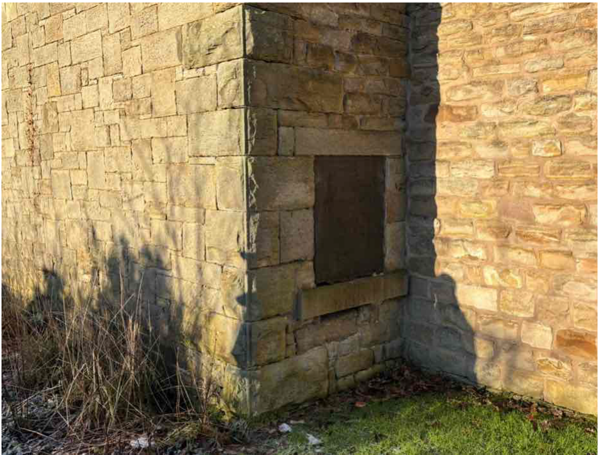
Photo 15 - South East Elevation and return on North East Elevation
