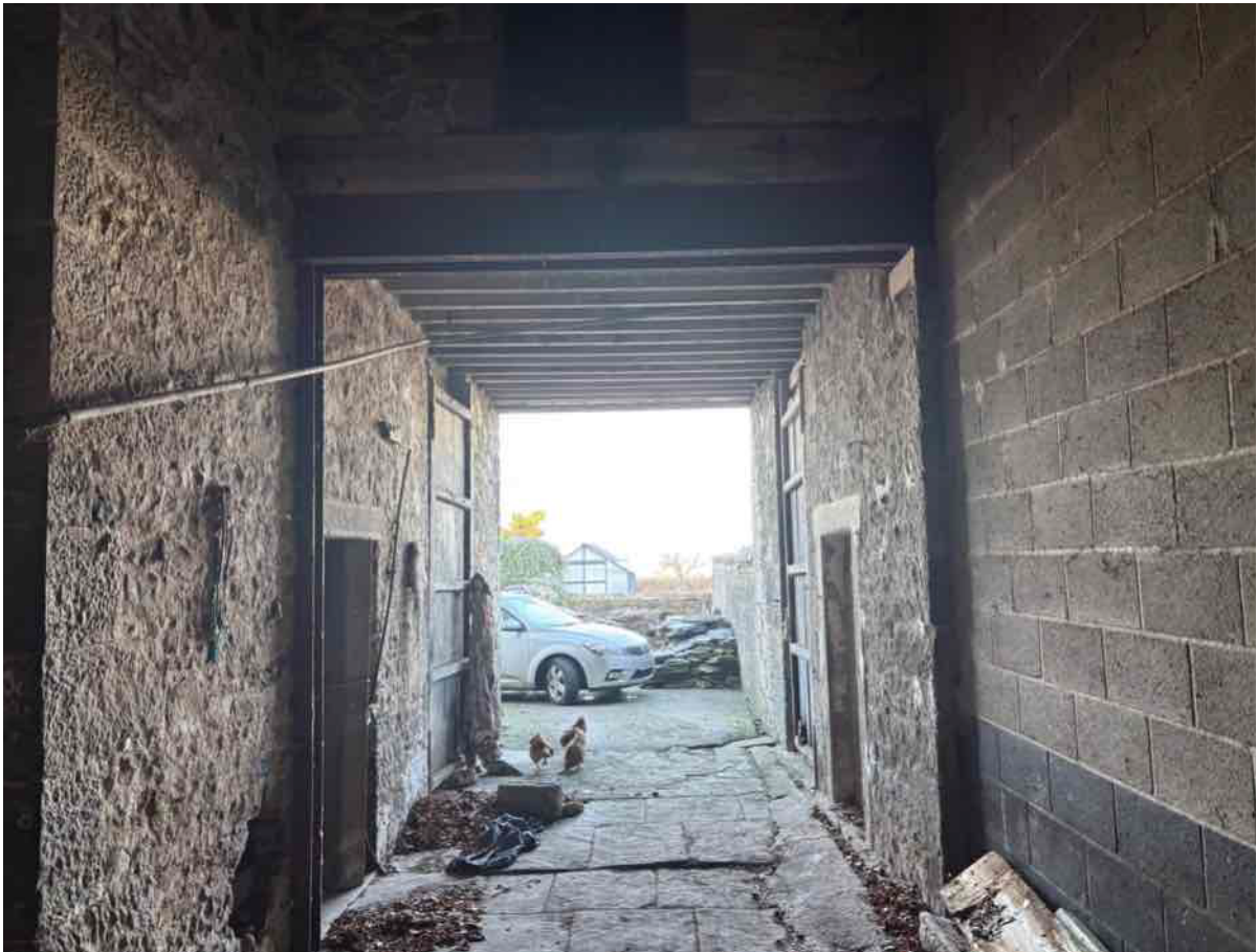
Photo 28 – Internal view to main barn door on north west elevation
