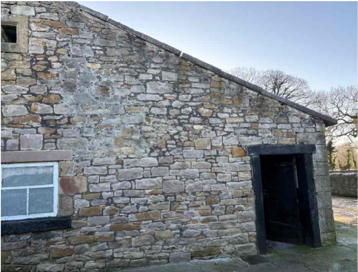
Photo 2 – North West Elevation
