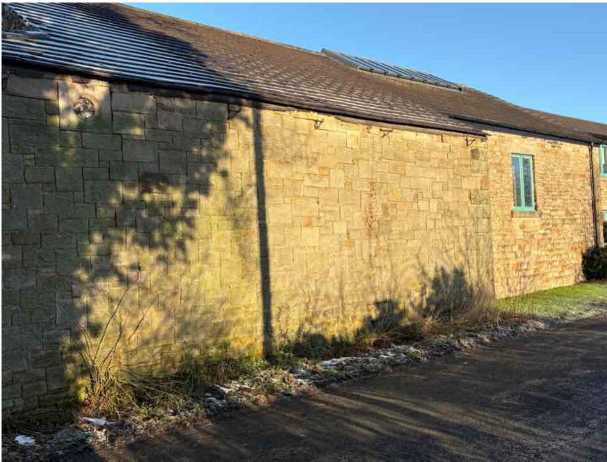
Photo 13 - South East Elevation
