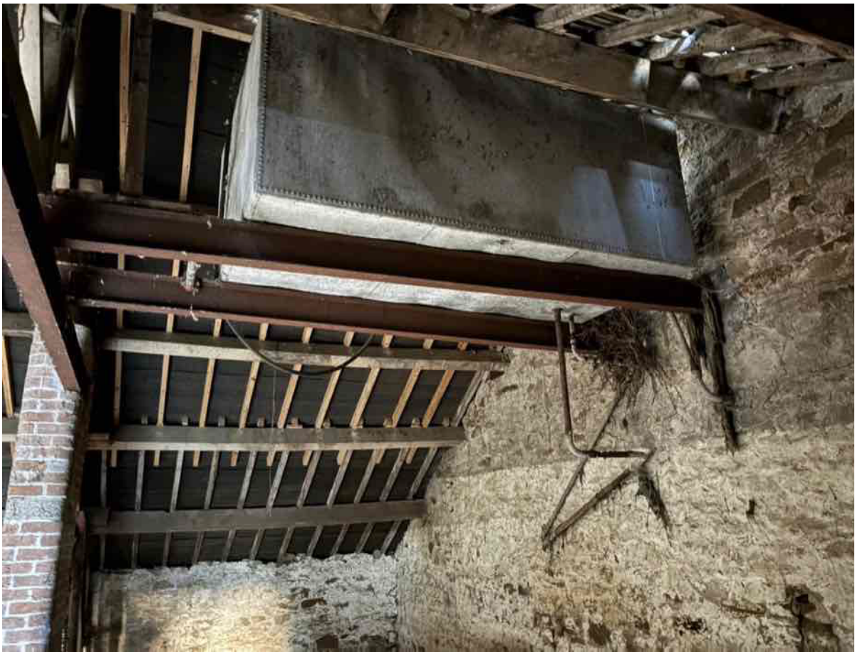
Photo 25 – Internal – tank and steel supports over loft
