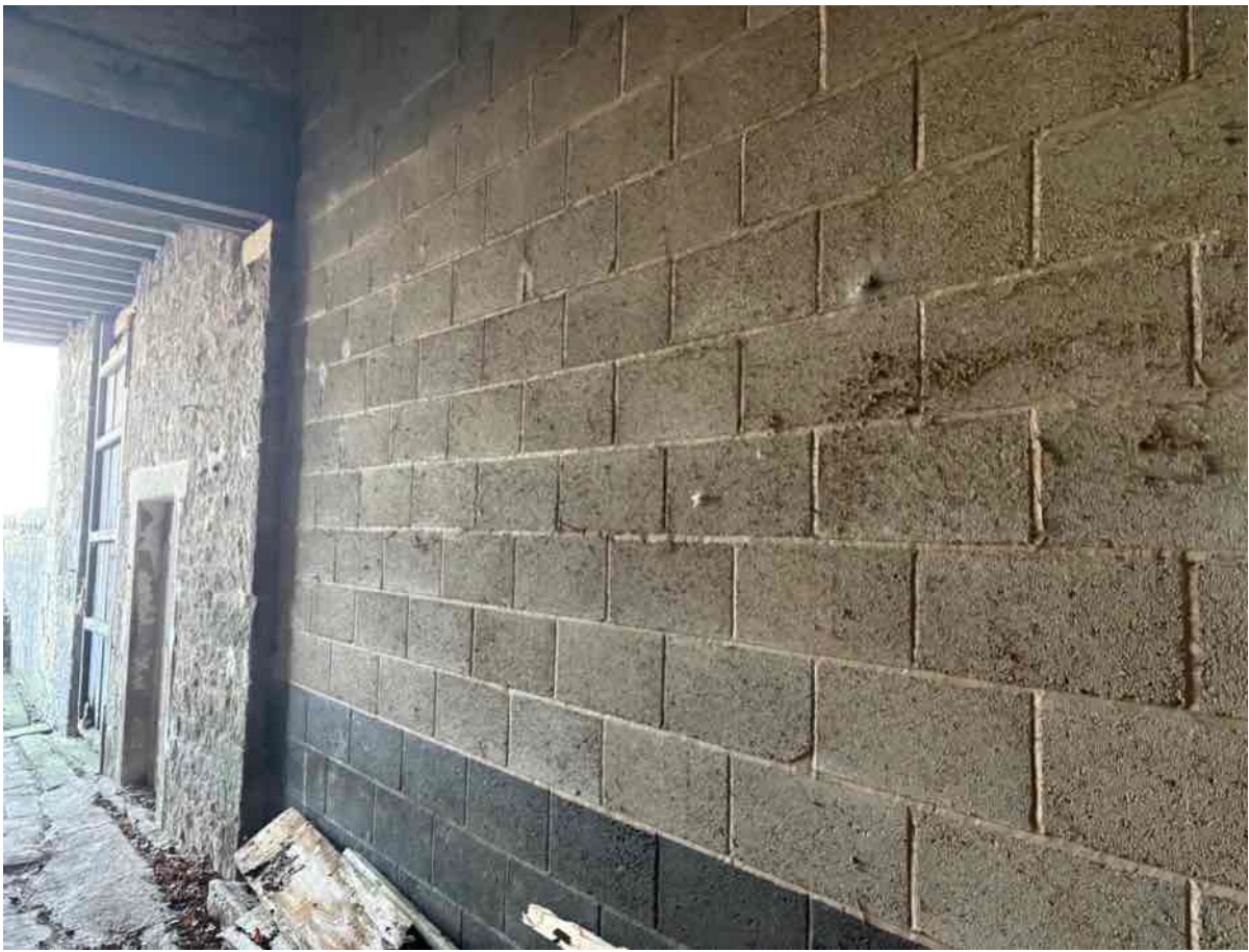
Photo 29 – New party wall to adjacent property on north east elevation
