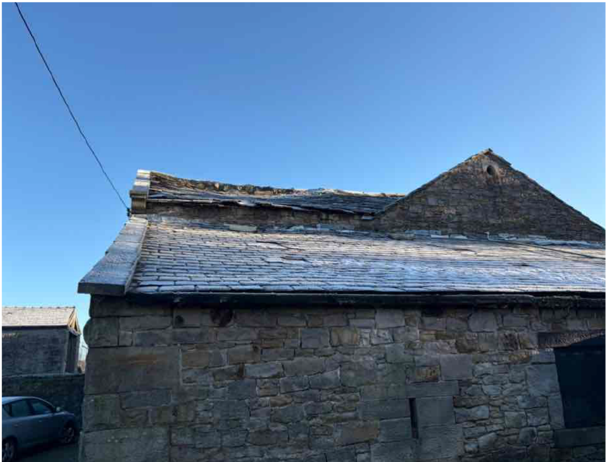
Photo 3- South West Elevation
