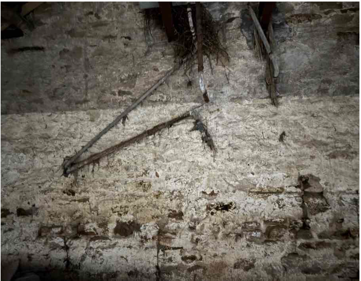
Photo 19 – Internal south east wall
