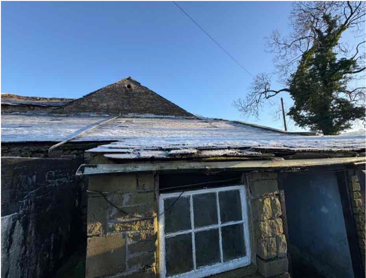
Photo 10 – South West Elevation
