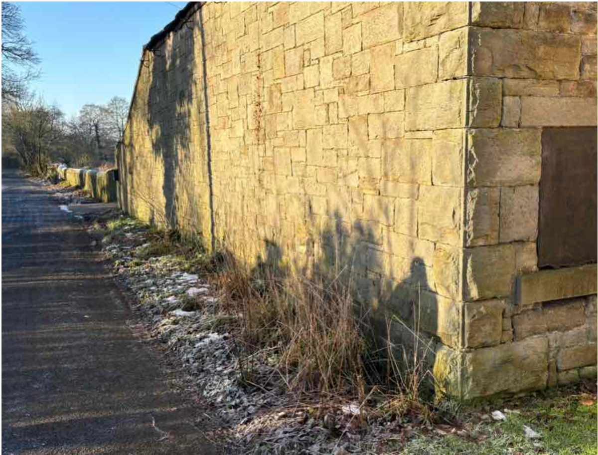
Photo 16 - South East Elevation and return on North East Elevation
