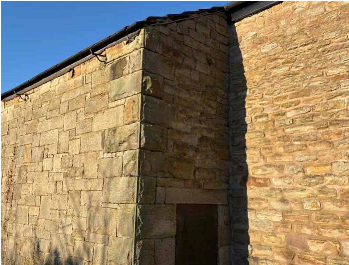
Photo 14 - South East Elevation and return on North East Elevation
