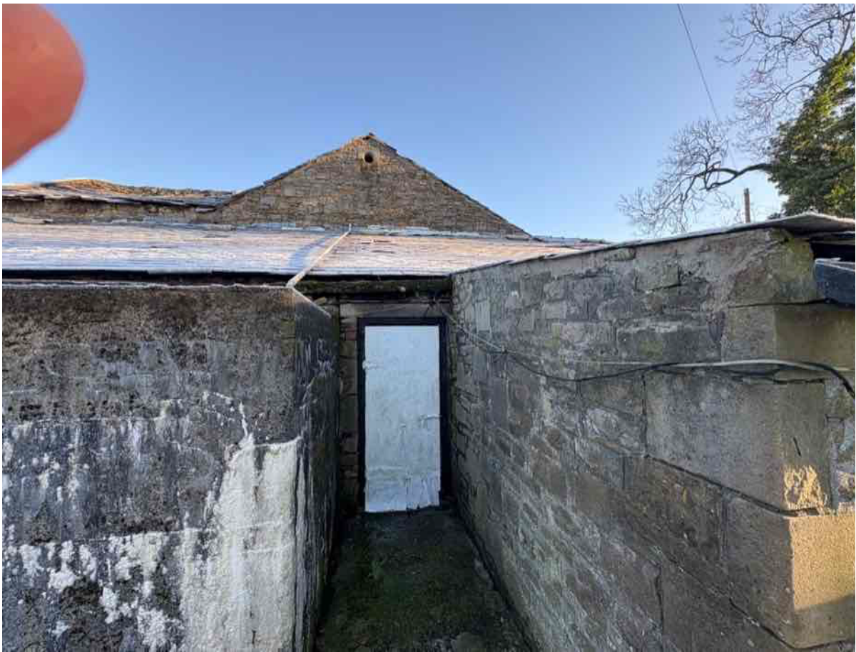
Photo 9 – South West Elevation
