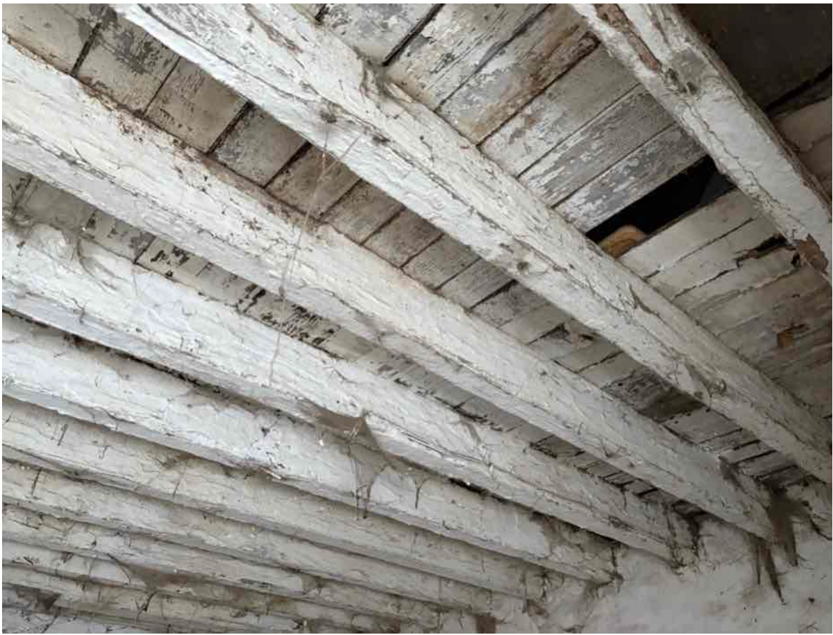
Photo 31 – Timber to loft area
