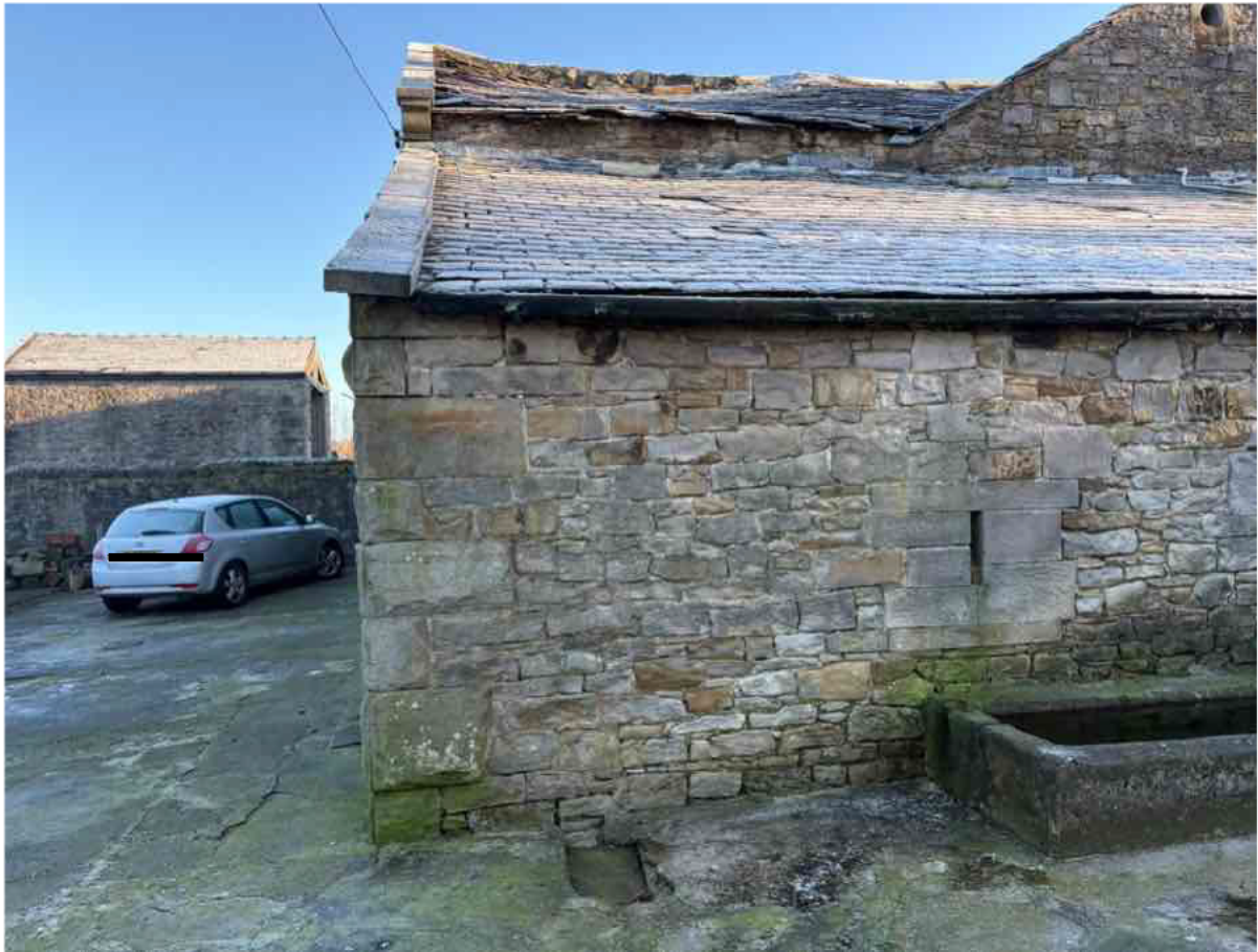
Photo 4 - South West Elevation
