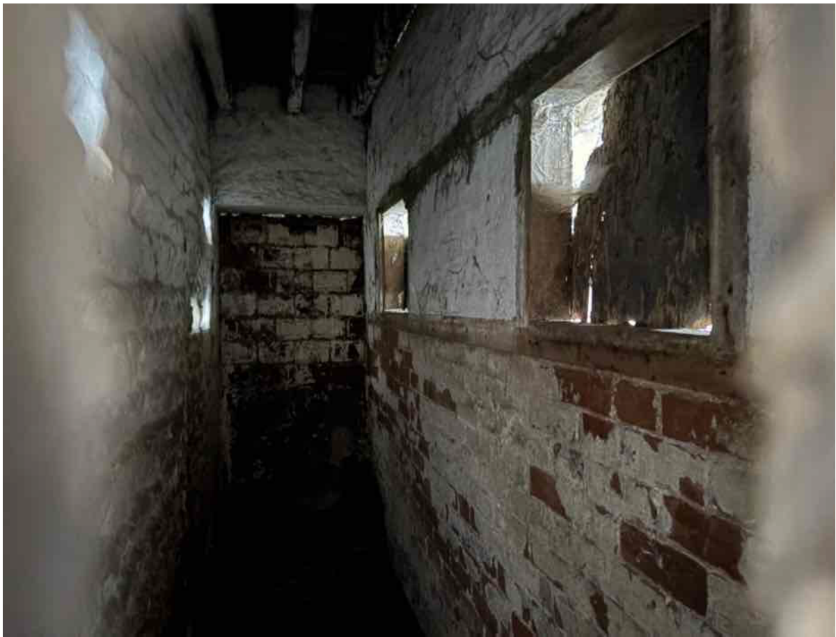
Photo 33 – Corridor adjacent to stable
