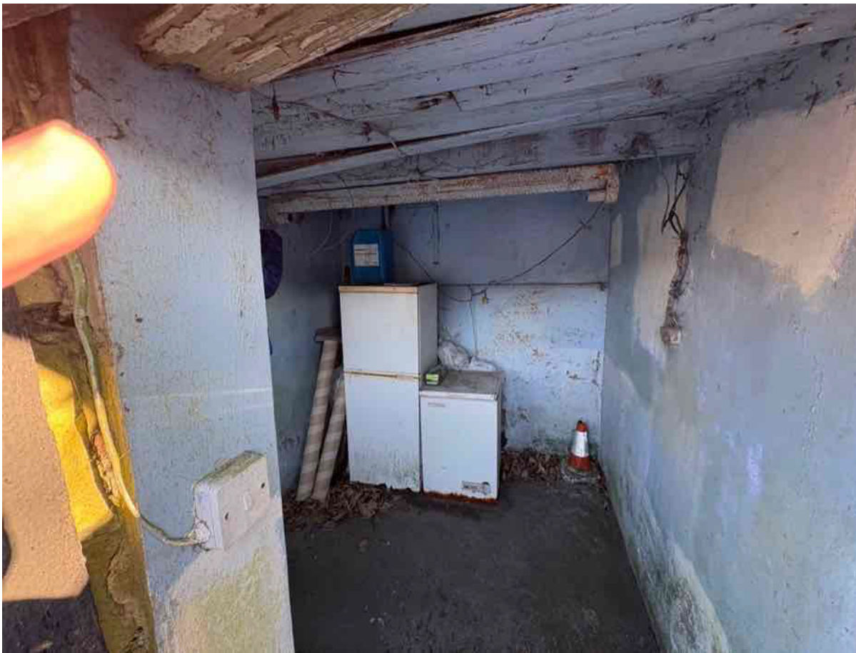
Photo 41 – Outbuilding on south west elevation
