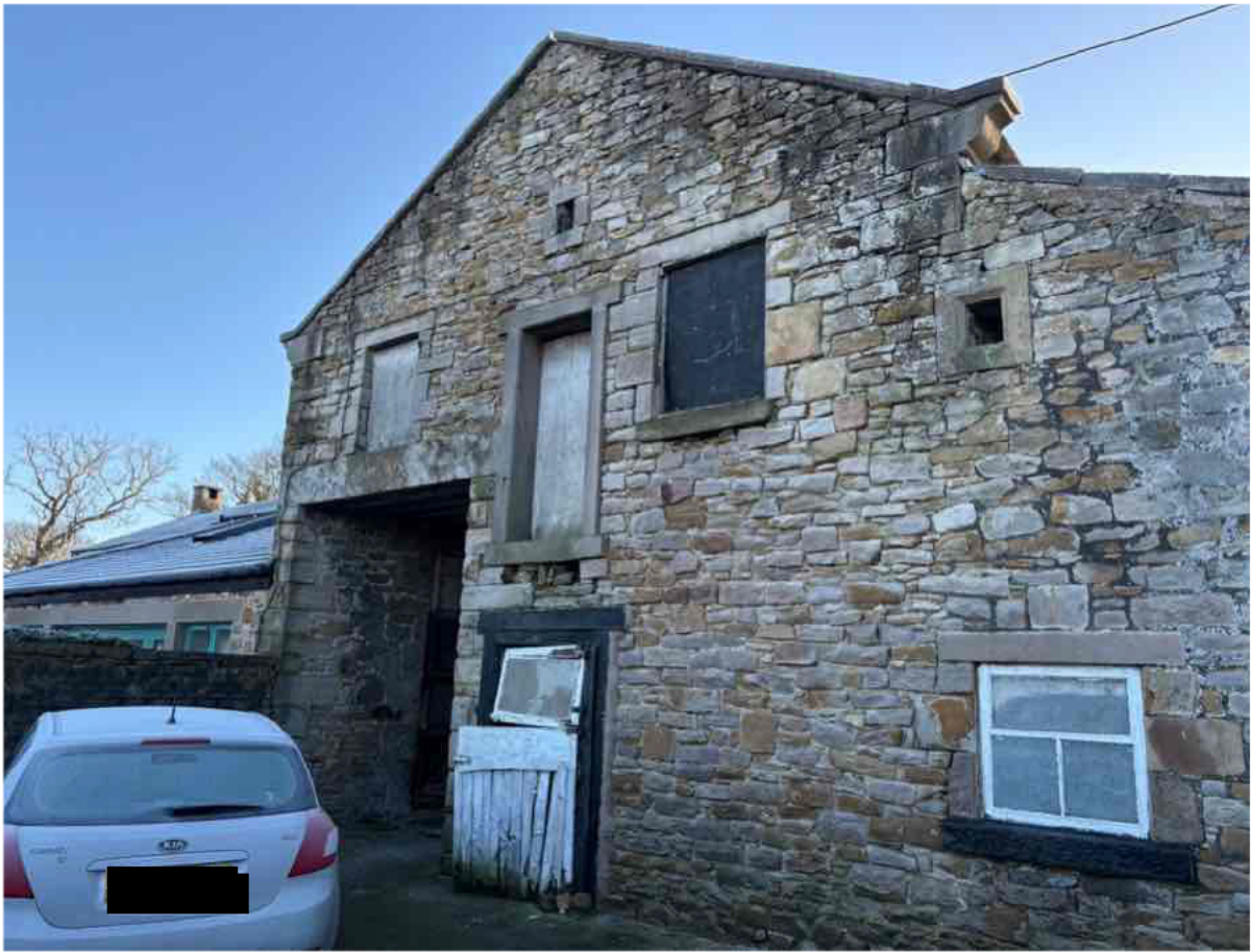
Photo 1 - North West Elevation
