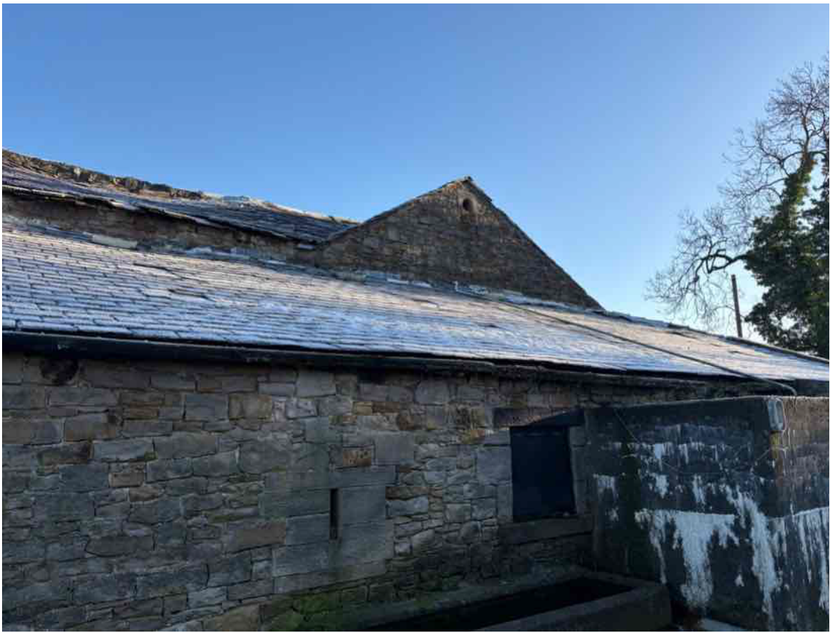
Photo 5 – South West Elevation
