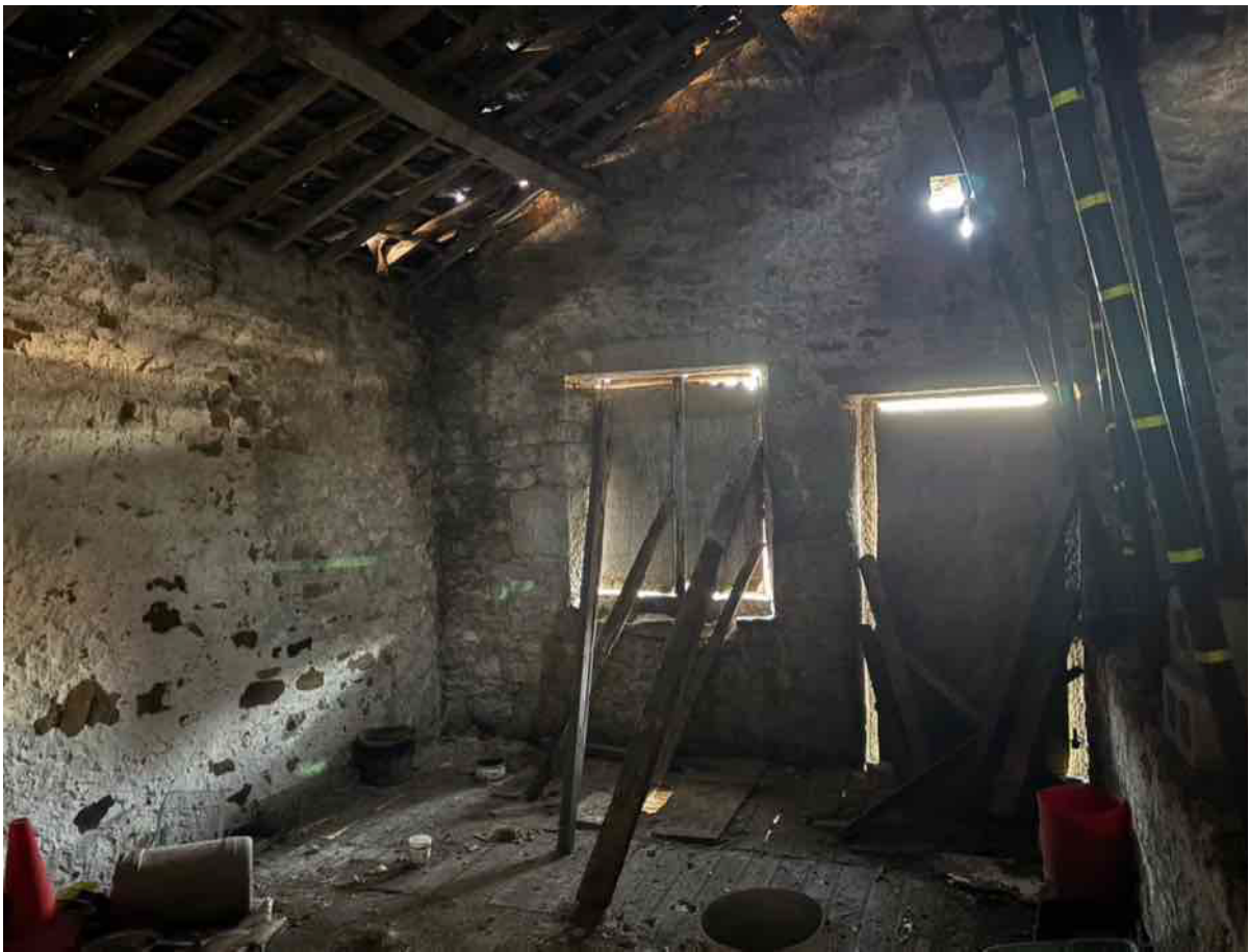
Photo 23 – Loft area looking to north west elevation
