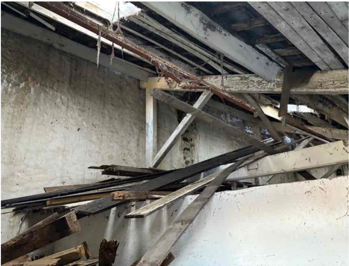
Photo 37 – Lean to stable area to south west elevation
