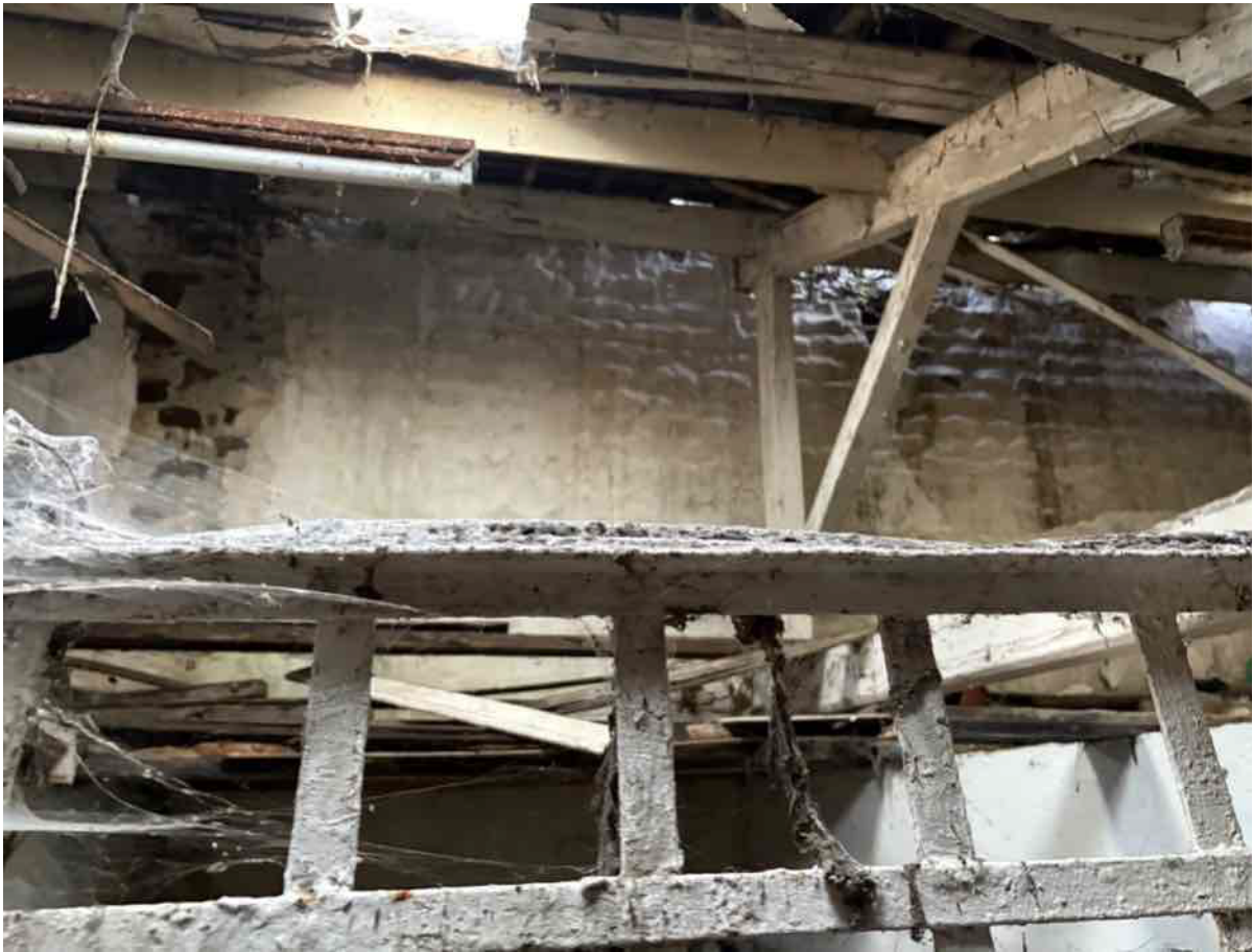
Photo 38 - Lean to stable area to south west elevation
