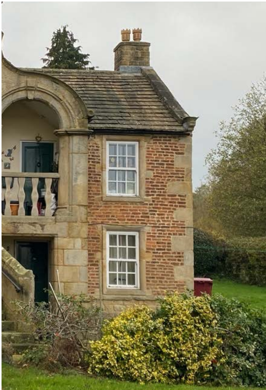
Photo 01: Front elevation brickwork
