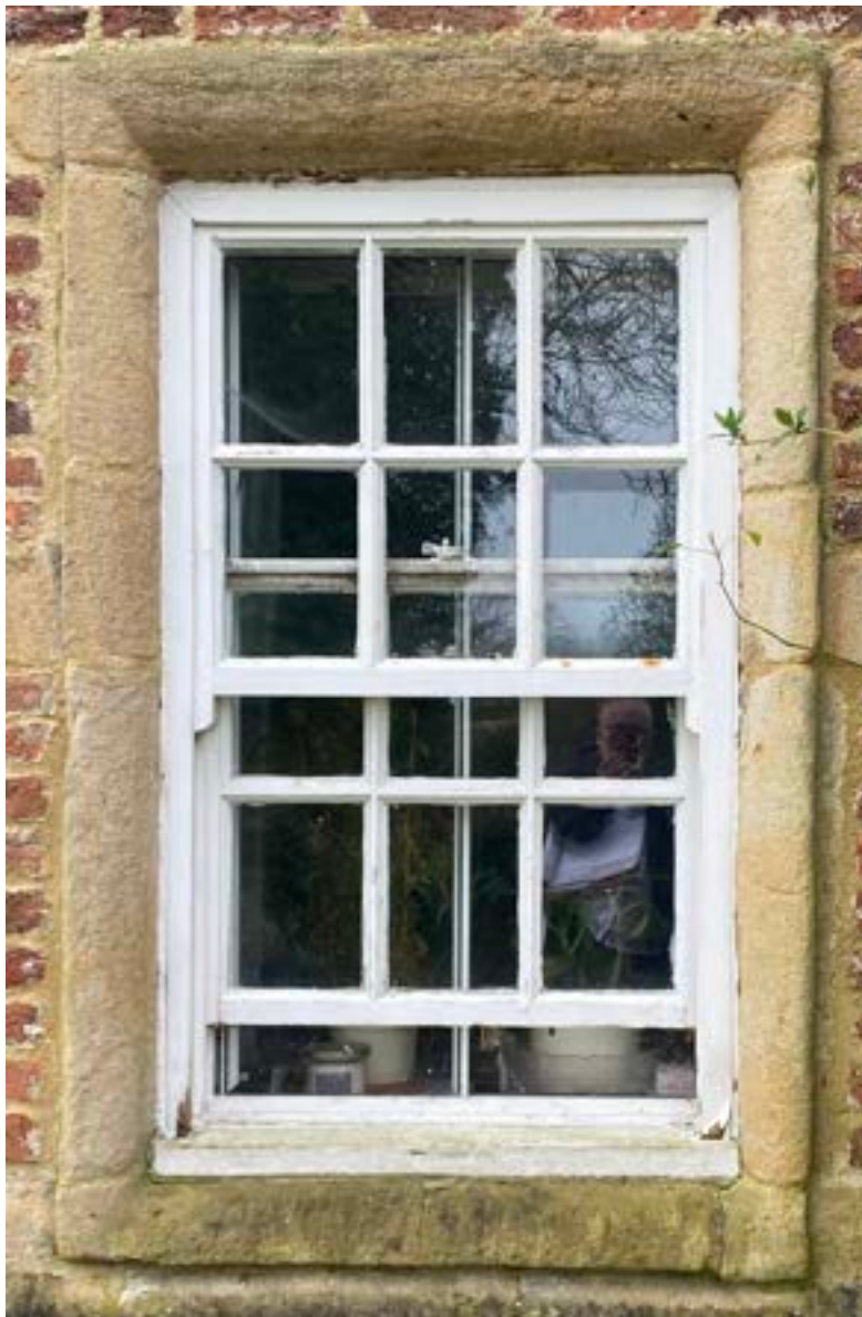
Photo 13: External view of typical Livingroom window
