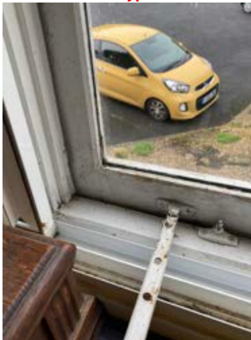
Photo 09: Typical rear elevation casement stay
