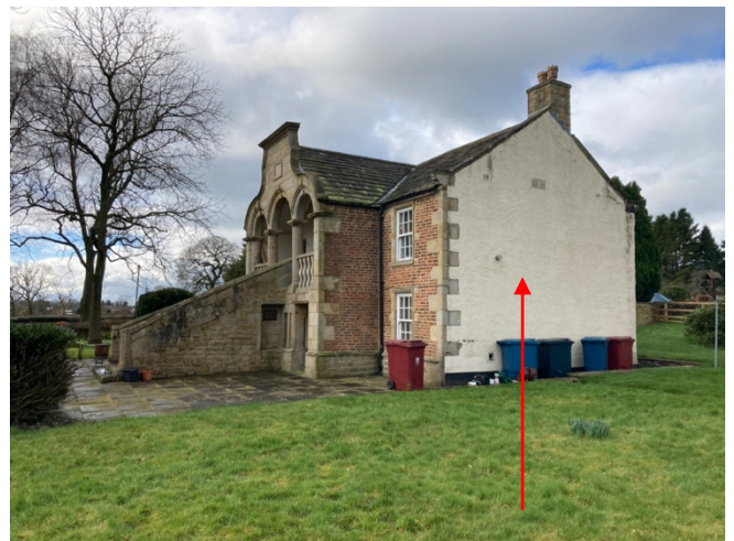
North east gable
