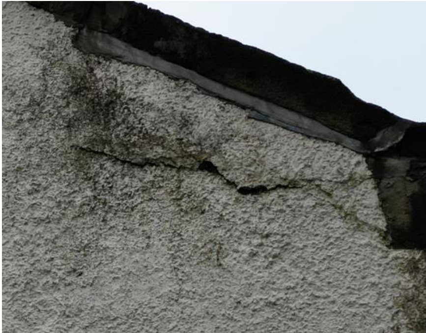
Photo 1 – Cracked render
