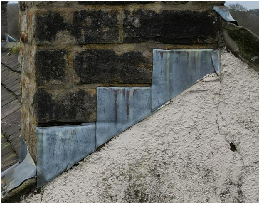
Photo 8 – Render not completely covering head of render
