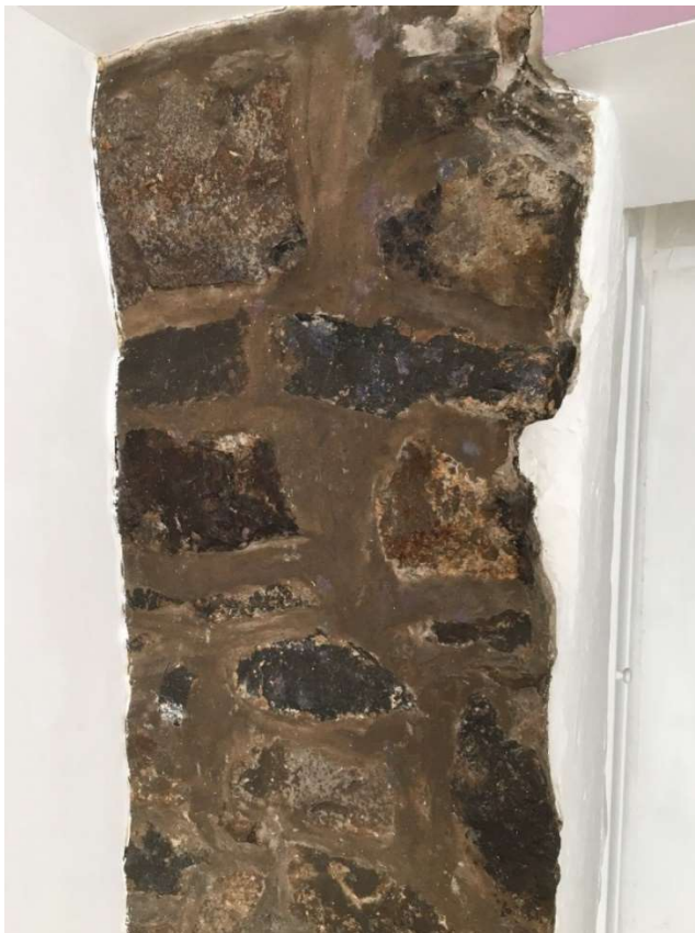
Figure 2: Photo showing a section through the width of part-exposed previously separating wall between 70 and 74 Bawdlands
