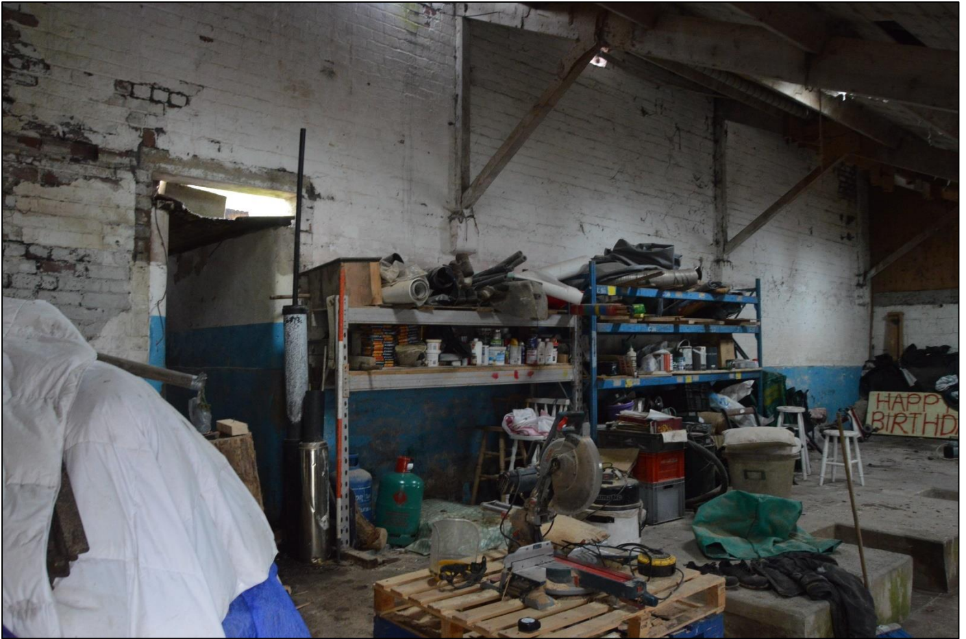
PL70: View north west within the former milking parlour [GF-08].
