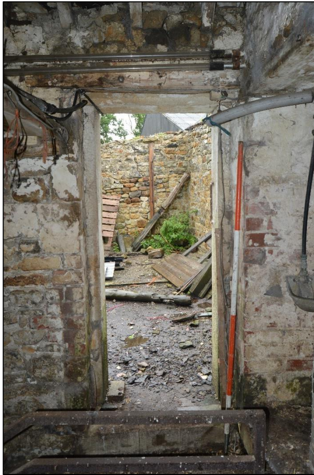
PL45: Internal view of the north doorway of the shippon [GF-03].
