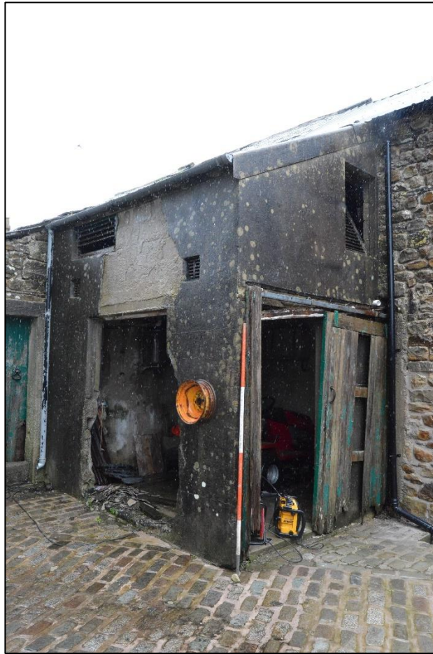
PL12: View of the modern concrete blockwork structure to the north west elevation.
