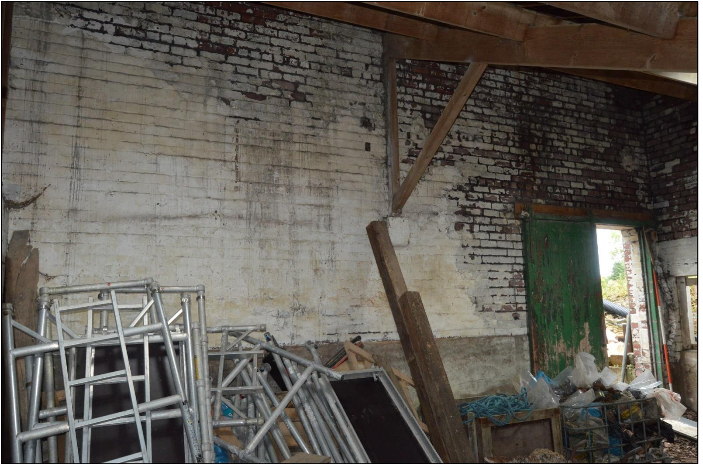
PL76: View north east within the wood store [GF-09].
