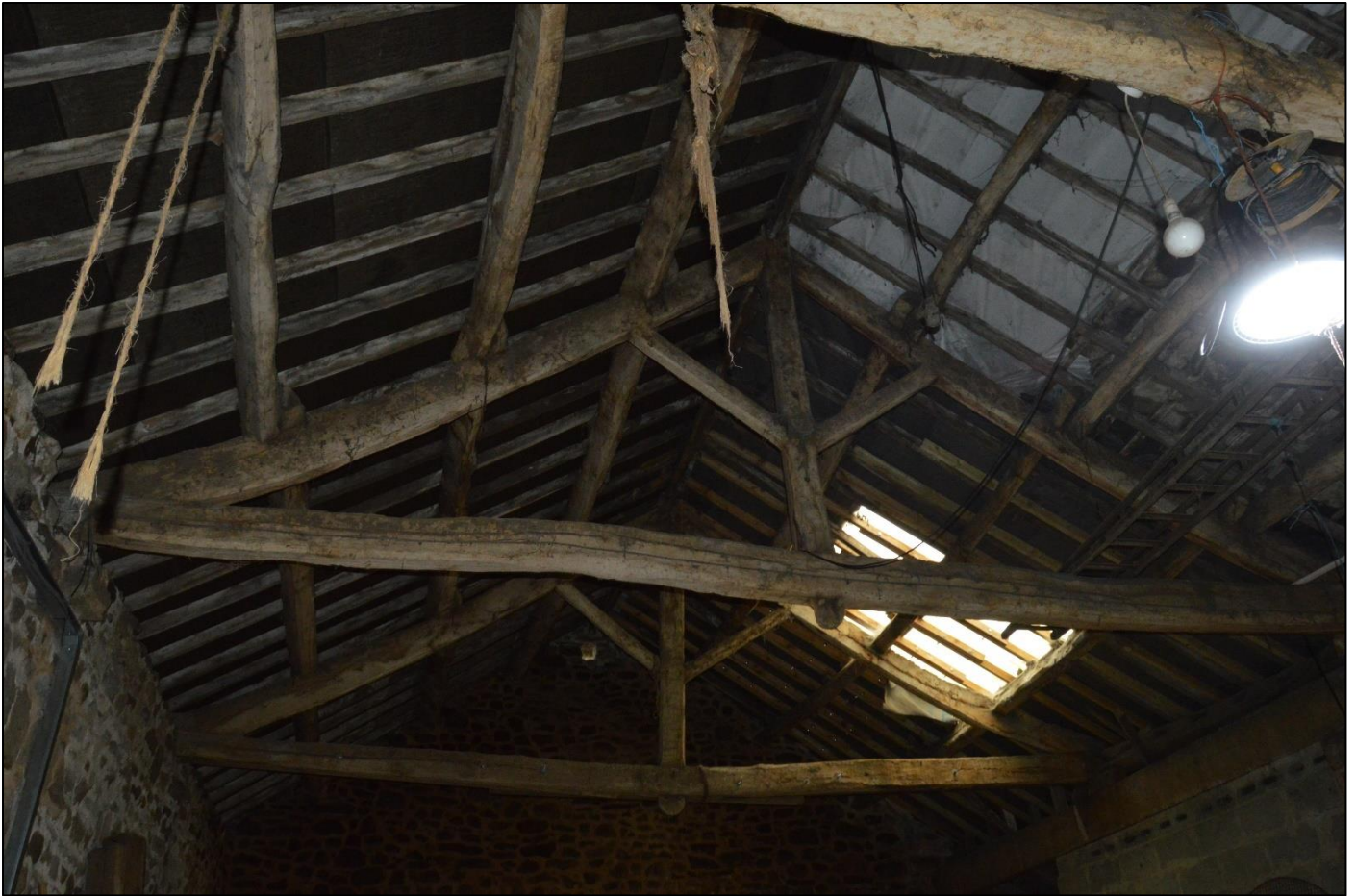
PL38: View of the timber king post roof trusses and associated roof structure preset over the south end of the barn core.
