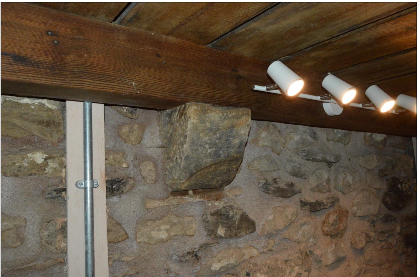
PL27: View of a stone corbel detail to the south west side of the former shippon to the south end of the barn [GF-01].
