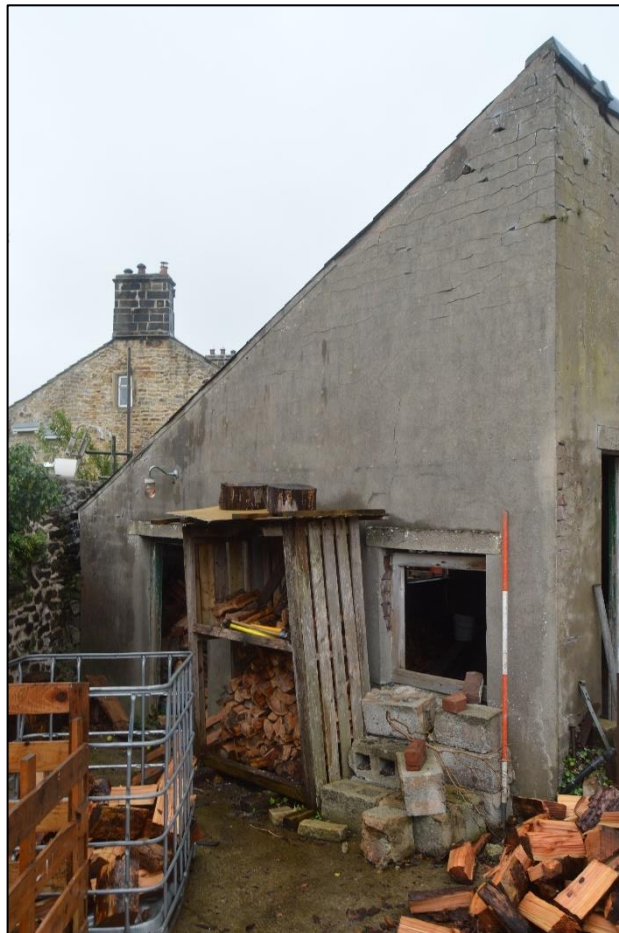
PL67: View of the east elevation of the woodstore [GF-09].
