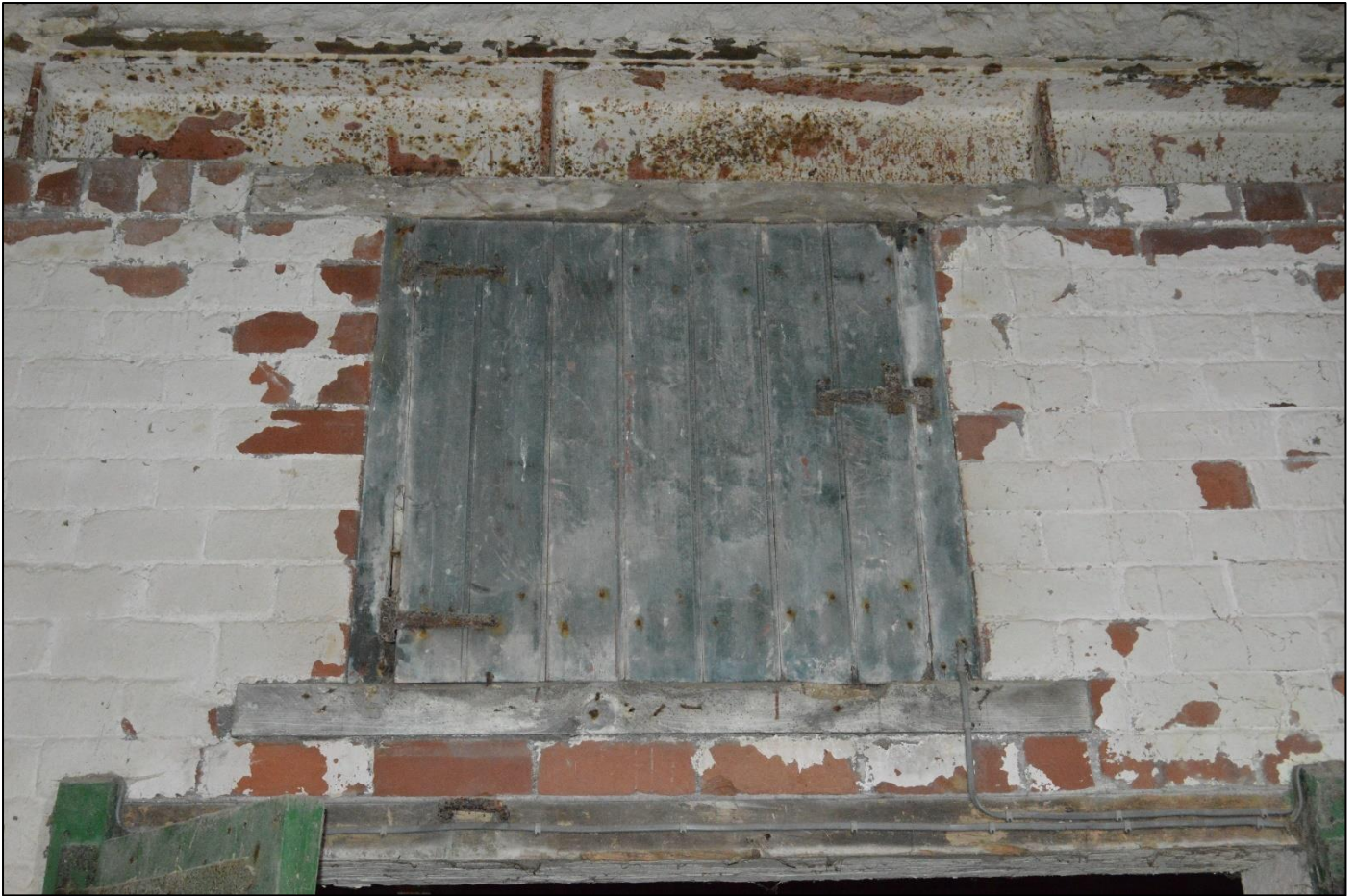
PL36: View of possible forking hole present over the doorway to the north west side of the barn core.
