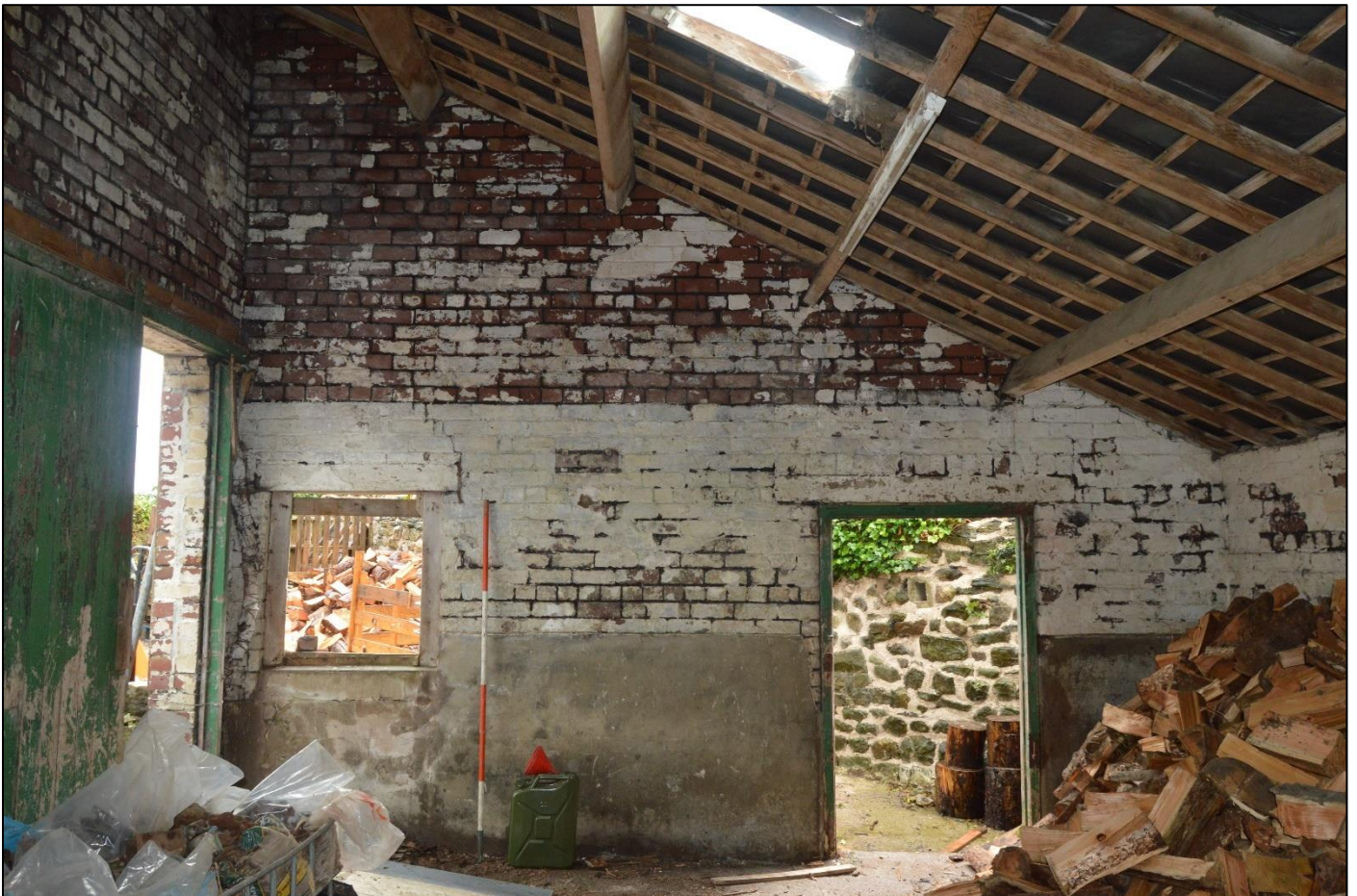
PL75: View east within the wood store [GF-09].
