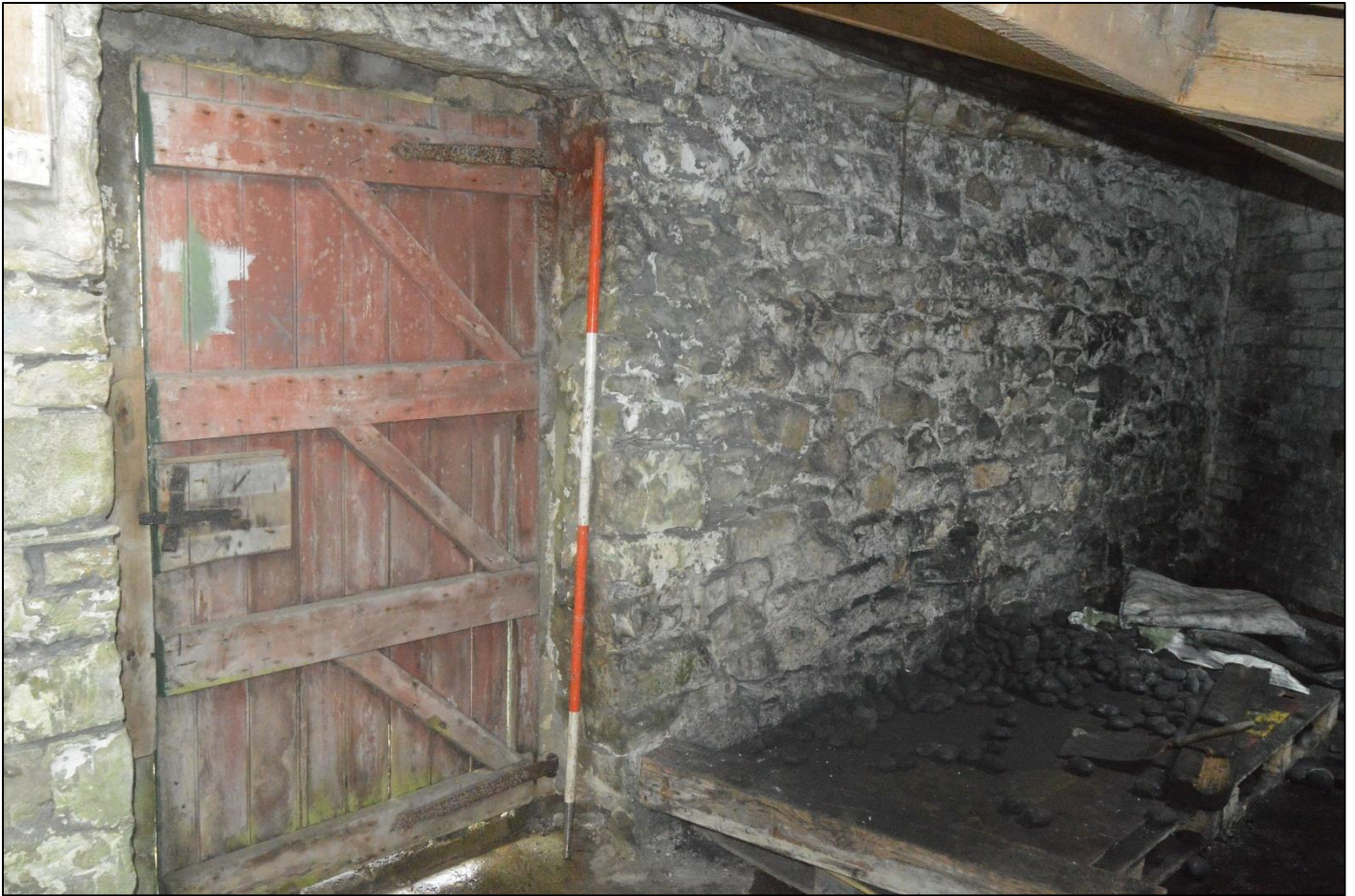
PL64: View west within the coal store [GF-10].
