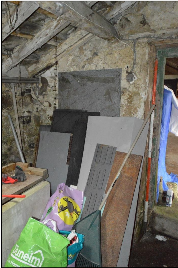
PL52 (left): View south east within store 03 [GF-07].
