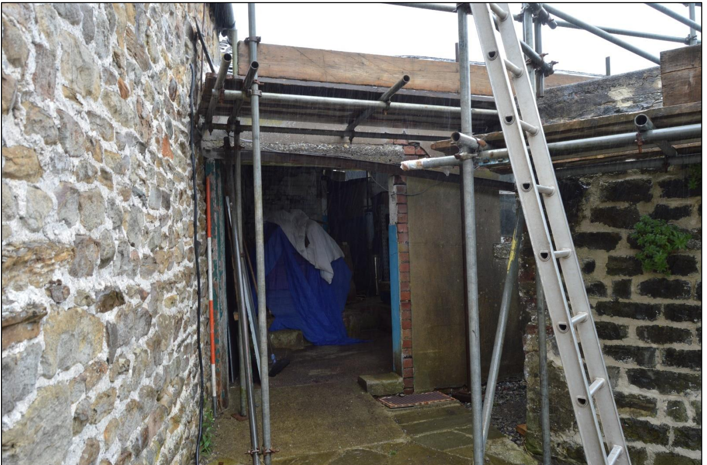
PL65: View of the external doorway to the south elevation of the former milking parlour [GF-08].
