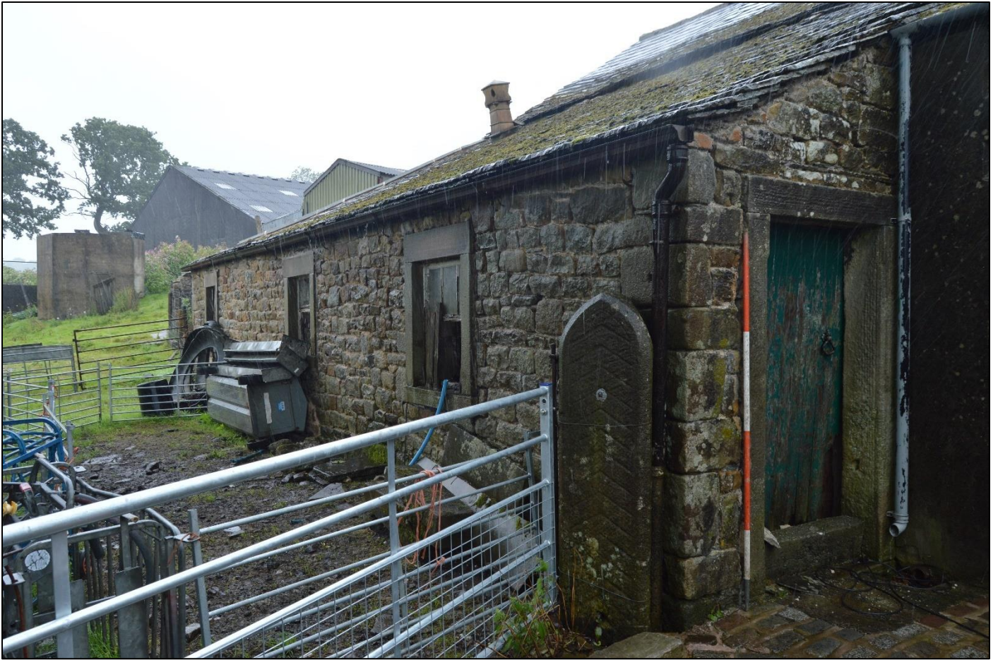
PL17: View of the shippon to the north west side of the barn from the south west.
