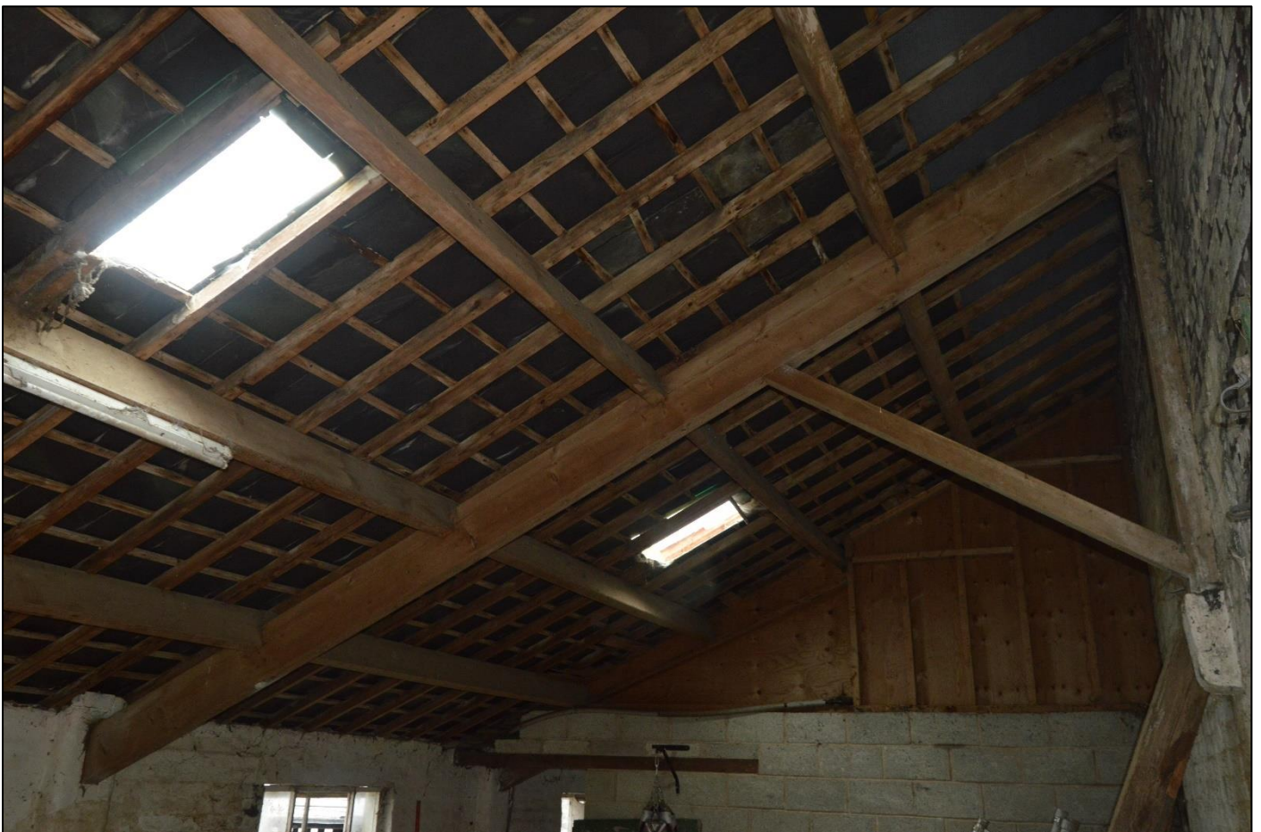
PL79: View of the timber roof structure over the wood store [GF-09].
