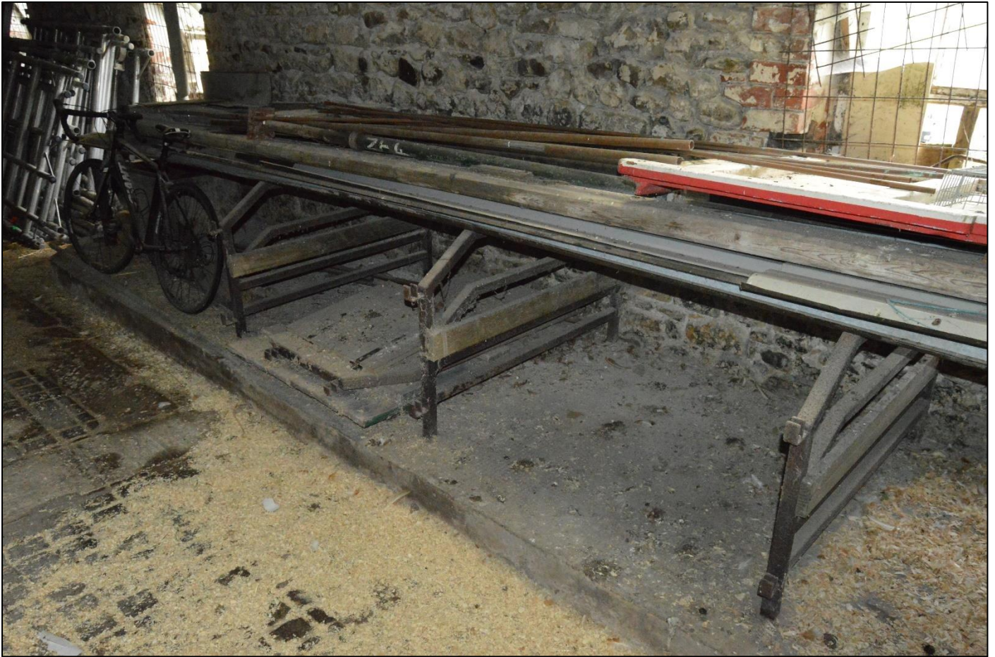
PL47: View of the stalls to the west side of the shippon [GF-03].
