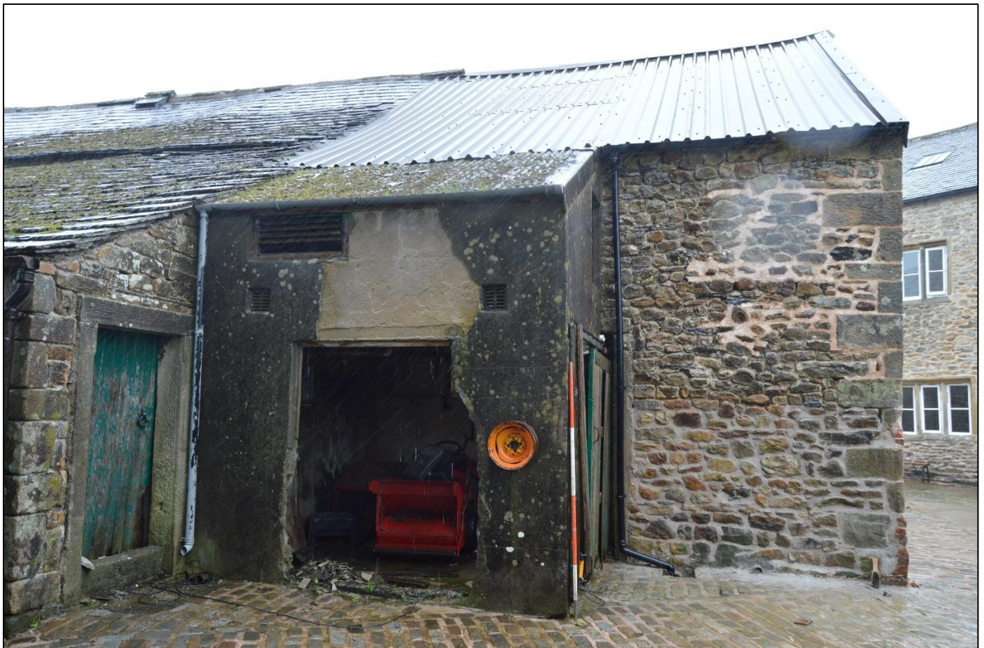
PL11: View of the south end of the north west elevation of the barn.
