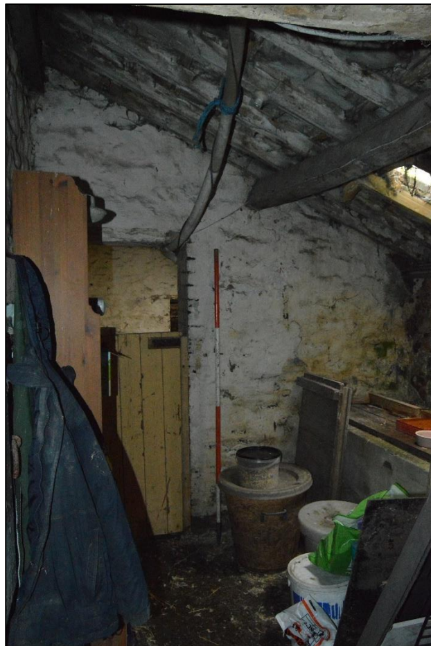
PL51: View North west within store 03 [GF-07].
