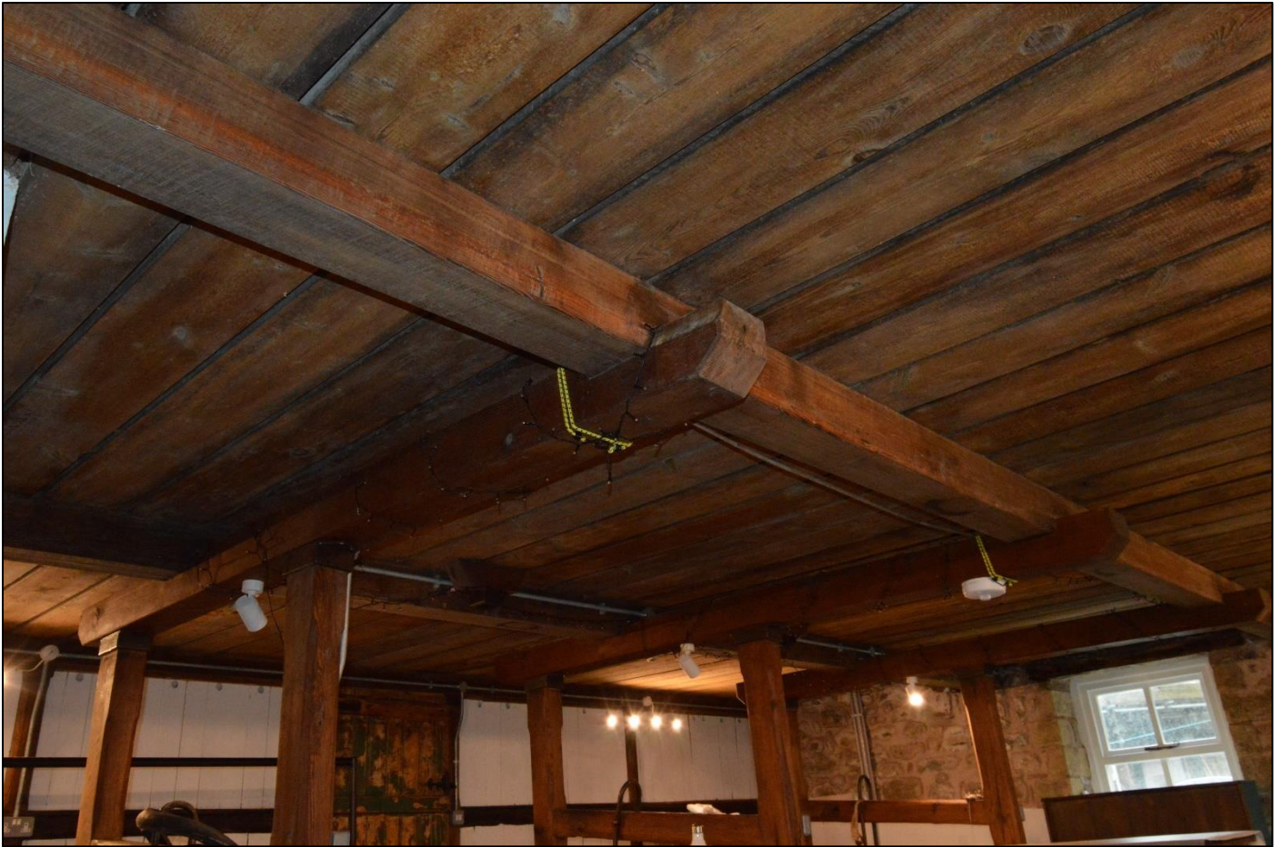
PL28: View of the floor structure over the former shippon to the south end of the barn [GF-01].
