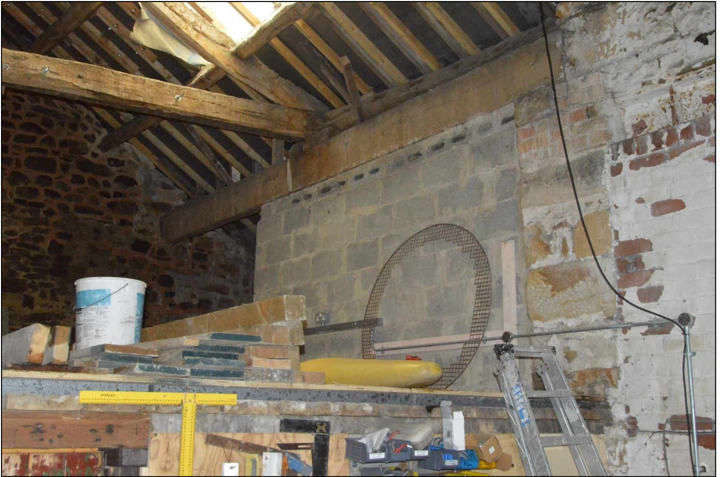
PL34: View of modern concrete blockwork present to the west side of the hay loft [FF-01].
