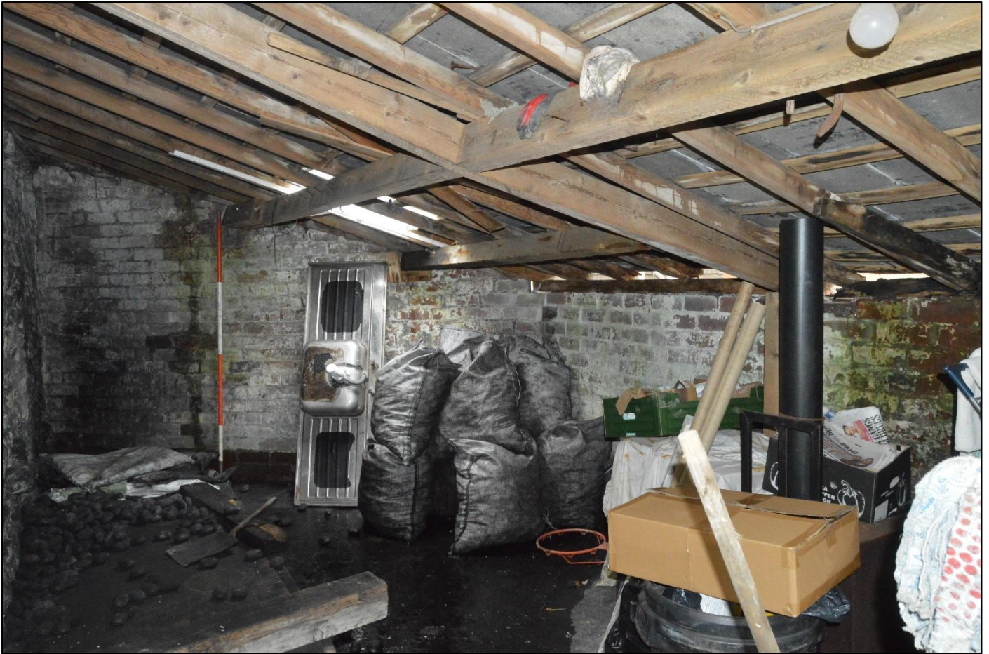
PL62: View north west within the coal store [GF-10].
