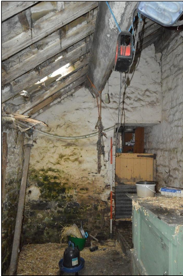
PL49 (left): View south east within store 02 [GF-06].
