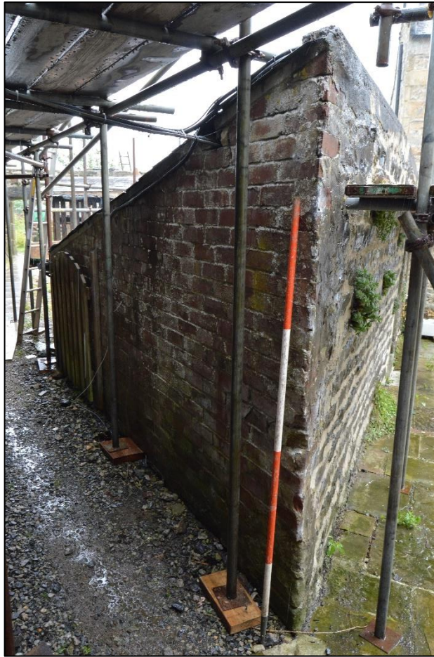
PL58: View of the coal store outbuilding from the north west.
