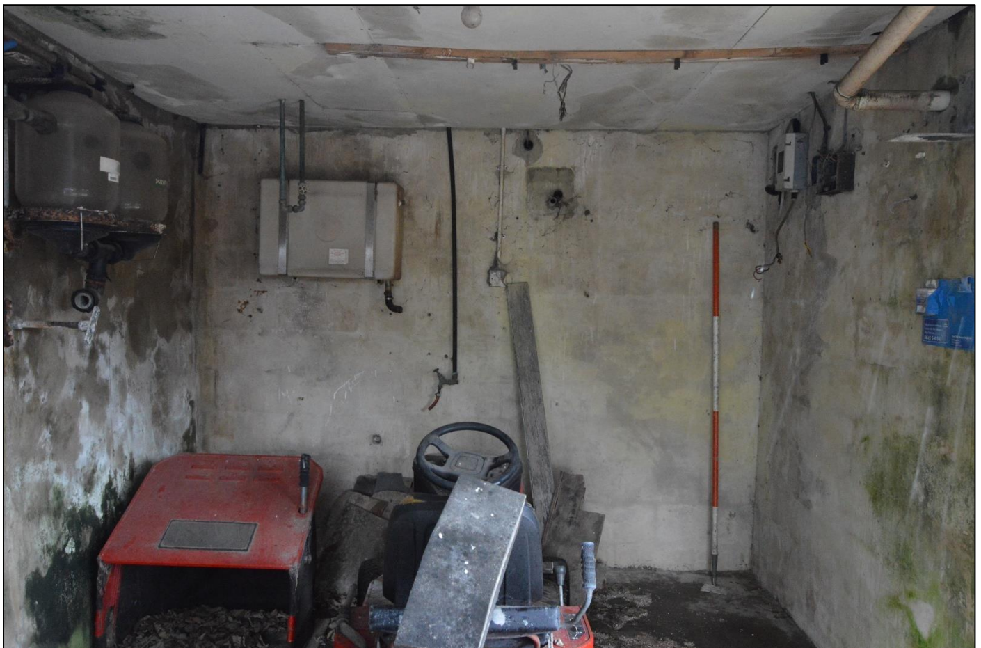
PL13: View within the modern concrete blockwork structure to the north west elevation.
