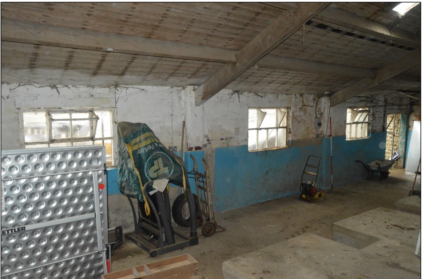
PL73: View south west within the former milking parlour [GF-08].
