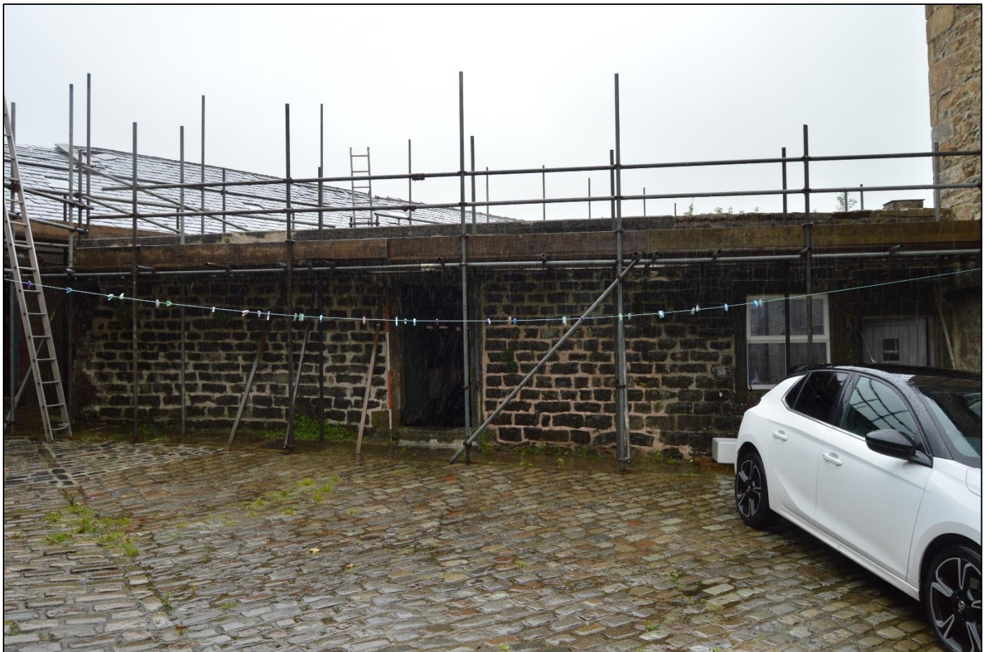
PL54: View of the south west elevation of the coal store [GF-10] and wash room [GF-11].
