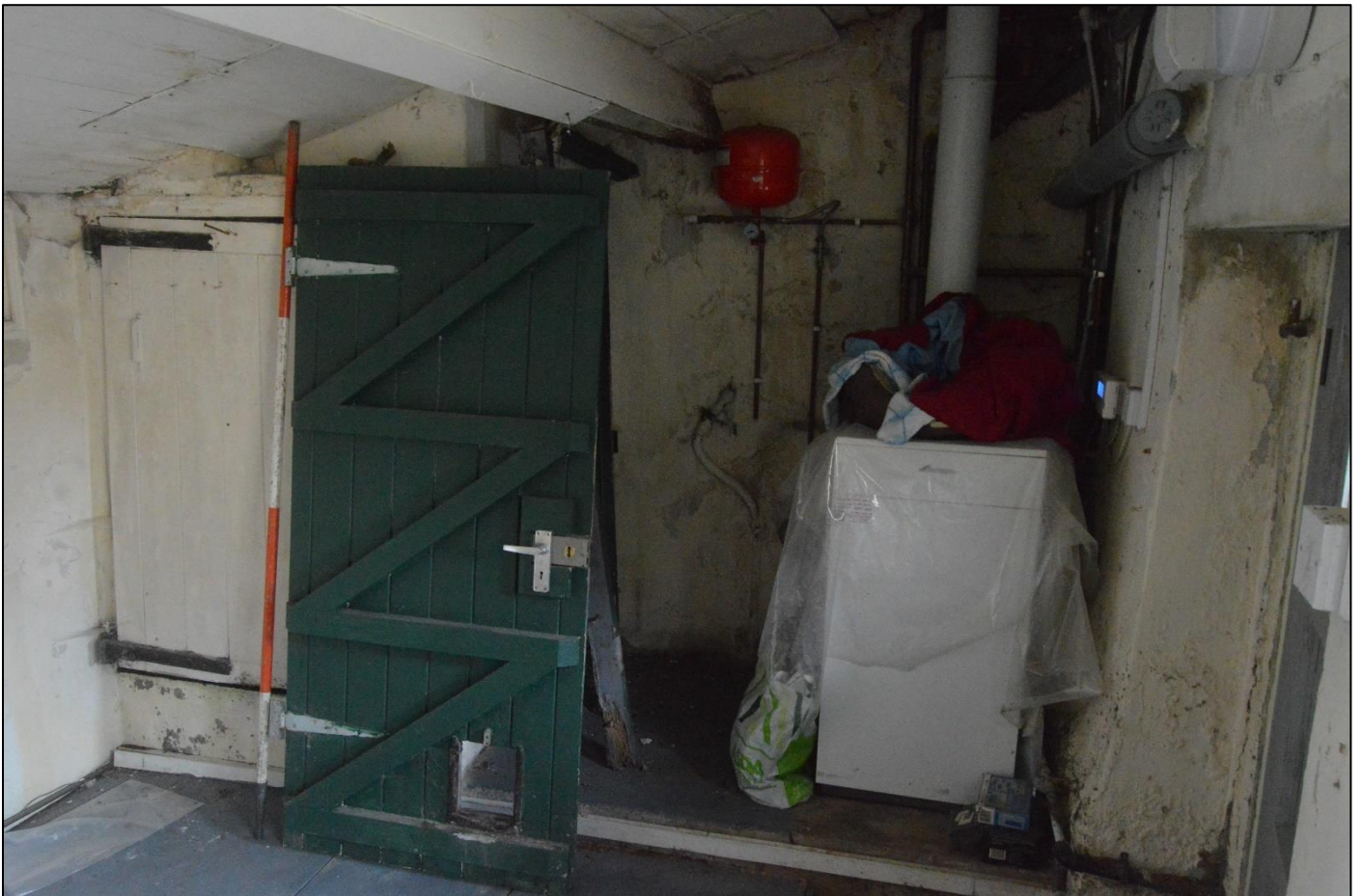
PL61: View south east within the wash house [GF-1 I].
