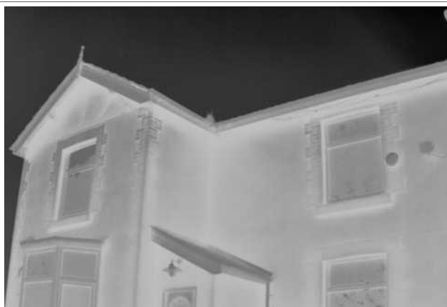
Thermal Camera Coverage
