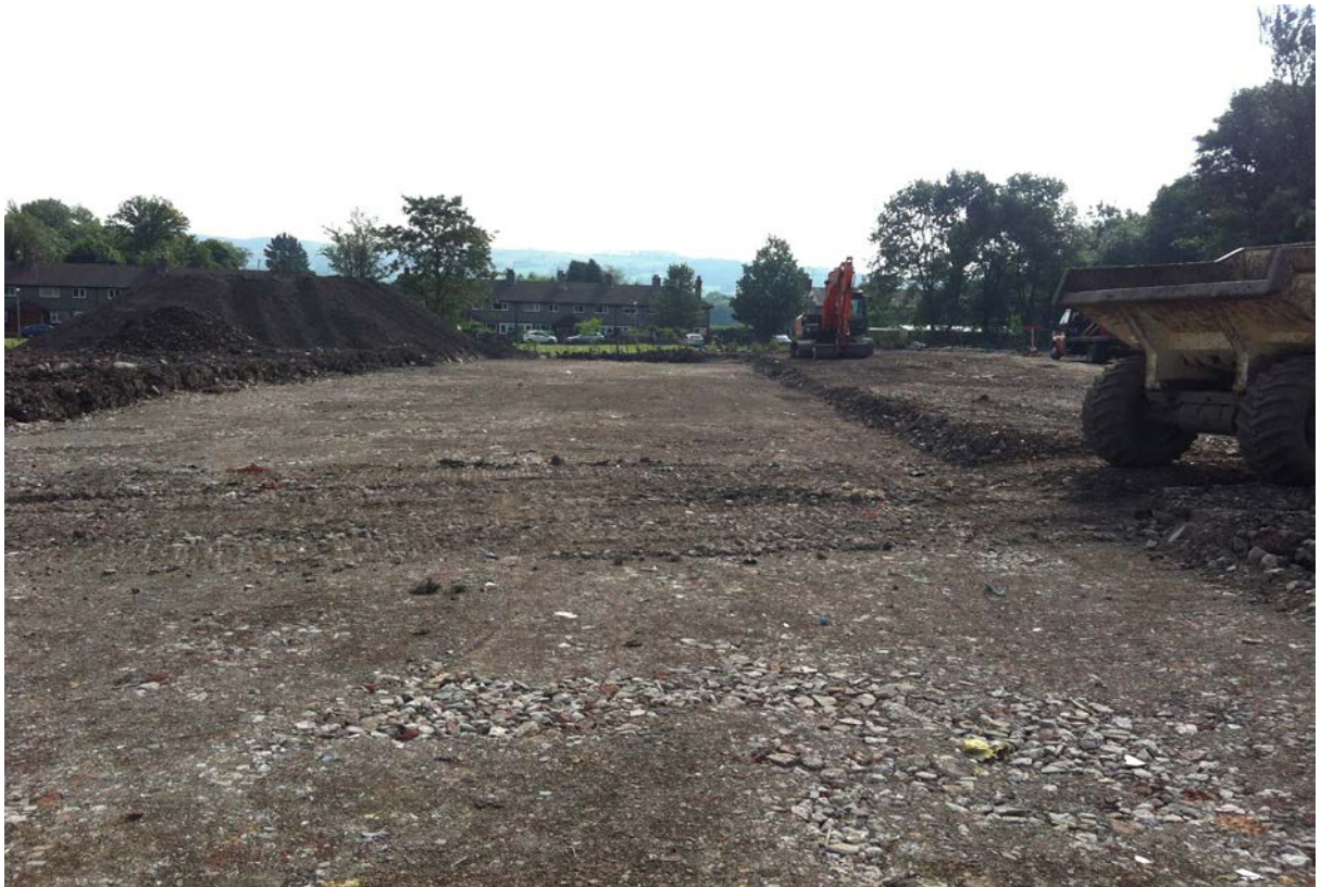
Plate 2 – Placement of Piling Matt Beneath Plot 8 to 17
