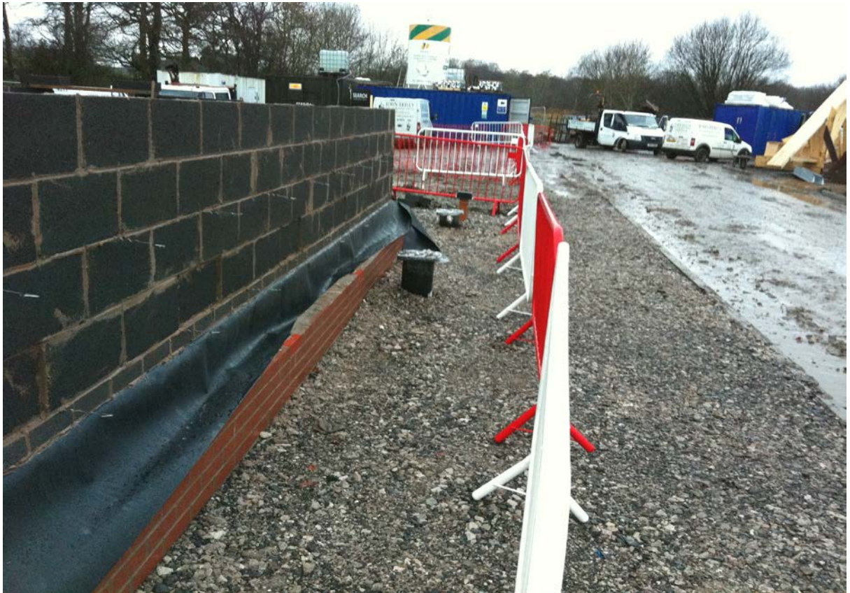
Plate 13 & 14 – Compacted 6F2 Around Plots 1 to 2
