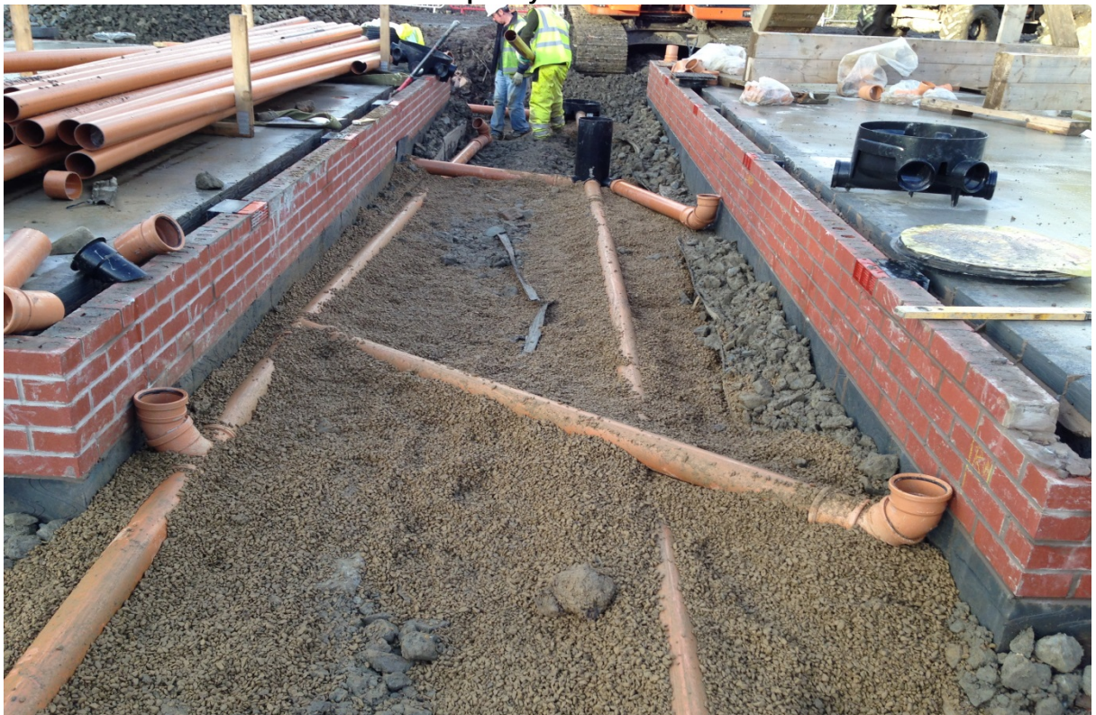
Plate 7 - Placement of 6F5 Fill materials around Plots 42 to 46
