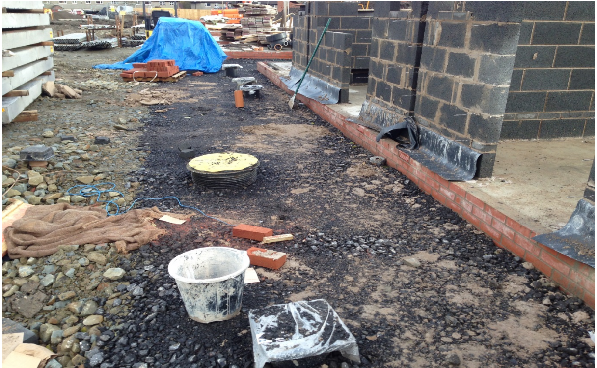
Plate 8 - Placement of 6F5 Fill materials around Plots 42 to 46
