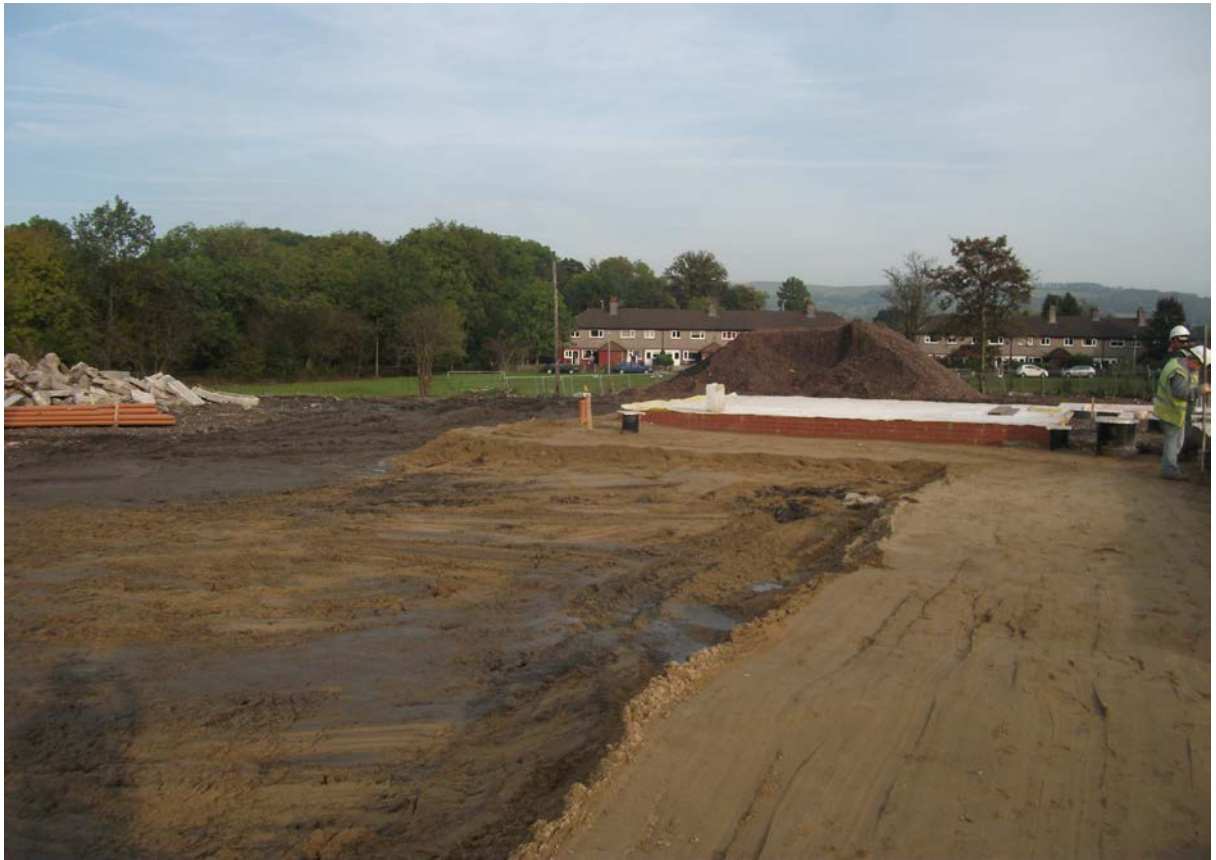
Plate 12 - Replacement of Soils Around Plots 8 to 15 with Class 2B Sand
