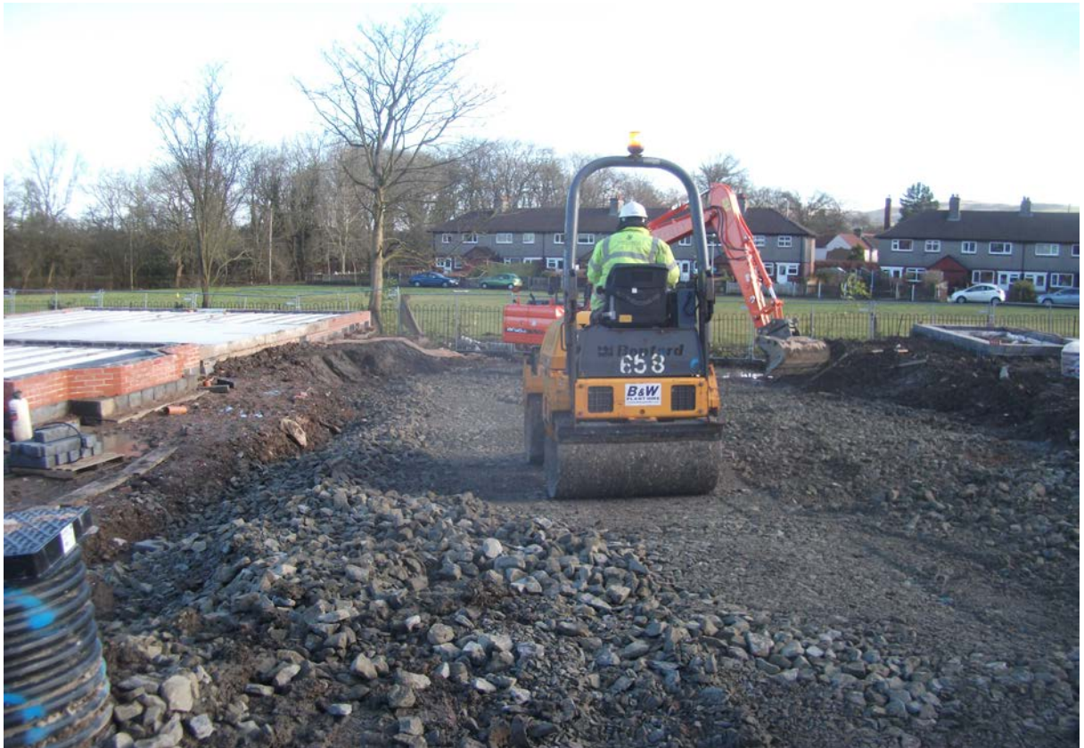
Plate 7 Removal of Soft Ground and Replacement with 6F5 Around Plots 16 to 18
