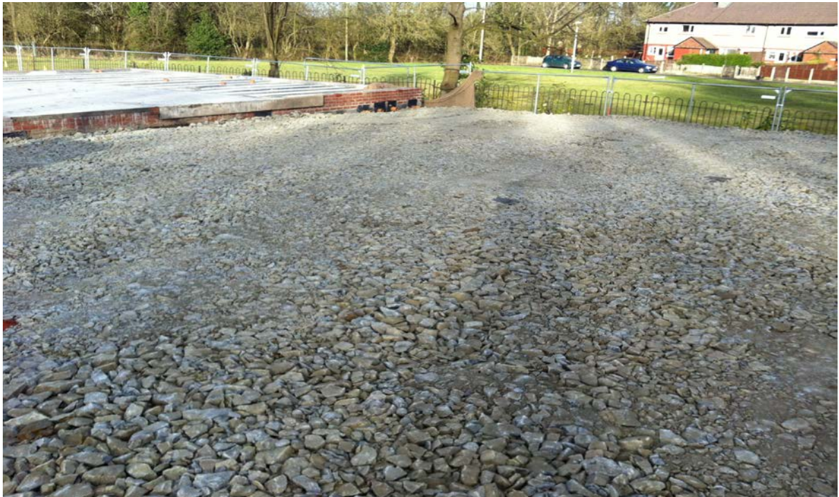
Plate 8 & 9 - Replacement of Soils Around Plots 16 to 20 with 6F5 Limestone Gravel
