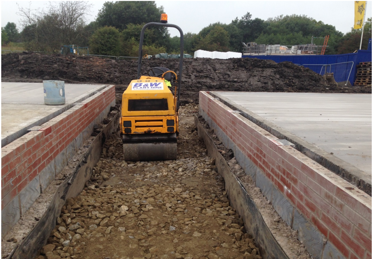
Plate 5 – Placement of 6F5 around Plots 24 to 29
