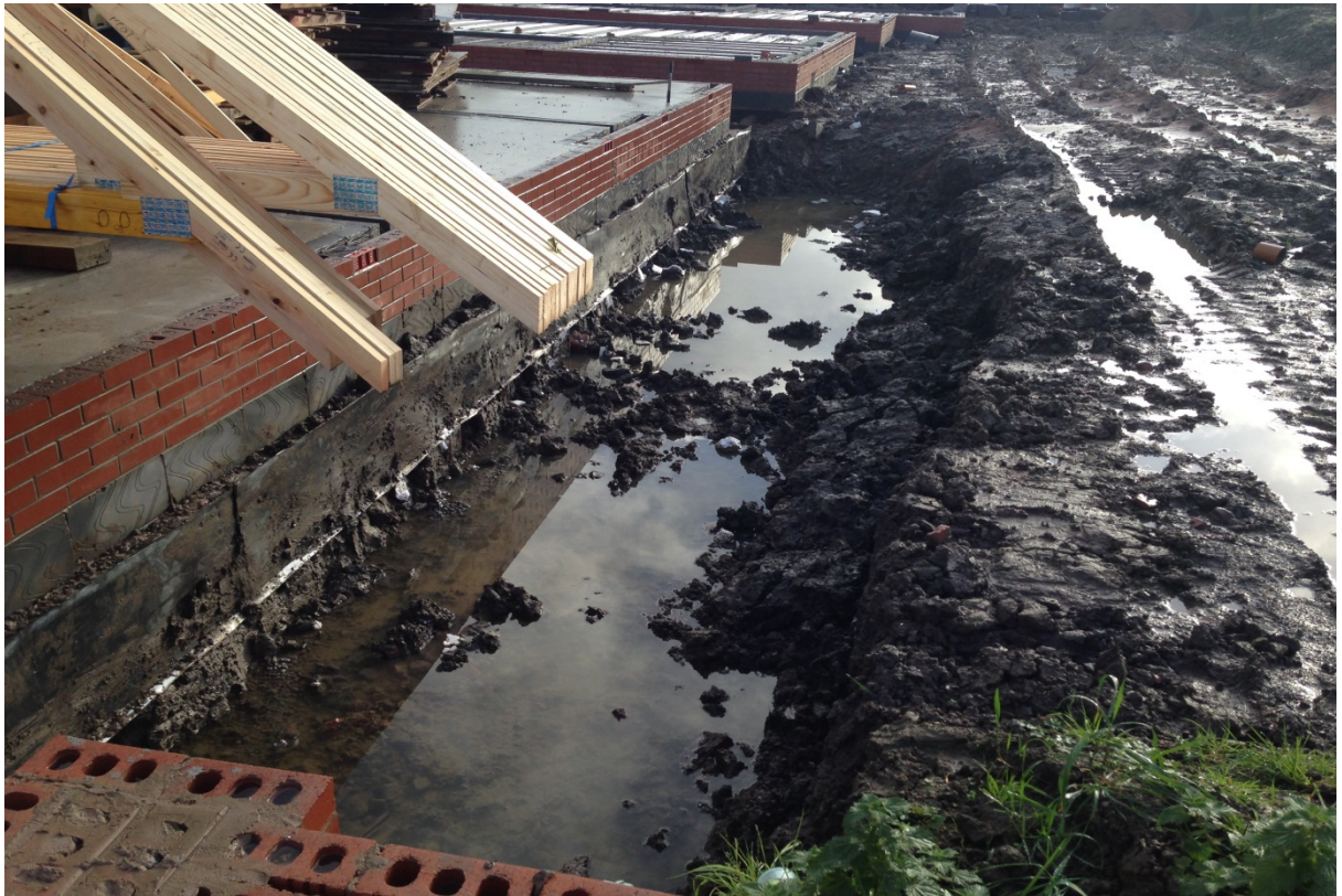
Plate 6 – Excavation of Temporary Fill materials around Plots 42 to 46
