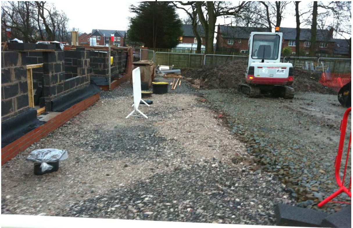
Plate 13 – Compacted 6F2 & 6f5 Around Plots 1 to 5
