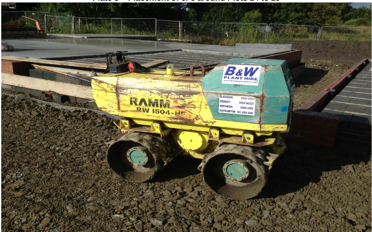
Plate 4 – Placement of 6F5 around Plots 24 to 29
