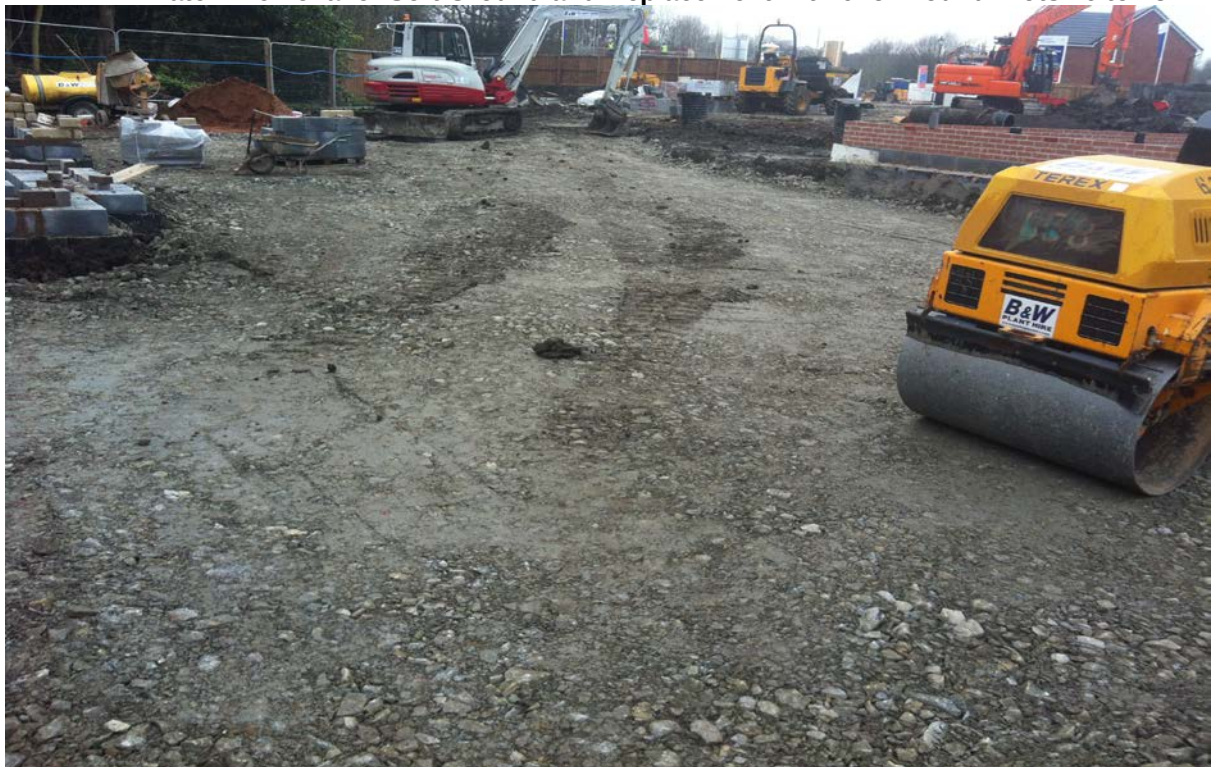
Plate 7 – Replacement of Soils Around Plots 16 to 20 with 6F5 Limestone Gravel
