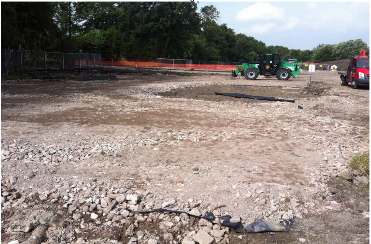
Plate 4 – Piling Matt Placement & Membrane Beneath Plots 20 to 23
