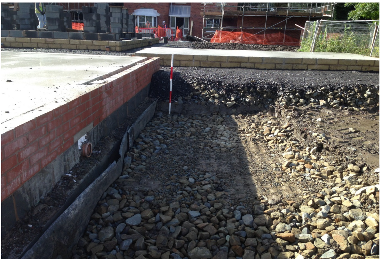
Plate 2 – Placement of 6F5 Around Plots 24 to 29
