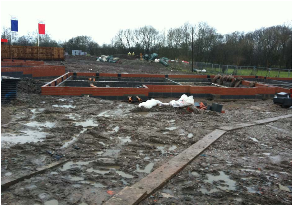
Plate 5 – Plot 18 Class 2A/2B ‘wet’ Soils Removed to be removed and Replaced with 6F5
