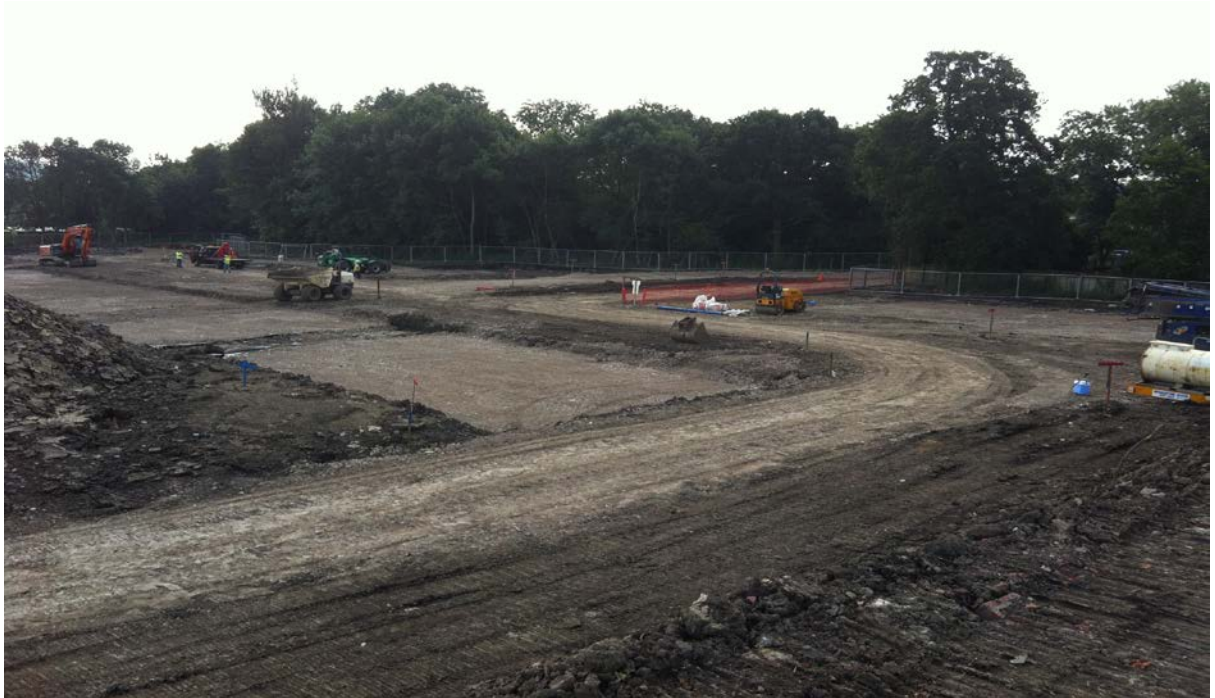
Plate 1 Placement of Piling Mats beneath Plots 1 to 23
