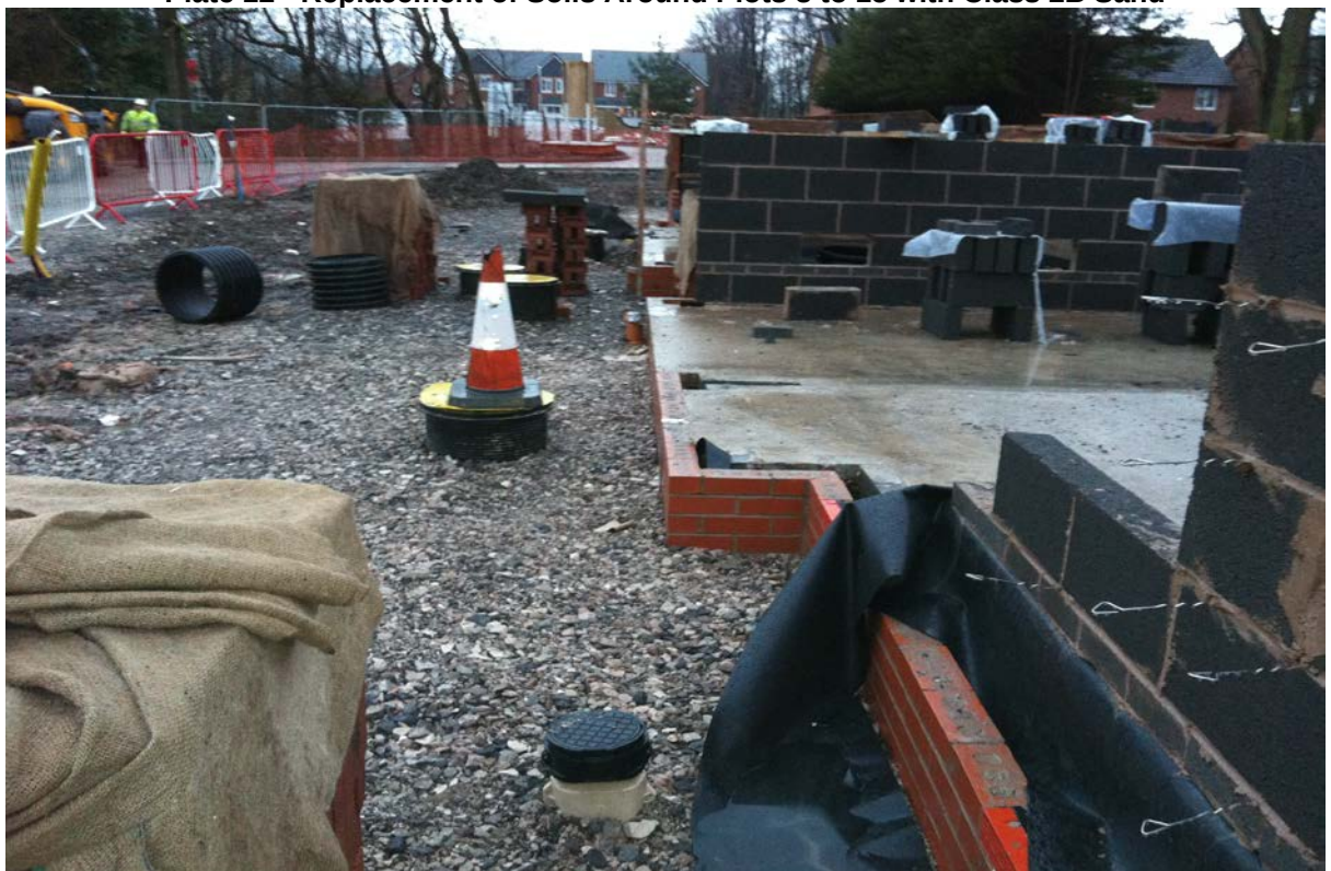
Plate 12 – Compacted 6F2 Around Plots 1 to 2
