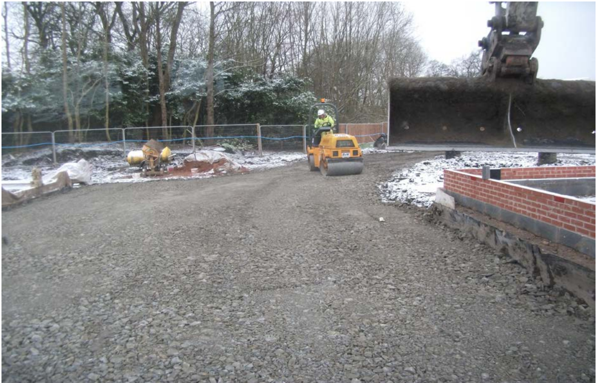
Plate 10 - Replacement of Soils Around Plots 19 & 20 with 6F5 Limestone Gravel
