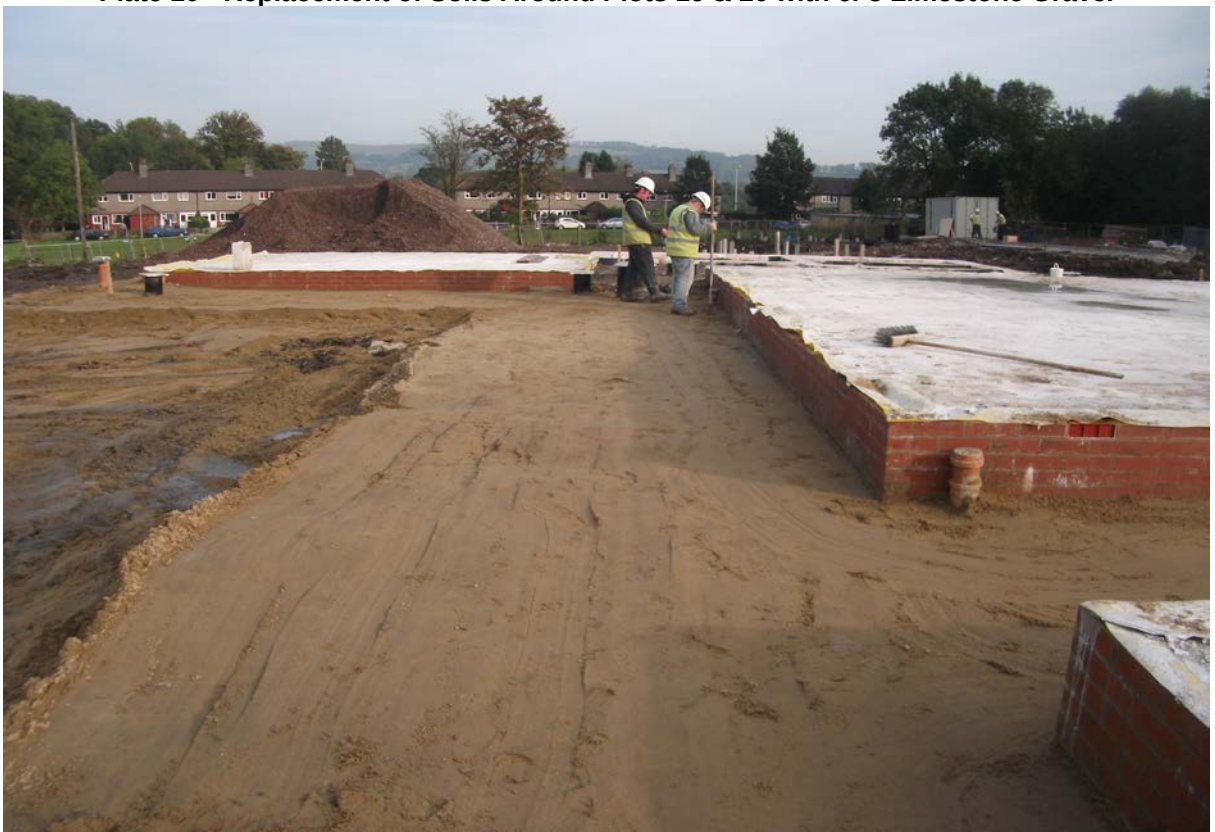
Plate 11 - Replacement of Soils Around Plots 8 to 15 with Class 2B Sand
