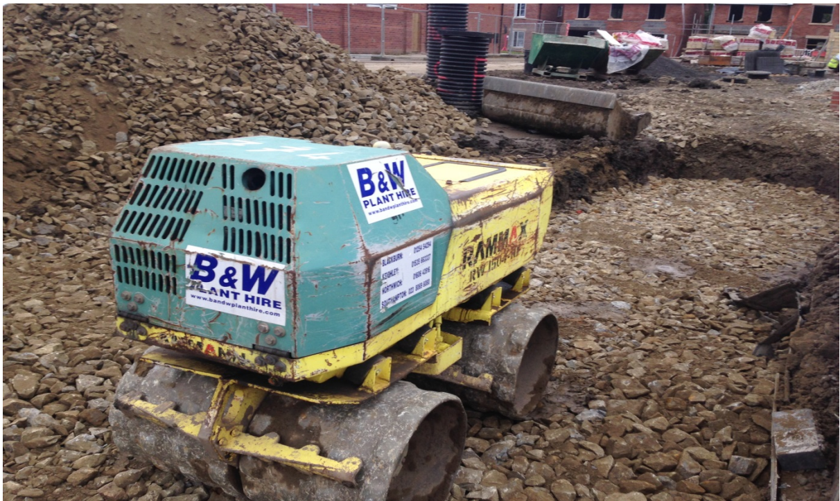
Plate 3 – Placement of 6F5 around Plots 24 to 29
