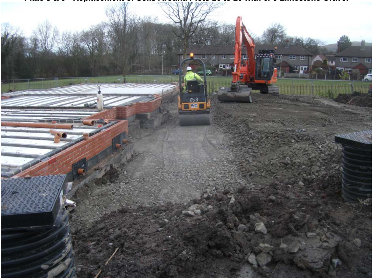
Plate 8 & 9 - Replacement of Soils Around Plots 16 to 20 with 6F5 Limestone Gravel
