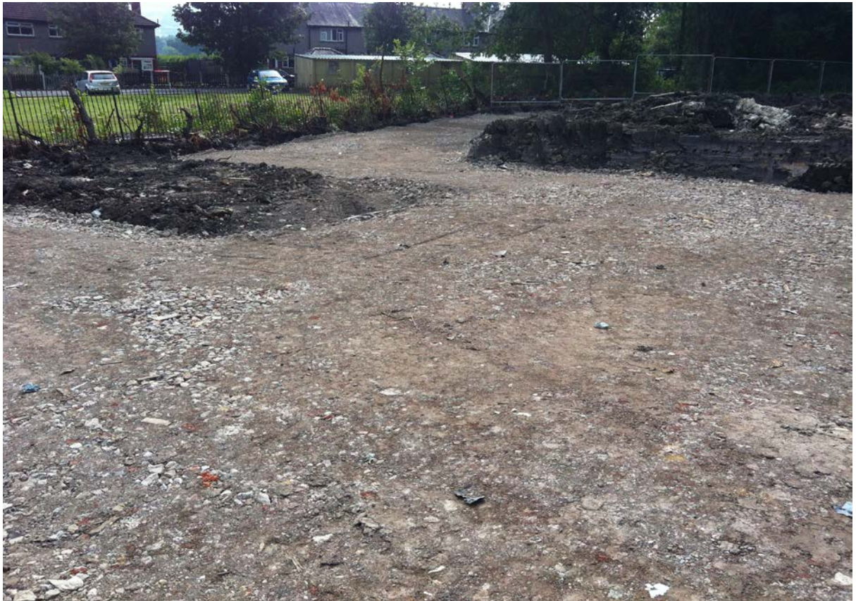
Plate 3 – Reduced Levels & Piling Mats Beneath Plots 16 & 18
