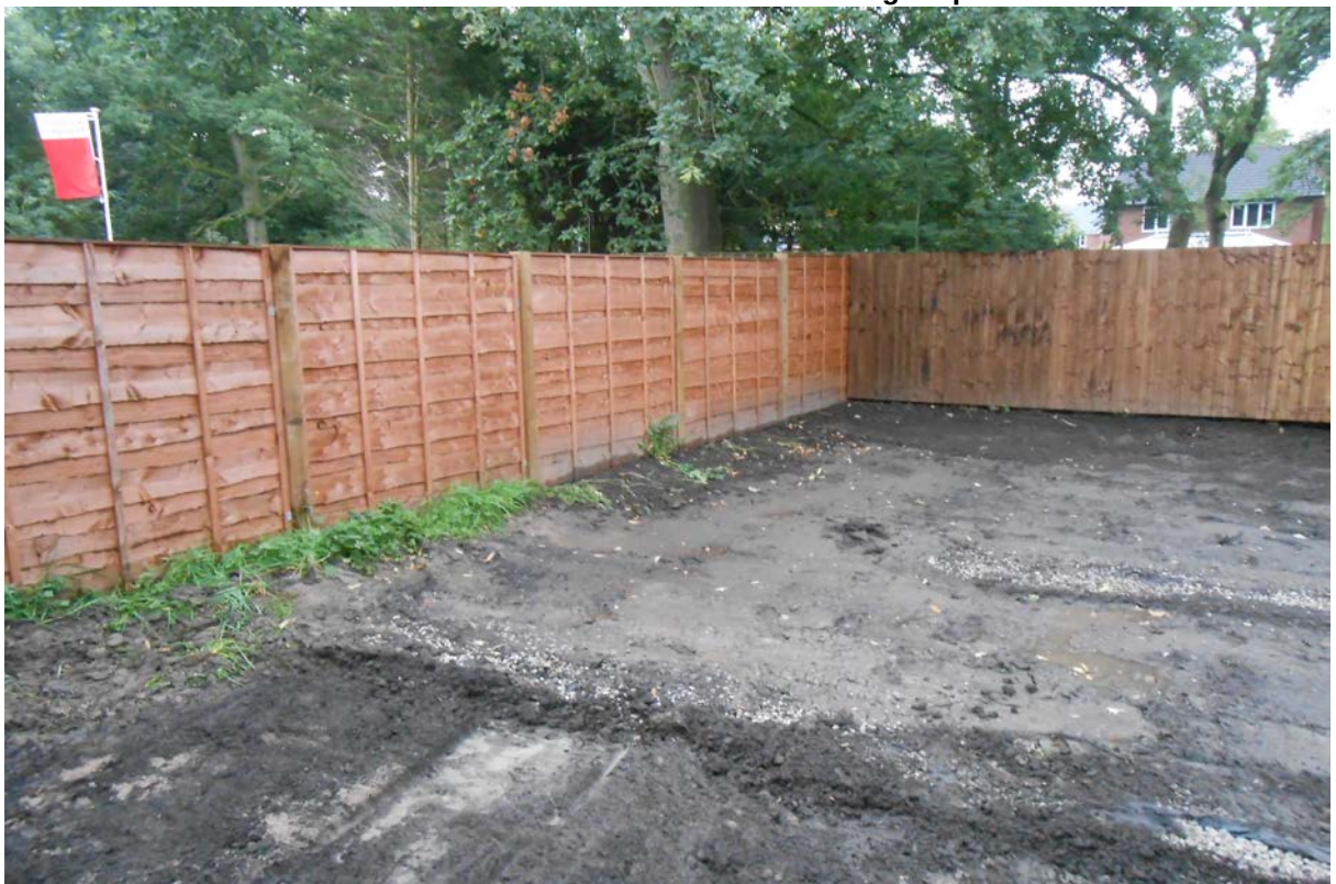
Plate 2 – Removal of Blackledge unsuitable topsoil
