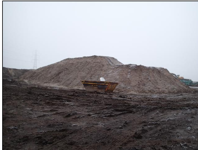
Photograph 4: Showing the Taylor Wimpey Topsoil during inspection. Photograph taken on 12 December 2012.
