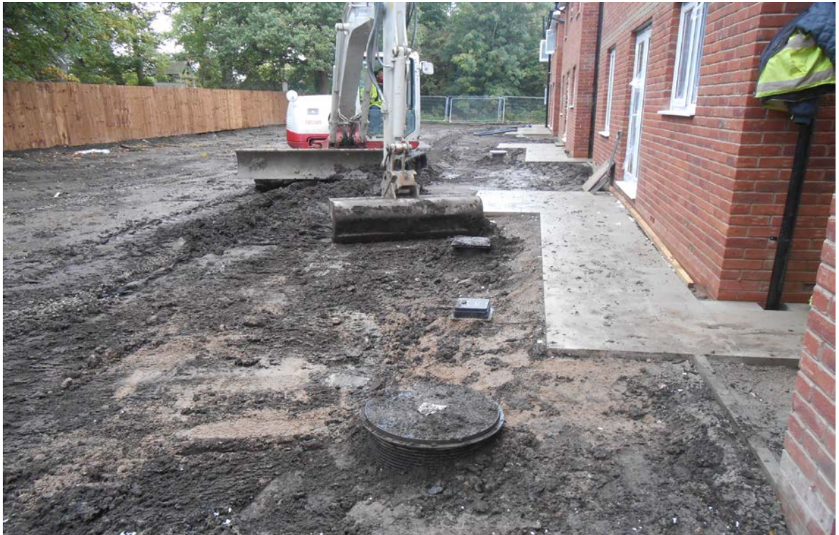
Plate 1 – Removal of unsuitable Blackledge topsoil
