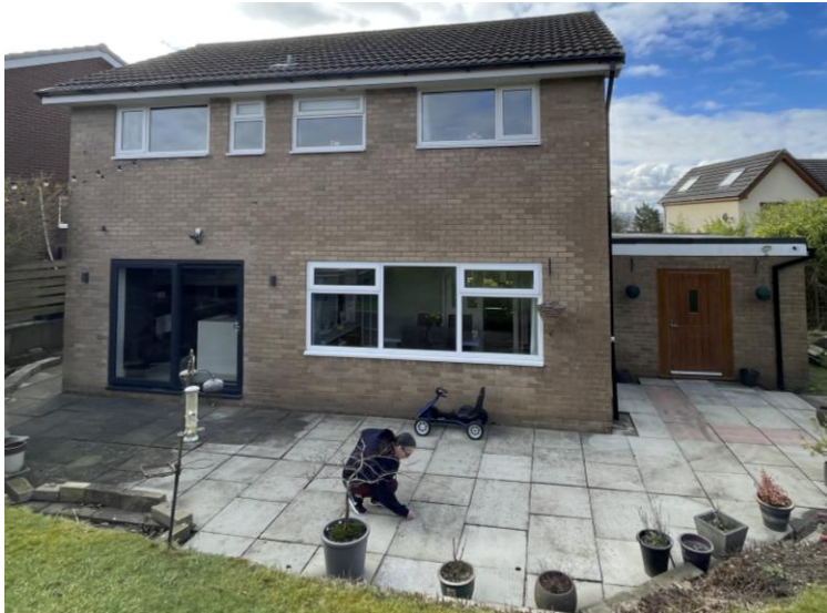
Rear Northeast Elevation of House and Garage
