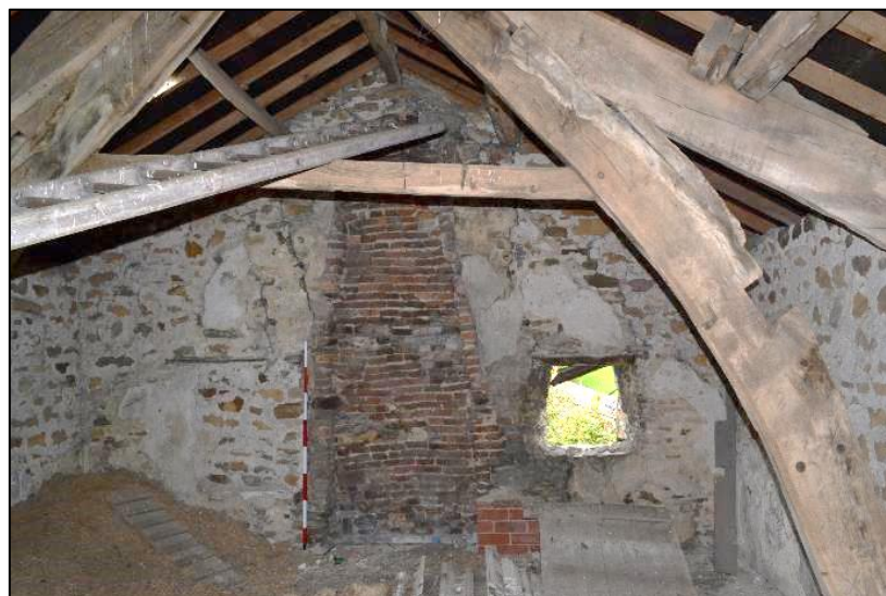
Plate 12. First floor. West elevation interior (scale 1.6m)
