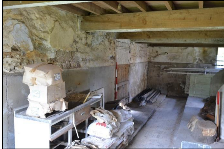
Plate 16. Ground floor general shot (scale 1.6m)
