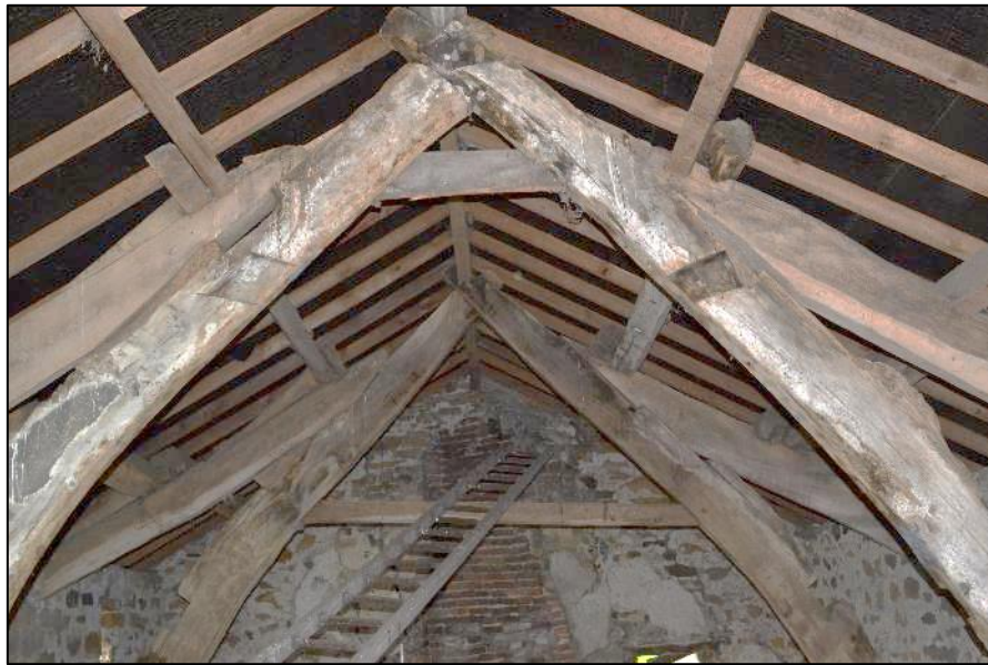
Plate 21. Detail of crucks and other roof timbers
