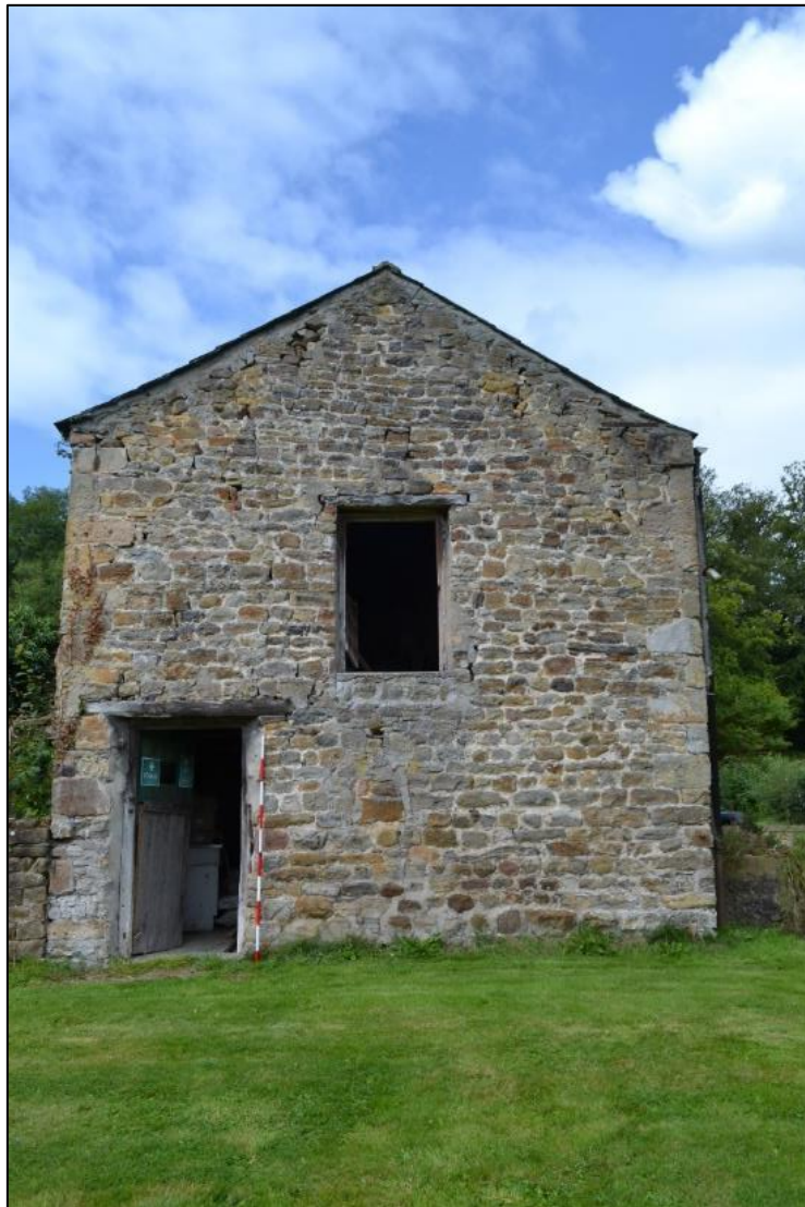
Plate 9. The east elevation (scale 2m)
