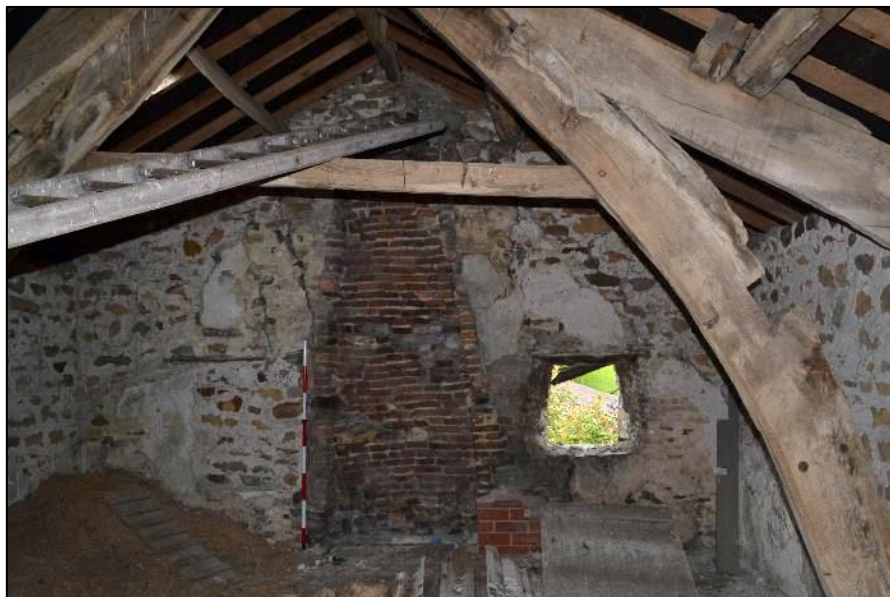
Plate 19. General shot first floor. Looking west (scale 1.6m)
