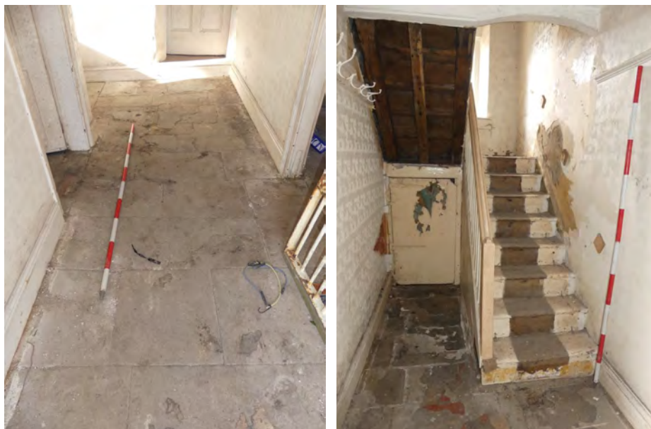
Plate 45 (left): Floor in G5 (farmhouse), viewed from the south-east
