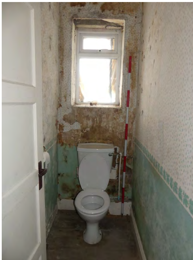
Plate 91: Window to the south-east in F5 (farmhouse), viewed from the north-east
