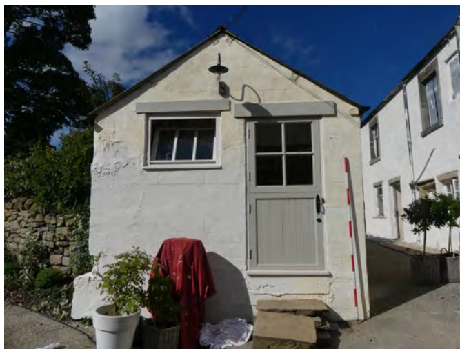
Plate 207: The south-east elevation of the outbuilding, viewed from the south-east
