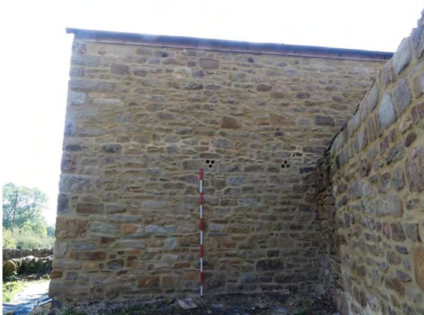
Plate 160: Main part of the north-west external elevation of the barn, viewed from the north-west
