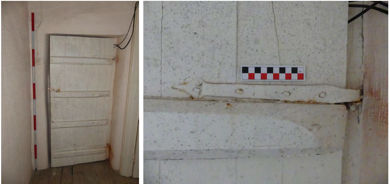
Plate 87 (left): Door to the south-east in F4 (farmhouse), viewed from the north-west
