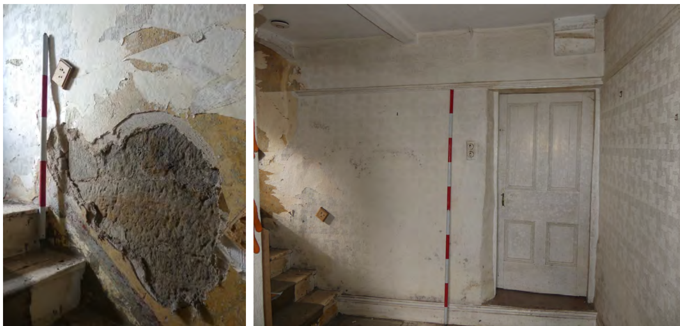
Plate 49 (left): Butt in north-west wall of G5 (farmhouse), viewed from the east
