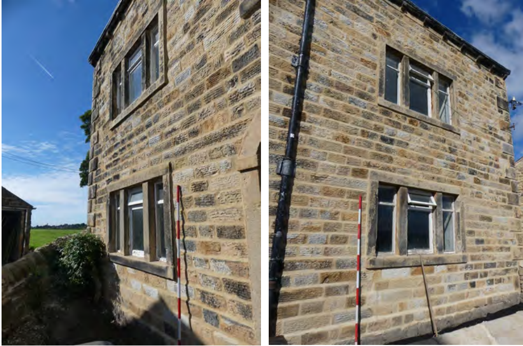
Plate 11 (left): South-west windows on the south-east external elevation of the farmhouse, viewed from the east
