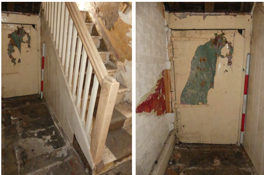
Plate 47 (left): Side of the stairs in G5 (farmhouse), viewed from the east
