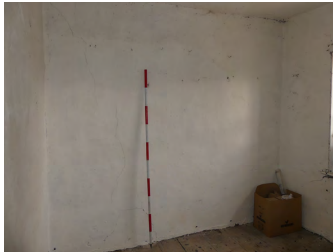
Plate 82: North-west elevation of F2 (farmhouse), viewed from the south-east
