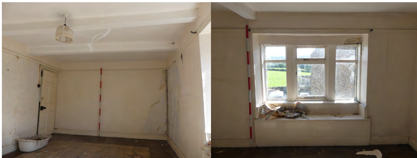
Plate 109 (left): North-east end of F8 (farmhouse), viewed from the south-west
