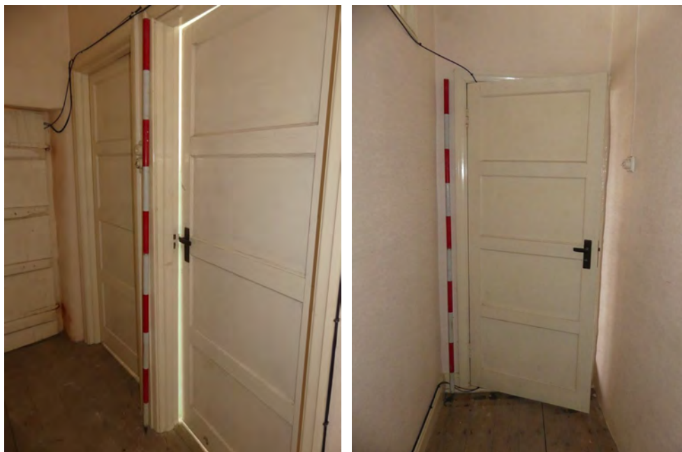
Plate 89 (left): Doors to the south-west in F4 (farmhouse), viewed from the north
