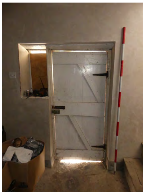
Plate 32: Door to the north-east in G2 (farmhouse), viewed from the south-west
