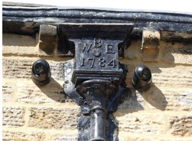
Plate 17: Hopper, viewed from the south-east
