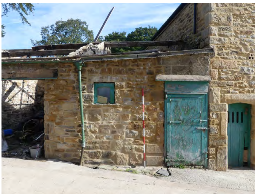
Plate 163: Centre of the south-west external elevation of the barn, viewed from the south-west
