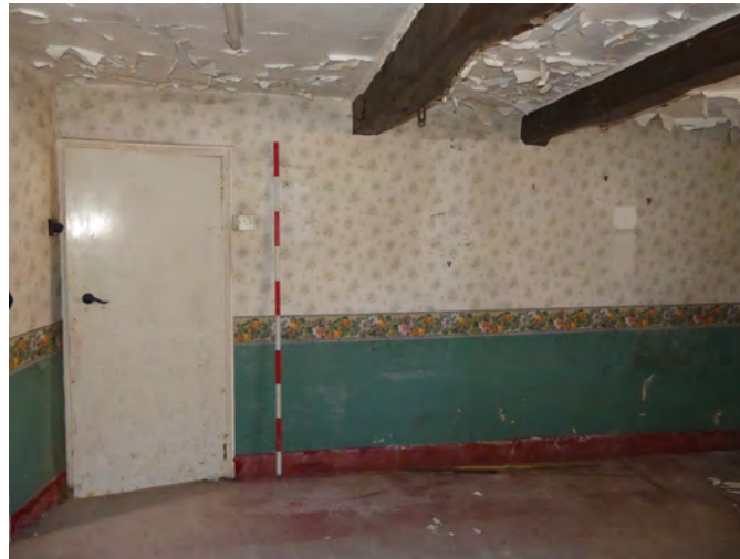
Plate 44: North-west elevation of G4 (farmhouse), viewed from the south-east
