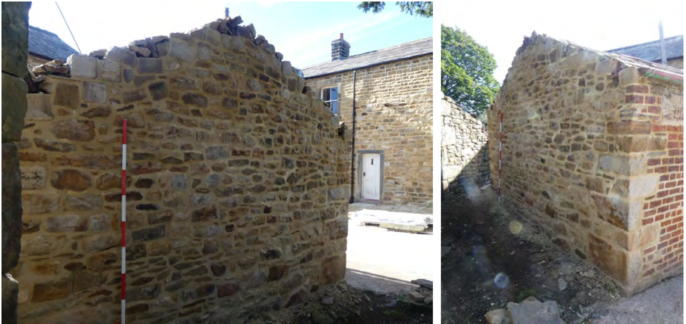
Plate 158 (left): North-west gable of the north-west external elevation of the barn, viewed from the north Plate 159 (right): North-west gable of the north-west external elevation of the barn, viewed from the west
