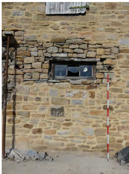
Plate 171: North-east window in the south-east external elevation of the barn, viewed from the south-east
