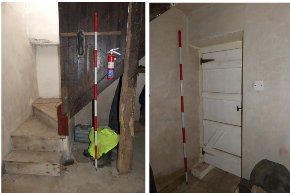
Plate 30 (left): Stairs in G2 (farmhouse), viewed from the north-west
