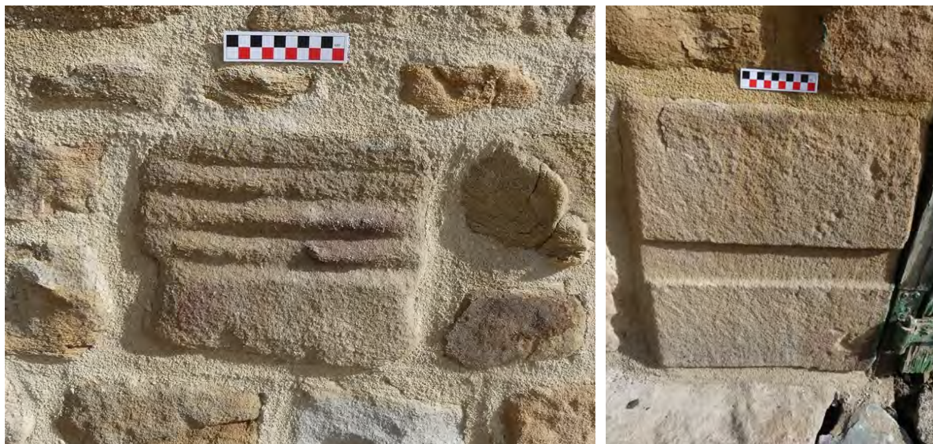
Plate 164 (left): Ribbed stone in the south-west external elevation of the barn, viewed from the south-west
