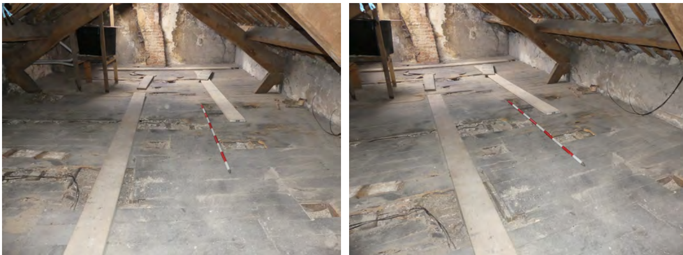
Plate 130 (left): Floor in A3 (farmhouse), viewed from the south-west
