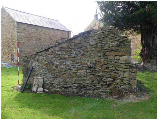
Plate 197: North external elevation of the outbuilding, viewed from the north
