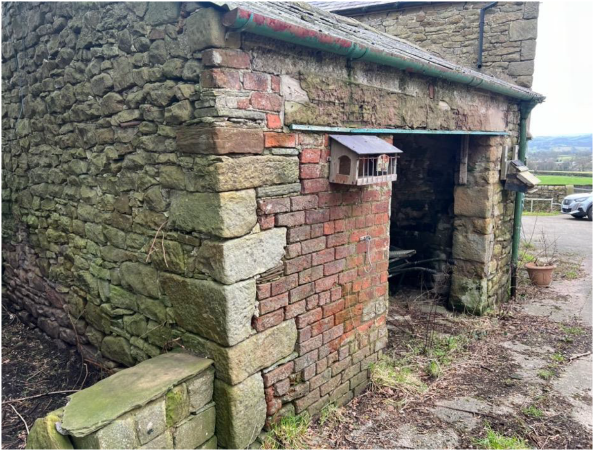
Photo 16 – South West Elevation of outtrigger
