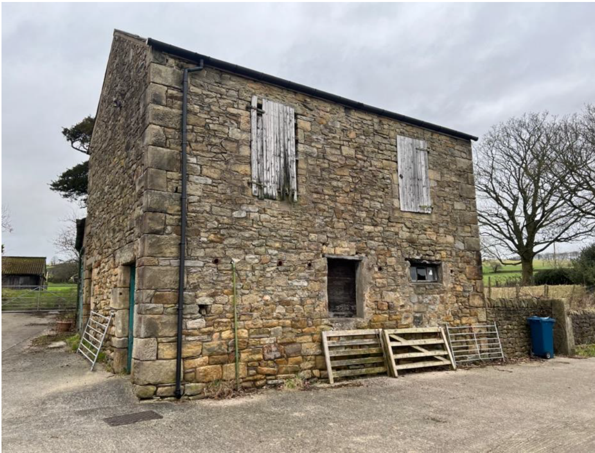
Photo 1 - South East Elevation
