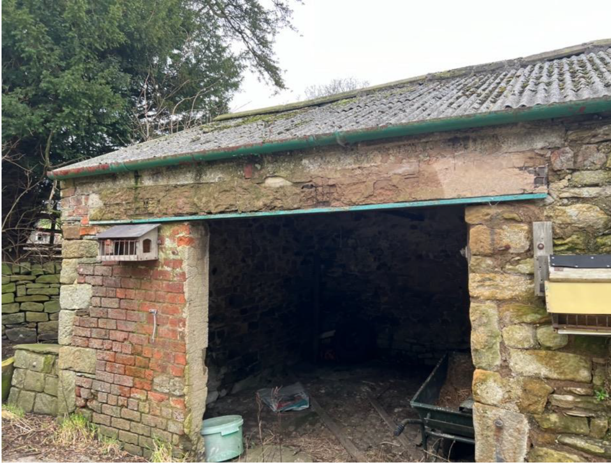
Photo 12 - South West Elevation outrigger
