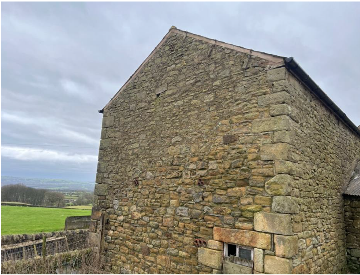
Photo 21 – North East Elevation
