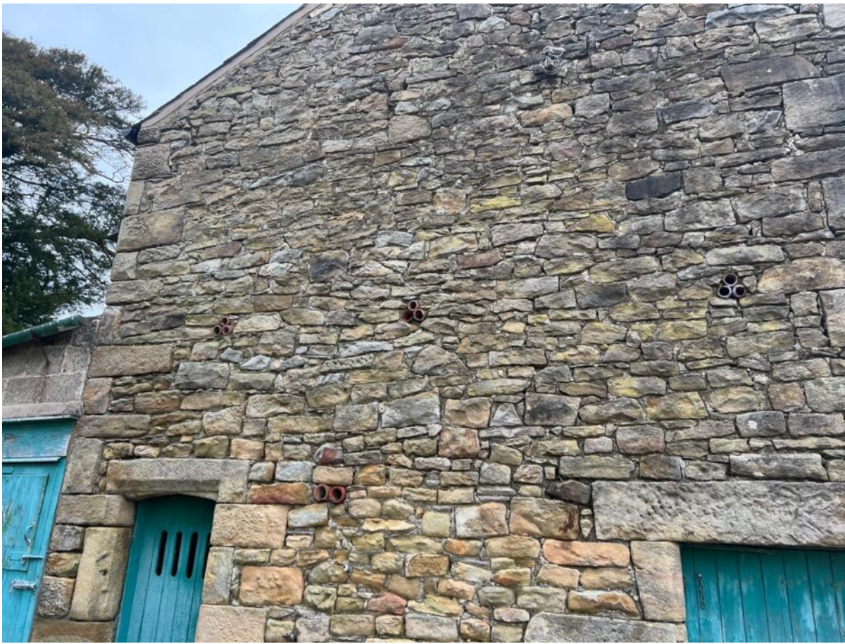
Photo 9 – South West Elevation
