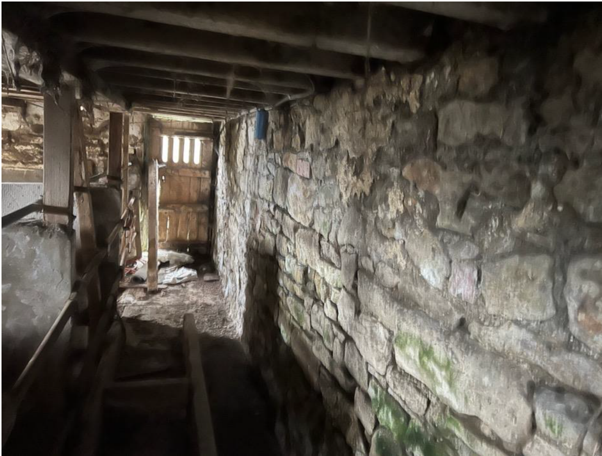
Photo 28 – Internal looking south west along North West Wall to main barn
