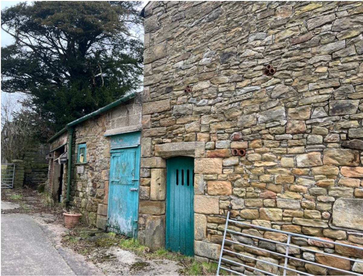
Photo 8 – South West Elevation
