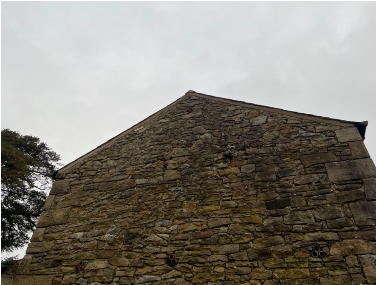
Photo 6 – South West Elevation
