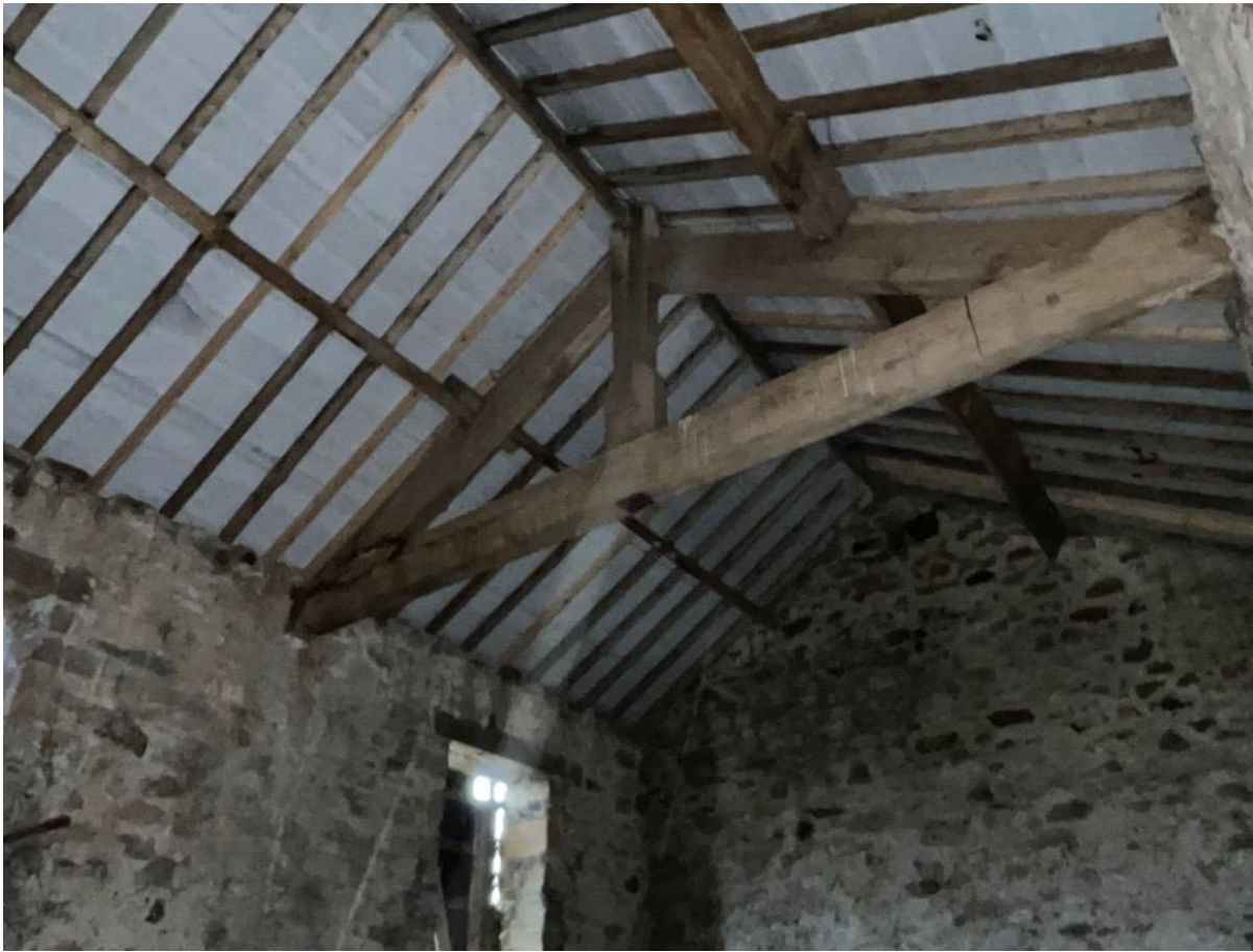
Photo 32 – Internal roof and truss
