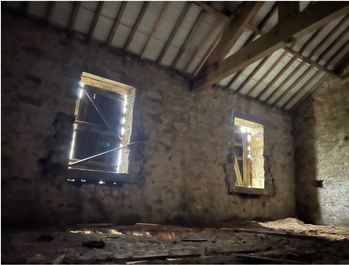
Photo 30 – Internal loft area looking south east
