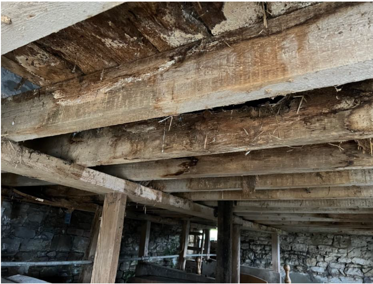
Photo 25 – Intrnal joists to upper loft
