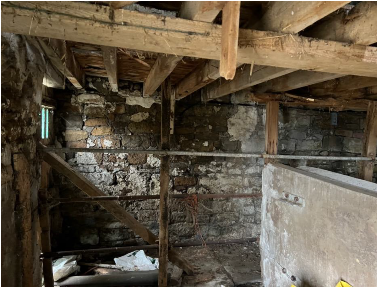
Photo 24 – Internal looking North West
