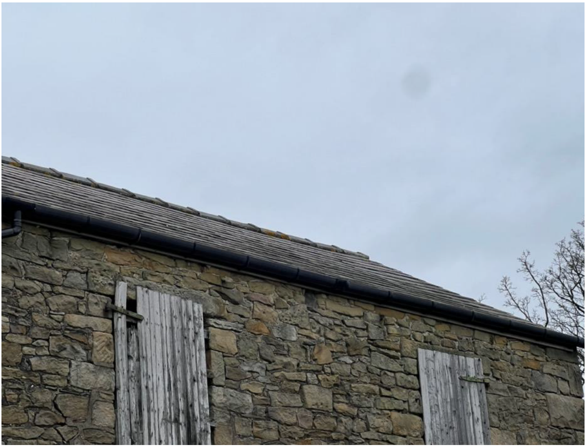
Photo 5 – South East Elevation and roof
