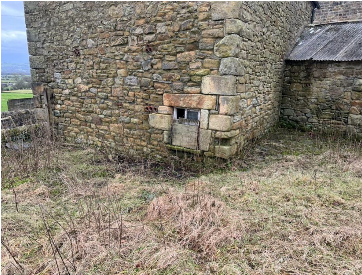
Photo 22 – North East Elevation
