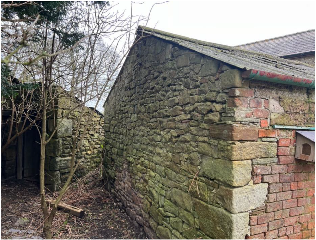
Photo 15 - North West Elevation - outtrigger
