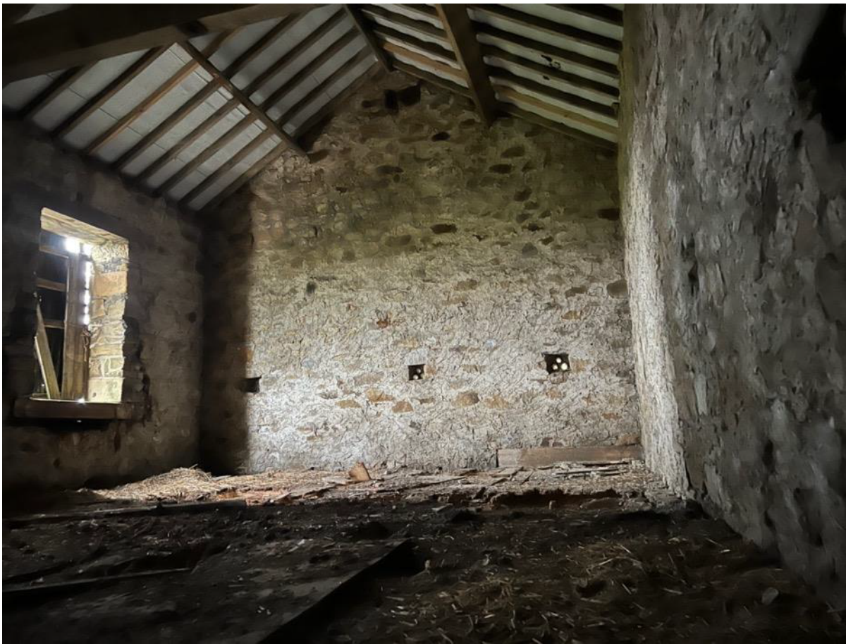
Photo 31 - Internal loft area looking south west
