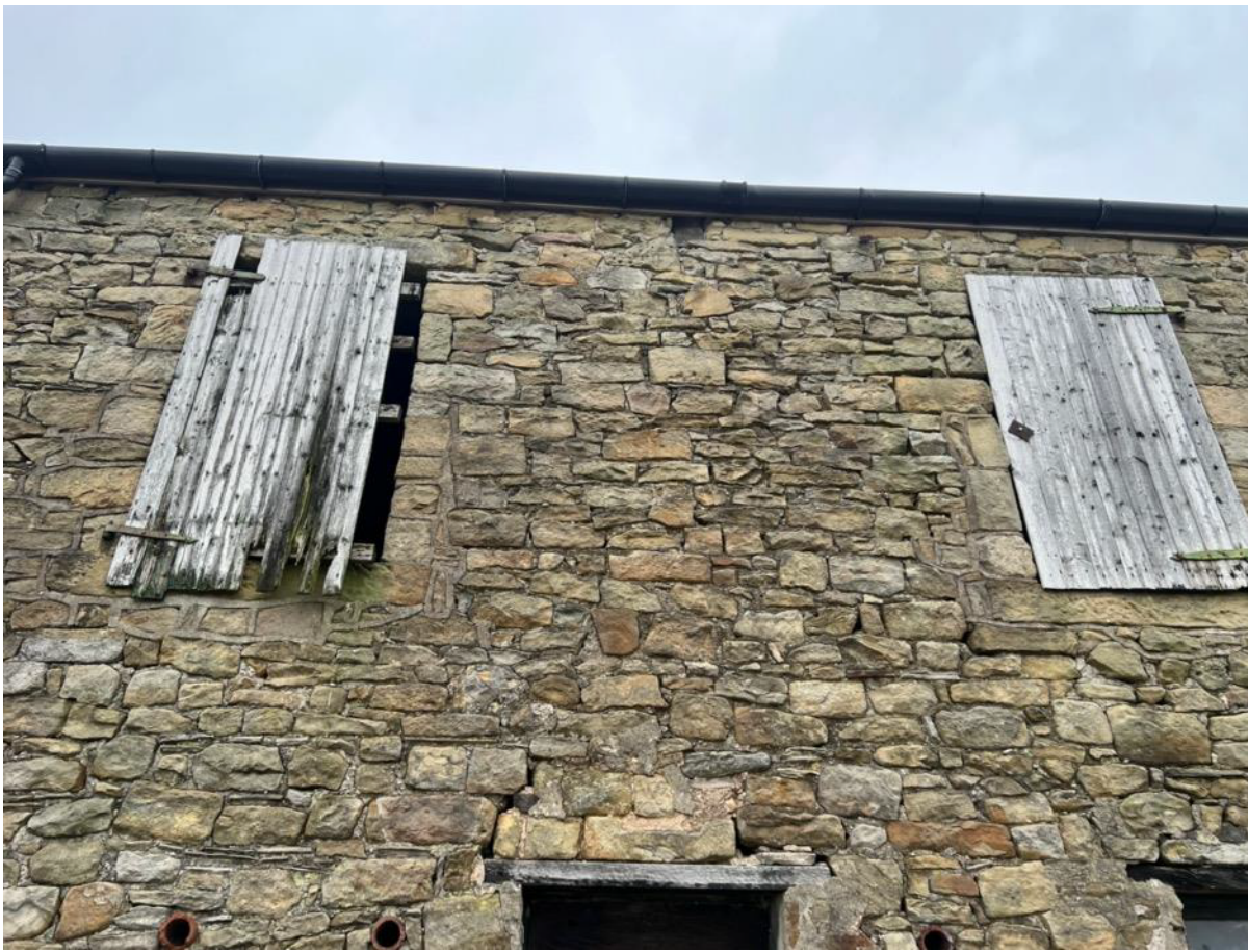
Photo 3- South East Elevation
