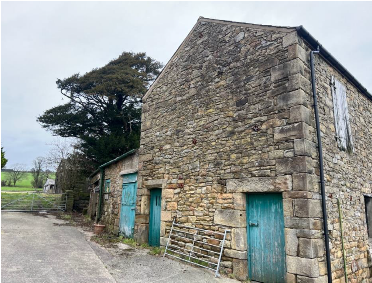
Photo 2 – South West Elevation
