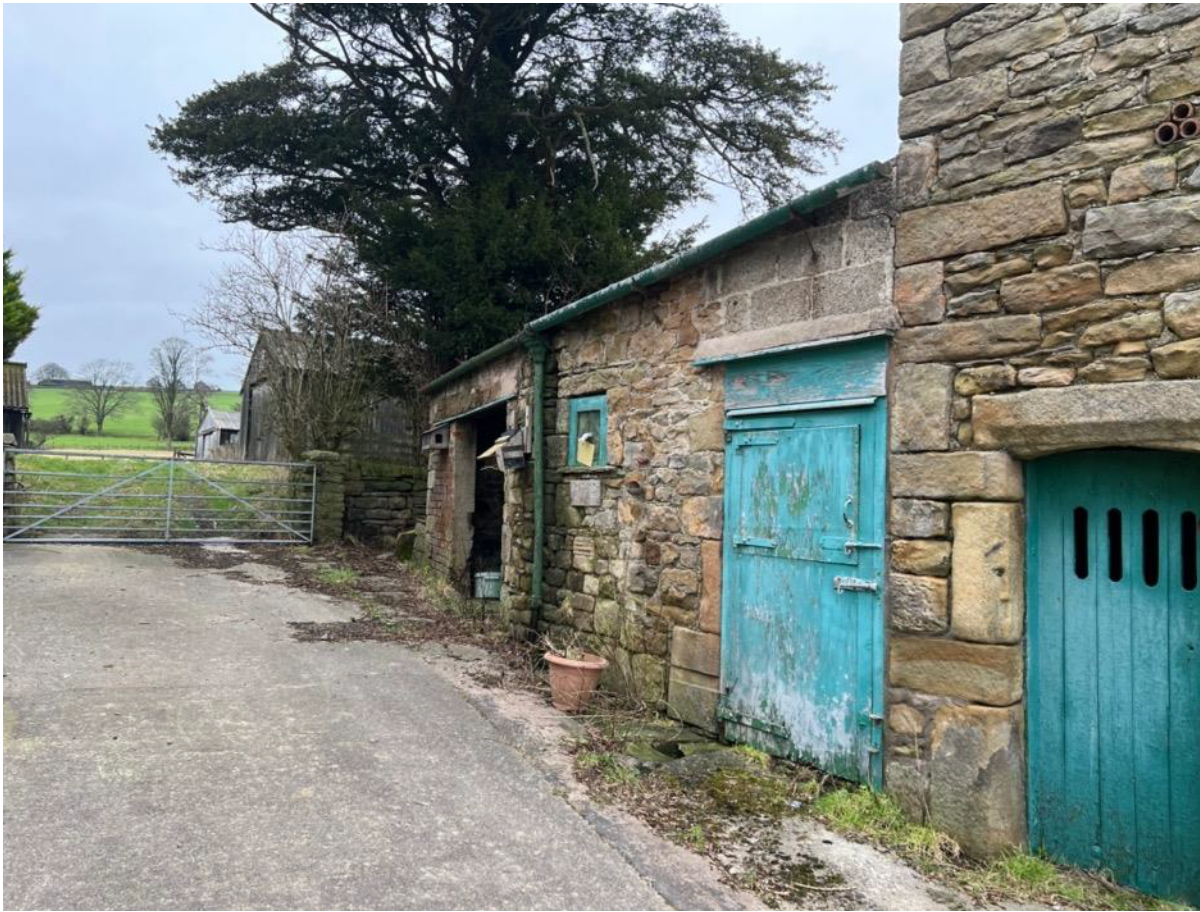
Photo 10 – South West Elevation – outrigger and main barn
