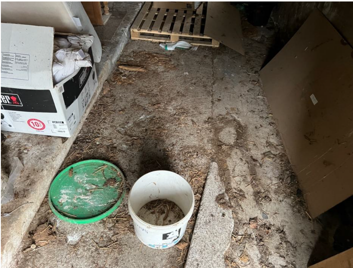
Photo 23 – Internal concrete floor
