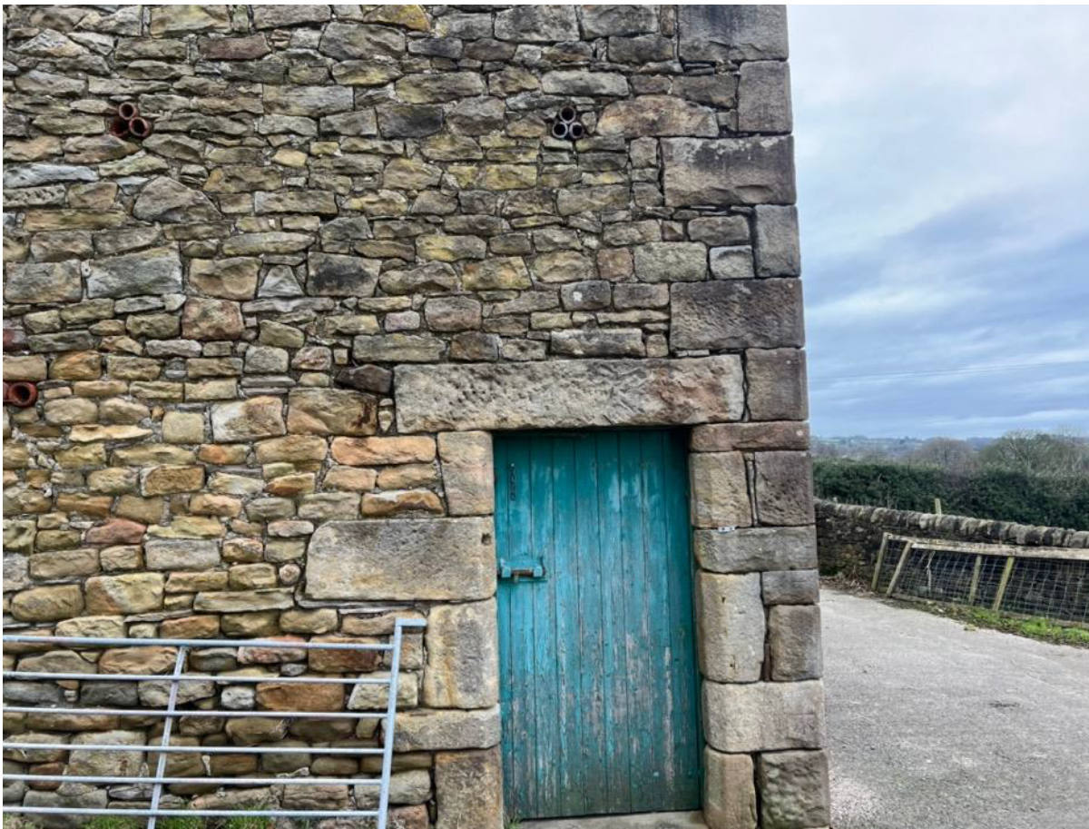
Photo 7 – South West Elevation
