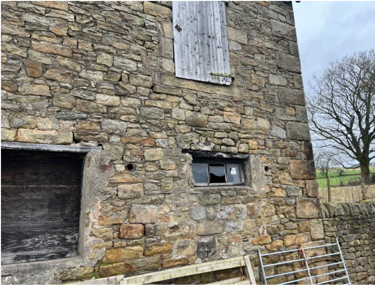
Photo 4 – South East Elevation
