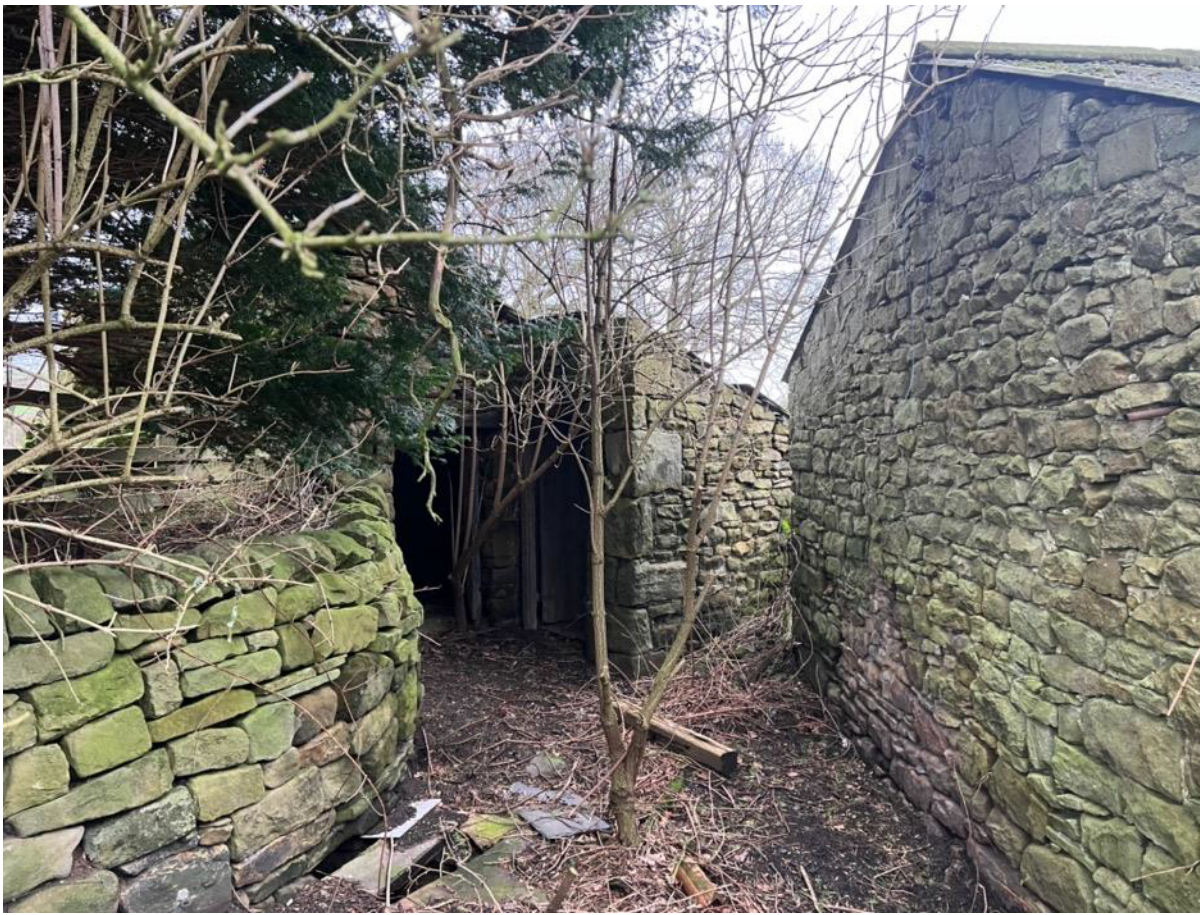
Photo 17 - North West Elevation - outrigger
