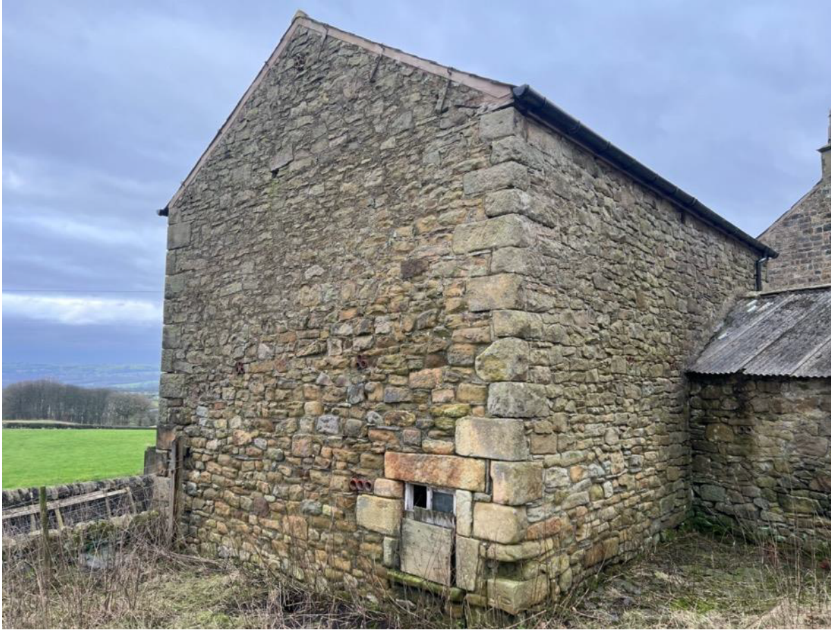
Photo 18 – North East Elevation
