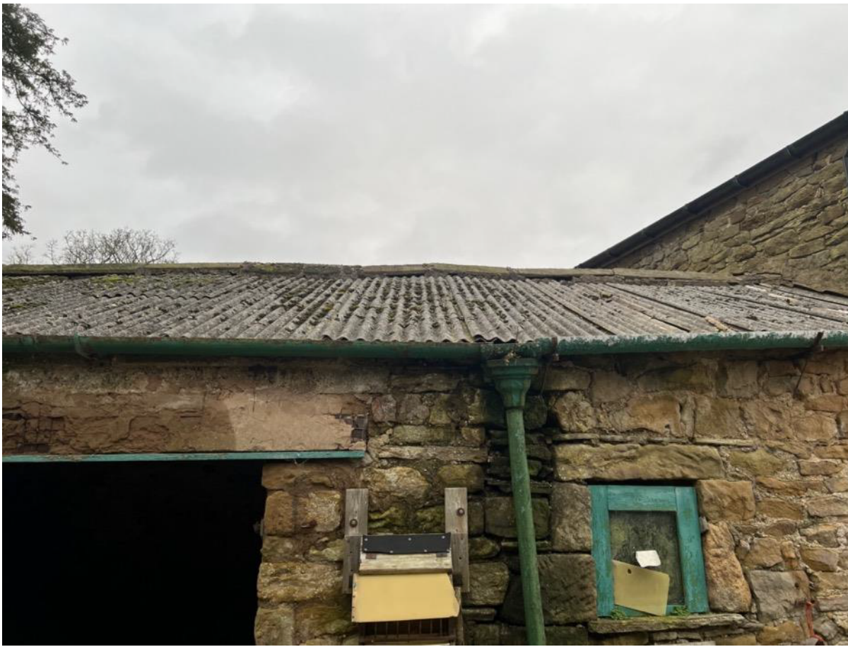
Photo 13 - South West Elevation outrigger and roof
