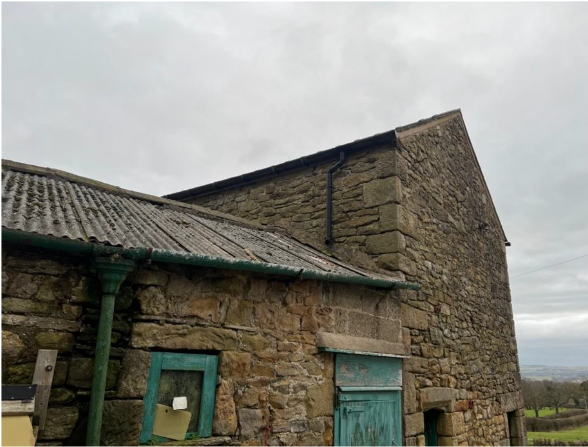
Photo 14 - South West Elevation and upper North West Elevation
