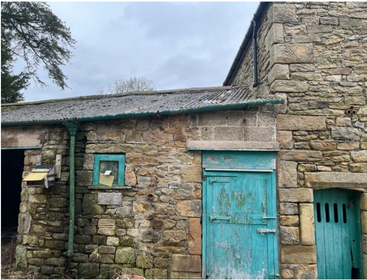
Photo 11 - South West Elevation – outrigger and main barn
