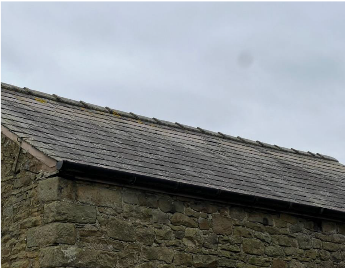
Photo 20 – Roof – North West
