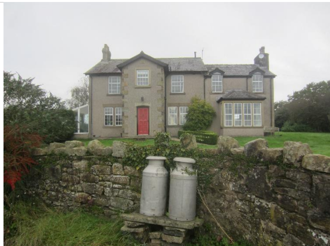
Photo 1: South-eastern elevation of the farmhouse
