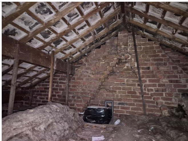
Photo 29: Roof void at farmhouse
