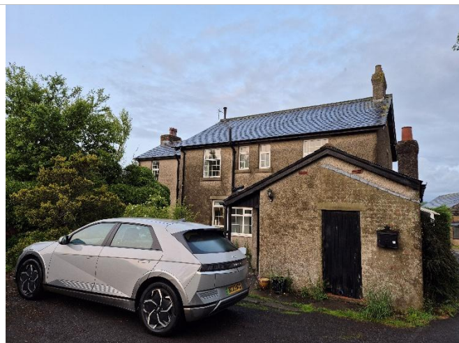
Photo 28: North-western elevation of the farmhouse
