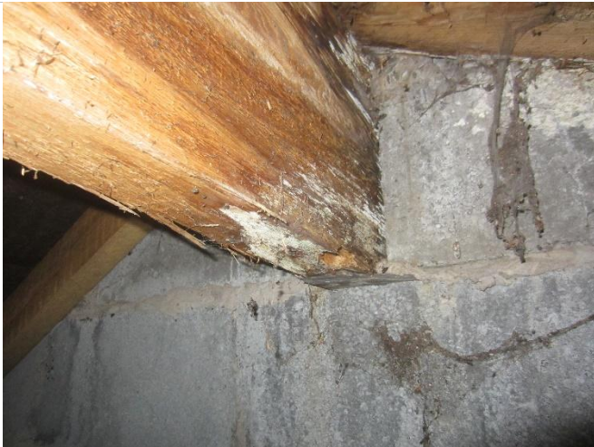
Photo 21: Internal side of north-east facing gable elevation wall of the farmhouse
