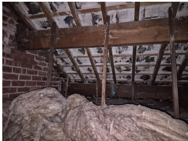
Photo 30: Roof void at farmhouse
