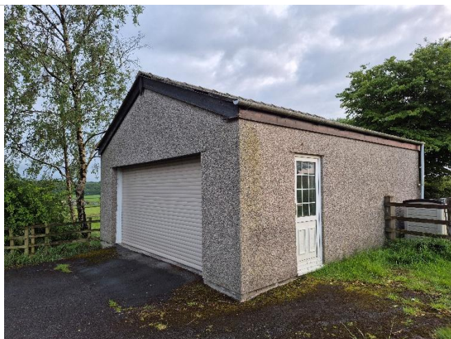
Photo 31: Eastern and northern elevations of the garage
