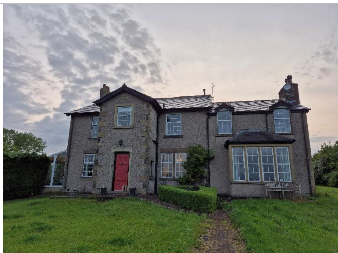
Photo 27: South-eastern elevation of the farmhouse
