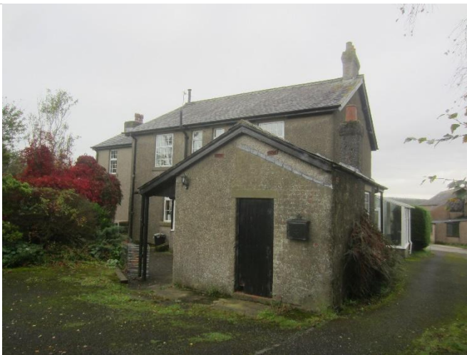
Photo 7: North-western elevation of the farmhouse showing single storey utility section
