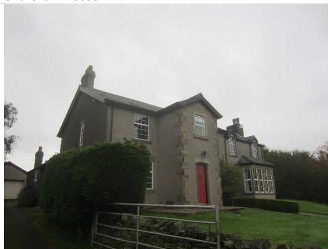
Photo 4: South-western and south-eastern elevations of the farmhouse
