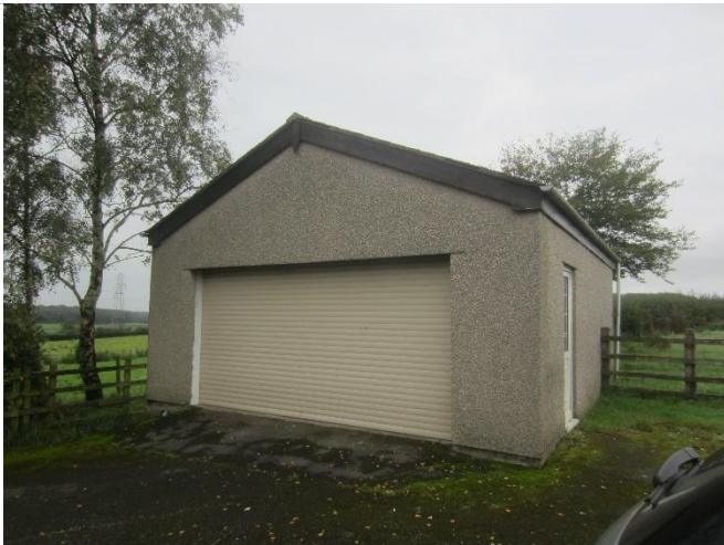
Photo 23: Eastern elevation of garage
