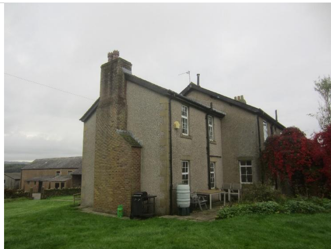
Photo 6: North-eastern and north-western elevations of the farmhouse
