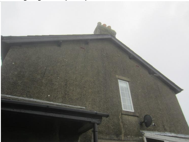
Photo 9: South-western elevation of the farmhouse
