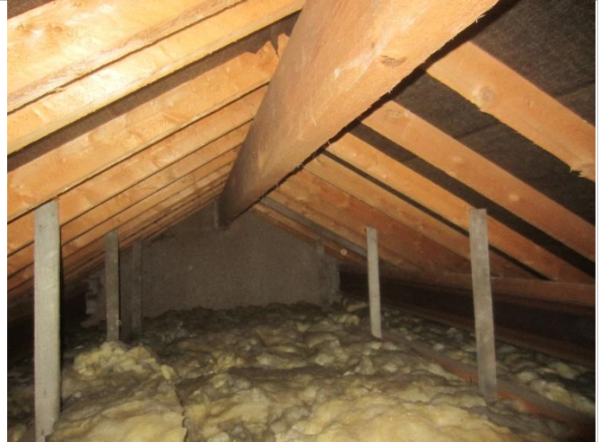
Photo 20: Roof void at eastern section of farmhouse
