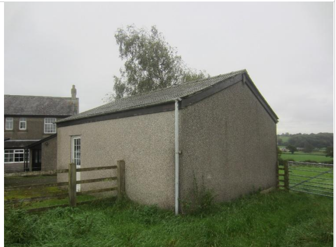
Photo 24: Northern and western elevations of garage
