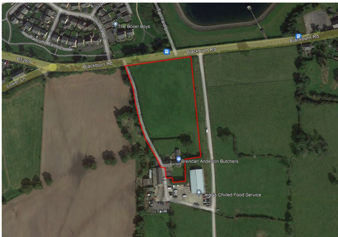
Figure 1: An aerial image of the site in its wider setting
