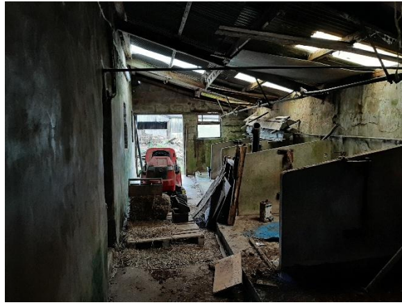
Figure 5: Internal view of extension area
