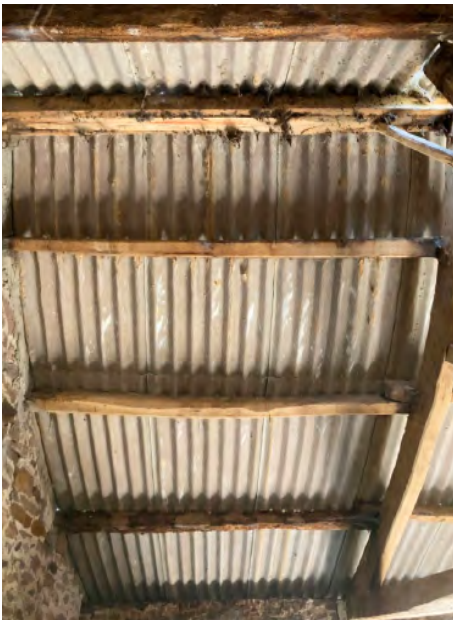
East end bay south slope of main barn
