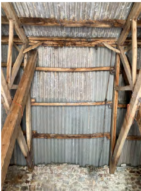
Central bay north slope of main barn
