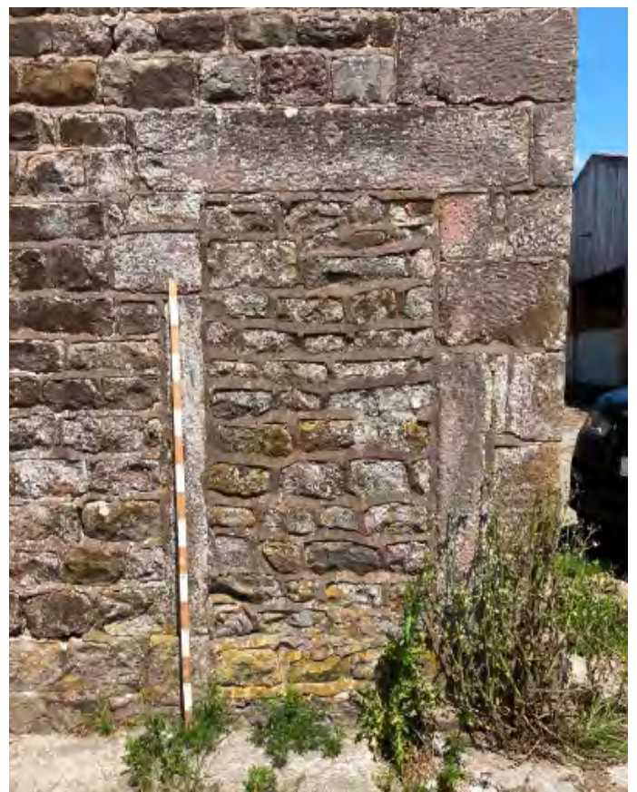
Blocked right hand / east byre door
