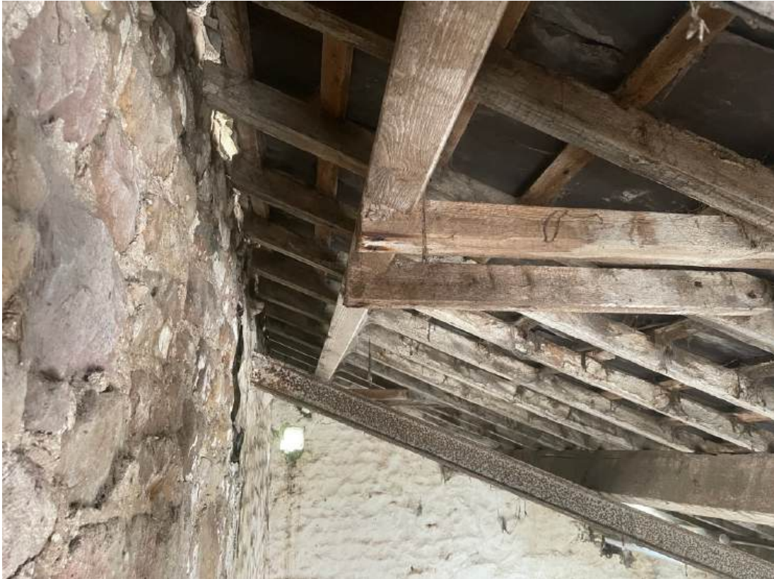
Photo Five: Shippon – General Roof Structure
