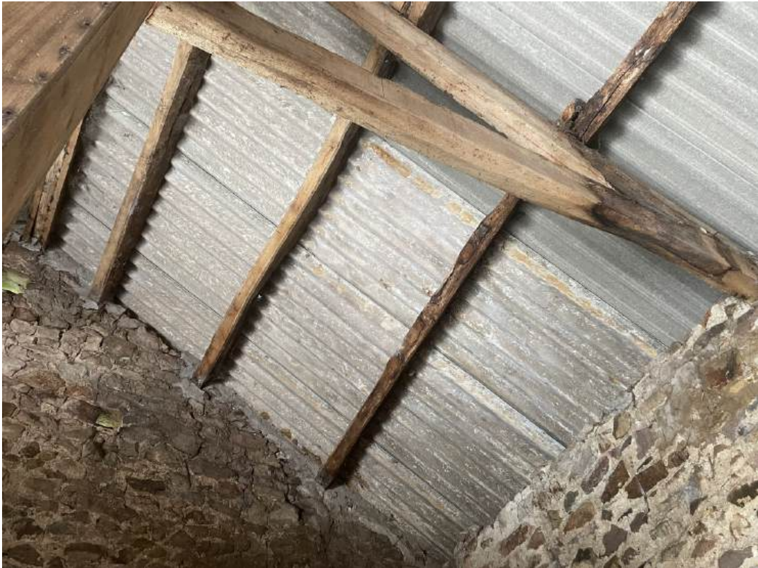
Photo Two: Main Barn – Lefthand Side of Roof
