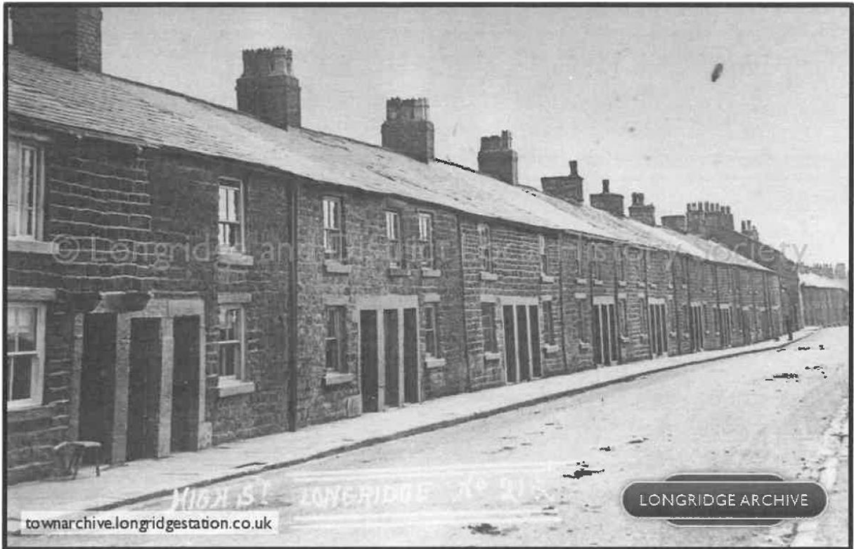
Historic streetscape photo showing Club Row from the front (Higher Road)
