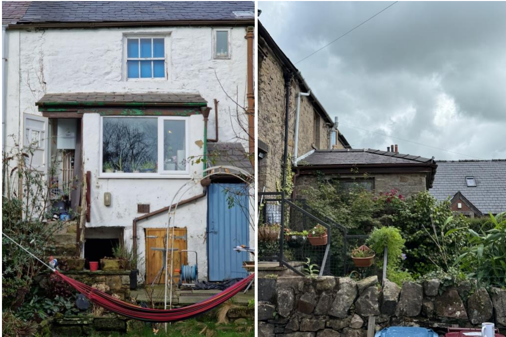
Rear elevation of No. 38 showing current and surrounding extensions]
