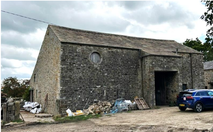
Figure 9 Gable of B2, PRF;s in the wall and at the eaves
