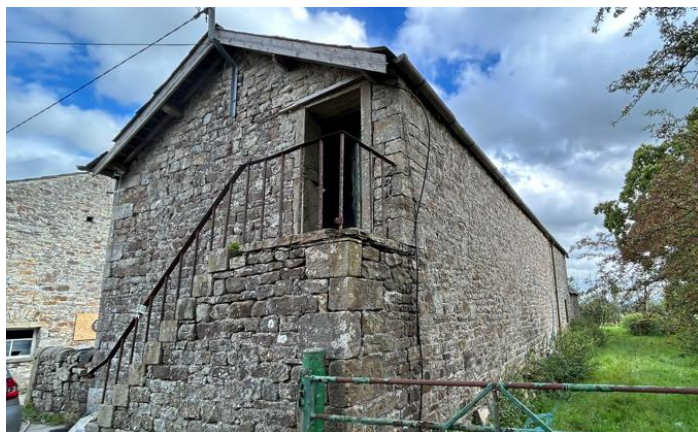
Figure 5 Gable of B2, PRF;s in the wall and at the eaves
