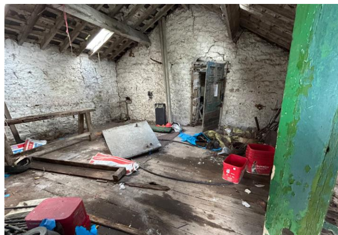
Figure 8 Interior of B2
