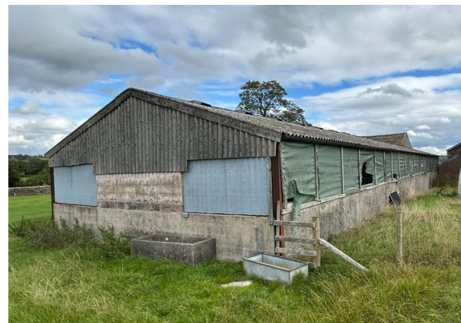
Figure 4 A&B Construction of B1
