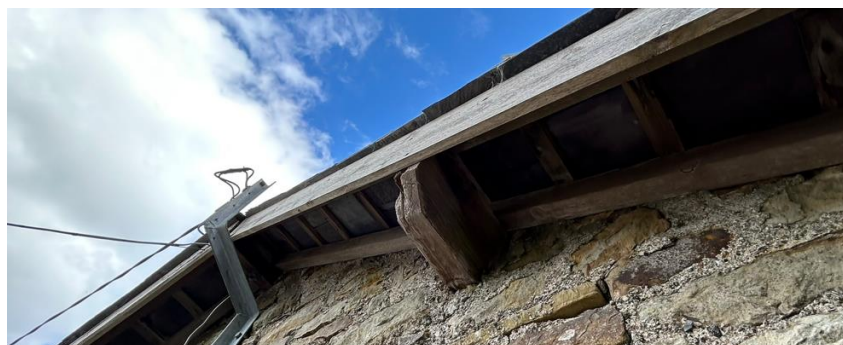
Figure 6 PRFs at eaves
