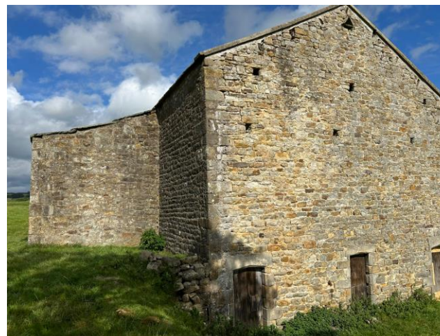
Figure 15 showing ventilation holes on southern gable.
