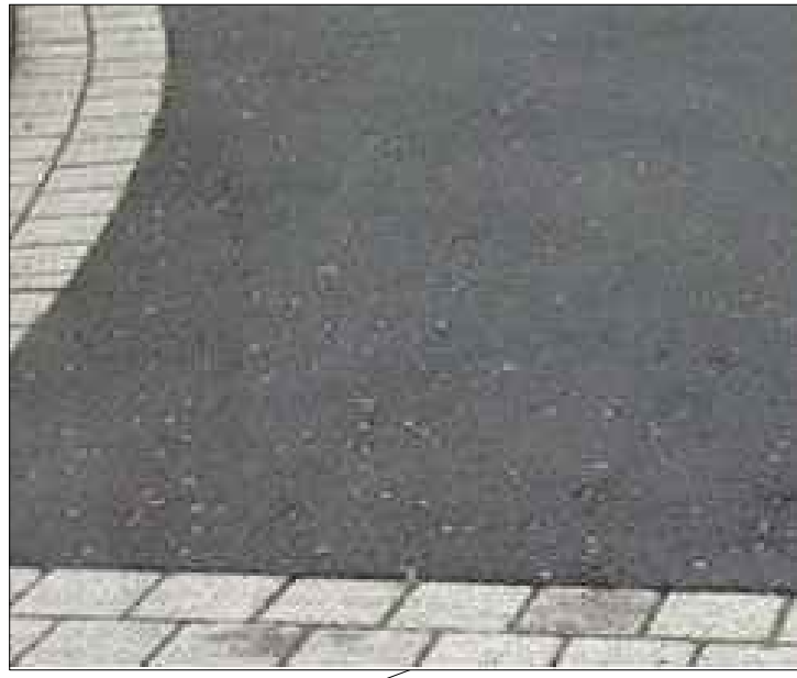
Chiptex Macadam Surfing with Flush Sett Edging
