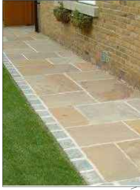
Sandstone flag paving with sett edging
