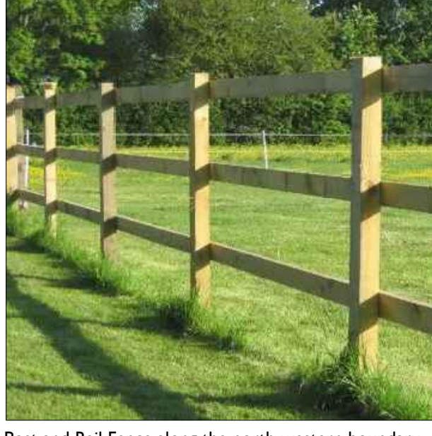
Post and Rail Fence along the north-western boundary
