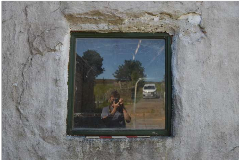
Plate 111 (shot 135): Detail of window in northwestern elevation of outbuilding, 0.5m scale
