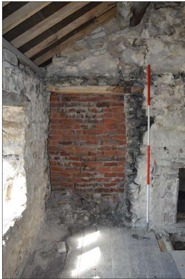
Plate 55 (shot 82): Detail of blocked doorway, southwestern wall of Room 4, 2m scale
