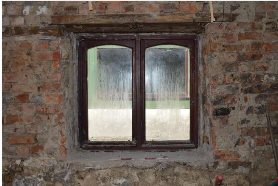
Plate 17 (shot 46): Detail of window, southwestern wall, Room 1, 0.5m scale
