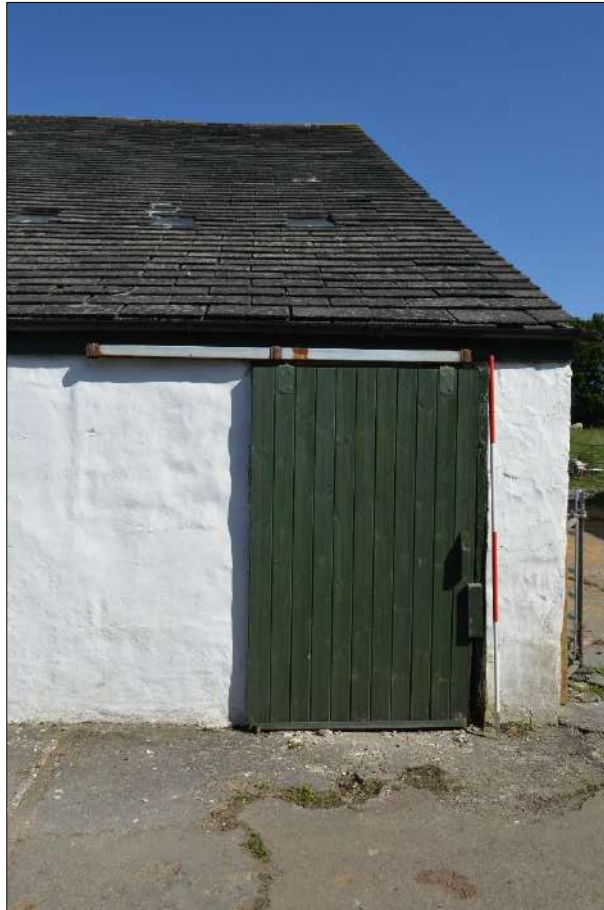
Plate 86 (shot 14): Detail of door of outshut, northeast end of main range, 2m scale
