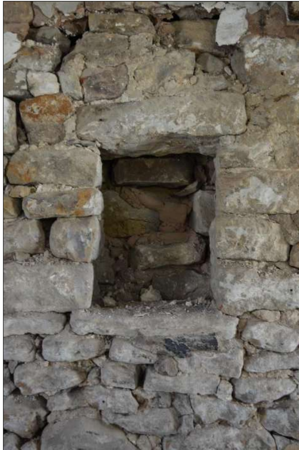
Plate 103 (shot 115): Detail of blocked opening in southeastern wall of outshut, Room 6, no scale
