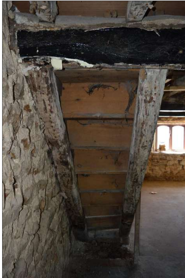
Plate 39 (shot 70): Detail of staircase, Room 2, 2m scale
