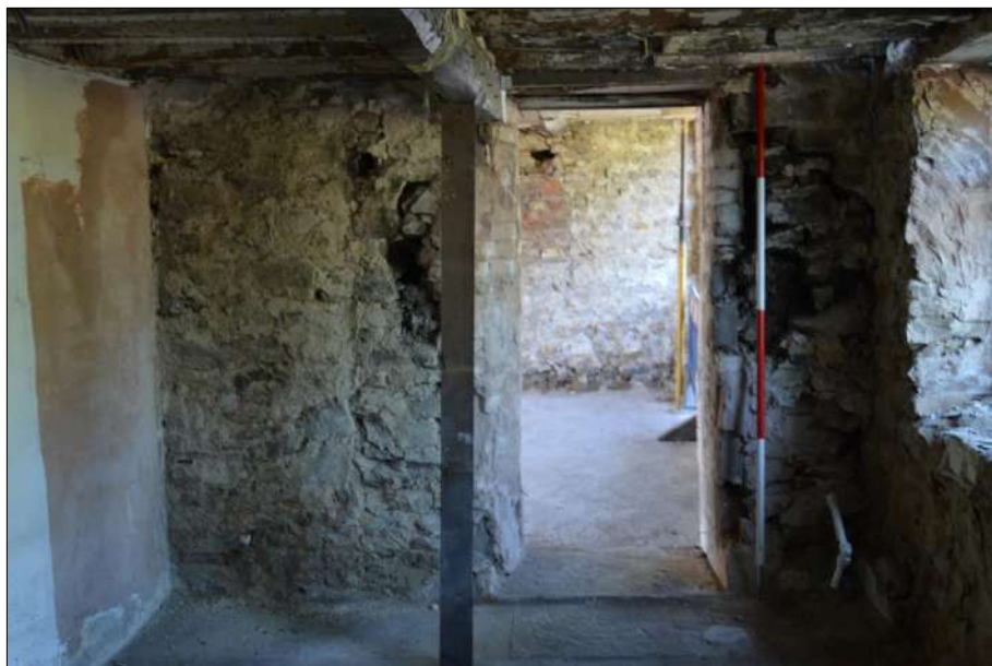
Plate 46 (shot 68): Southwestern wall of Room 3, 2m scale
