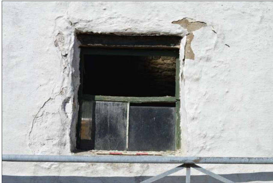
Plate 80 (shot 17): Detail of window in northeast elevation of barn, 0.5m scale
