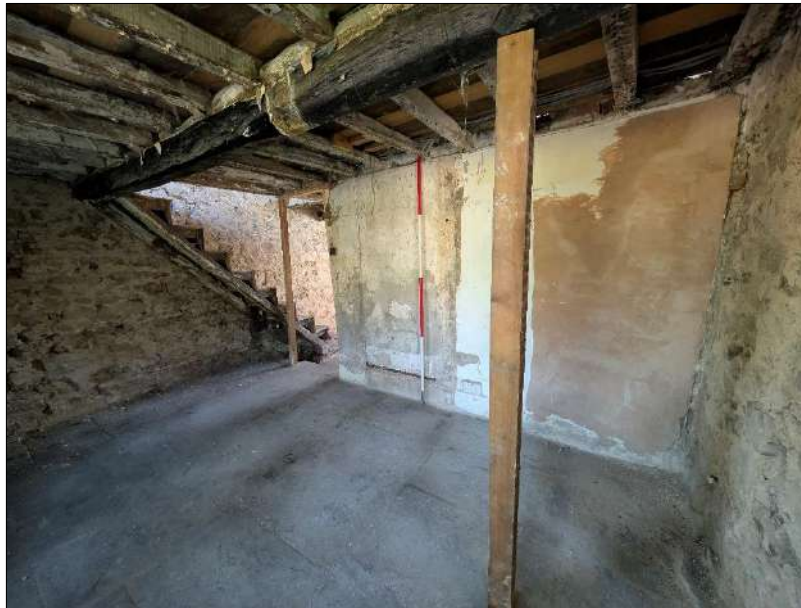
Plate 47 (shot 180): Southwestern wall of Room 3, 2m scale
