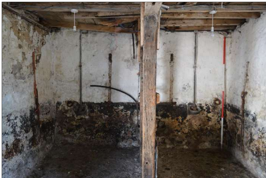
Plate 123 (shot 140): Northeastern wall of Room 7, 2m scale
