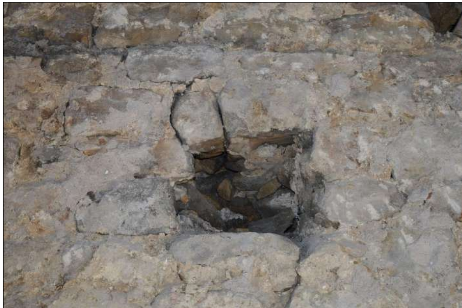
Plate 63 (shot 91): Detail of possible socket for ceiling beam, northeastern wall of Room 5, no scale
