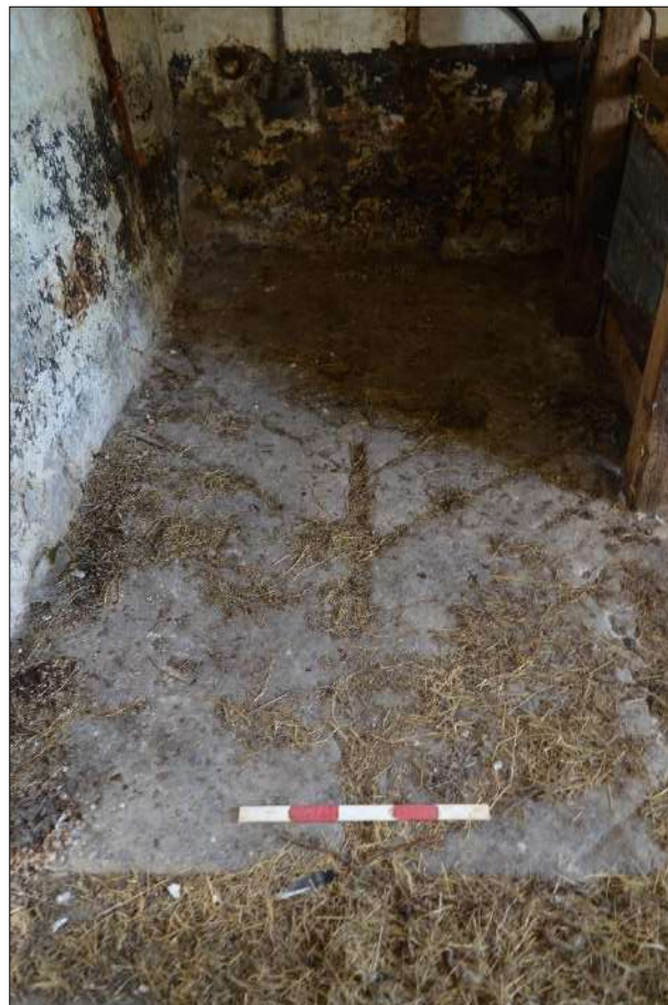
Plate 125 (shot 145): Detail of floor, northwestern stall at northeastern end of Room 7, 0.5m scale
