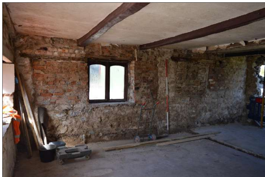
Plate 16 (shot 43): Interior of Room 1, looking northwest, 2m scale
