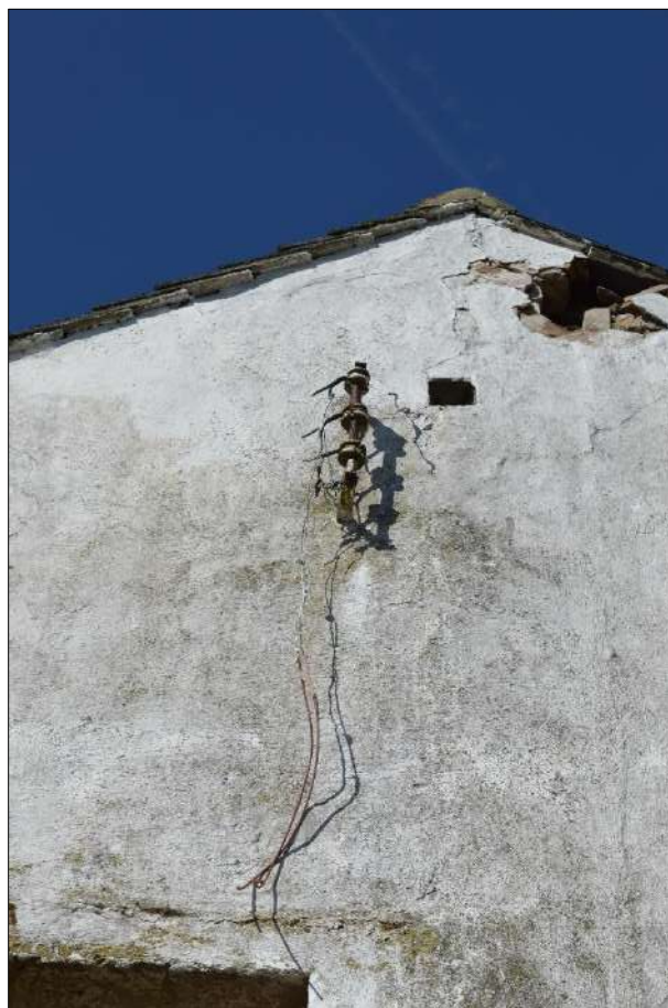
Plate 81 (shot 21): Detail of bracket and vent in northeast elevation of barn, no scale
