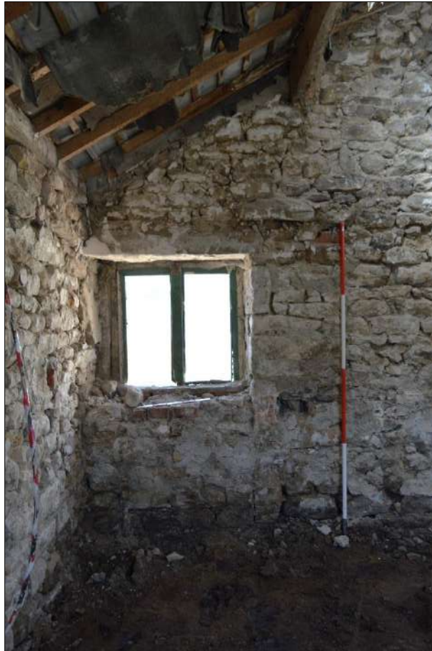
Plate 106 (shot 118): Detail of window in southwestern wall of outshut, Room 6, 2m scale
