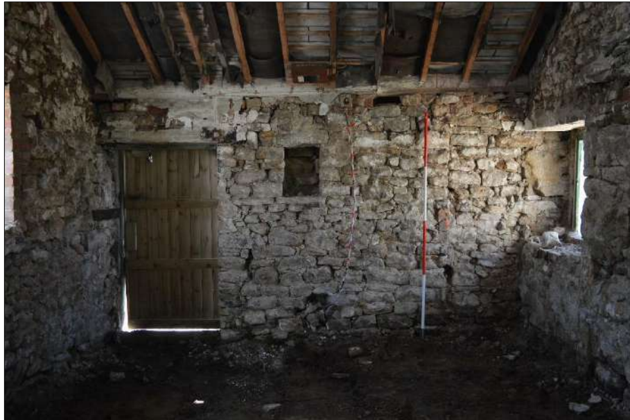
Plate 100 (shot 113): Southeastern wall of outshut, Room 6, 2m scale
