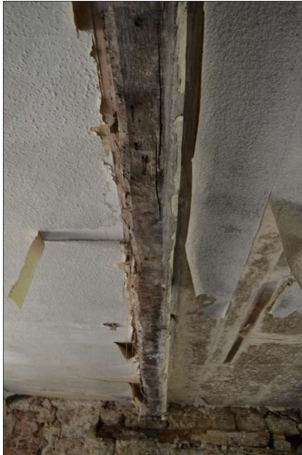
Plate 31 (shot 54): Detail of ceiling beam, Room 1, no scale
