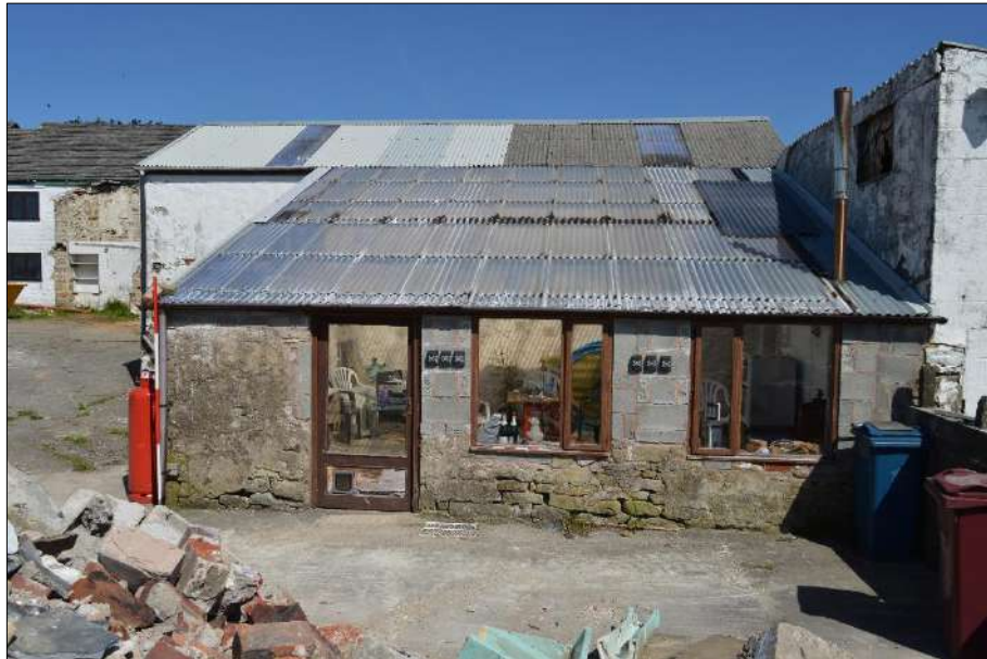
Plate 118 (shot 131): Southeastern elevation of extension to outbuilding, 2m scale
