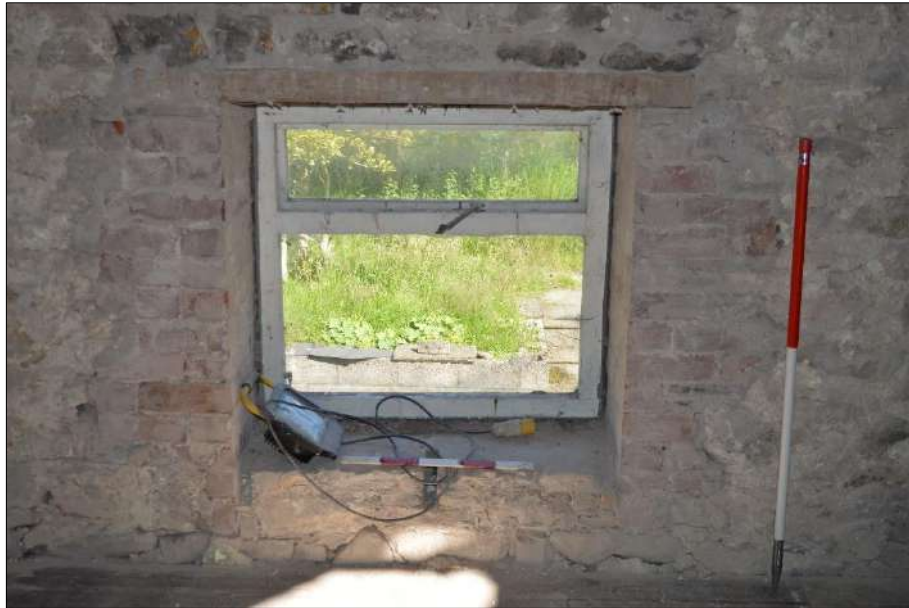
Plate 70 (shot 95): Detail of window, northwestern wall of Room 5, 1m and 0.5m scales
