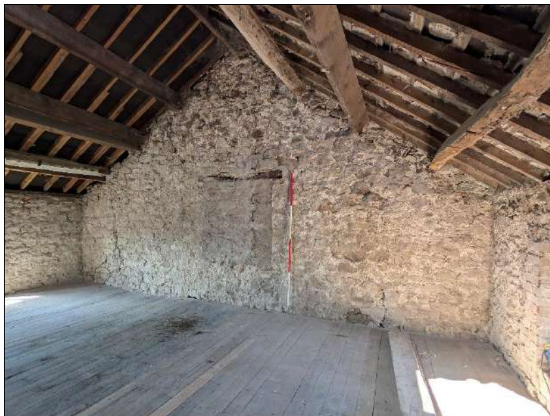
Plate 67 (shot 187): Southwestern wall of Room 5, 2m scale
