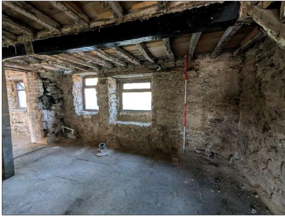
Plate 41 (shot 182): Interior of Room 3, looking northwest, 2m scale
