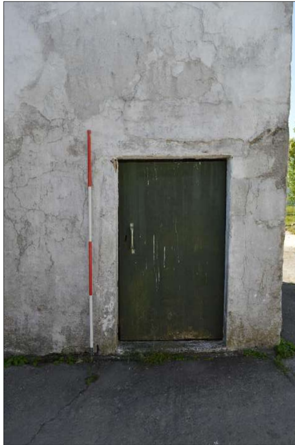
Plate 113 (shot 137): Detail of door in northwestern elevation of outbuilding, 2m scale
