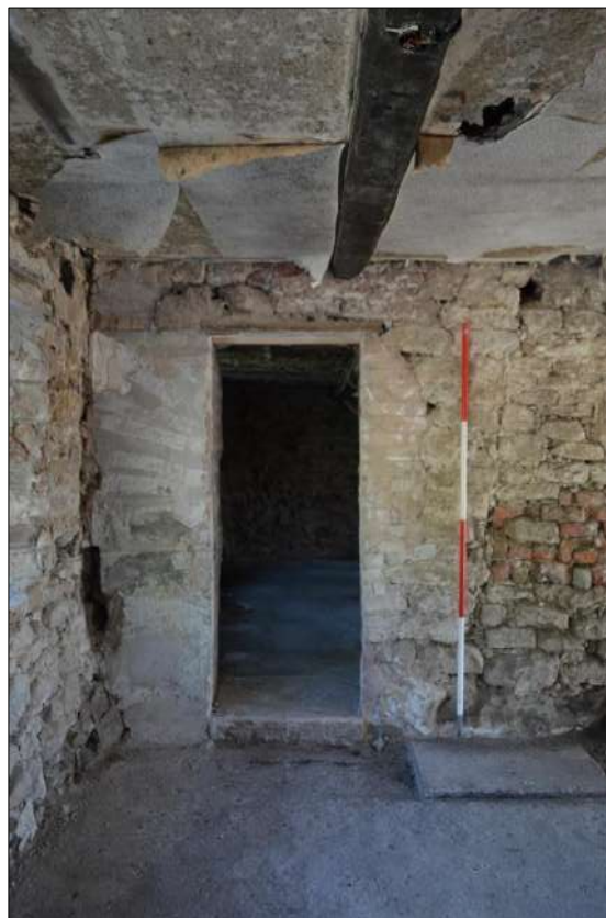
Plate 24 (shot 52): Detail of doorway in northeastern wall of Room 1, 2m scale
