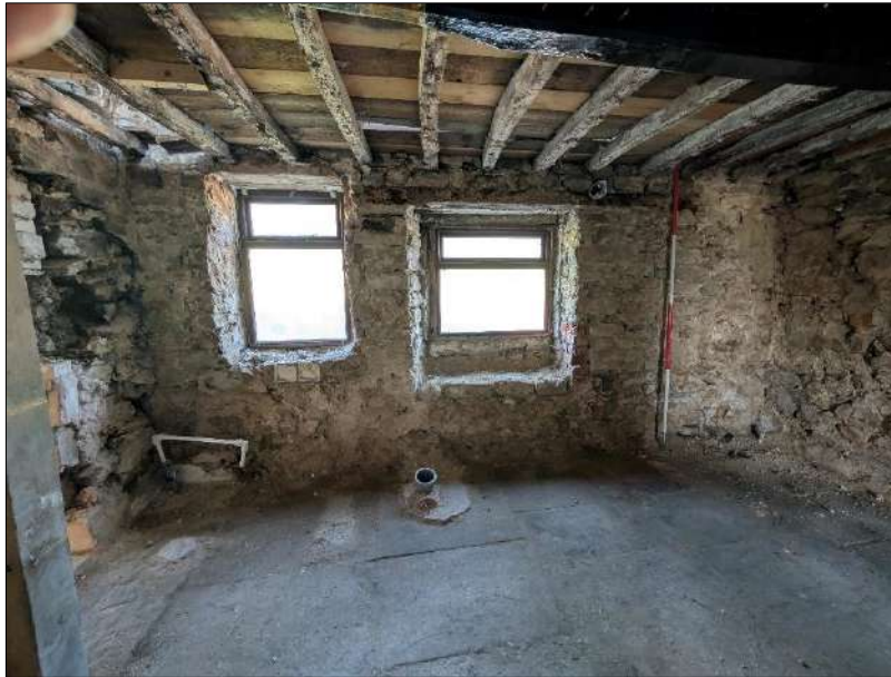
Plate 43 (shot 181): Northwestern wall of Room 3, 2m scale
