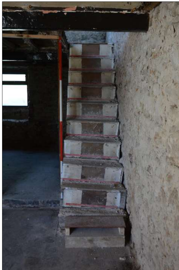
Plate 38 (shot 67): Detail of staircase, Room 2, 2m scale
