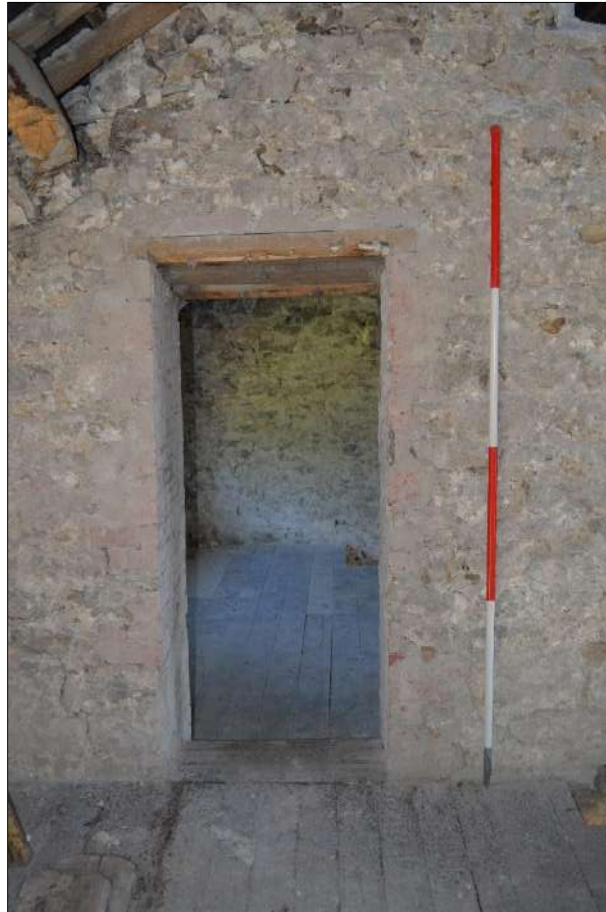
Plate 61 (shot 89): Detail of doorway, northeastern wall of Room 5, 2m scale
