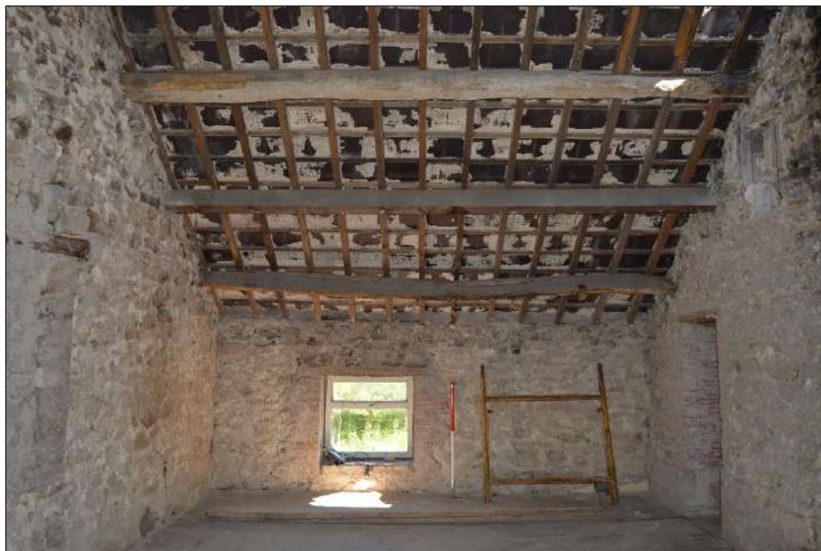
Plate 71 (shot 93): Northwest side of Room 5 showing roof construction, 1m and 0.5m scales
