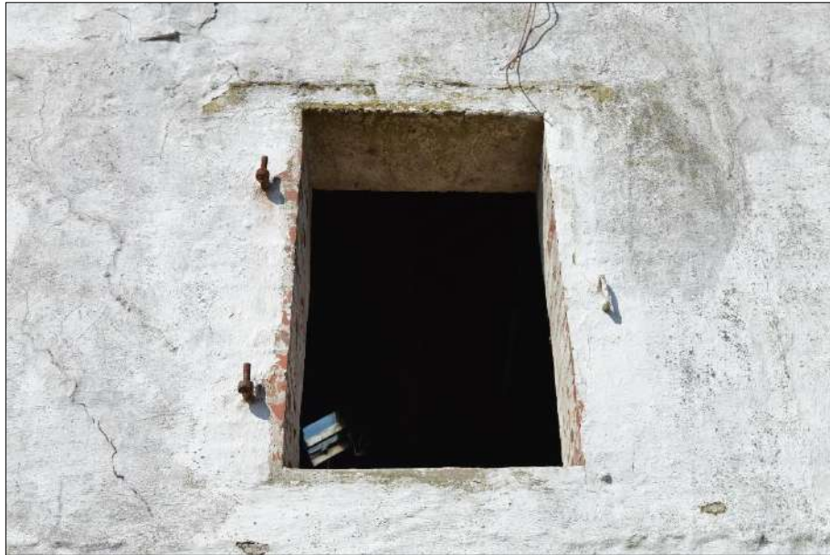
Plate 78 (shot 20): Detail of doorway in northeast elevation of barn, no scale
