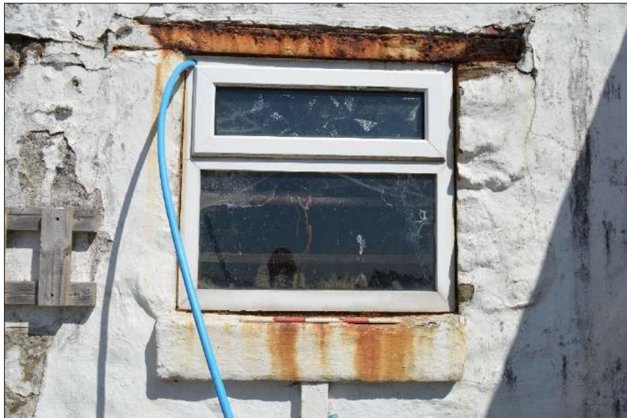
Plate 115 (shot 128): Detail of window in southeastern elevation of outbuilding, 0.5m scale
