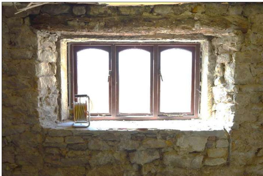
Plate 33 (shot 57): Detail of window, southeastern wall, Room 2, 0.5m scale
