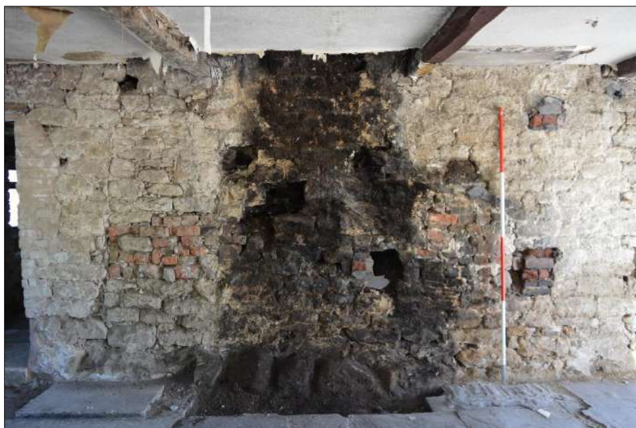
Plate 26 (shot 50): Detail of demolished fireplace on northeastern wall, Room 1, 2m scale
