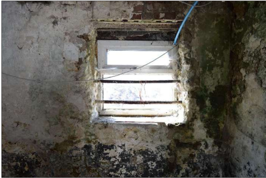
Plate 128 (shot 139): Detail of window in southeastern wall of Room 7, 0.5m scale
