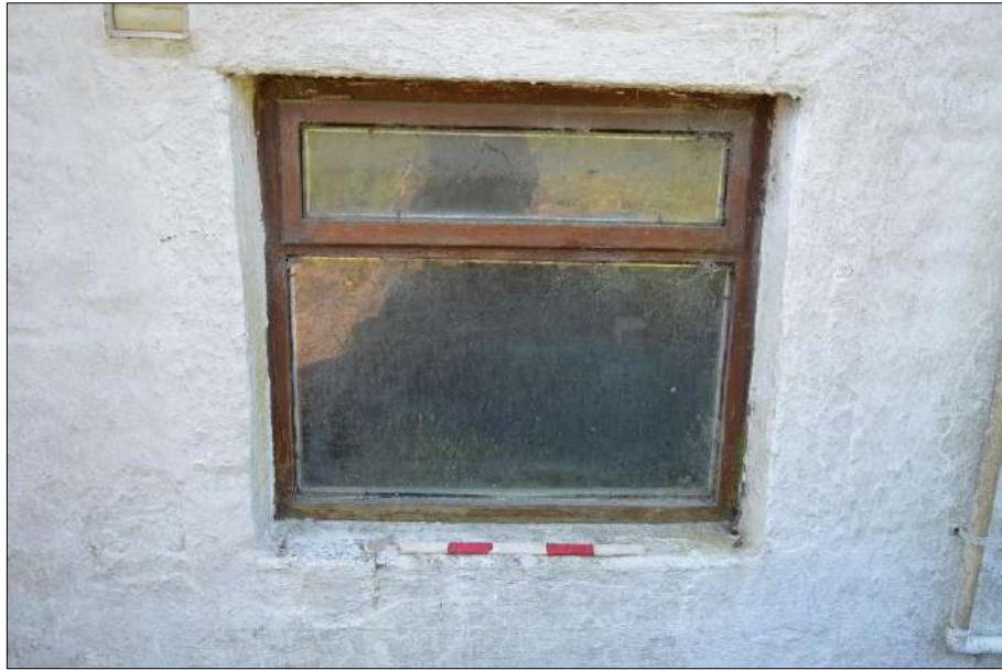
Plate 12 (shot 28): Detail of ground floor window, northwest elevation of farmhouse, 0.5m scale
