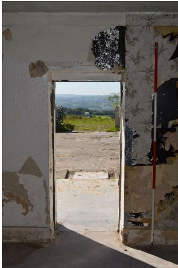
Plate 22 (shot 48): Detail of doorway in southeastern wall, Room 1, 2m scale
