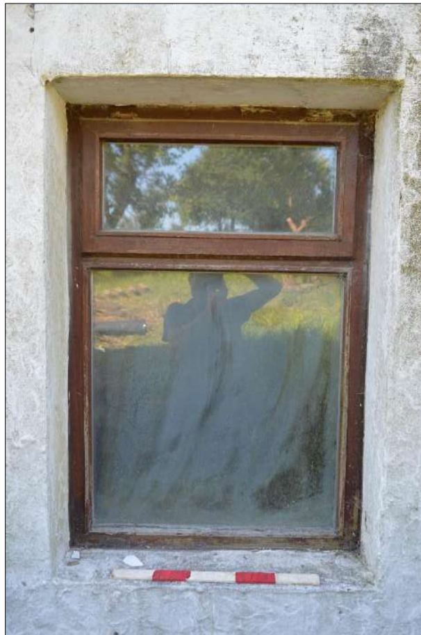
Plate 11 (shot 30): Detail of ground floor window, northwest elevation of farmhouse, 0.5m scale
