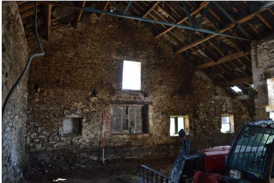
Plate 94 (shot 107): Northeastern wall of Room 6, 2m scale
