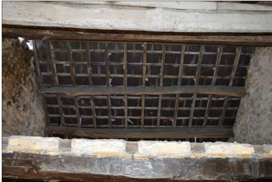
Plate 59 (shot 77): Detail of roof structure, Room 4, no scale
