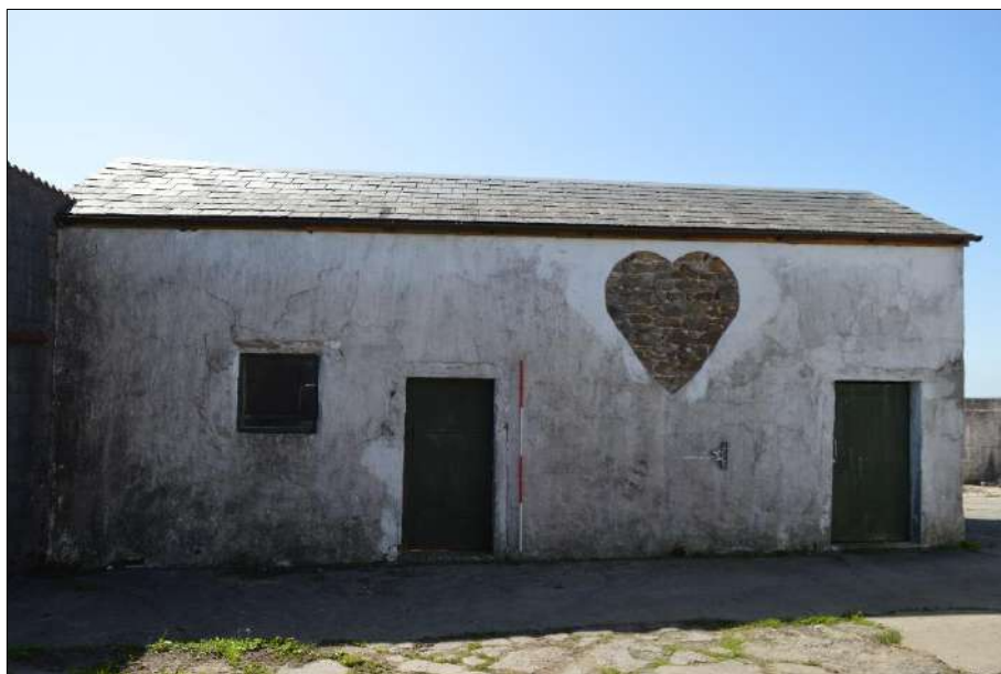
Plate 109 (shot 133): Northwestern elevation of outbuilding, 2m scale
