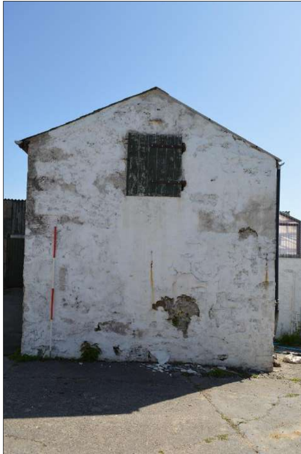
Plate 107 (shot 122): Southwestern elevation of outbuilding, 2m scale
