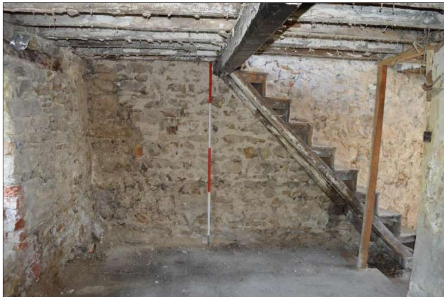
Plate 40 (shot 69): Northeastern wall of Room 2, 2m scale
