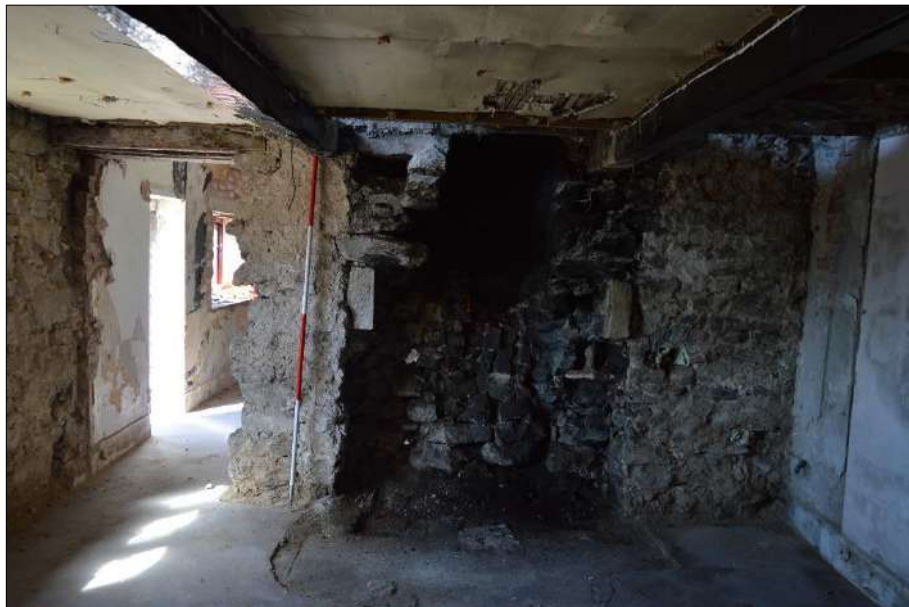
Plate 35 (shot 61): Southwestern wall of Room 2, 2m scale
