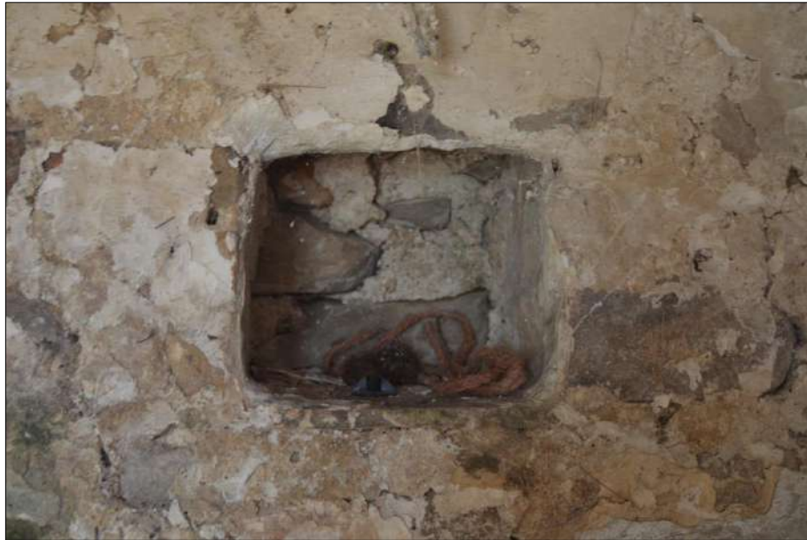
Plate 122 (shot 143): Detail of recess in northwestern wall of Room 7, no scale
