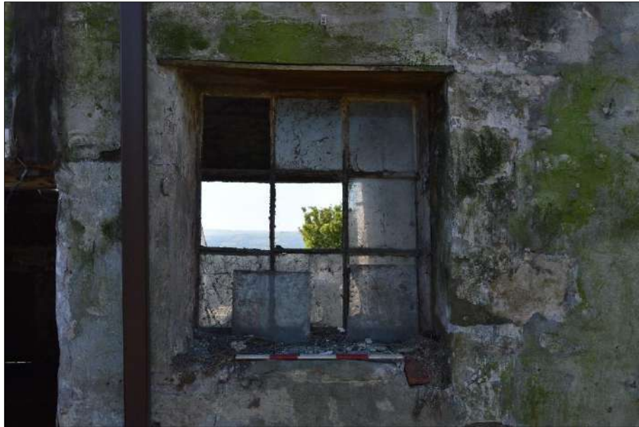
Plate 74 (shot 26): Detail of window in northwest elevation of barn, 0.5m scale
