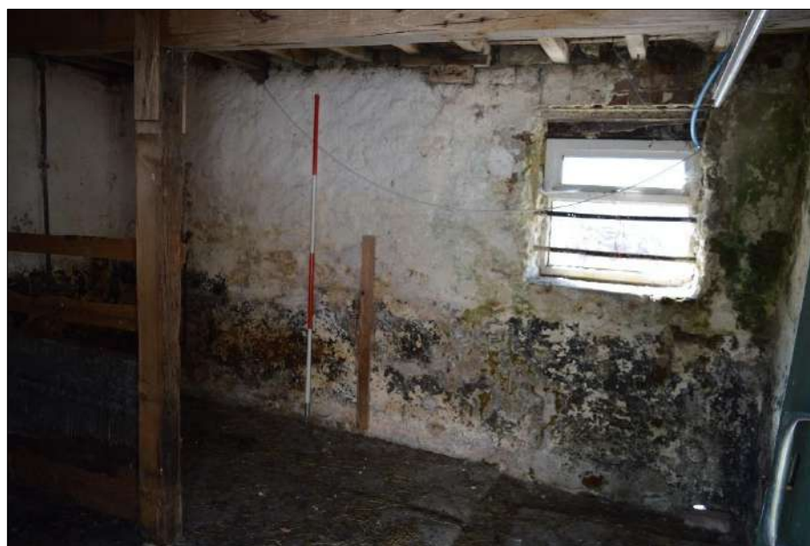
Plate 127 (shot 138): Southeastern wall of Room 7, 2m scale
