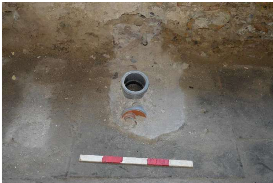
Plate 48 (shot 74): Detail of pipework associated with modern bathroom fittings, Room 3, 0.5m scale
