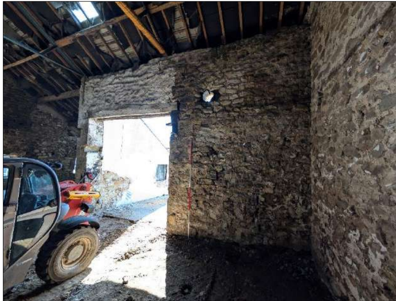
Plate 104 (shot 196): Southeastern wall of barn, Room 6, 2m scale
