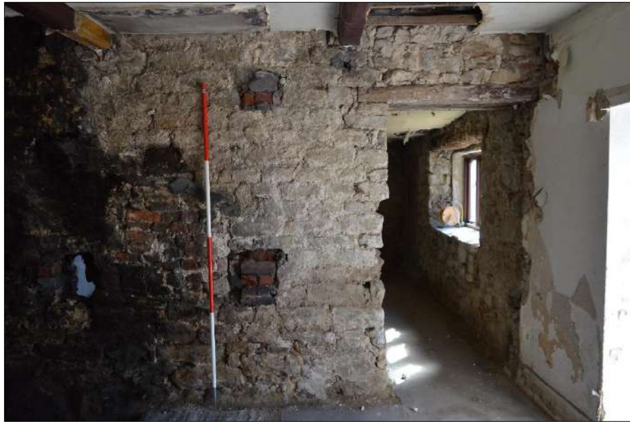
Plate 25 (shot 51): Detail of doorway in northeastern wall of Room 1, 2m scale
