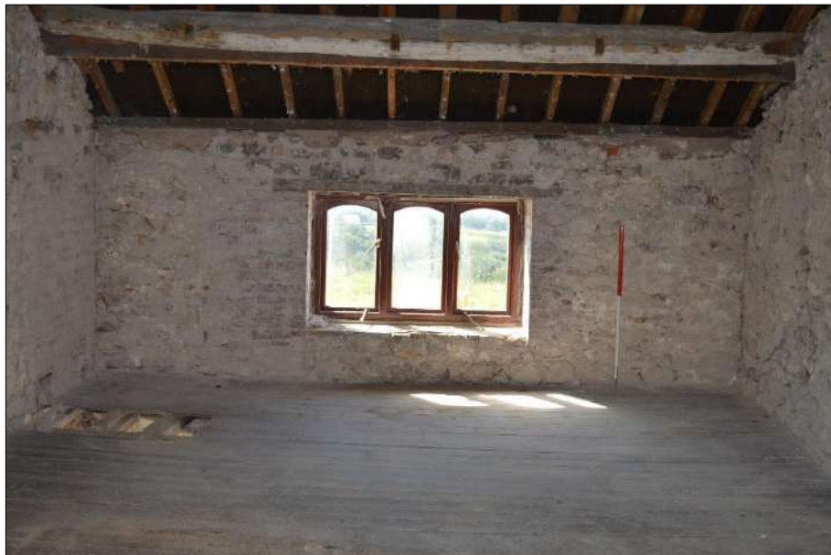
Plate 65 (shot 97): Southeastern wall of Room 5, 2m scale
