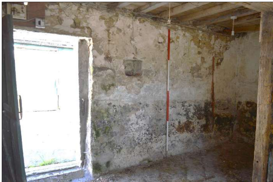
Plate 121 (shot 142): Northwestern wall of Room 7, 2m scale
