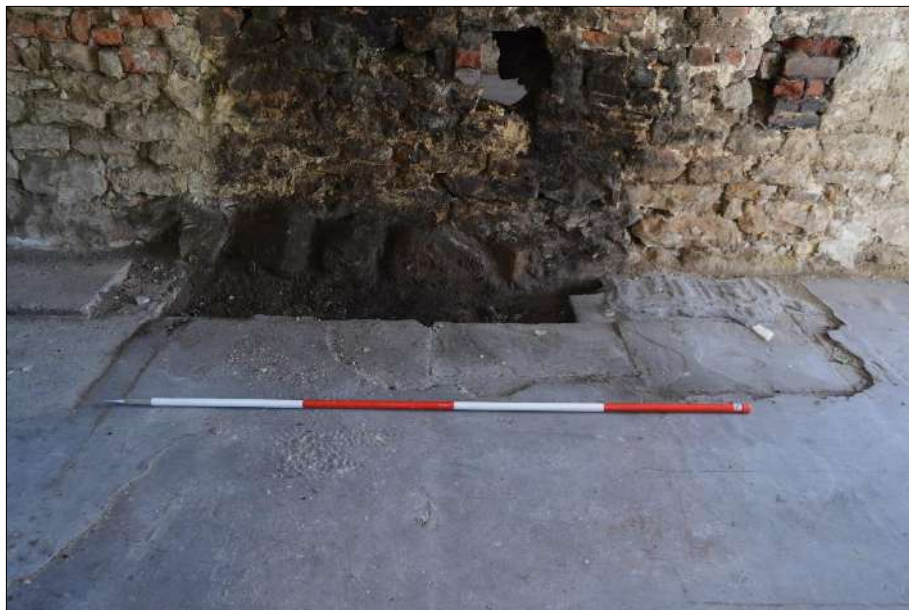
Plate 28 (shot 53): Base of demolished fireplace, 2m scale
