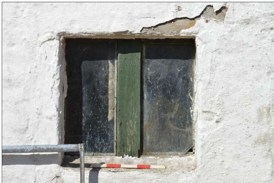
Plate 79 (shot 18): Detail of window in northeast elevation of barn, 0.5m scale
