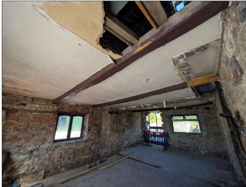
Plate 27 (shot 178): Interior of Room 1, looking northwest, showing extent of demolished fireplace on ceiling, no scale
