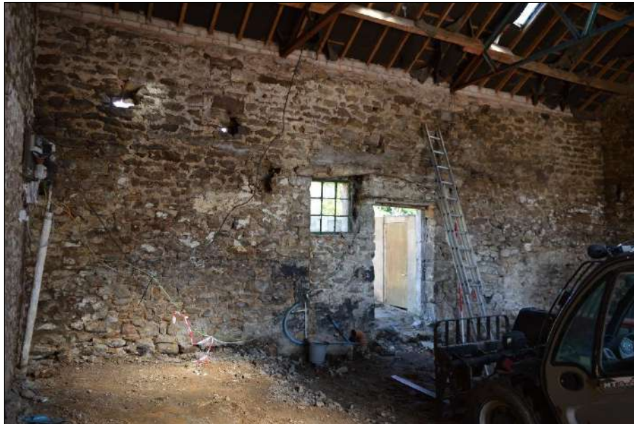
Plate 92 (shot 100): Northwestern wall of Room 6, 2m scale
