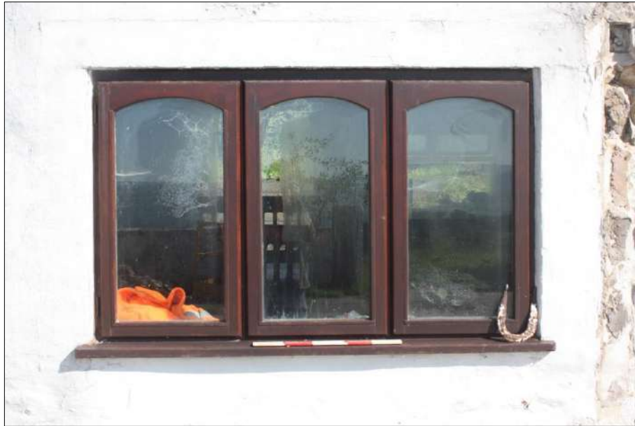
Plate 2 (shot 160): Detail of window, southeast elevation of farmhouse, looking northwest, 0.5m scale
