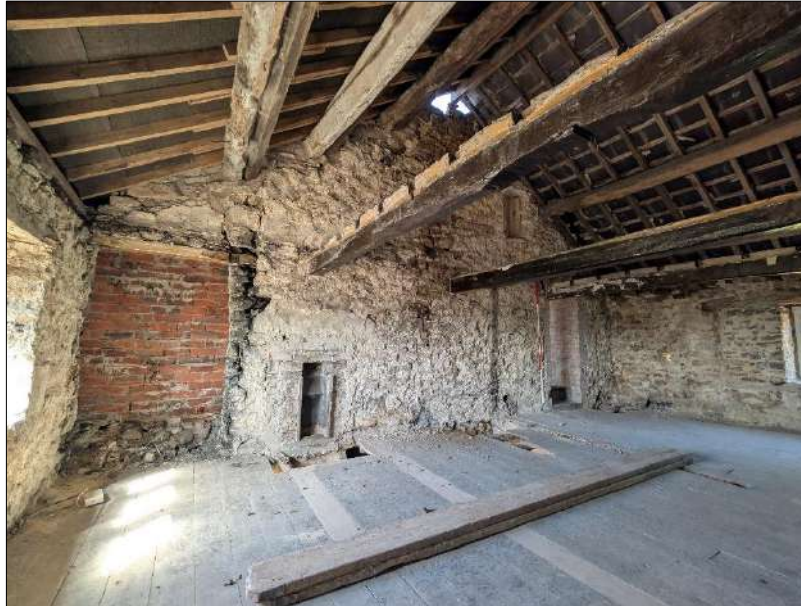
Plate 49 (shot 183): Interior of Room 4, looking northwest, 2m scale
