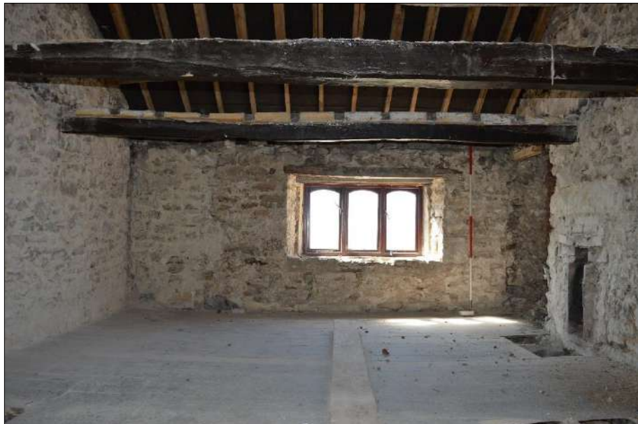
Plate 52 (shot 83): Southeastern wall of Room 4, 2m scale
