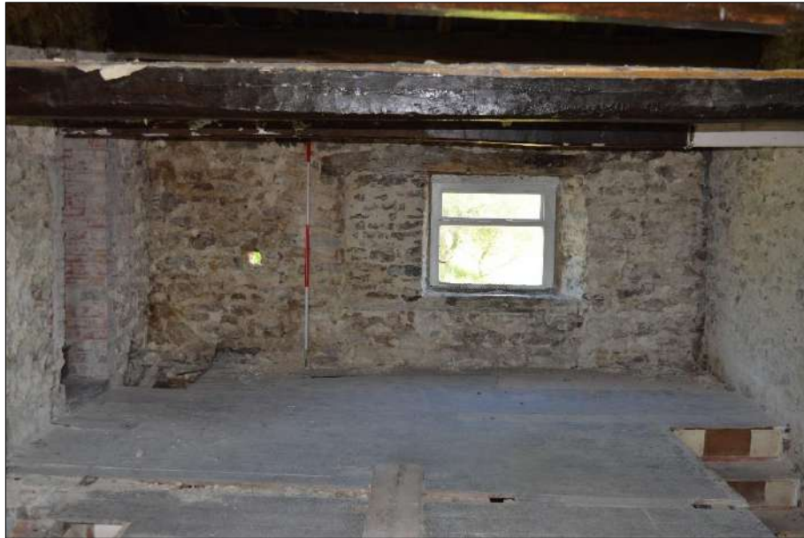
Plate 57 (shot 76): Northwestern wall of Room 4, 2m scale
