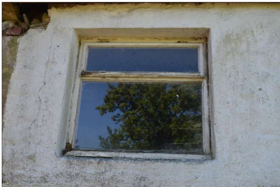
Plate 13 (shot 29): Detail of first floor window, northwest elevation of farmhouse, no scale
