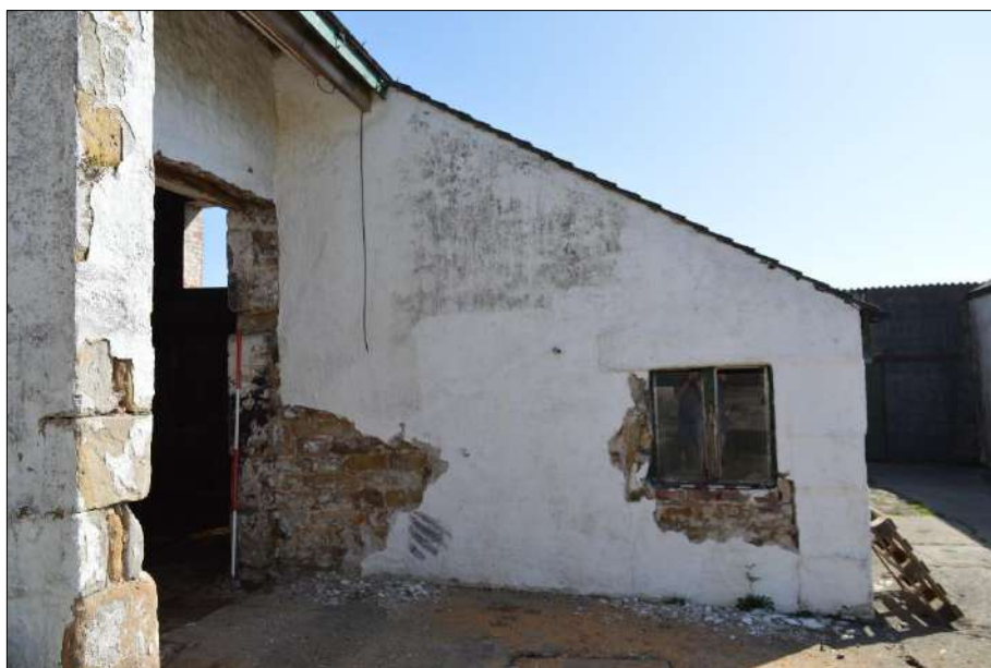
Plate 87 (shot 12): Southwest elevation of outshut, northeast end of main range, 2m scale
