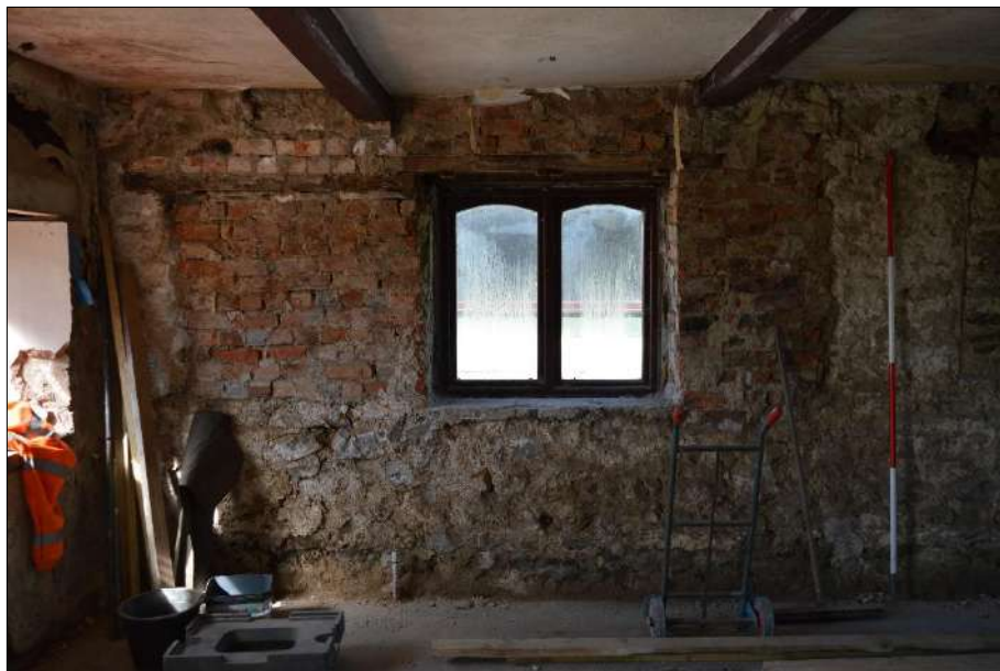
Plate 18 (shot 40): Southeastern part of southwestern wall, Room 1, 2m scale
