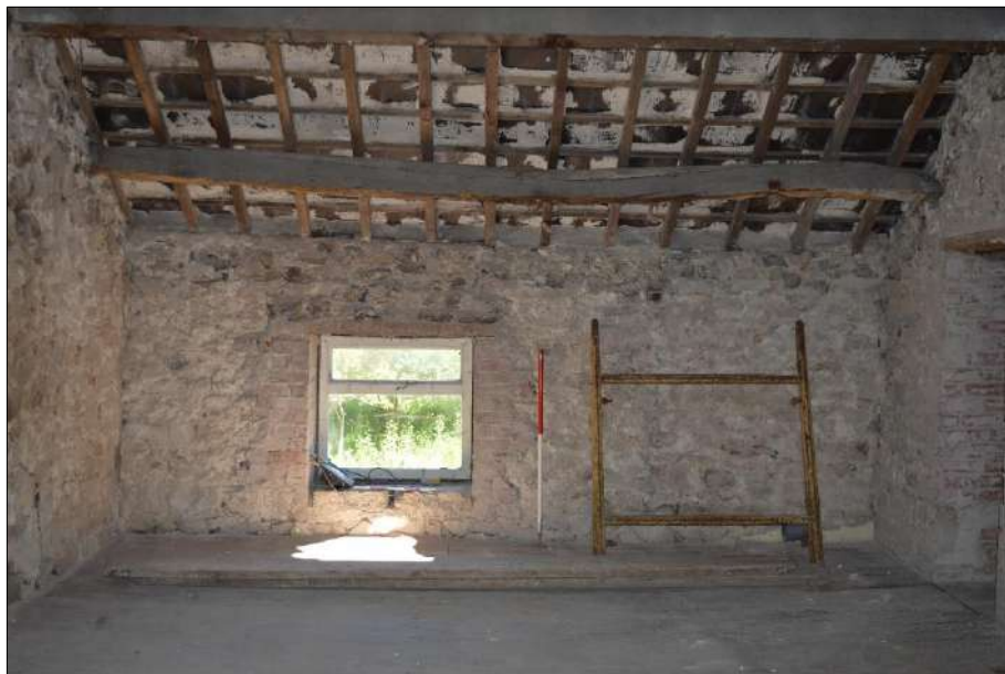
Plate 69 (shot 94): Northwestern wall of Room 5, 1m and 0.5m scales
