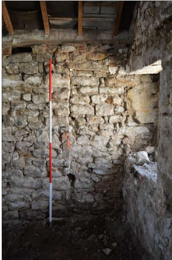
Plate 102 (shot 114): Detail of blocked doorway in southeastern wall of outshut, Room 6, 2m scale
