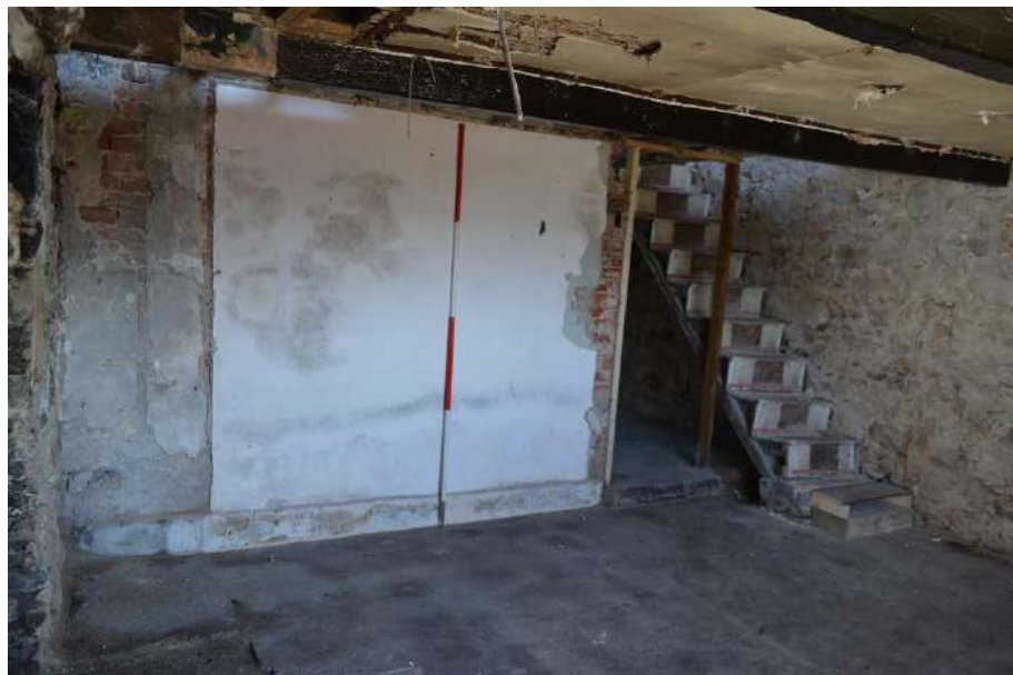
Plate 37 (shot 65): Northwestern wall of Room 2, 2m scale
