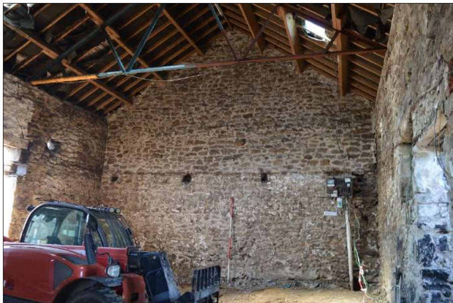
Plate 91 (shot 106): Southwestern wall of Room 6, 2m scale
